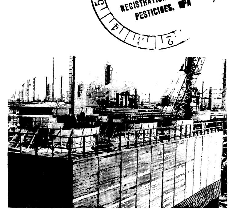
Microscopic organisms breed rapidly in open recirculating water systems and impair the efficient operation of cooling towers. Sunlight, warm water, oxygen and nutrients of air-borne or process origin can stimulate prolific growth of algae, mold, diatoms or bacteria in the absence of a suitable microbiocide.
