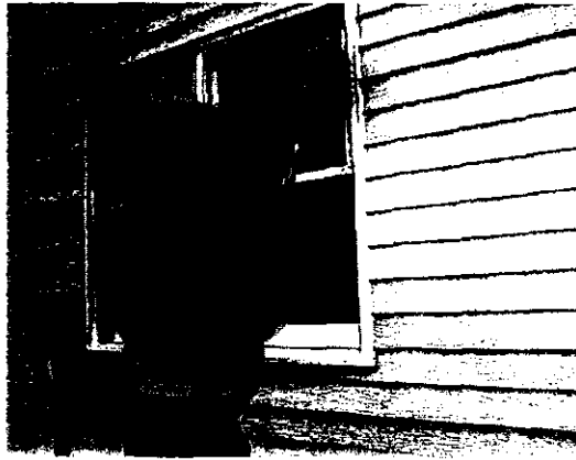
Apply around window and door frames
