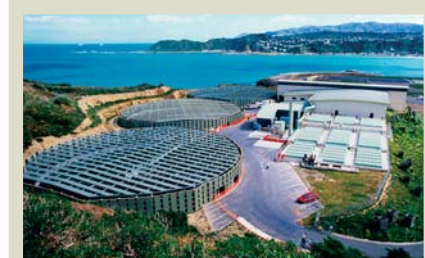
Clearwater at Moa Point Treatment Plant. Photo courtesy of Neil Price, Wellington City Council.
