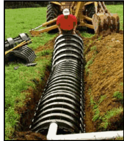
FIGURE 1 LEACHING CHAMBER
