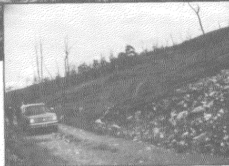
Above, truck spraying biosolids/fly ash mixture for revegetation at the Palmerton, Pennsylvania, hazardous waste site. Right, the same area after being reclaimed.
