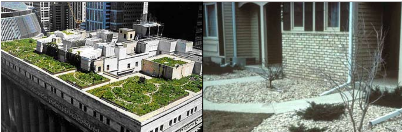
There are many innovative approaches to stormwater management that can be applied in urban and suburban areas. Chicago's City Hall (left) was retrofitted with a "green roof" to capture stormwater. Photo courtesy CDF Inc. The downspoutings on the house (right) drain onto a porous surface instead of onto a driveway. Photo by William Wenk.
