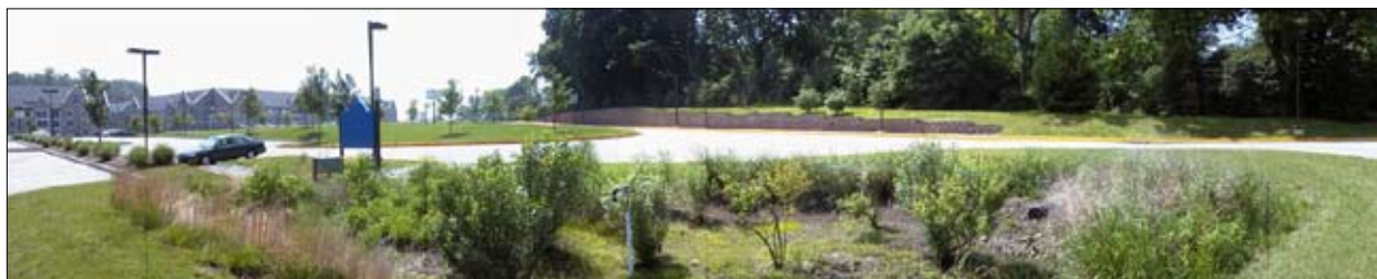
This traffic island on the Villanova University campus has a “bioinfiltration” system to capture water. Photo by Robert Traver.
