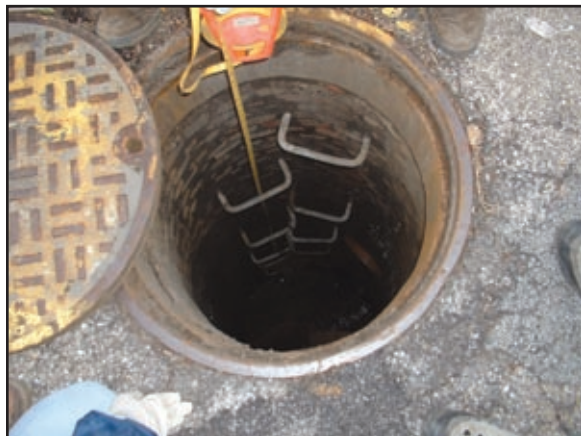
Figure 56: Techniques to sample from the storm drain
