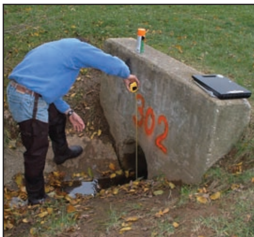
Figure 27: Measuring Outfall Diameter
