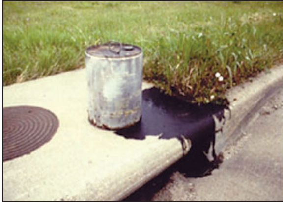
Figure 5: Dumping at a storm drain inlet
