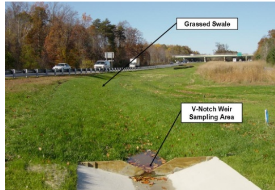
Grass Swale constructed in median on MD route 32 near Savage, MD. Courtesy of: James Stagge & Allen P. Davis, University of Maryland.
