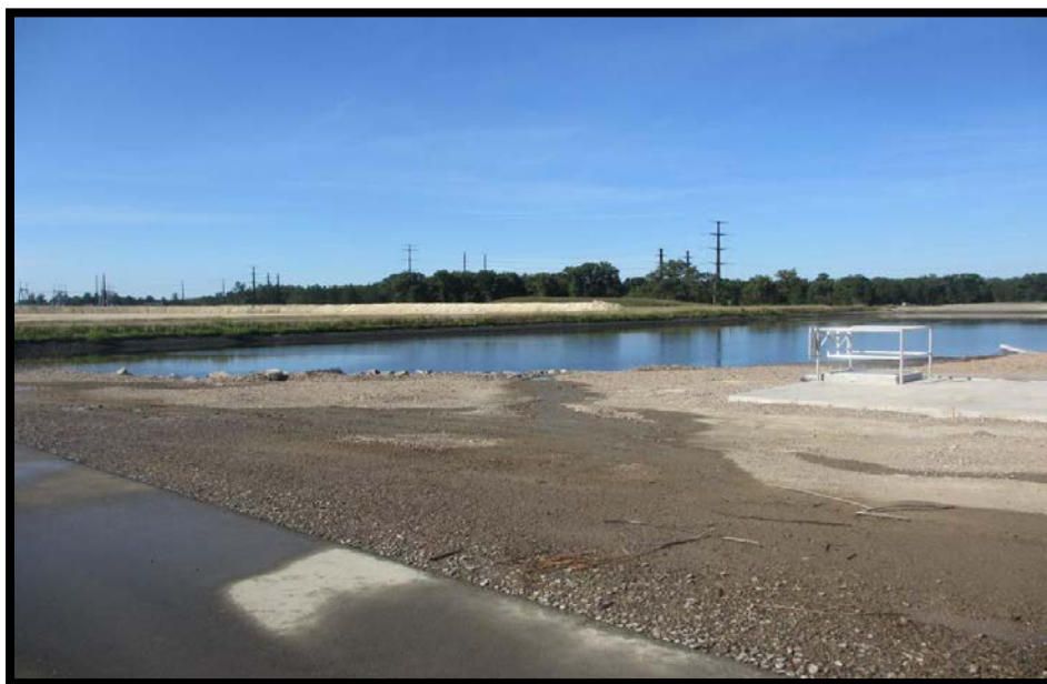
Photo 5.4.4a: Southeast Secondary Pond (water level ~4' deep)
