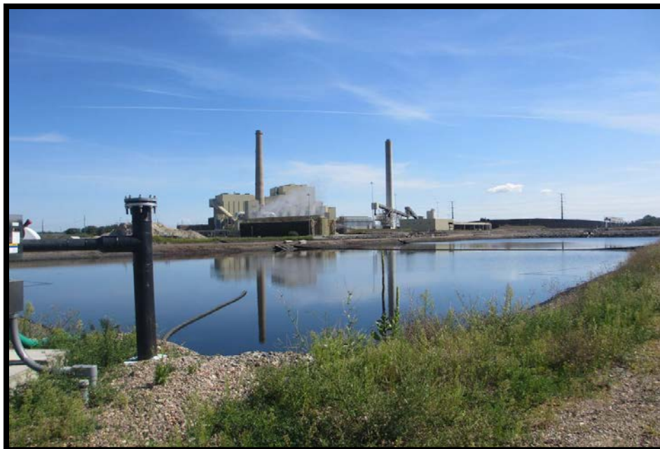
Photo 5.4.4b: Looking Northeast at Plant and Southeastern Secondary Pond
