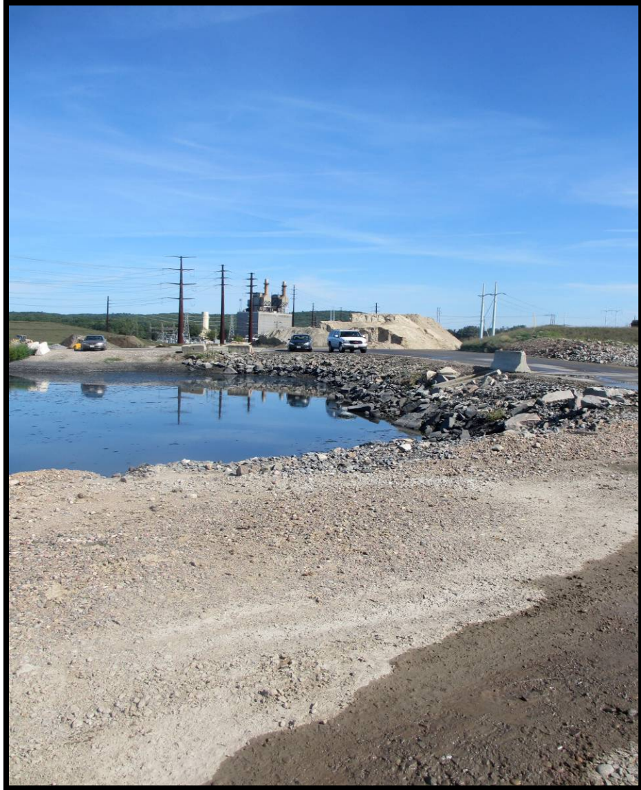
Photo 5.2.4c: Looking Northeast from berm between Northeastern and Southeastern Secondary Ponds
