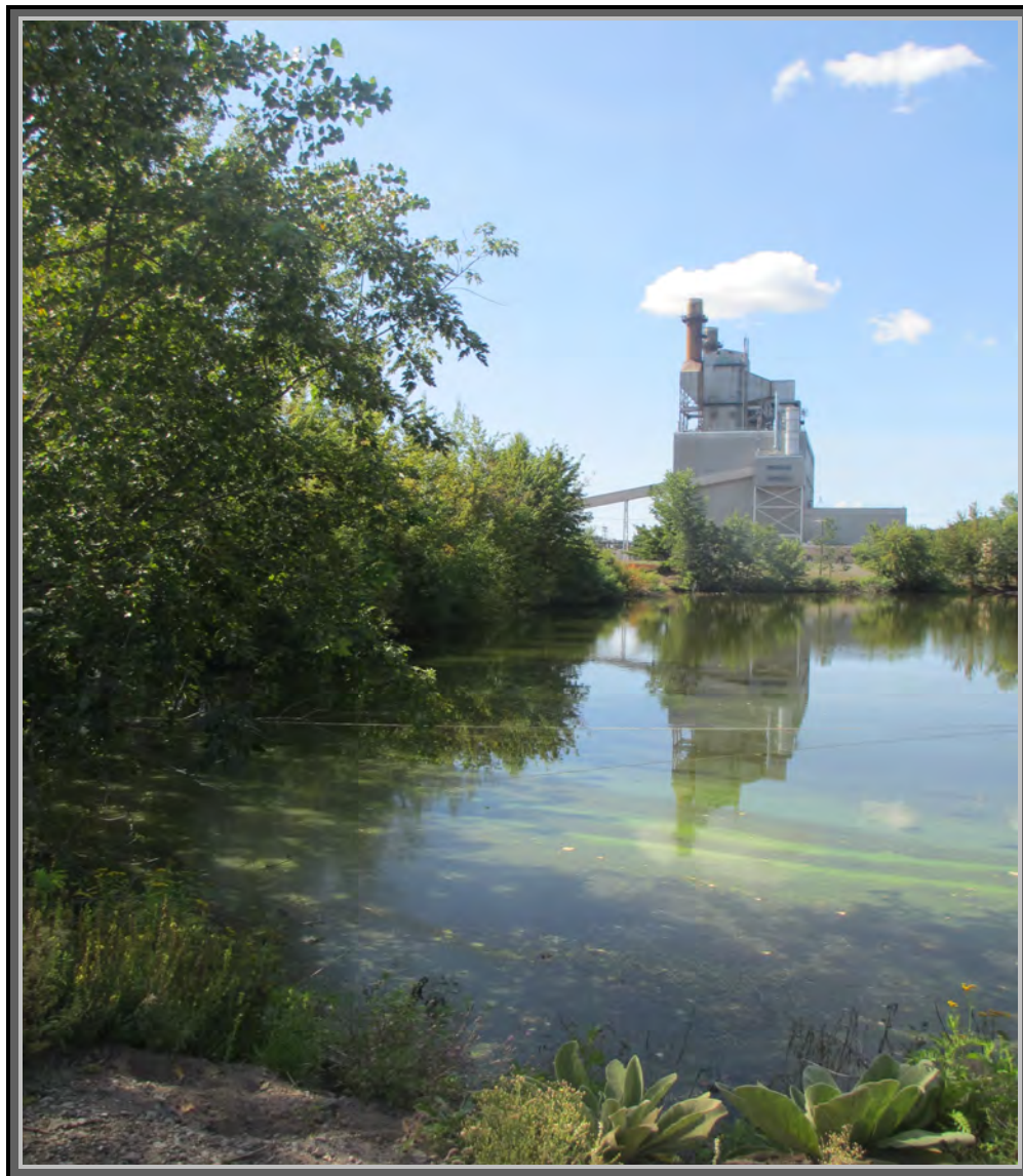
Photo 13. Looking S at Secondary incisions from berm between Secondary and Tertiary incisions _Weston Generating Station _082112
