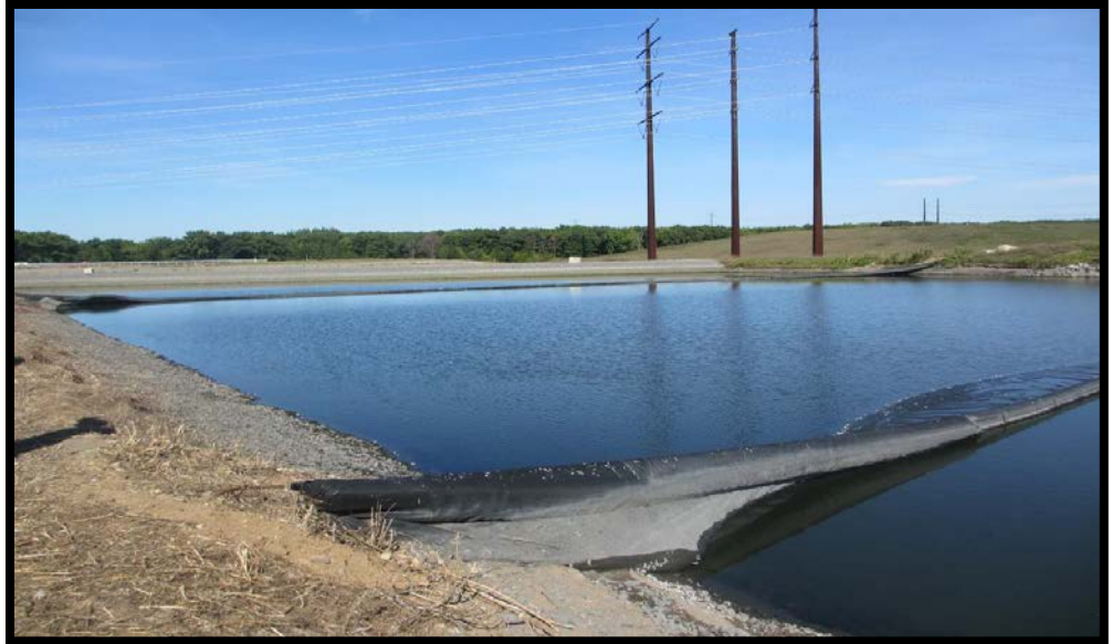
Photo 5.2.4d: Looking Northwest from midpoint of Northeastern Secondary Pond's Southern embankment (note silt curtain in foreground)
