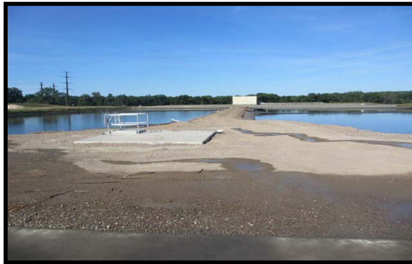
Photo 5.2.4a: Looking West at berm between Northern and Southern Secondary Ponds
