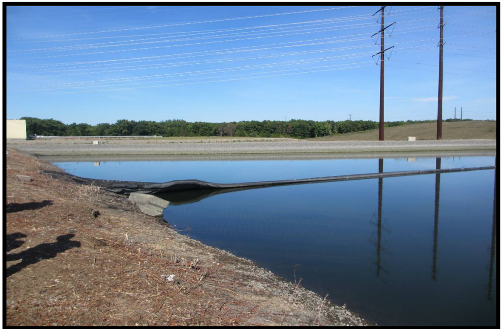
Photo 5.2.4e: Looking Northwest from midpoint of Northeastern Secondary Pond's Southern embankment (note silt curtain in foreground)
