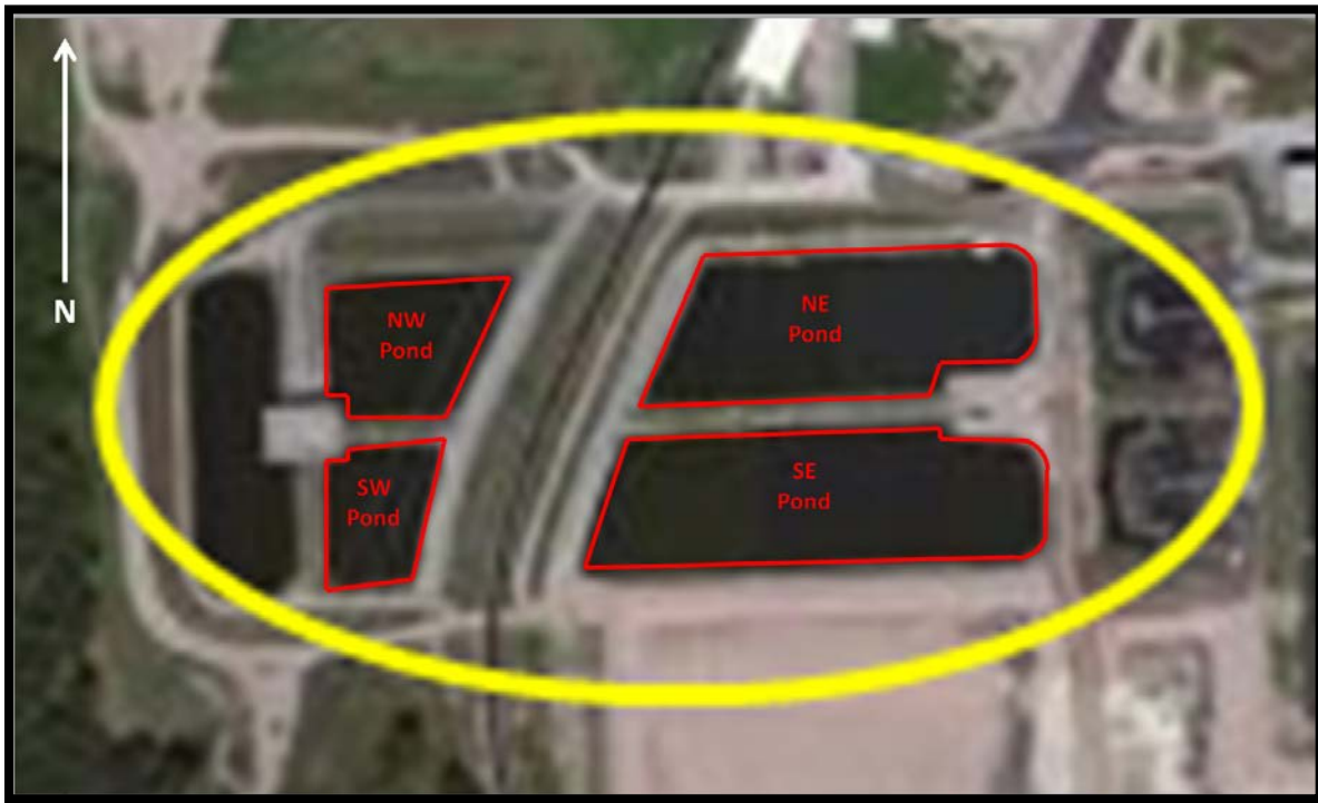
Figure 2.1d: Treatment Ponds at Weston Generating Station
