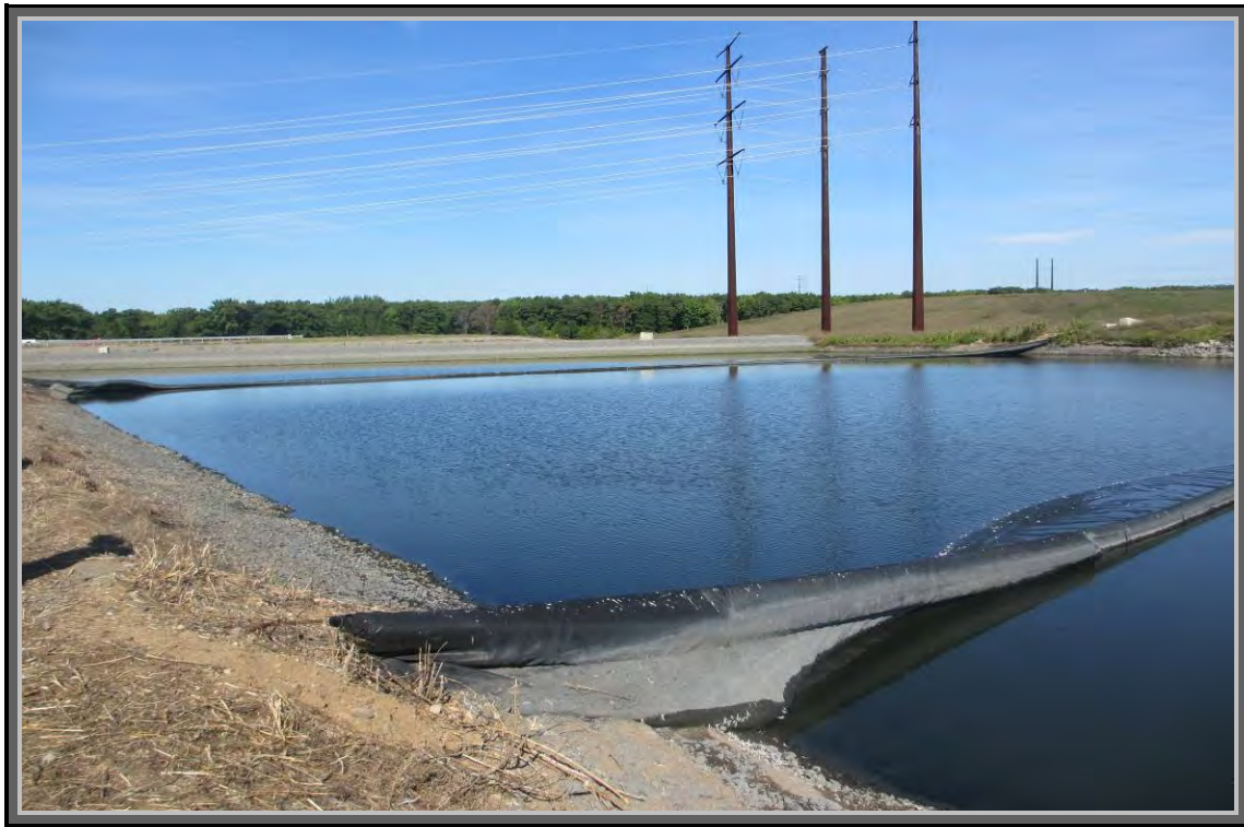
Photo 4. Looking NW from midpoint of NE Secondary Pond's S embankment (note silt curtain in foreground) _Weston Generating Station _082112
