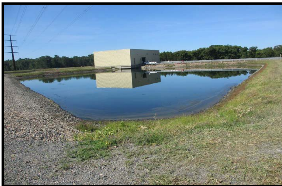
Photo 5.3.4a: Looking Southwest from Northeast corner of Northwest Secondary Pond; Treatment center at Southwest corner of Northwest Secondary Pond
