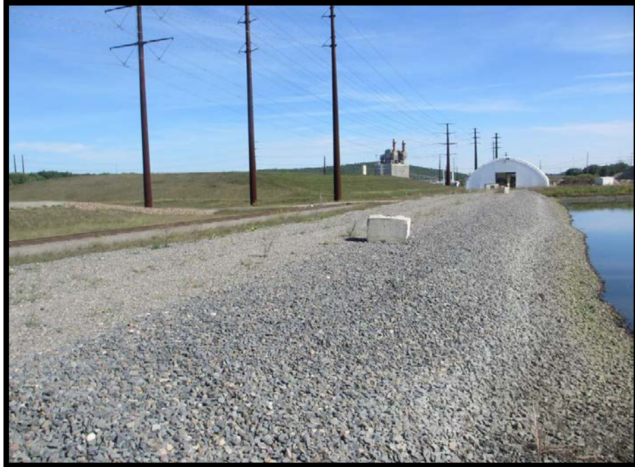
Photo 5.2.4f: Crest on West berm of Northeastern Secondary Pond
