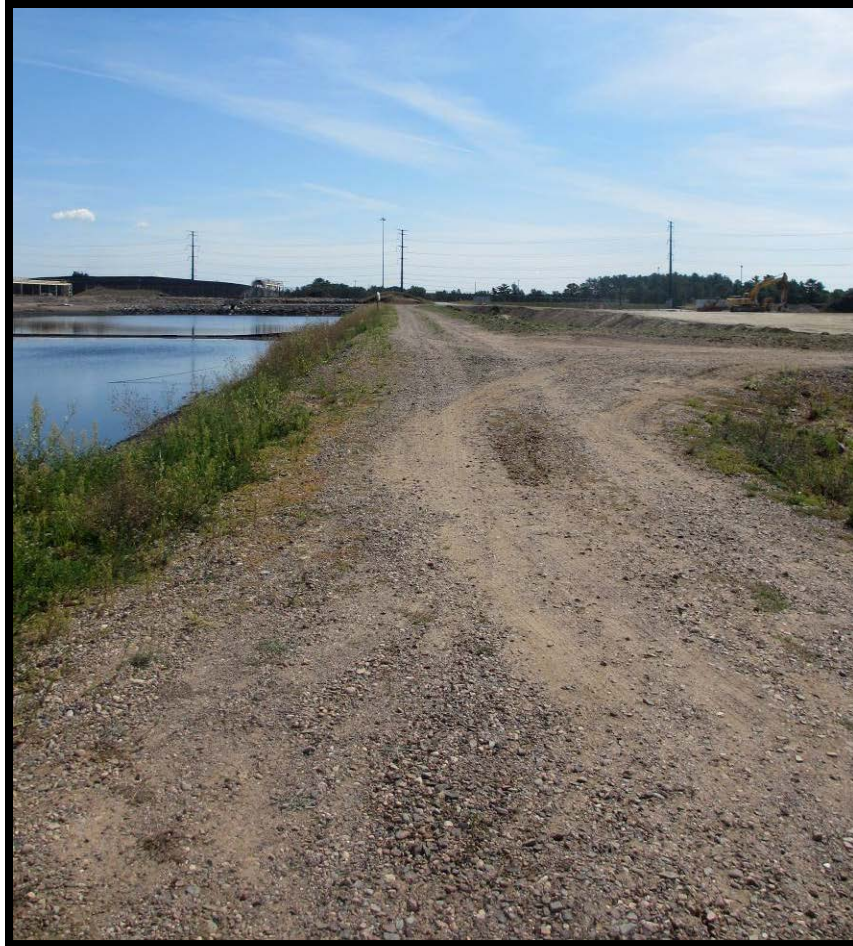
Photo 5.5.4b: Crest along Southwestern Secondary Pond's berm
