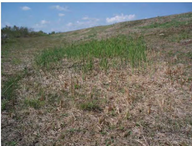
30. South Fly Ash Pond – Cattails growing on south embankment exterior face, looking west
