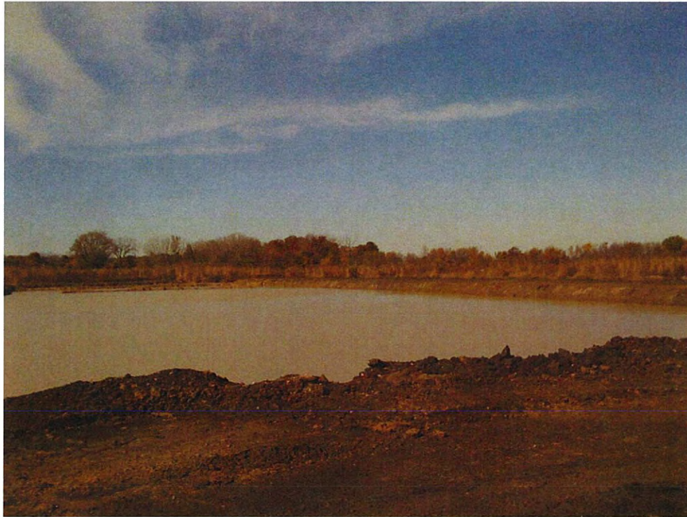
Photograph 1 – CCP storage facility (looking northwest)
