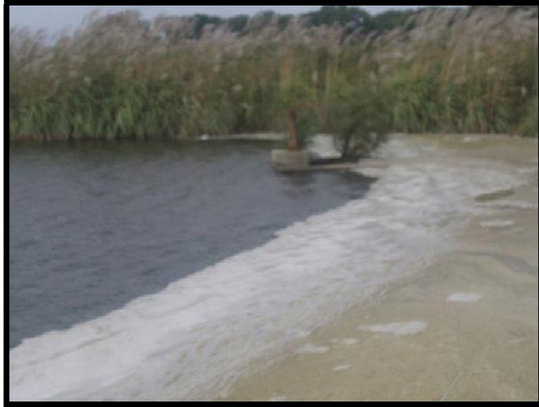
Figure 5.5.1-1: Overflow Outlet Structure.
