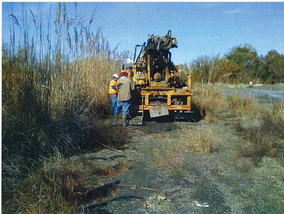
Photograph 8 – Drilling Borehole LEC-8 (looking north)
