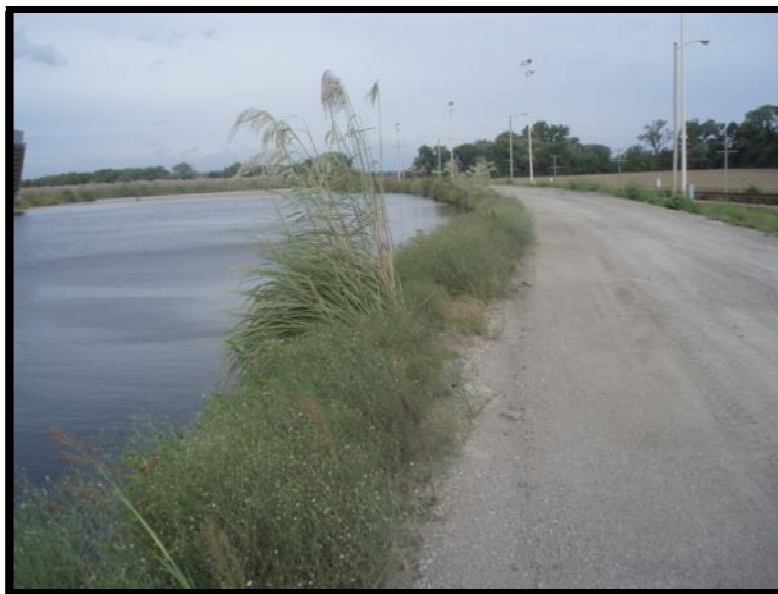
Figure 5.2.2-1: Inside Slope of the North Dike.
