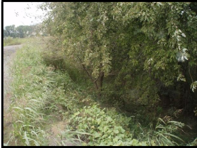
Figure 5.3.3-1: Typical Condition of Outside Slope of West Dike.
