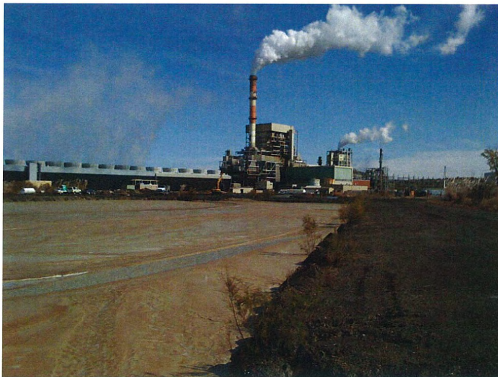
Photograph 2 – CCP storage facility (looking east)
