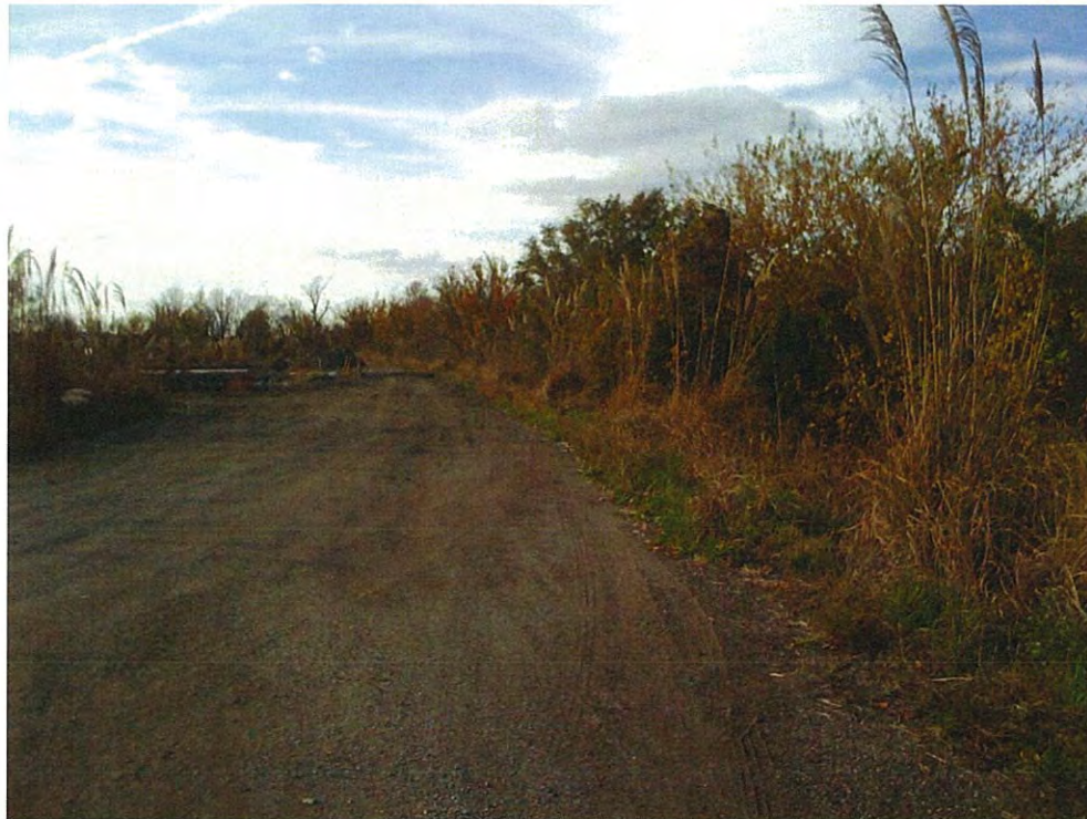
Photograph 5 – Berm crest (looking northwest)
