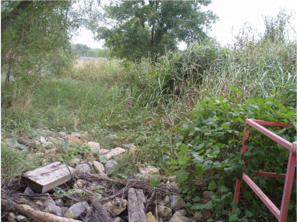
26. South dike – south side of storm water pond (Area 3).
