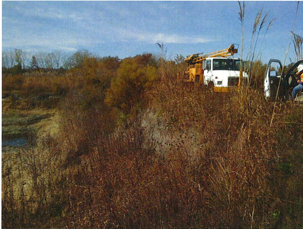
Photograph 5 – Drilling Borehole LEC-5 (looking west)
