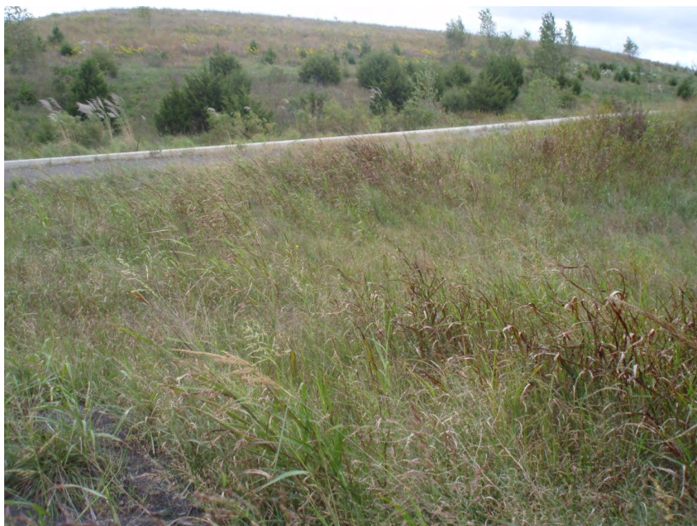
27. Exterior tie-in of south dike to existing grade/road embankment.
