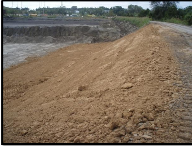
Figure 5.3.2-2: Inside Slope of West Dike (Area 3).
