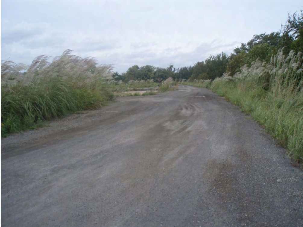
9. Top of northern dike – Taken from midpoint looking west.
