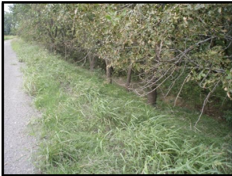
Figure 5.3.3-2: Trees on Outside of West Dike.
