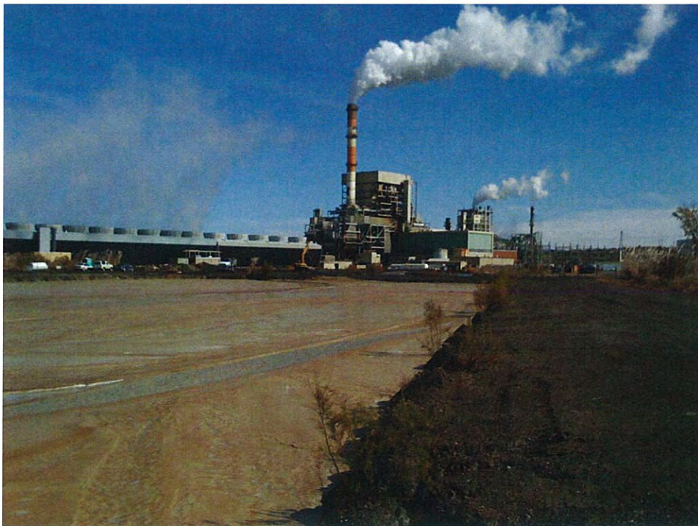
Photograph 2 – CCP storage facility (looking east)
