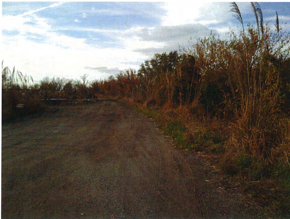
Photograph 4 – Berm crest near Borehole LEC-1 (looking northwest)
