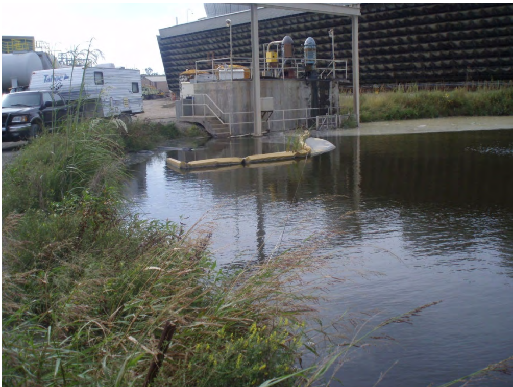
2. Discharge pipe at east end of Area 1
