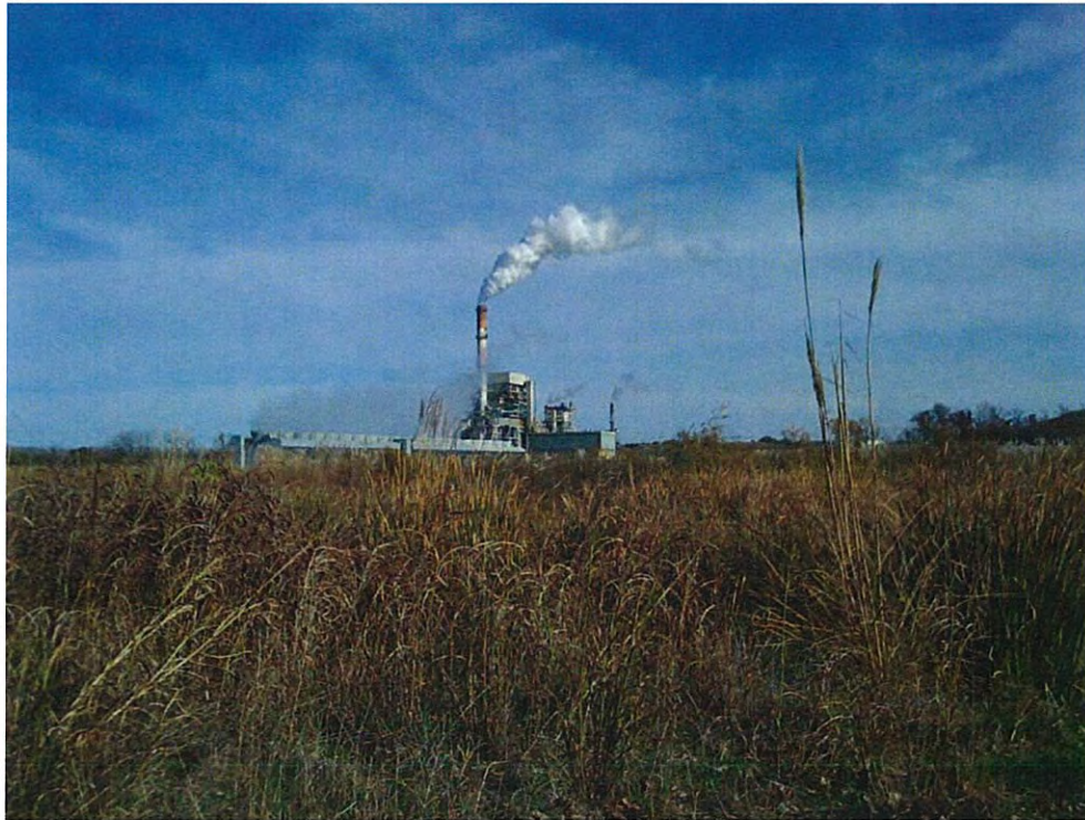
Photograph 3 – CCP storage facility (looking east)
