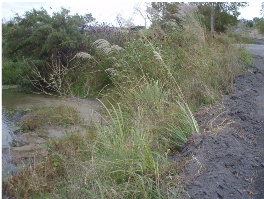
28. Interior tie-in of south dike to existing grade/road embankment.
