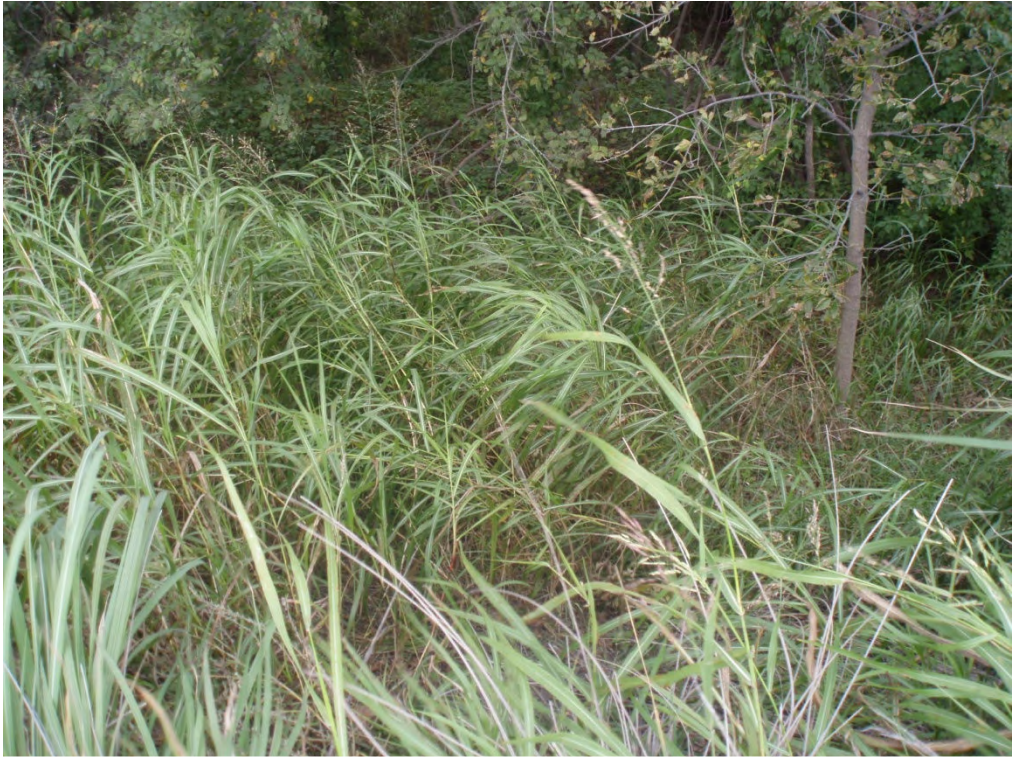
12. Exterior of northern dike (Area 4) – heavy vegetation observed.
