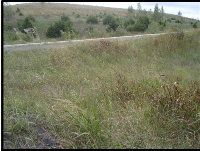
Figure 5.4.4-1: Tie-in of south dike to road embankment.
