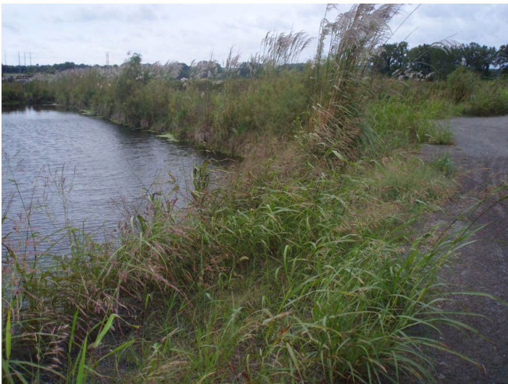
14. Interior of northwestern dike (Area 4)
