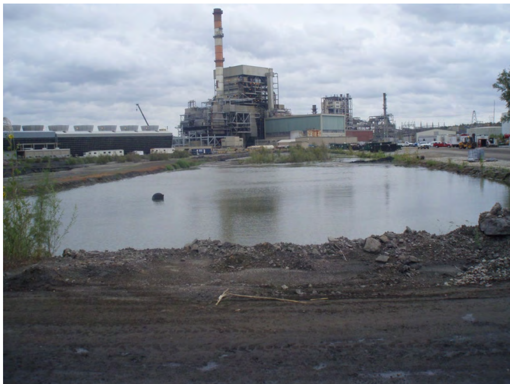
31. Area 2/south cell – Taken from southwest corner looking northeast.
