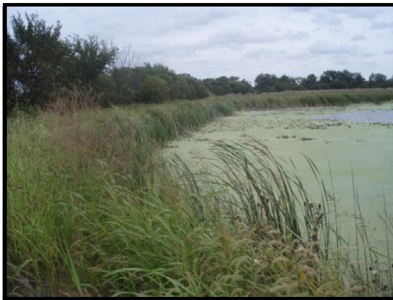
Figure 5.3.2-1: Inside Slope of Northwest Dike (Area 4).
