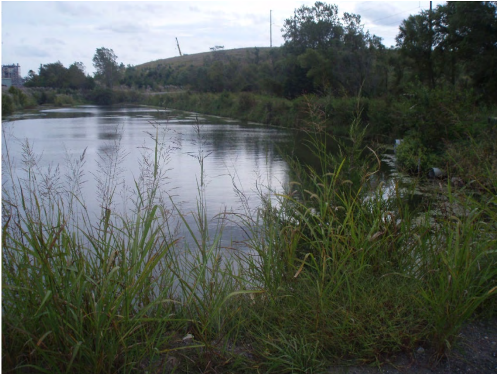
23. Storm water pond at south end of ash pond area/Area 3 – Taken from western dike looking east.
