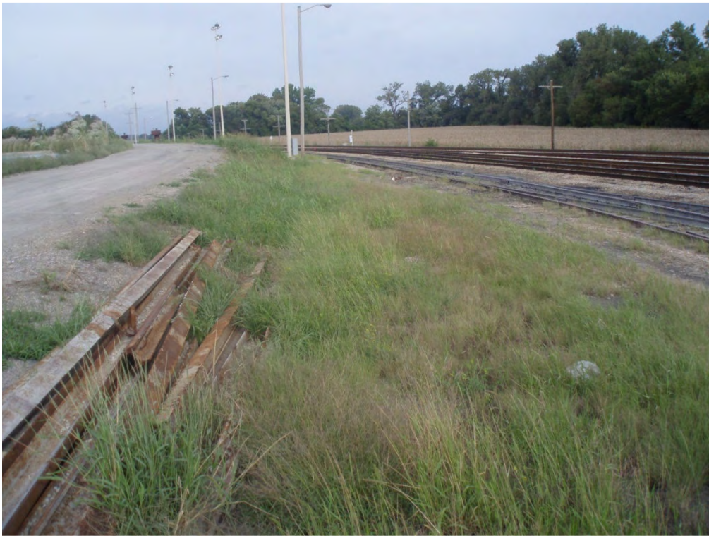
1. Exterior of north dike – Taken from east end of Area 1, looking west
