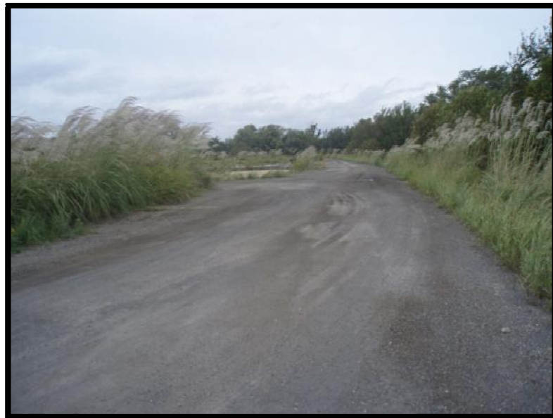
Figure 5.2.1-1: Crest of North Dike.
