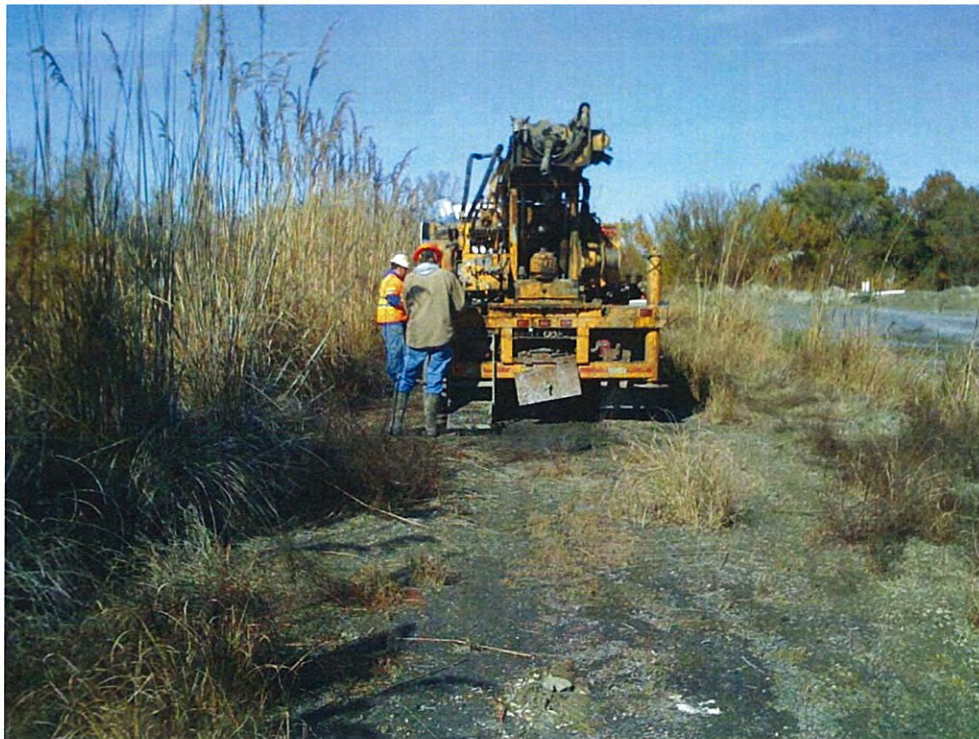
Photograph 4 – CME drill rig used to complete boreholes (looking north)
