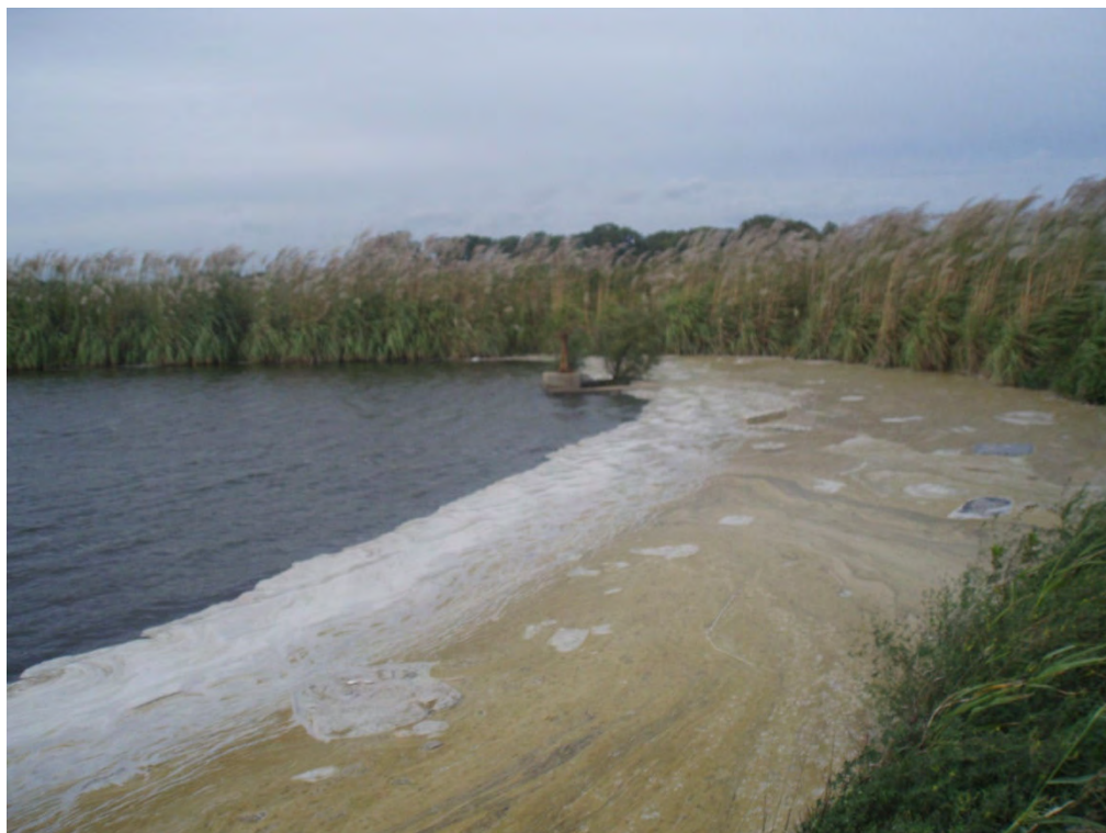
5. Emergency overflow structure – west end of Area 1
