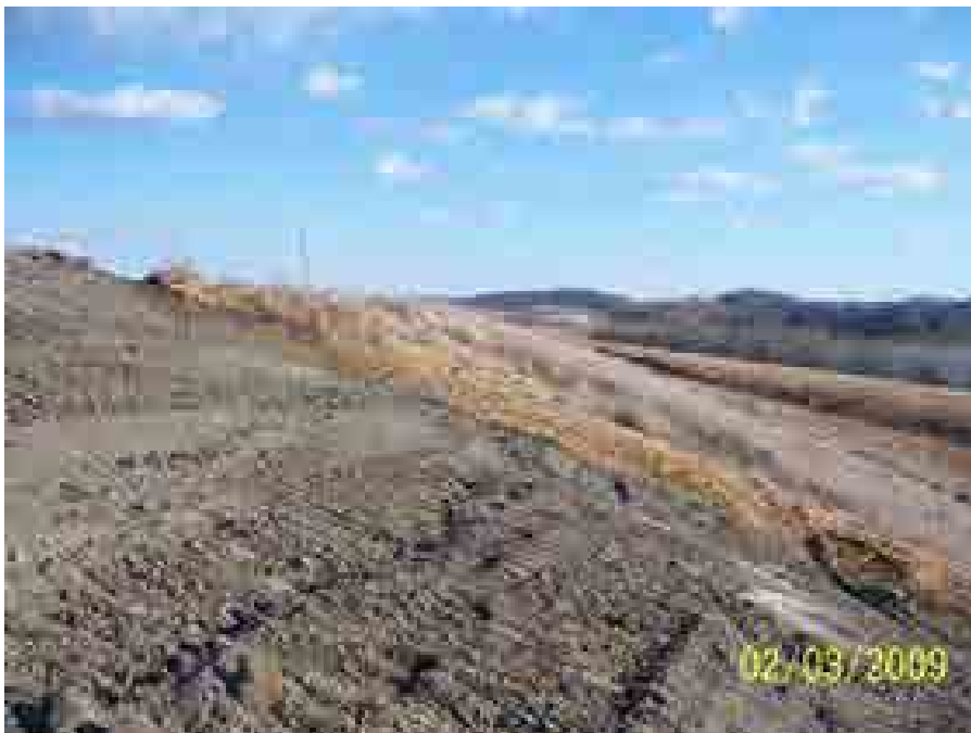
Drawing Mark DS-1-6 Uncompleted soil cover and vegetation along north end of Dry Ash Stack.
