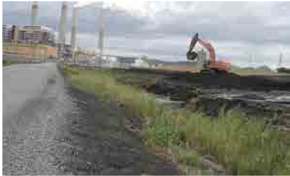
Figure 5.3.2-1 Photo showing inside slope, North Dike
