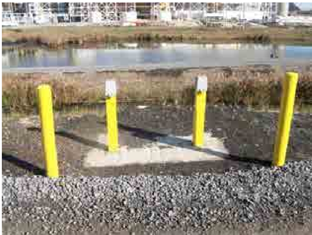
Figure 5. Typical Instrumentation (Slope Inclometers, Piezometers) Installation
