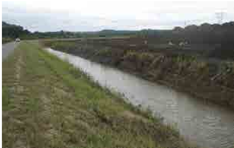
Figure 5.3.2-2 Photo showing inside slope, West Dike
