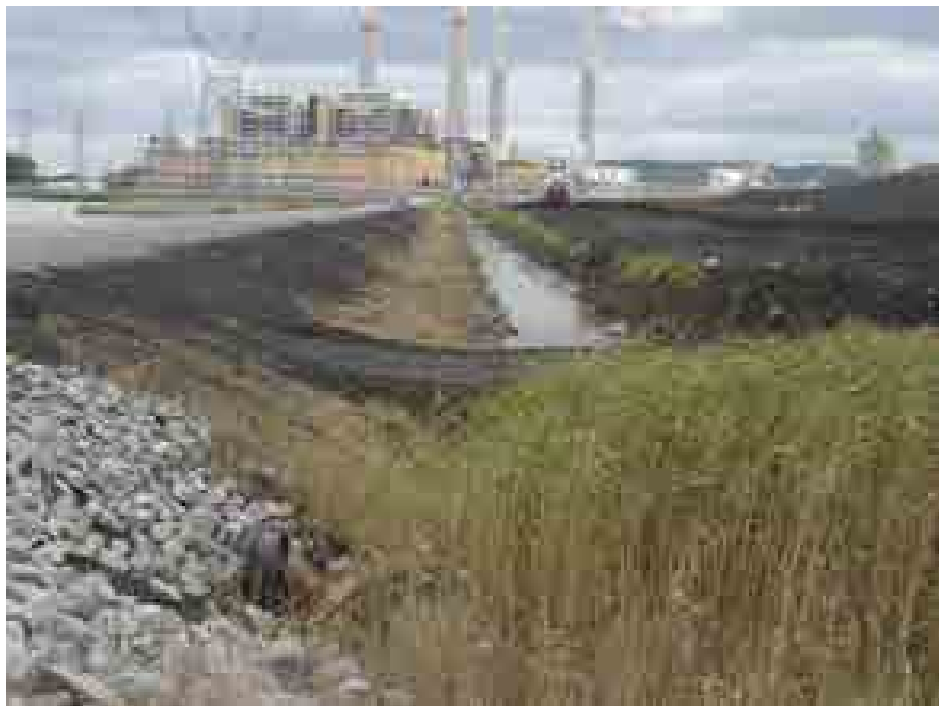
Figure 5.4.3-3 Photo showing outside slope, South Dike
