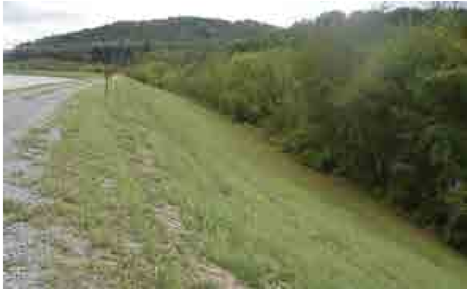
Figure 5.4.3-2 Photo showing outside slope, West Dike
