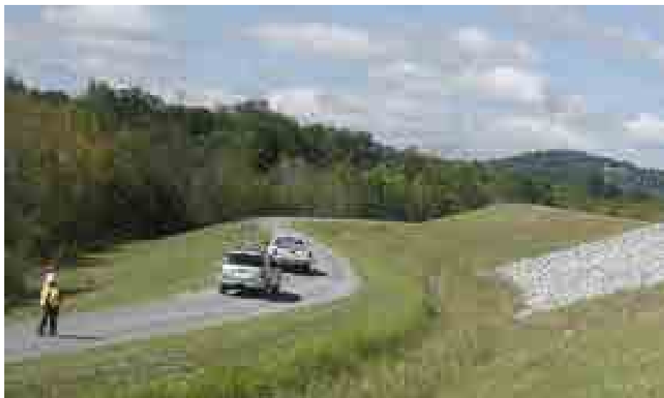
Figure 5.2.1-2 Photo showing Crest, South Dike
