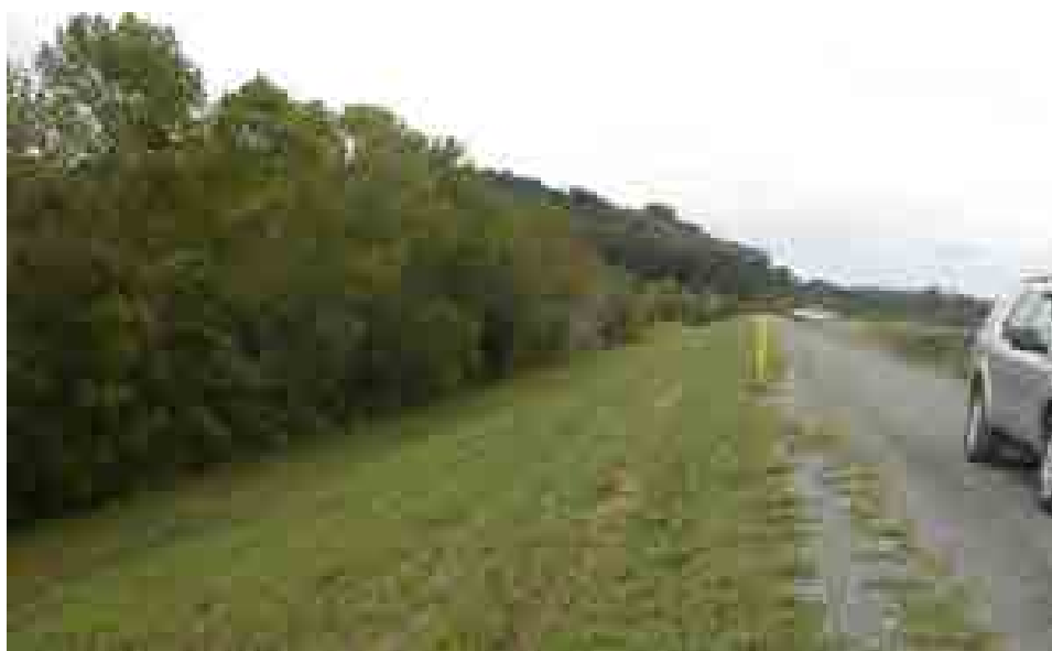
Figure 5.3.3-1 Photo showing outside slope, West Dike
