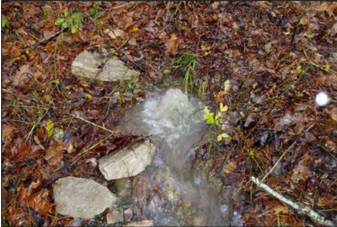
Figure 4. Example of Action Level 3 – Turbid Flowing – Seepage Boil
