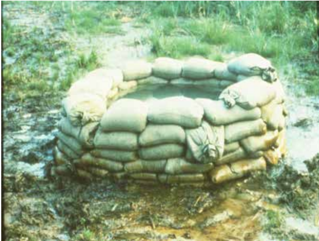
Figure 7. Sand Bag Treatment (Temporary)
