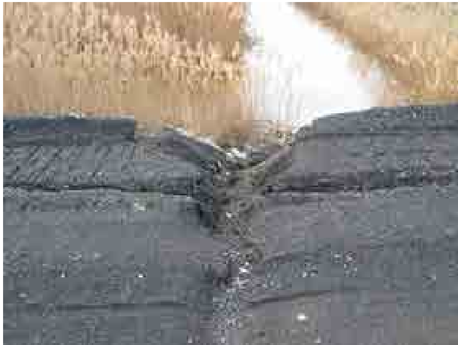
Drawing Mark AP-1-7 Erosion around 36" HDPE drain pipe along the west end of the divider dike.
