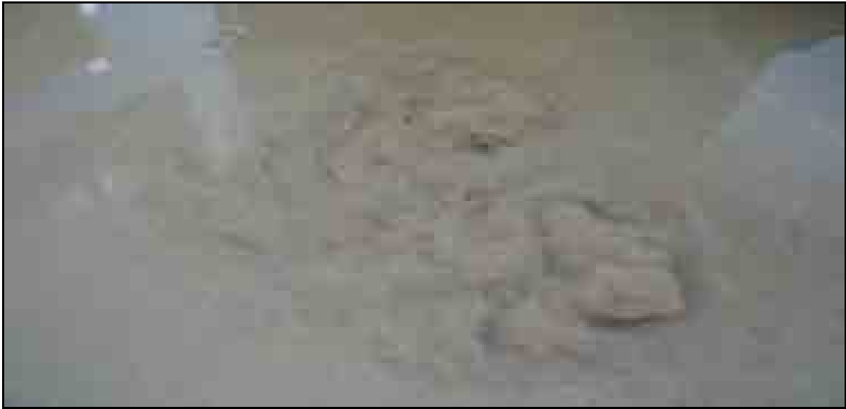
Figure 6. Example of Action Level 3 – Underwater Turbid Flowing – Seepage Boil
