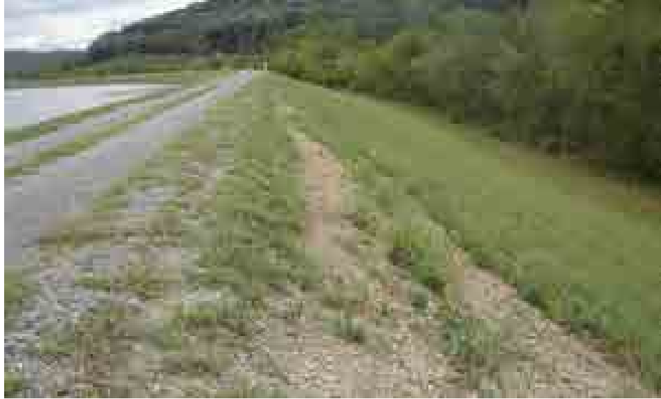
Figure 5.4.1-2 Photo showing crest, West Dike
