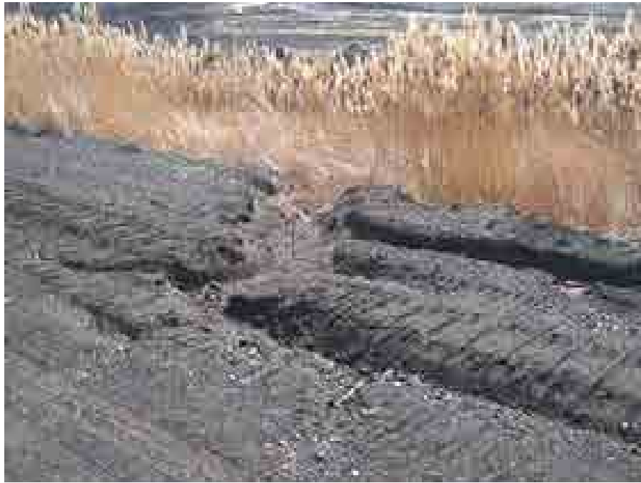
Drawing Mark AP-1-9 Erosion along divider dike between Dry Ash Stack and Ash Pond.
