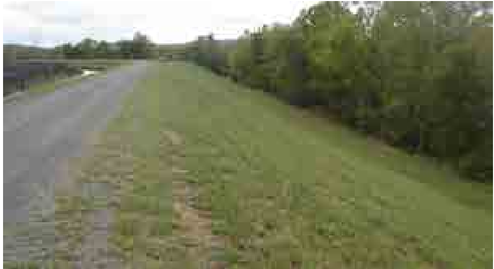
Figure 5.3.1-1 Photo showing crest, West Dike
