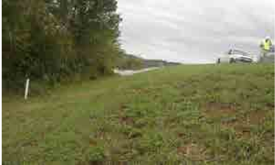
Figure 5.3.3-2 Photo showing outside slope, South/West Dike
