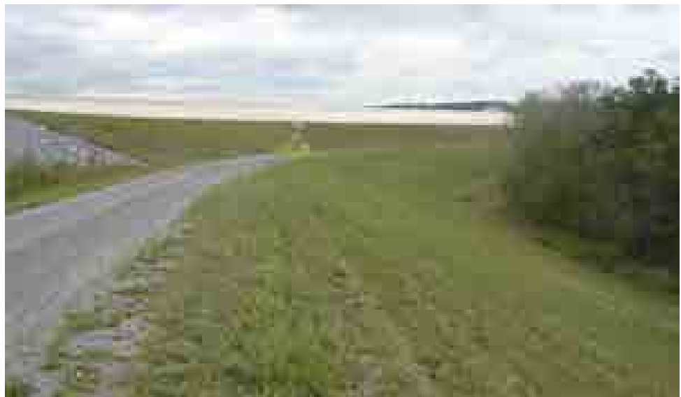
Figure 5.2.3-1 Photo showing outside slope, South Dike
