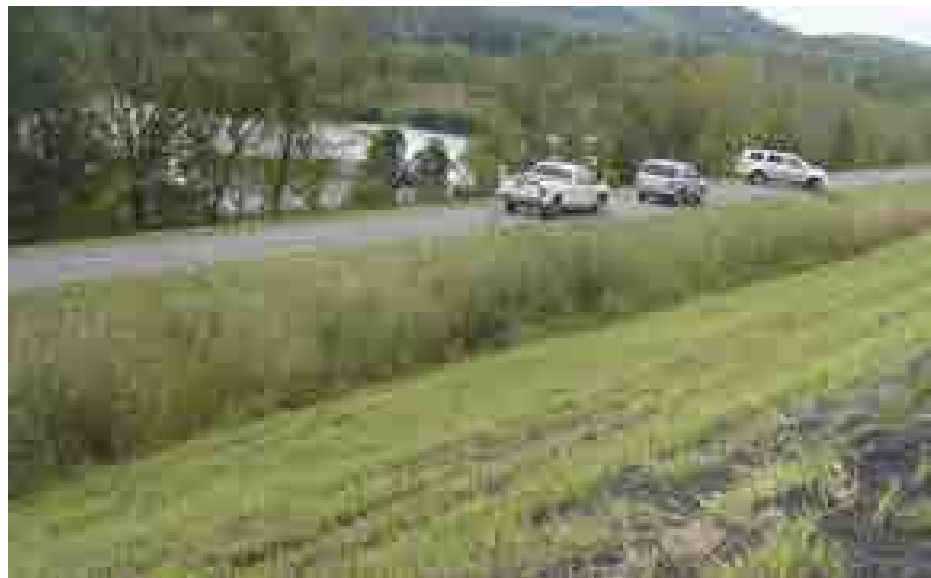
Figure 5.2.1-1 Photo showing Crest, East Dike
