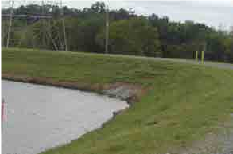
Figure 5.4.2-1 Photo showing inside slope, North Dike
