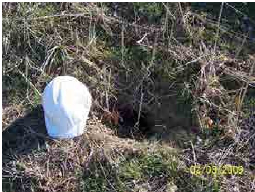
Drawing Mark AP-1-2 Animal burrow along north perimeter dike of Ash Pond.
