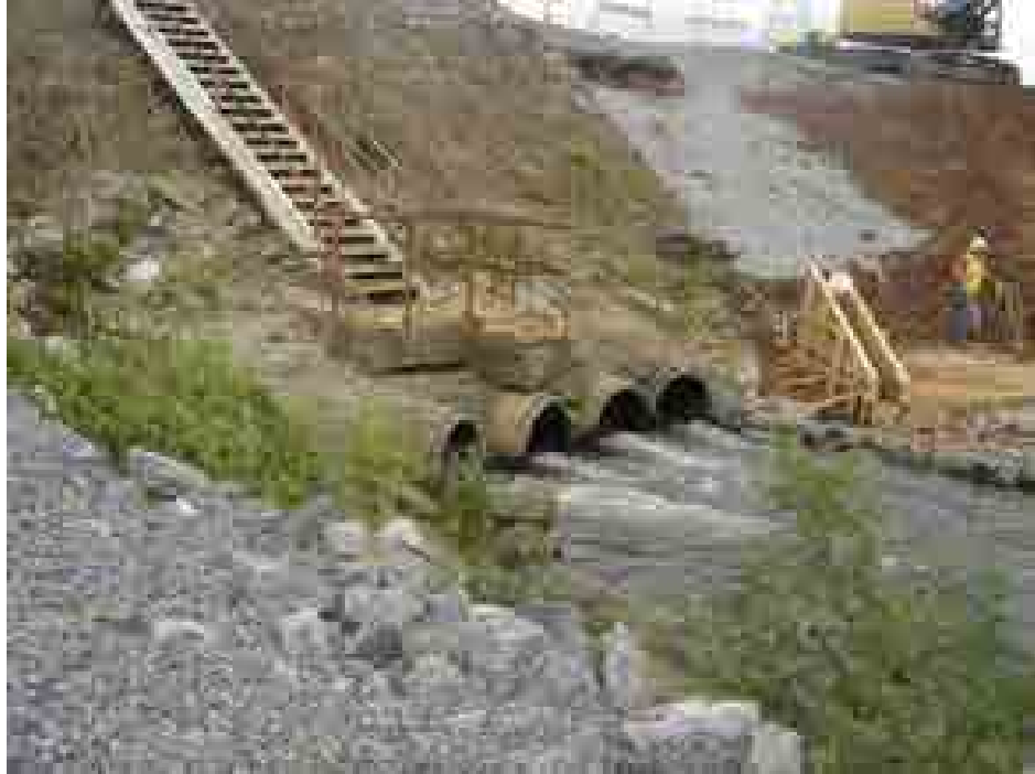
Figure 5.5.2 -1 Photo showing Outlet Conduits
