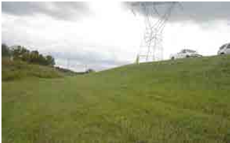
Figure 5.4.3-1 Photo showing outside slope, North Dike
