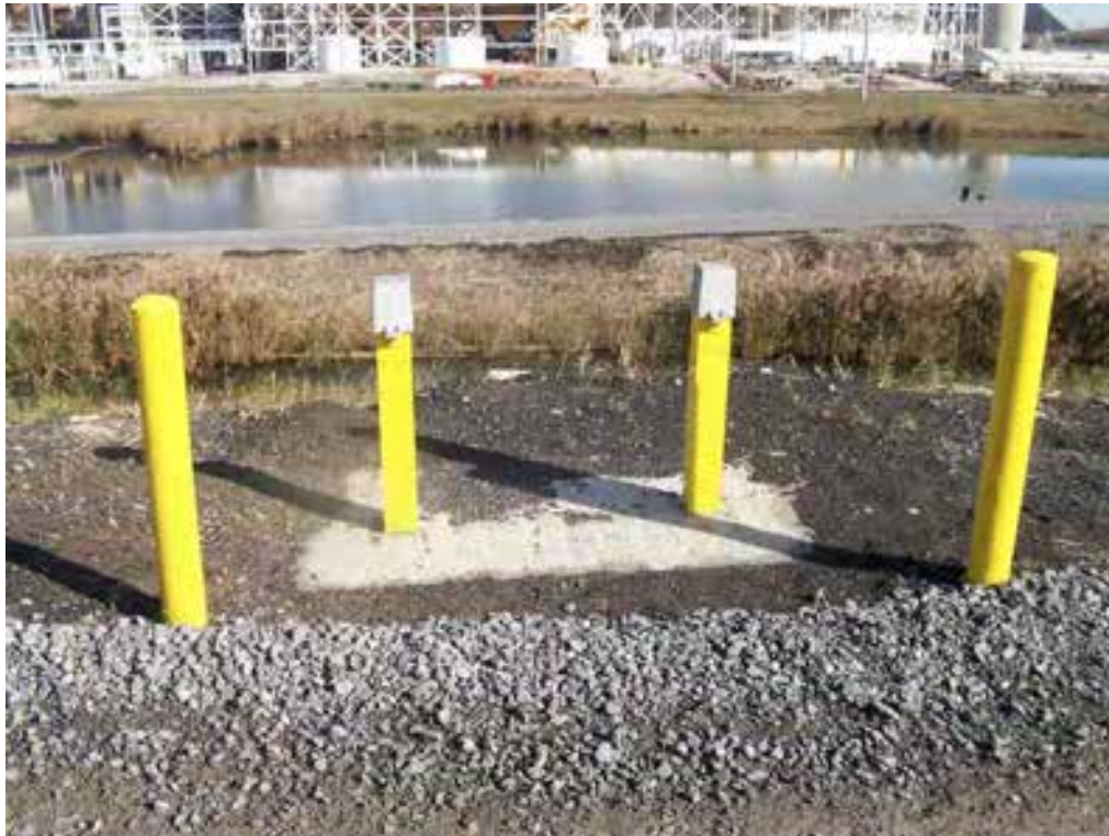
Figure 5. Typical Instrumentation (Slope Inclinometers, Piezometers) Installation
