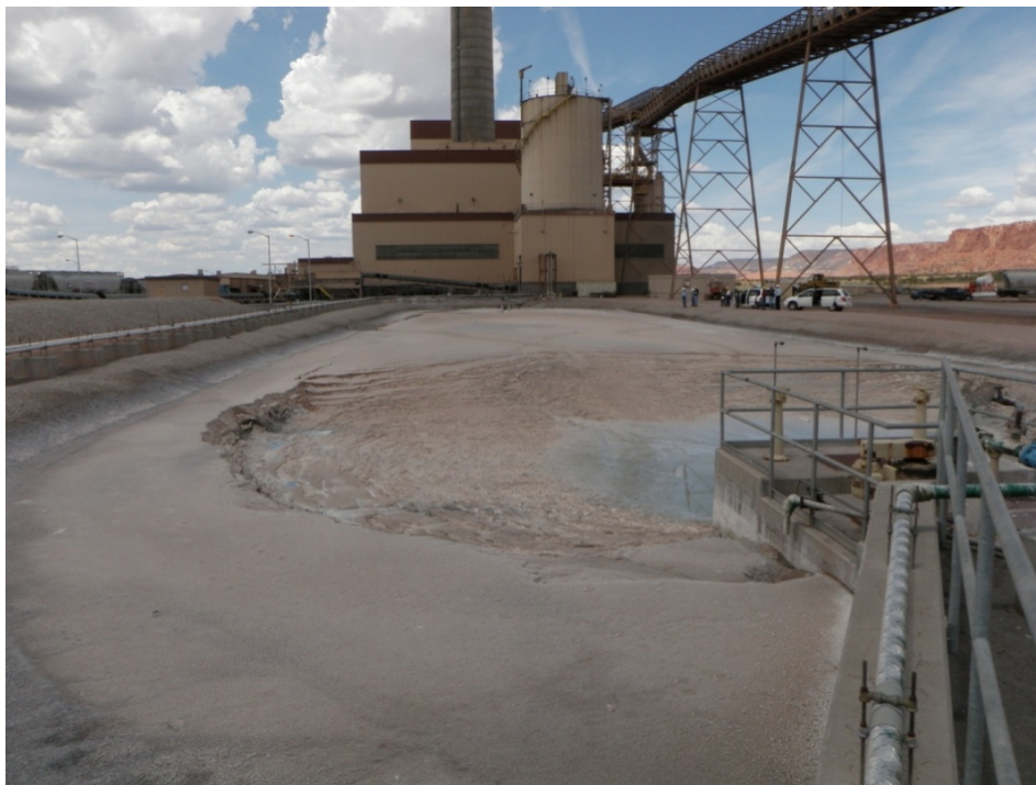
Photo 1: Emergency Scrubber Pond Looking West
