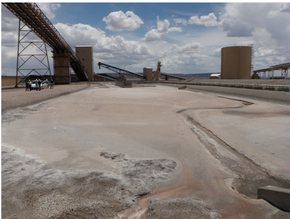
Photo 2: Emergency Scrubber Pond Looking East
