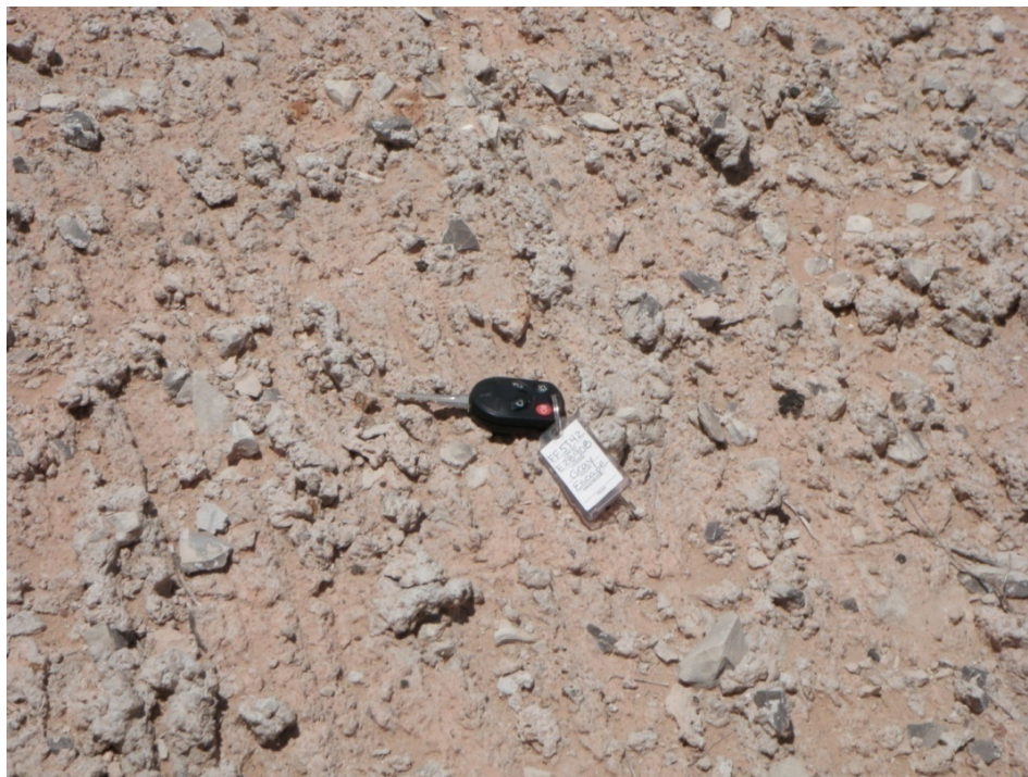
Photo 23: Evaporation Pond 5 : Raked liner finish
