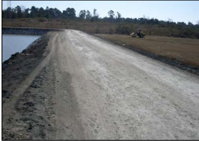
Photograph 5.8. Typical view of crest, southwest side looking southeast.
