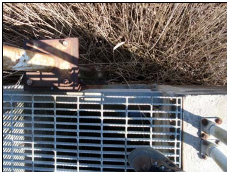
Photograph 5.11b. View (from above) down toward weir in emergency overflow structure.
