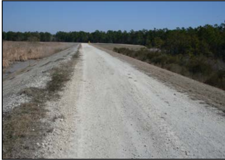
Photograph 5.1. View of crest and inside slope, southeast side looking northeast.
