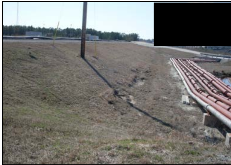
Photograph 5.5. View of outside slope and toe, northwest side looking southwest.
