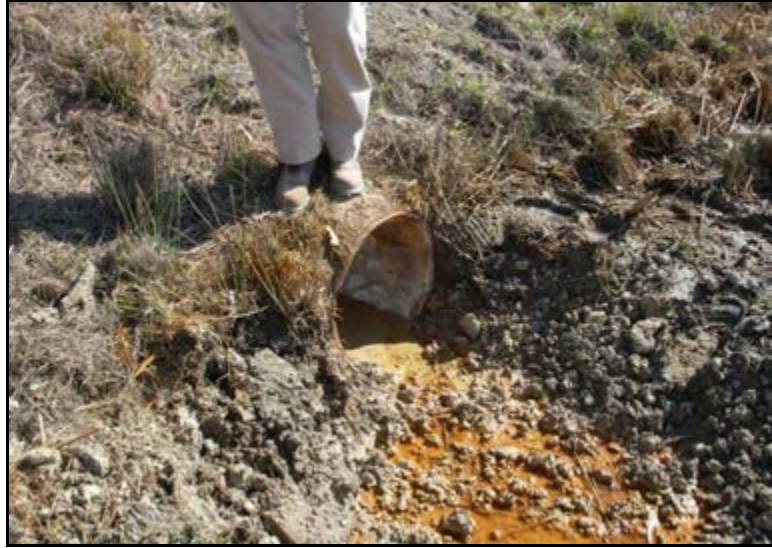
Photograph 5.16. Emergency outlet conduit.
