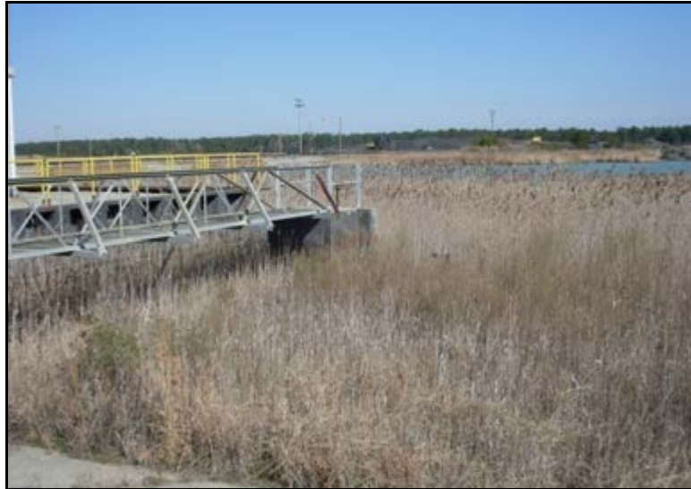
Photograph 5.11a. Emergency overflow structure.
