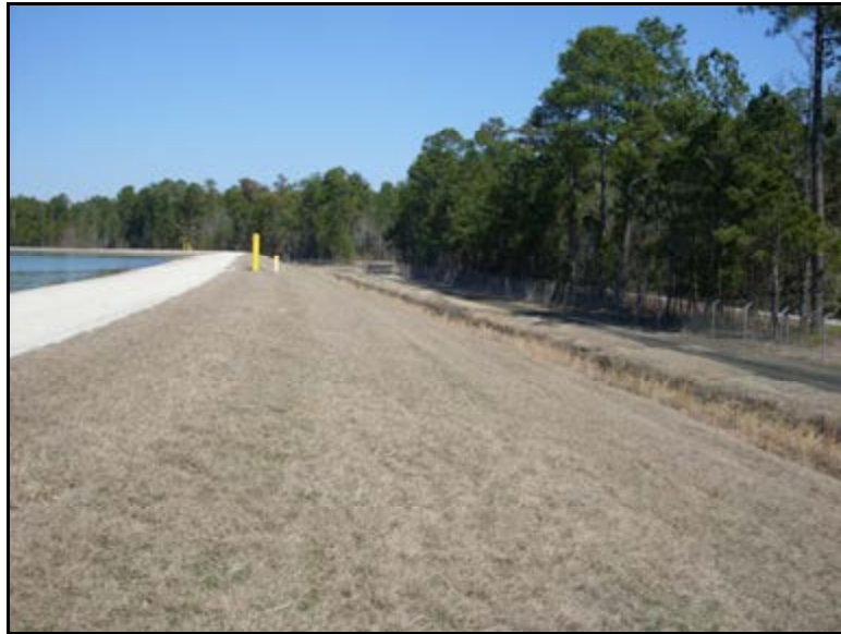
Photograph 5.7a. Typical view of outside slope and toe, east side looking north.
