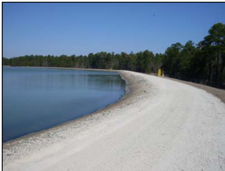
Photograph 5.6b. Typical view of inside slope and crest, east side looking north.
