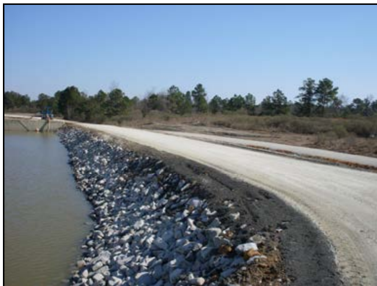
Photograph 5.9b. Typical view of inside slope, southeast side looking northeast.
