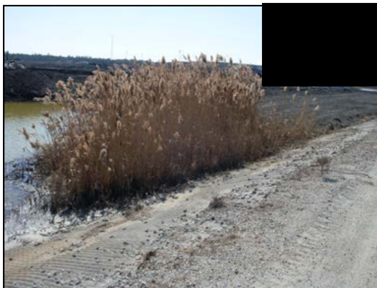
Photograph 5.6c. View of reeds (Phragmites) growing on inside slope, northwest side looking south.
