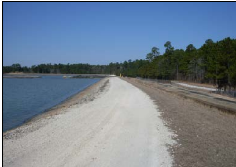
Photograph 5.6a. Typical view of crest and inside slope, northeast side looking northwest.
