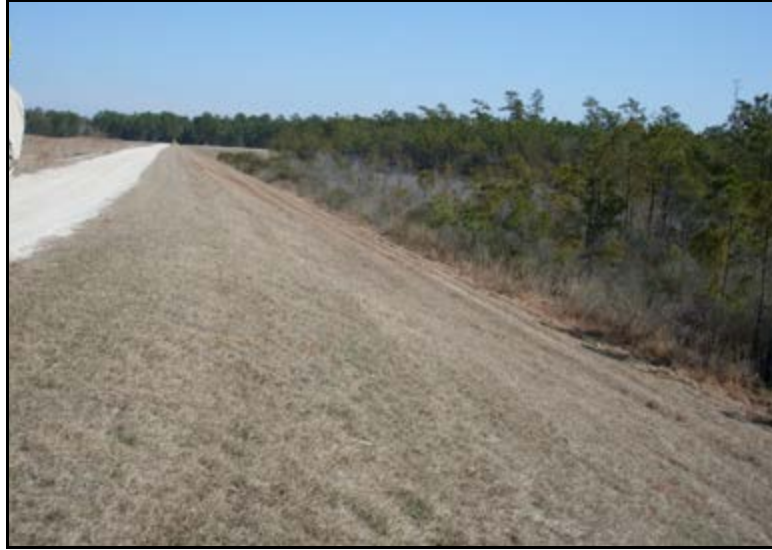
Photograph 5.4. Typical view of outside slope, southeast side looking northeast.
