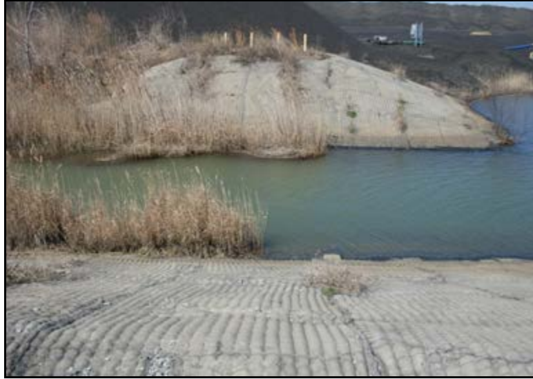
Photograph 5.14. Trapezoidal notch weir.
