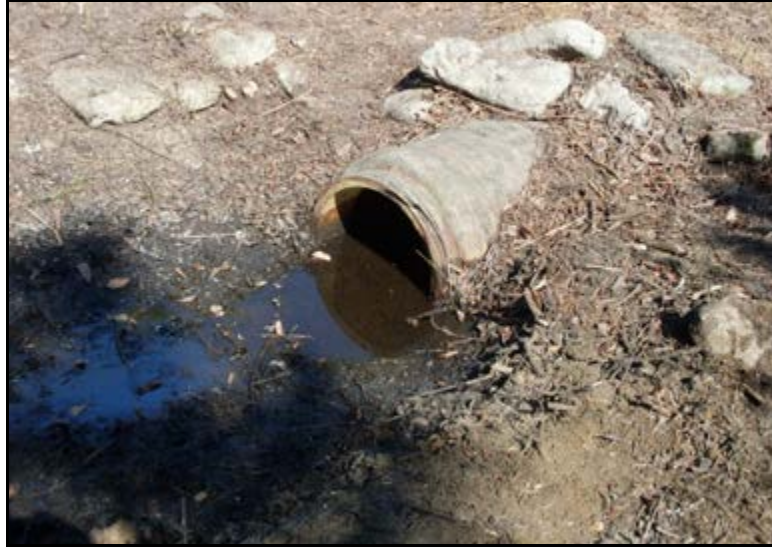
Photograph 5.12. Discharge end of emergency outlet conduit.
