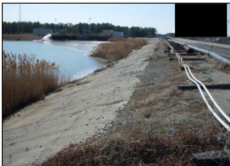
Photograph 5.3. Typical view of inside slope, northwest side looking southwest.
