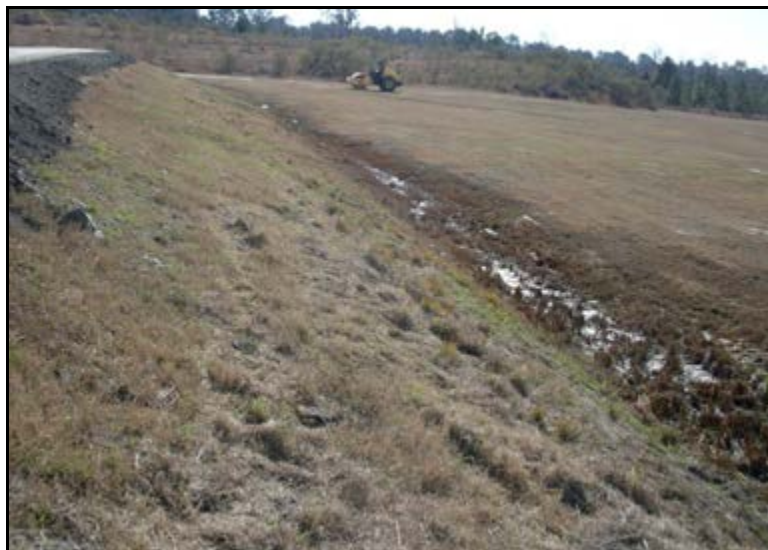
Photograph 5.10. View of outside slope and toe, southwest side looking southeast.
