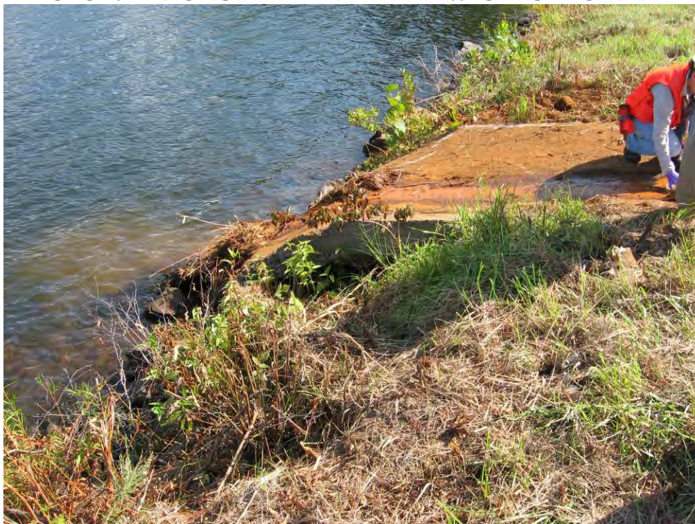
PHOTO 4: END OF CHIMNEY DRAIN AT WEST ASH POND DAM
