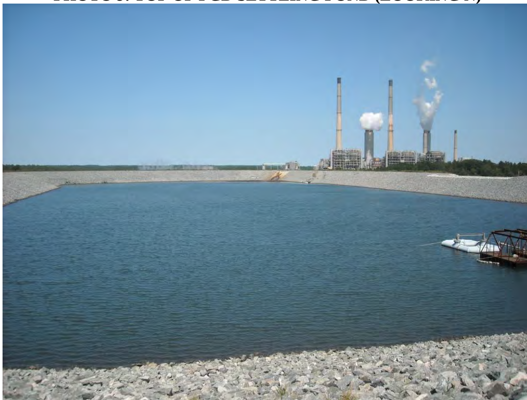
PHOTO 10: FLOATING SKIMMER OF FGD SETTLING POND (LOOKING N)
