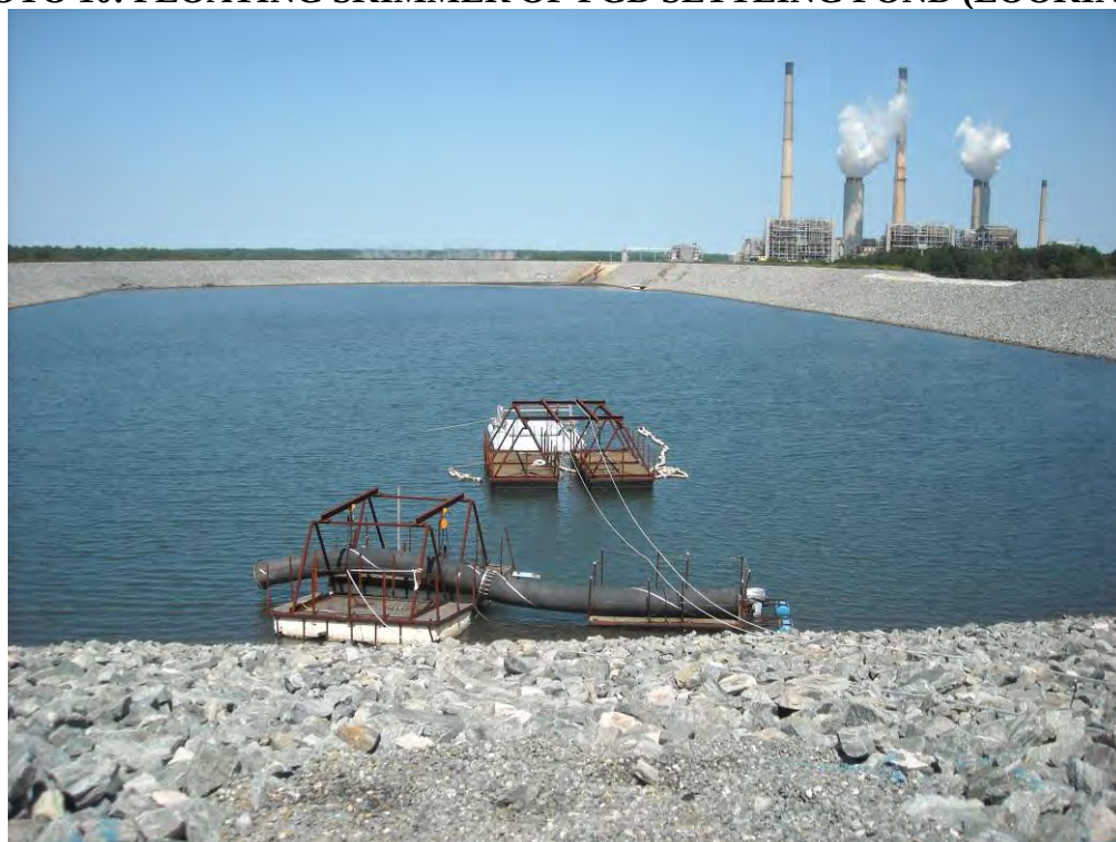
PHOTO 10: FLOATING SKIMMER OF FGD SETTLING POND (LOOKING N)
