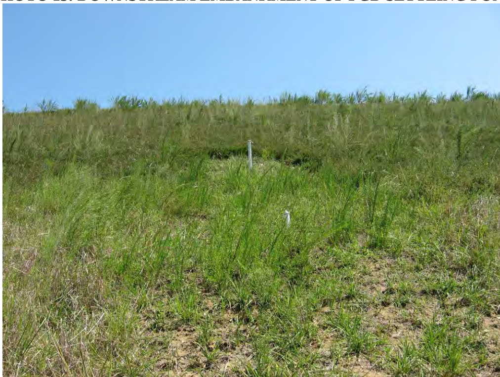
PHOTO 13: DOWNSTREAM EMBANKMENT OF FGD SETTLING POND
