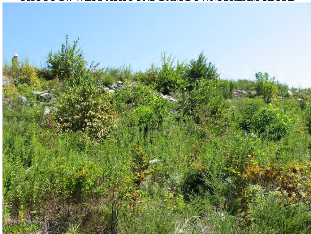
PHOTO 24: WEST ASH POND DAM DOWNSTREAM SLOPE
