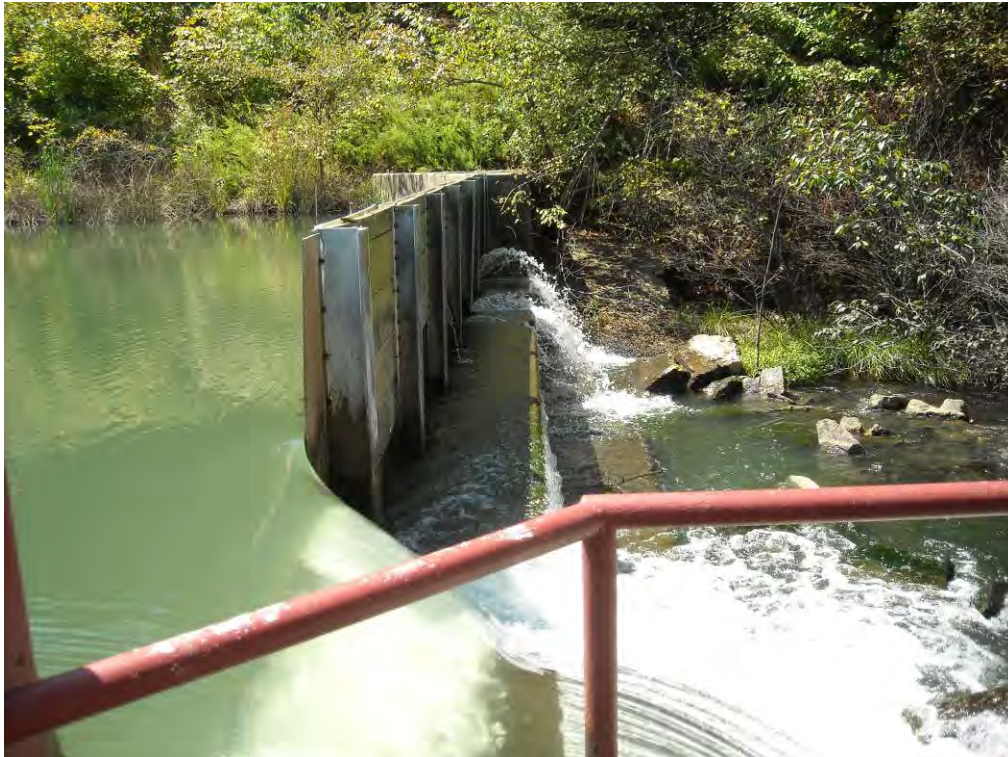
PHOTO 27: CLOSE UP OF WEST ASH POND DAM DISCHARGE WEIR STRUCTURE
