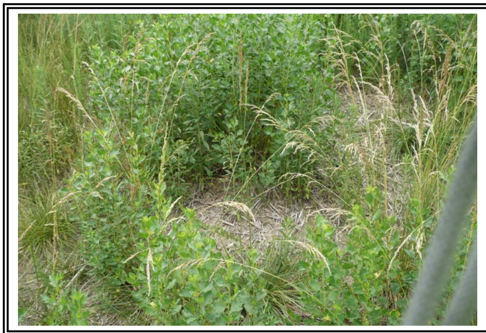
Sparse and weedy vegetation cover on the 1985 Ash Pond West Dike.
