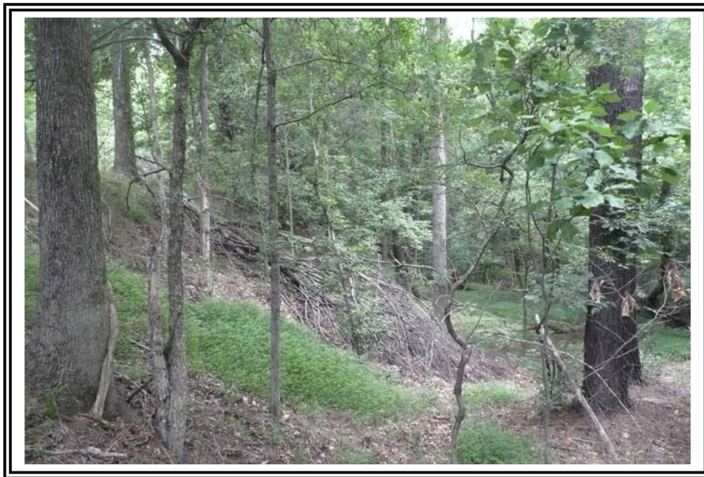
Typical slope sloughing and erosion on the 1956 Ash Pond Dikes.
