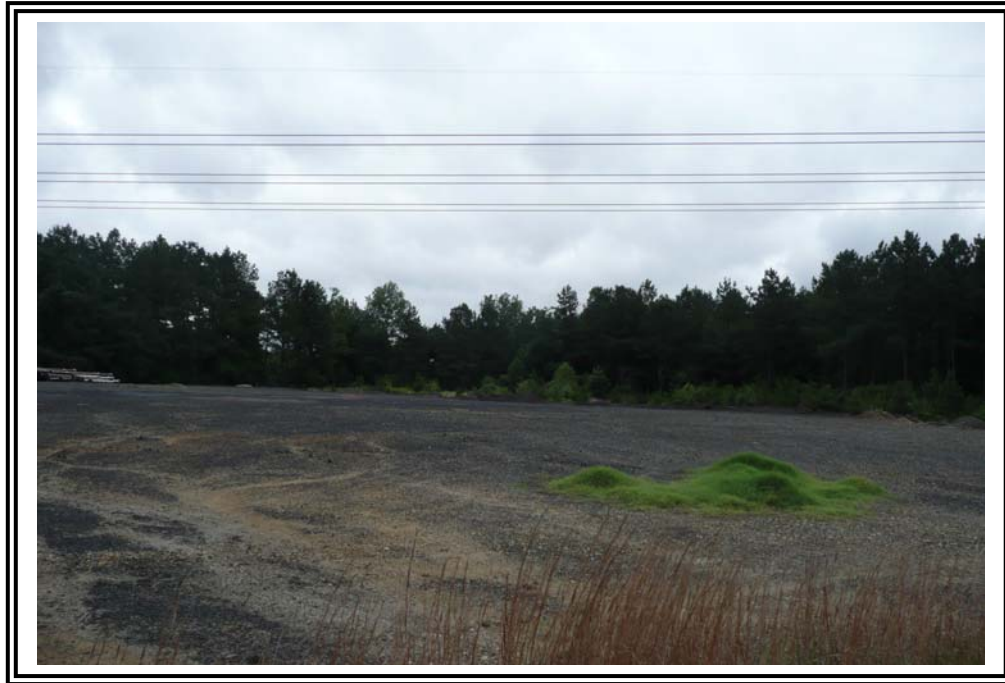
North end of 1963 Ash Pond.
