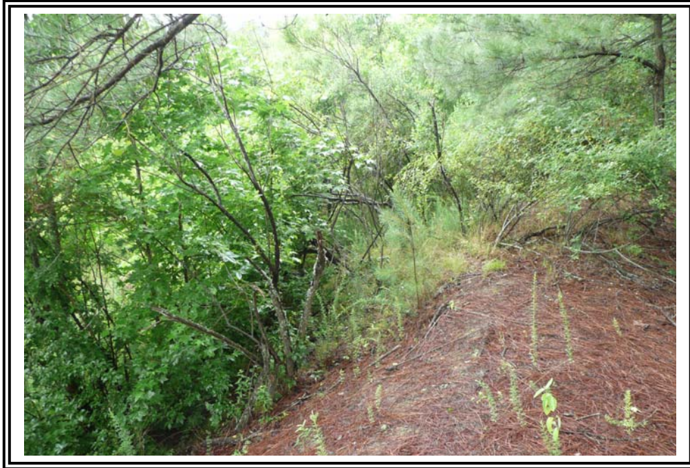
Upstream slope of 1970 Ash Pond east dike looking north.
