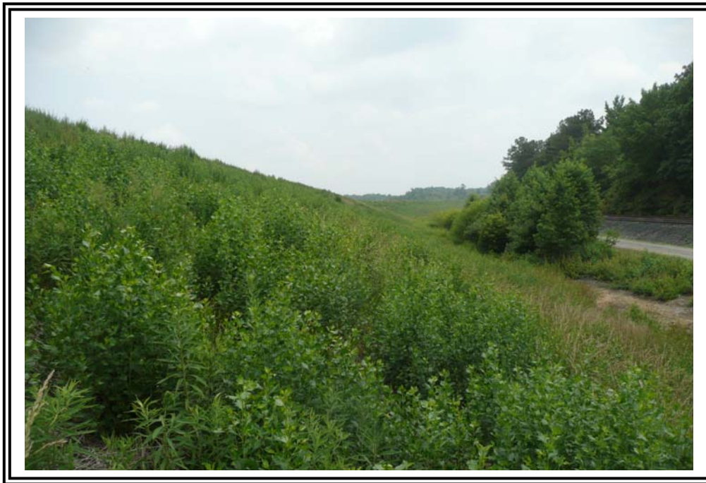
1985 Ash Pond West Dike approaching bend, looking southeast.
