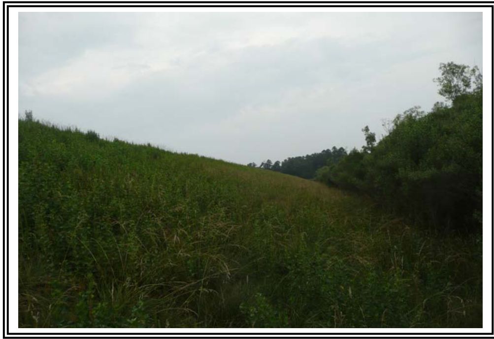
South Dike of the 1985 Ash Pond, looking northeast.
