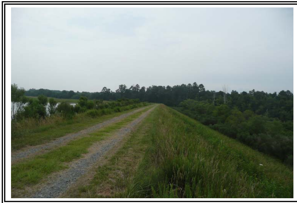
Crest of the east Dike of the 1985 Ash Pond, looking north.
