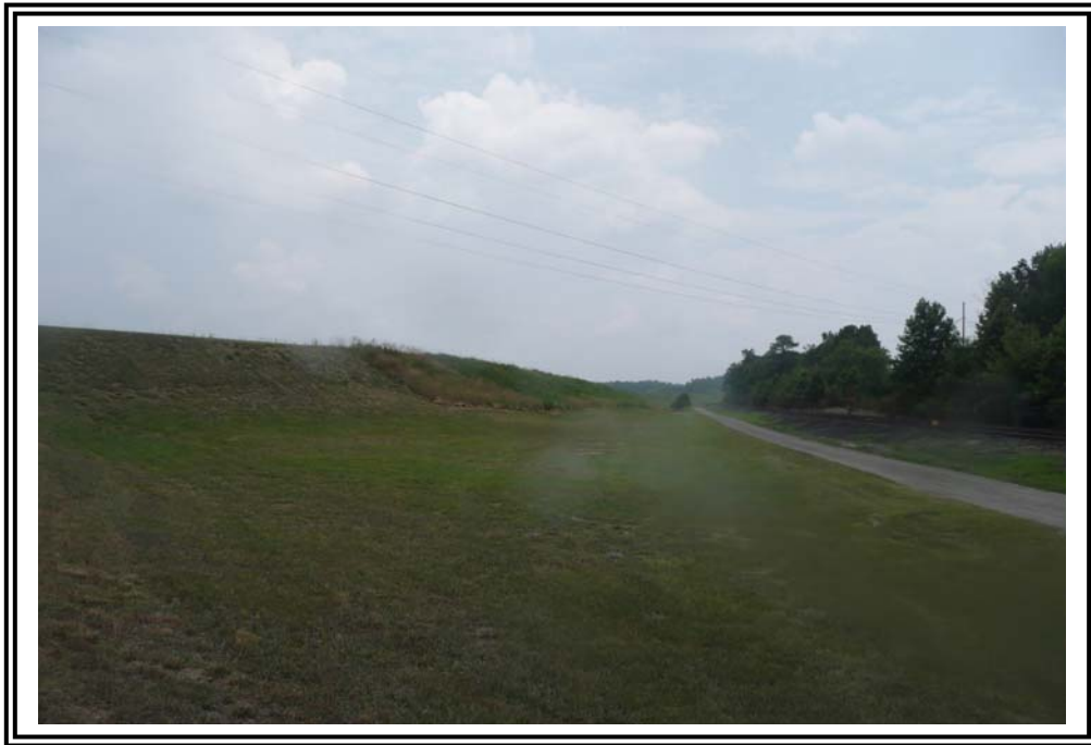
Northwest end of 1985 Ash Pond West Dike, looking southeast.
