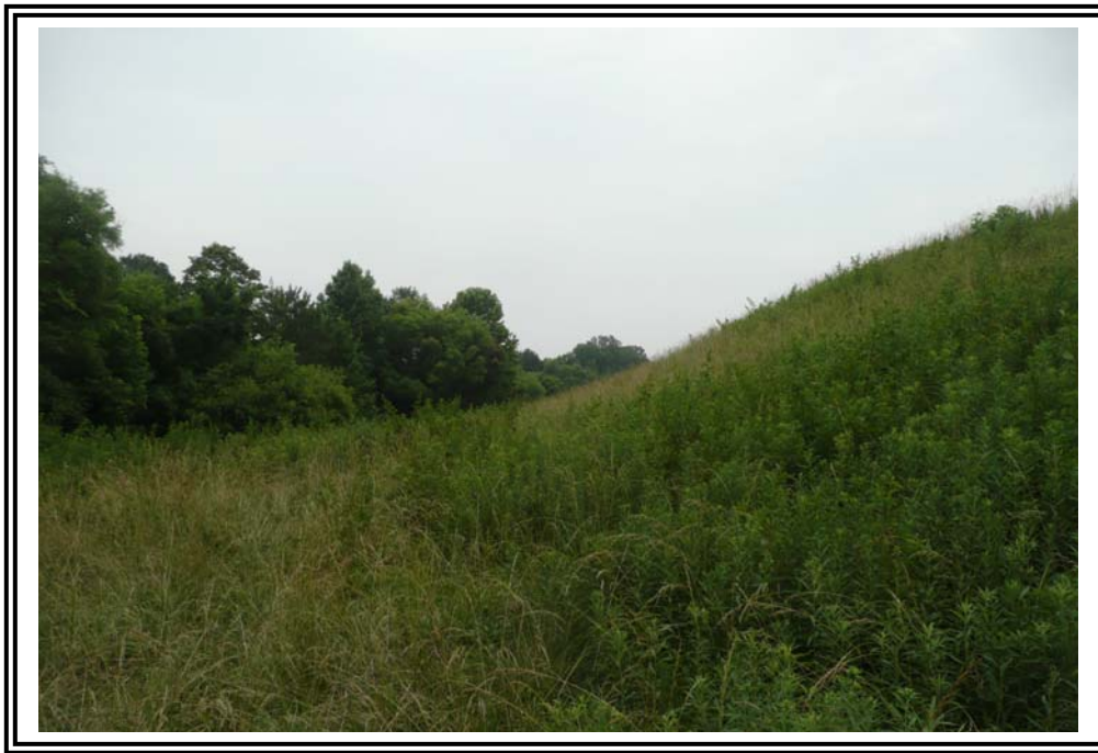
Corner at the north and northeast Dike of the 1985 Ash Pond, looking east.
