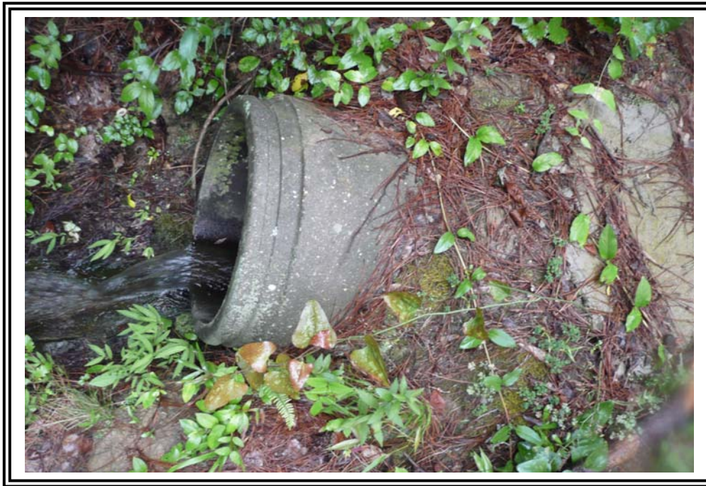
Discharge end of outlet pipe in the 1978 Ash Pond.
