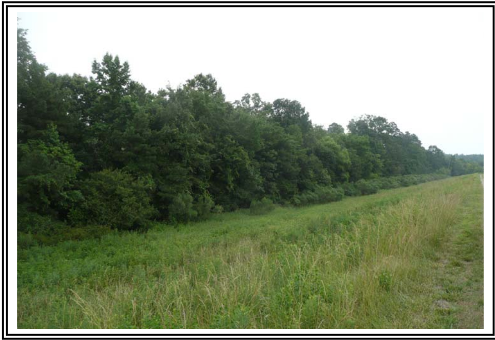
East Dike of the 1985 Ash Pond, looking southeast.
