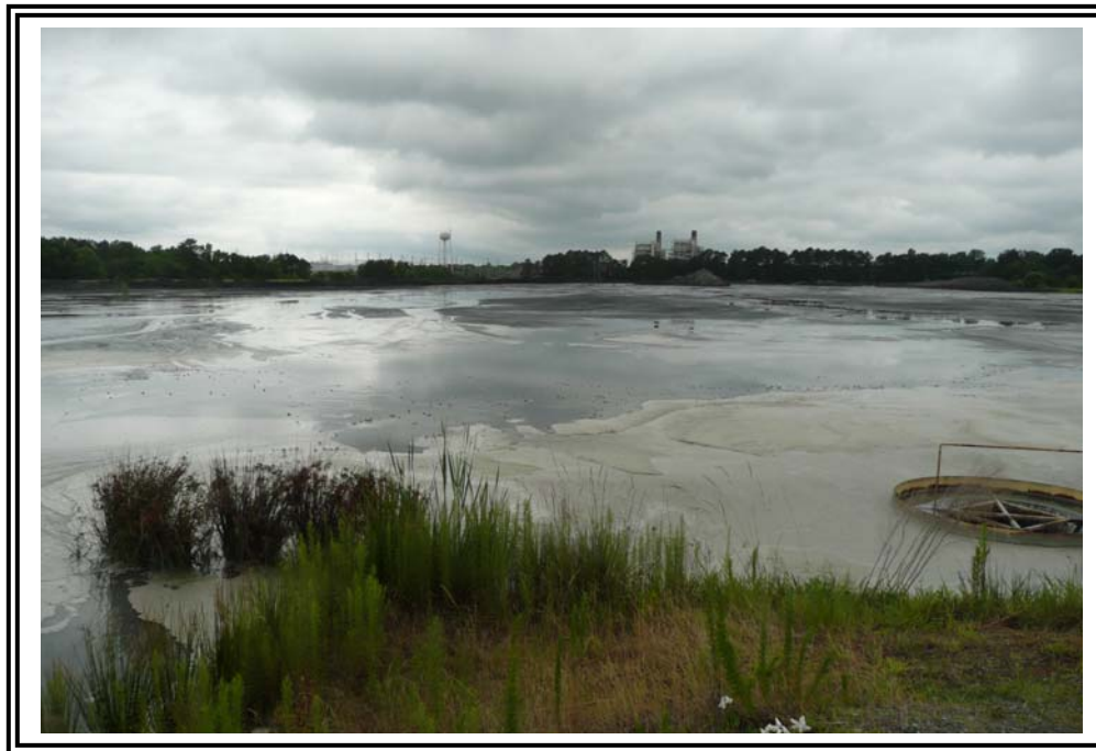
Current ash disposal in a "Pond within a pond". Pond was constructed with earthen dikes placed on top of ash in 1985 Pond, looking northwest.
