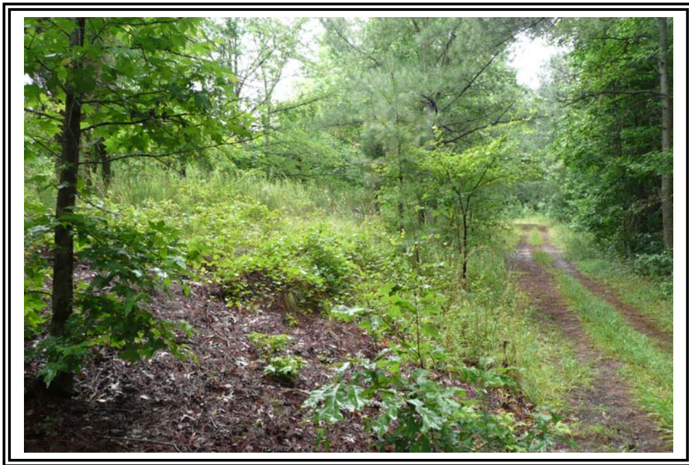
1970 Ash Pond south dike downstream slope looking east.
