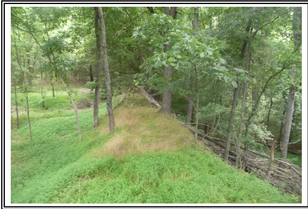
Crest of the 1956 Ash Pond Dike.
