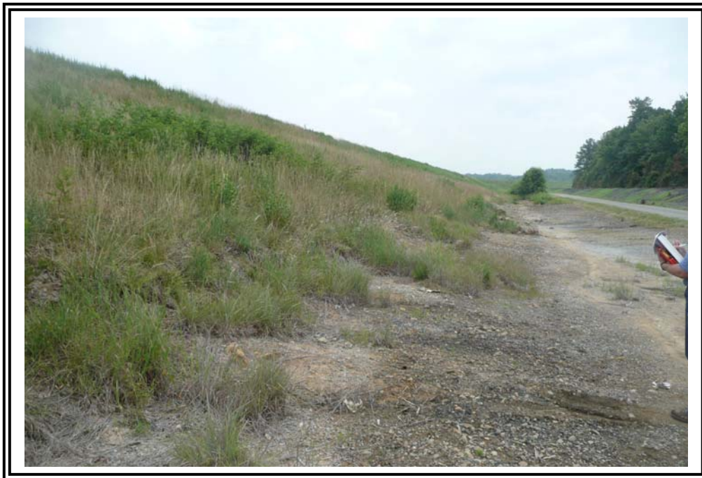
1985 Ash Pond West Dike toe along the northern portion of Dike.
