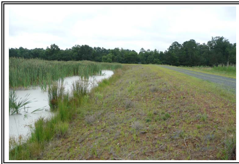
East Dike of "Pond within a Pond" upstream slope, looking northeast.
