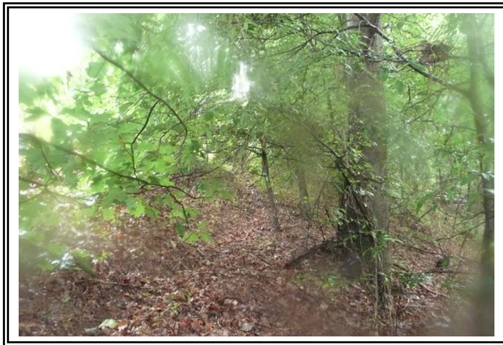
Generally wooded conditions along the east side of the 1978 Ash Pond Dike downstream slope.
