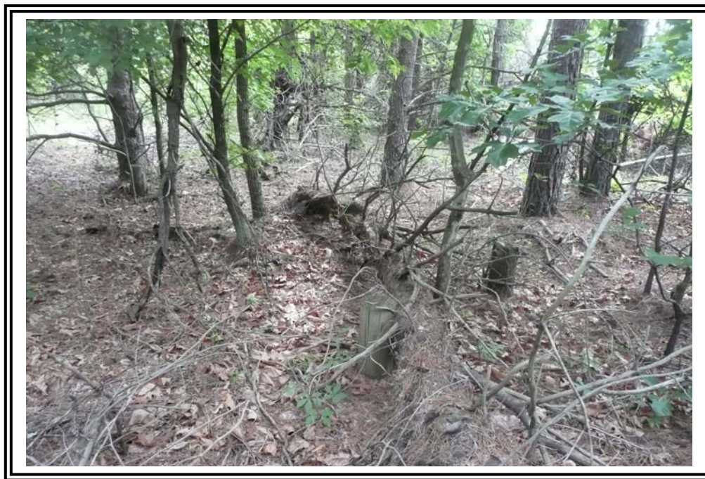
Remains of outlet structure at southwest corner of 1956 Ash Pond.
