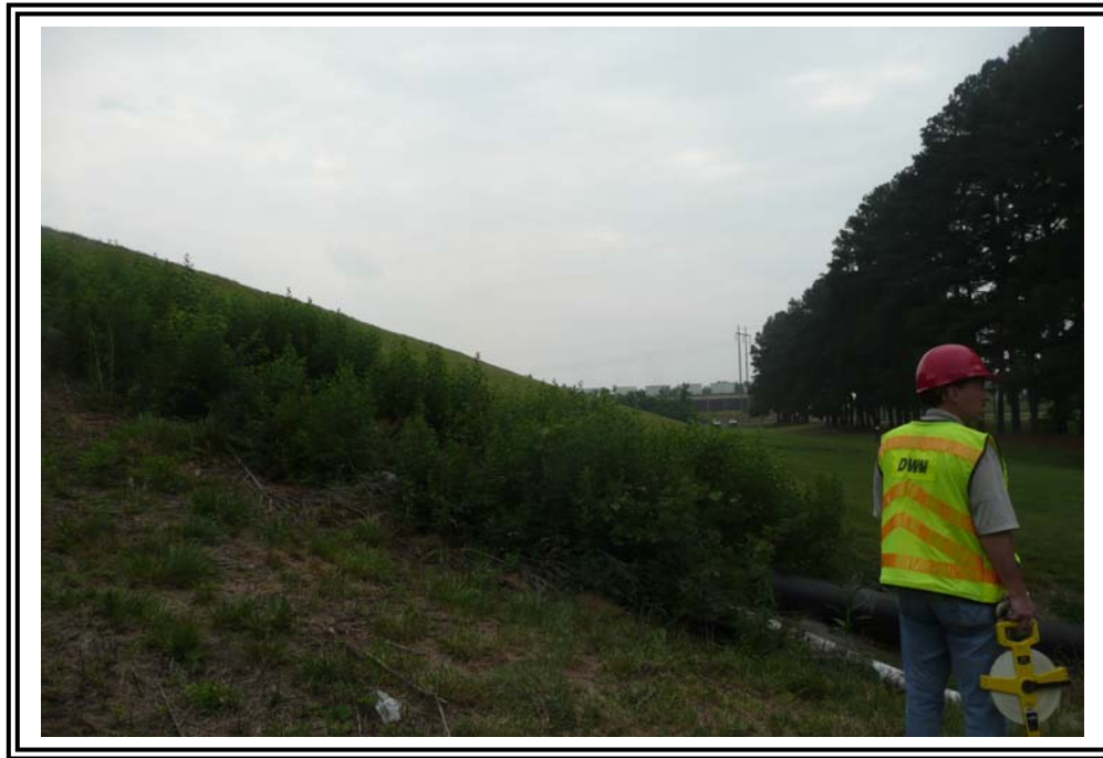
North Dike of the 1985 Ash Pond, looking southwest.
