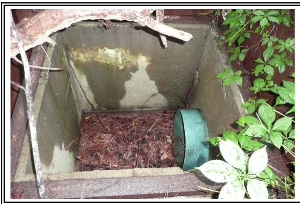
Close up of 1970 Ash Pond outlet control structure.
