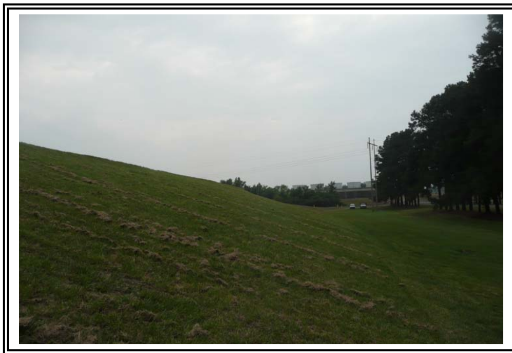
North Dike of the 1985 Ash Pond, looking southwest.
