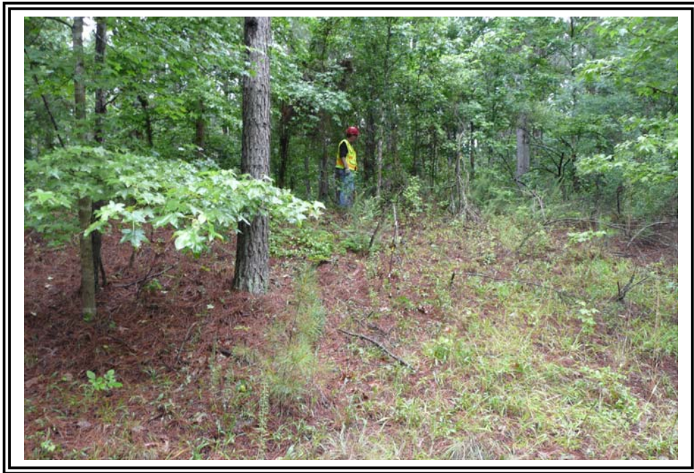
1970 Ash Pond east dike downstream slope. Note photographer is standing at the toe of the dike and the person in the photograph is standing at the crest.
