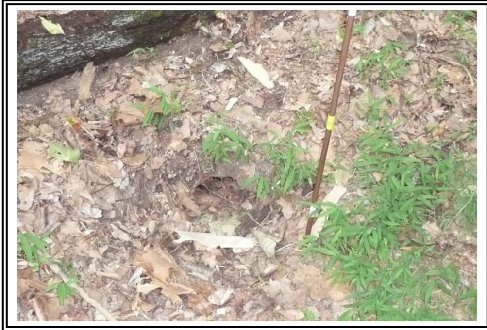
Top of probable stormwater outlet pipe on the 1956 Ash Pond Dike.
