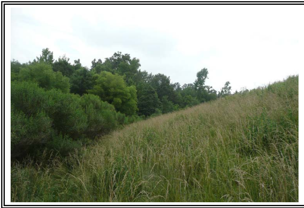
Southeast corner of the 1985 Ash Pond Dike, looking southwest.
