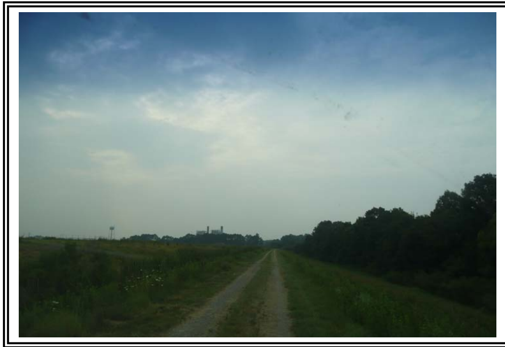
Northeast Dike crest of the 1985 Ash Pond, looking west.
