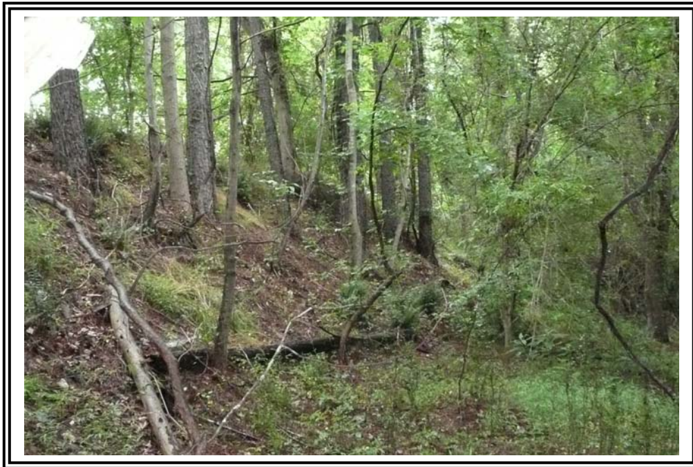
1970 Ash Pond downstream slope near southwest corner.
