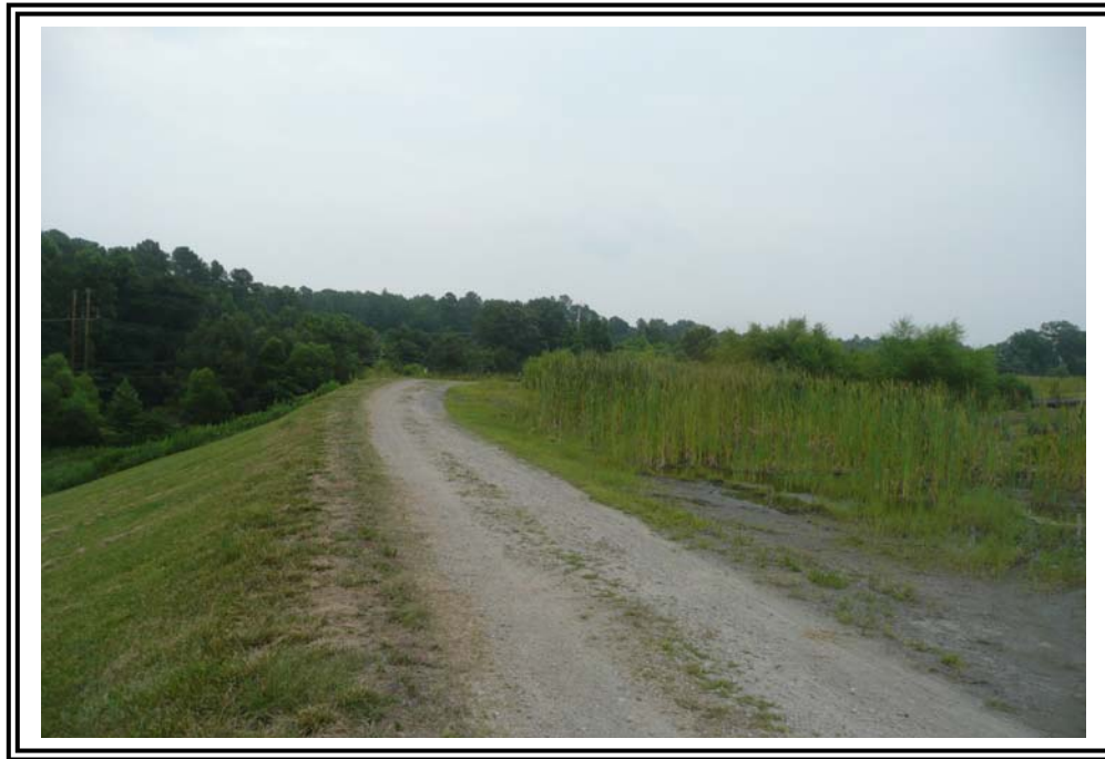
North Dike crest of the 1985 Ash Pond, looking northeast. Note: Ash level is approximately at the crest of the Dike.
