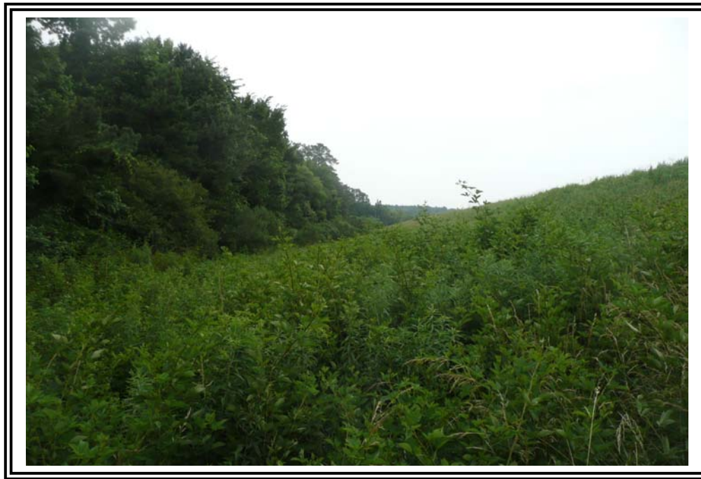
East Dike of the 1985 Ash Pond, looking south.
