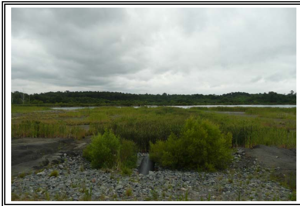
Outlet of "Pond within a Pond" into 1985 Ash Pond, looking southeast. Notice ash stockpiles within the pond.
