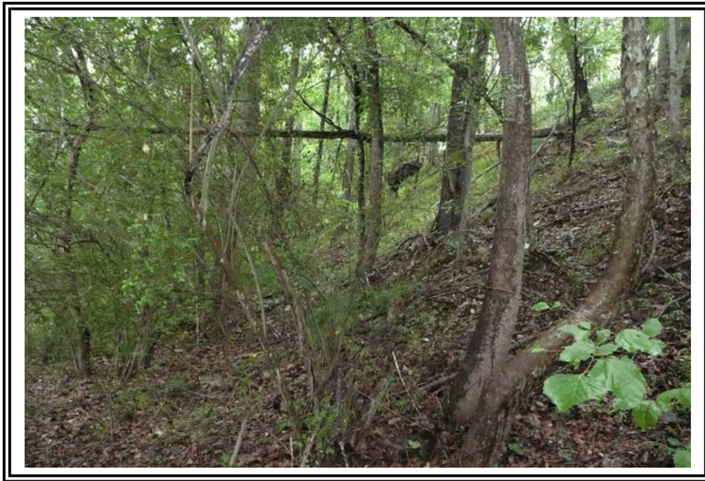
Typical condition of 1970 Ash Pond west dike downstream slope (looking north).
