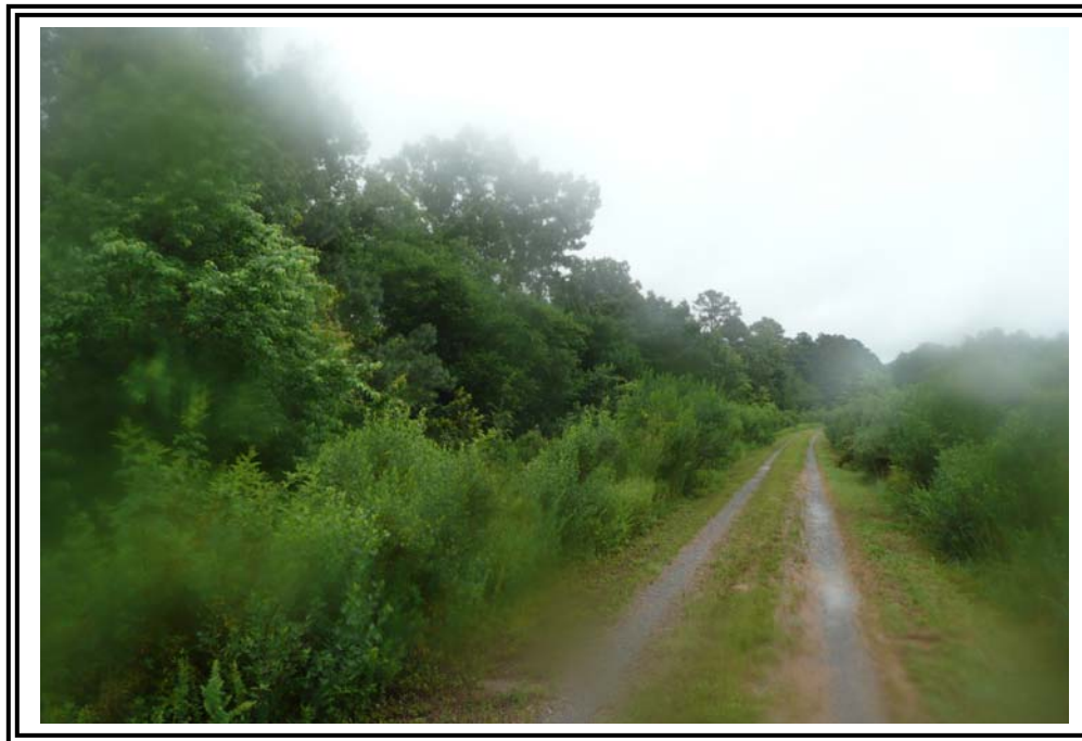
Crest of the 1978 Ash Pond Dike approaching the east corner of the Dike, looking south. Note: Taller trees are on the downstream slope in the left of the photo and shorter brush is on the upstream slope in right of the photo.
