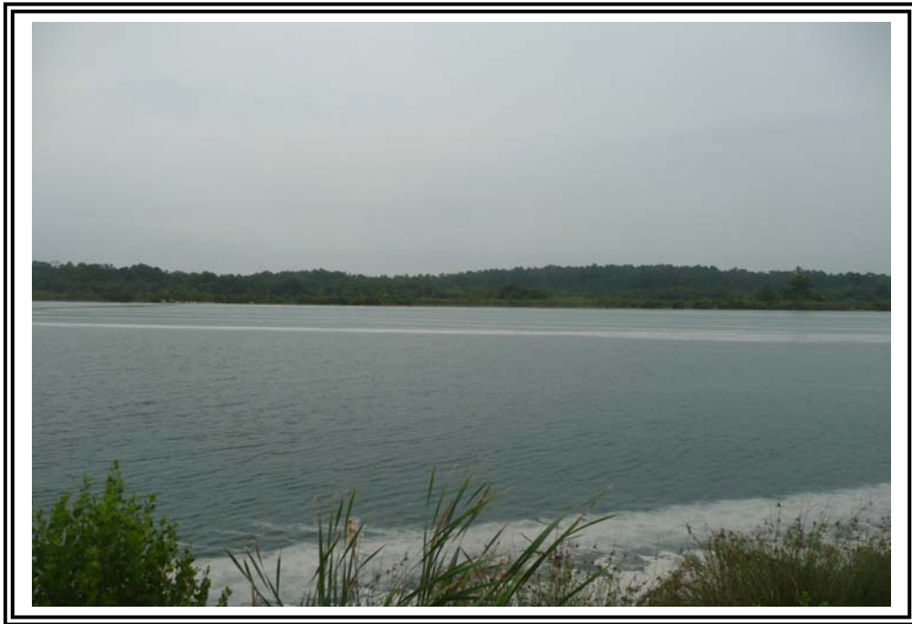
Looking east across the 1985 Ash Pond at the east Dike.
