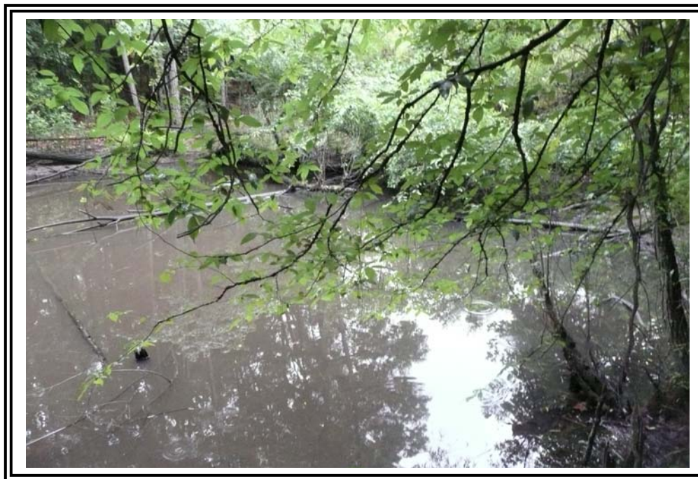
Ponded area south of the discharge pipe at the toe of the 1978 Ash Pond Dike. Reportedly excavated area from former adjacent property owner, who was a brick manufacturer.
