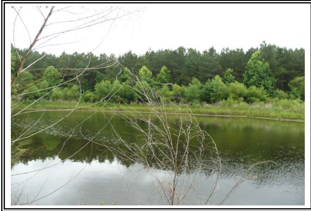
1970 Ash Pond looking north across the pond from the south dike.
