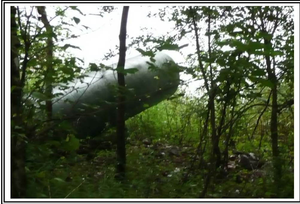
Downstream end of 1970 Ash Pond outlet.
