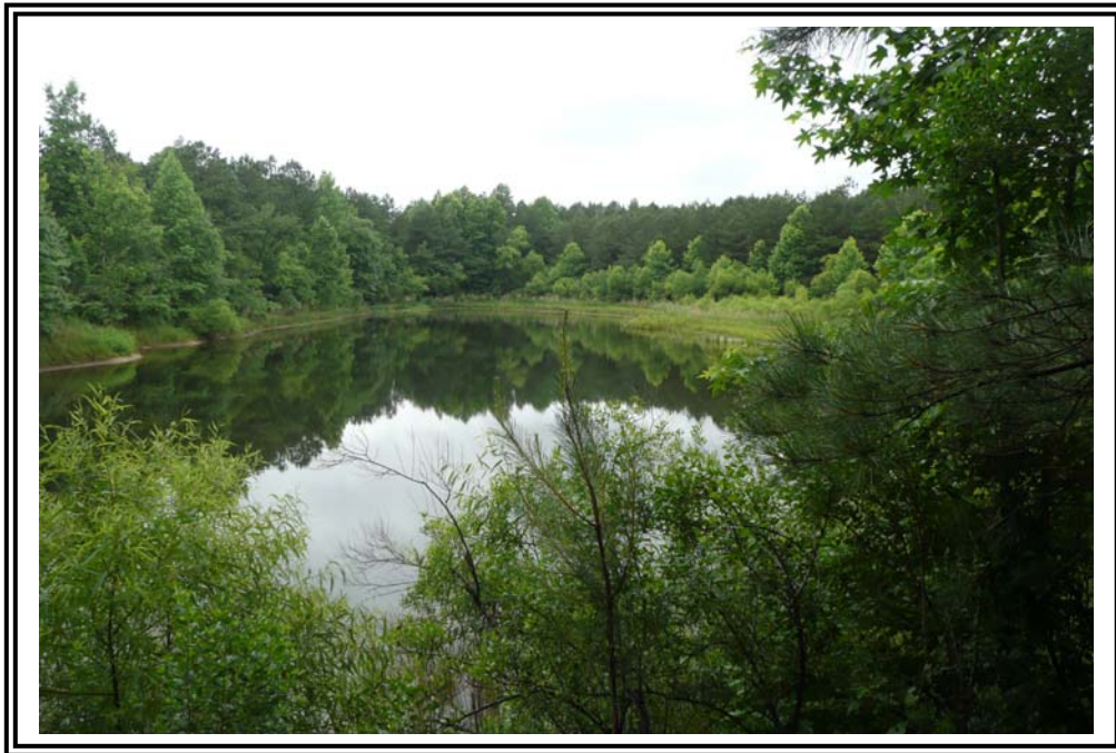
Southern portion of 1970 Ash Pond contains water. Looking west from east dike.
