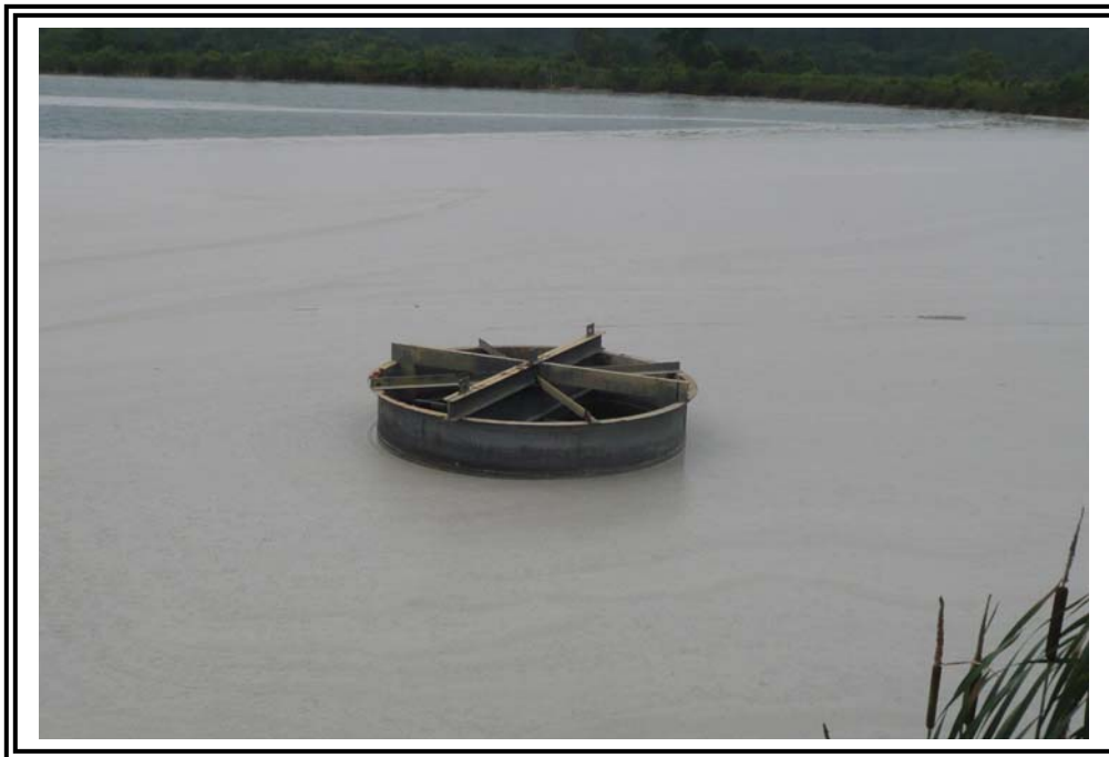
Outlet structure in the 1985 Ash Pond.
