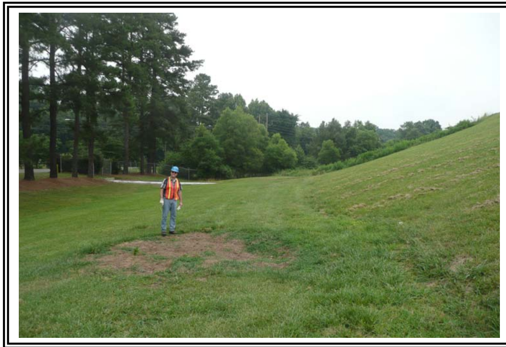
Toe of the North Dike of the 1985 Ash Pond, looking northeast. Note: Bare patch at the toe of the Dike.
