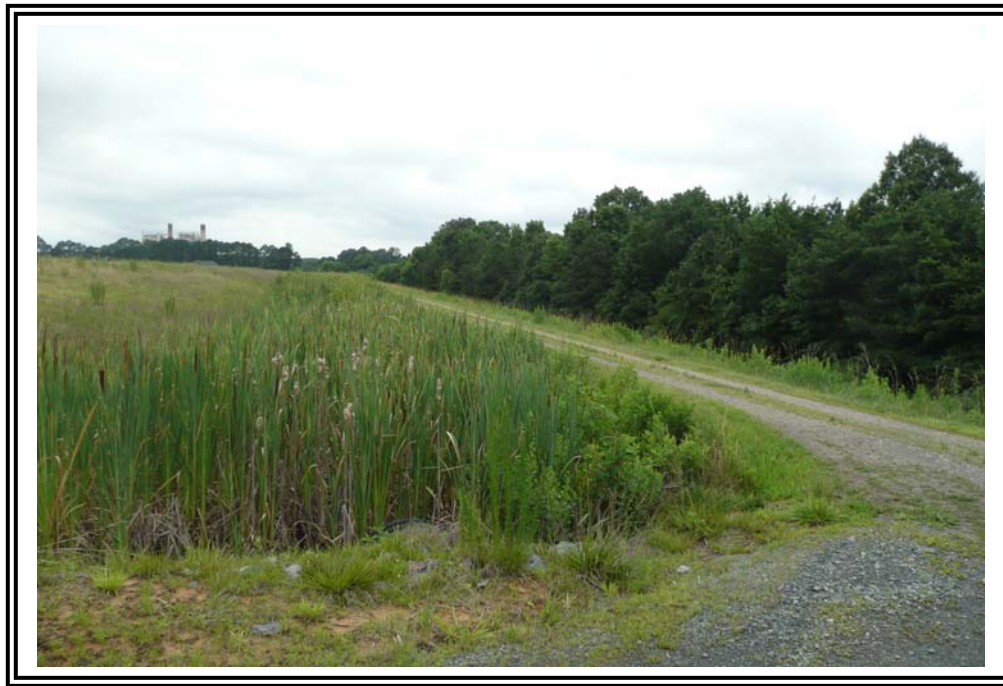
Space between "Pond within a pond" north Dike and 1985 Ash Pond northeast Dike, looking northwest.
