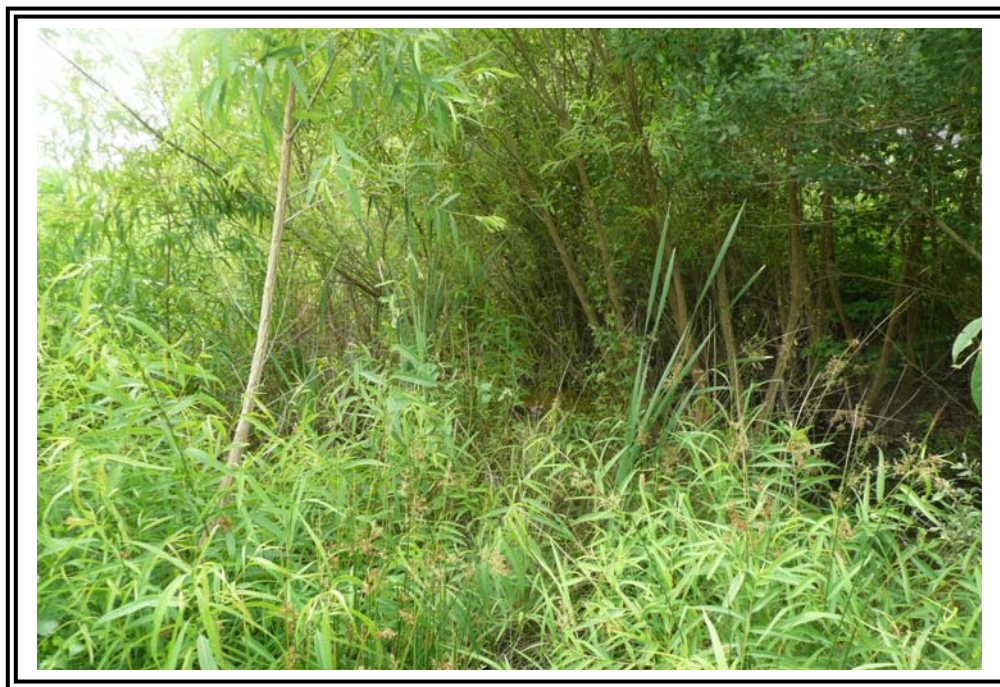
Woody growth along the West Dike of the 1985 Ash Pond.
