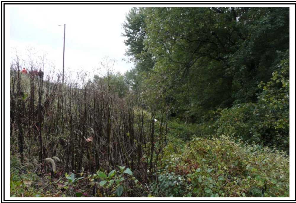
Exterior slope of south dike (Clearwater Pond section), looking east.
