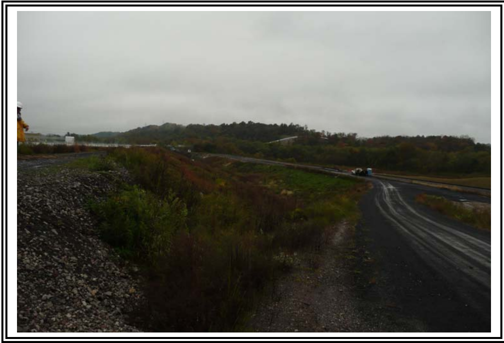
West dike exterior slope, looking south.
