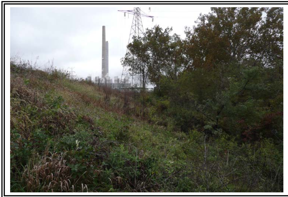
Exterior slope of east dike (Clearwater Pond section), looking north.
