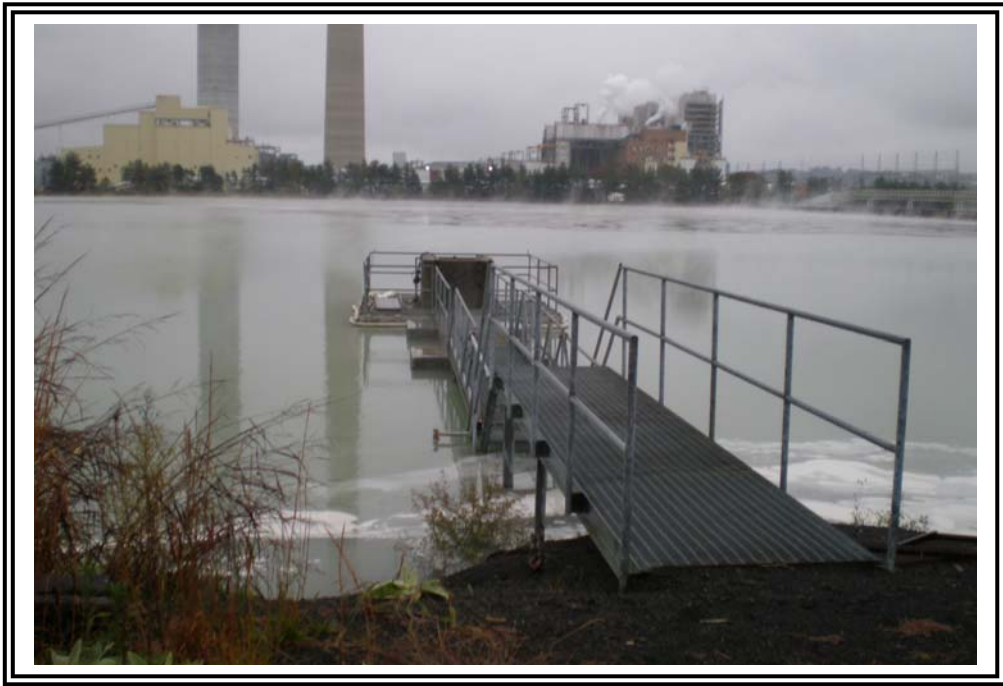
South Fly Ash Pond outlet structure, looking southeast.
