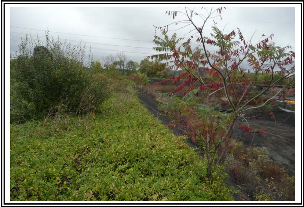
Interior slope of north dike, looking east.
