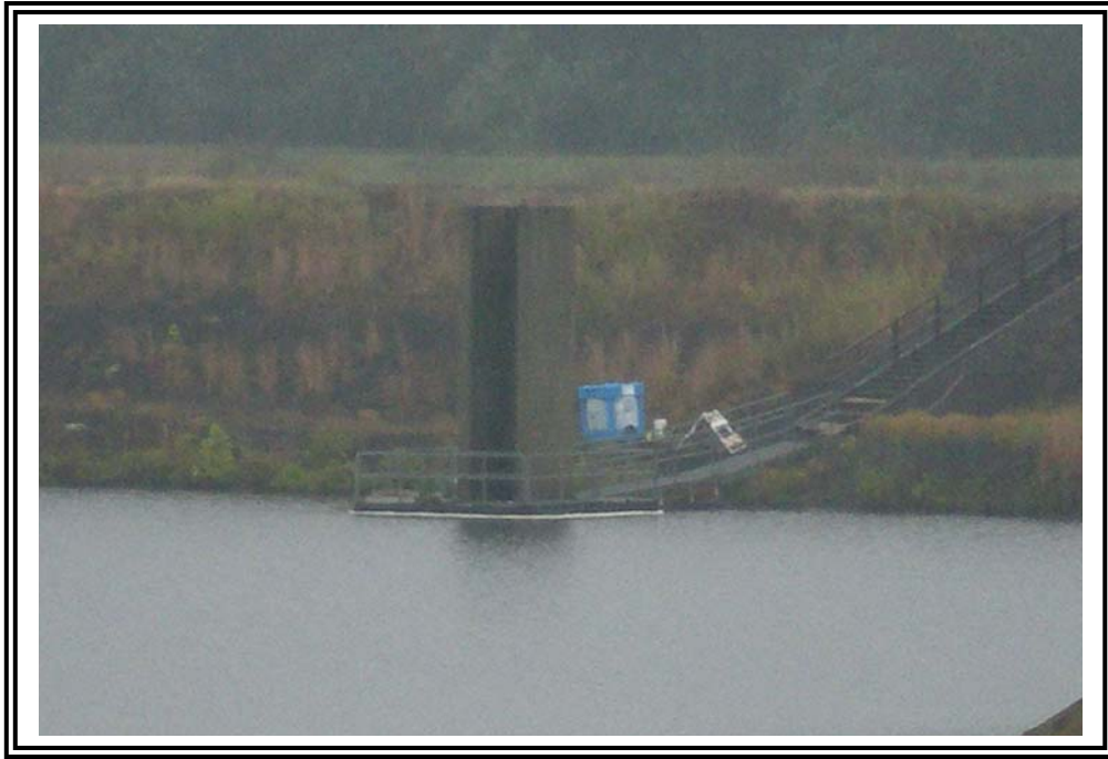
Overflow structure, looking south.
