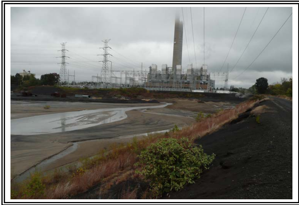
East dike interior slope, looking north. Note isolated woody vegetation on slope.
