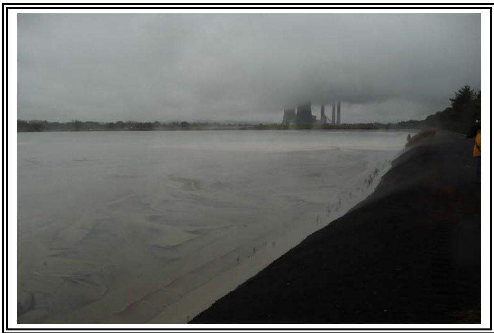
Interior slope of east dike, looking north. Slope is covered predominately with ash with little vegetation.
