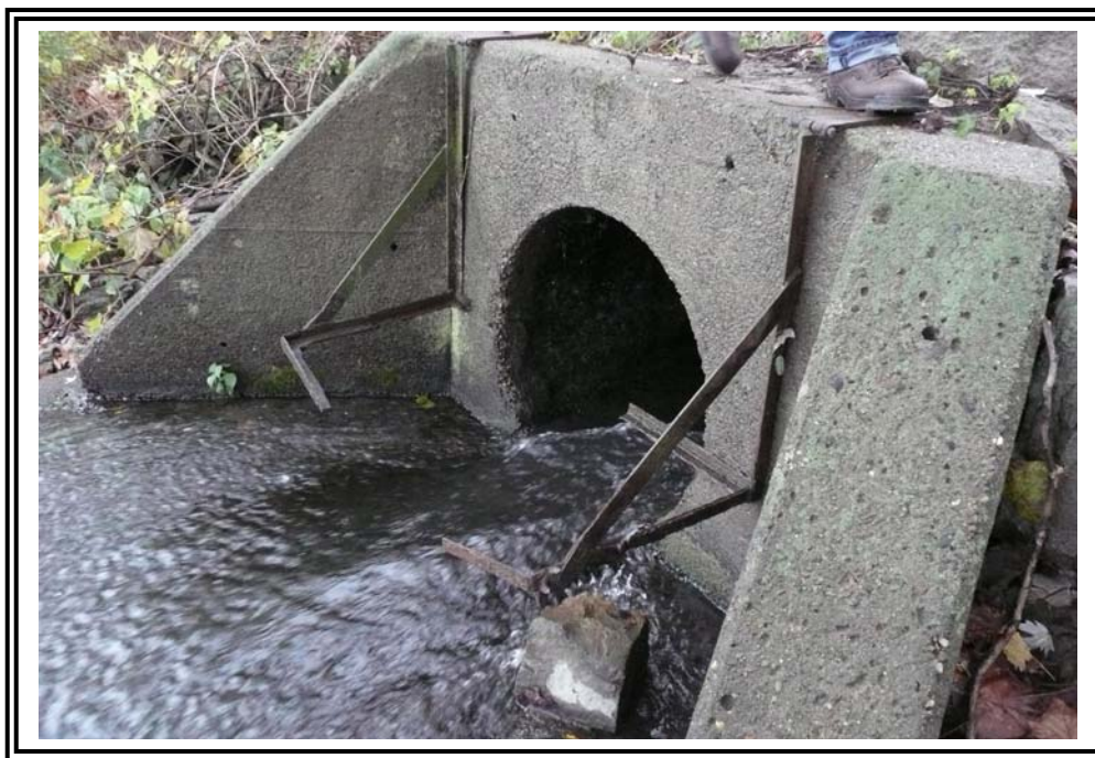
36-inch diameter Bottom Ash Pond outlet.
