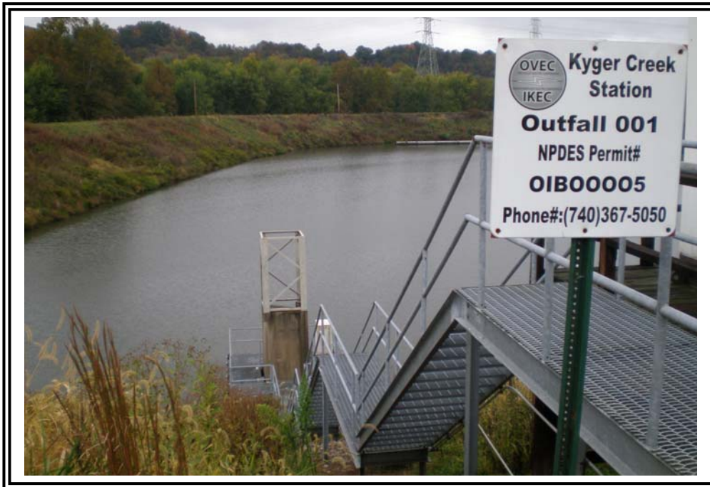
Clearwater Pond outfall structure.
