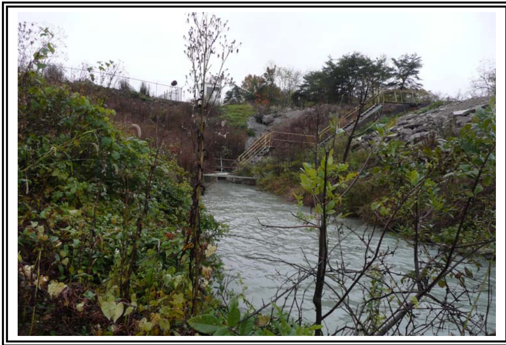
Drainage ditch near South Fly Ash Pond outlet. Note pooling water and heavy vegetation.
