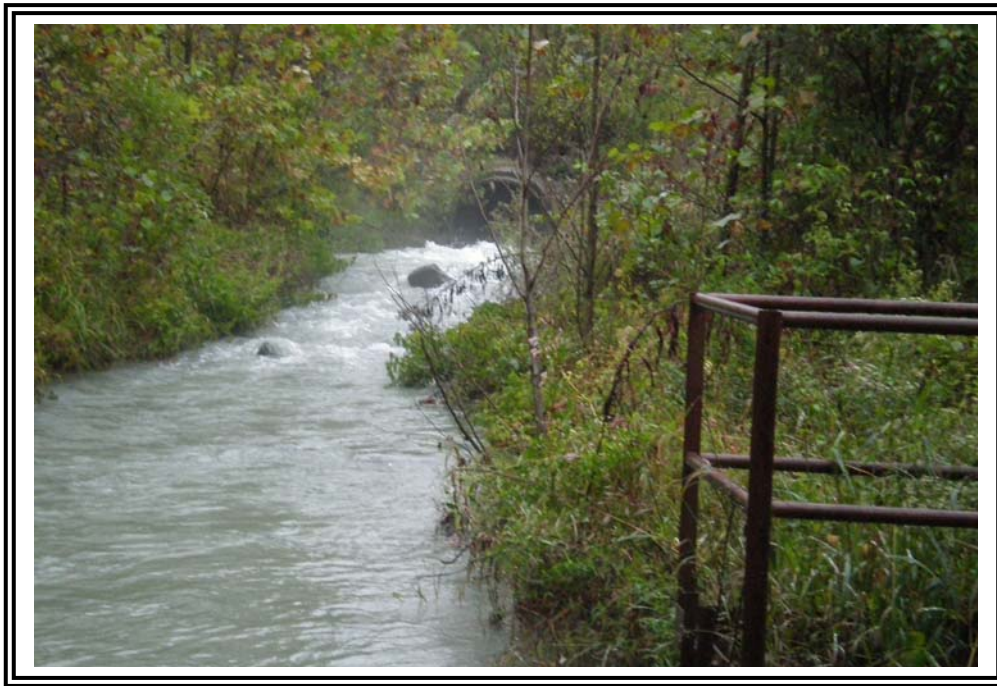
Outfall, facing north.
