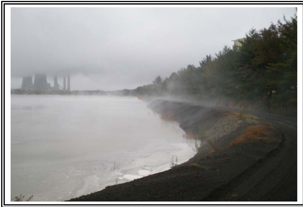
Interior slope of east dike, facing northeast.
