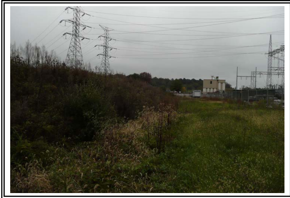
Exterior slope of north dike, looking west. Dike is approximately 5 to 8 feet high in this location where the pond is predominately incised.
