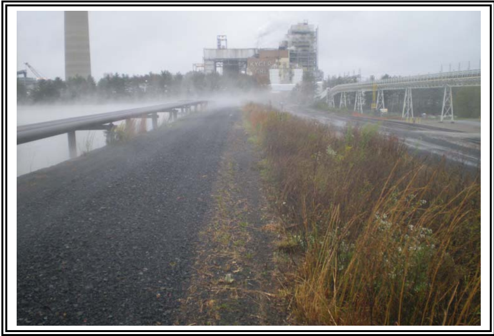
South dike crest, facing southeast.
