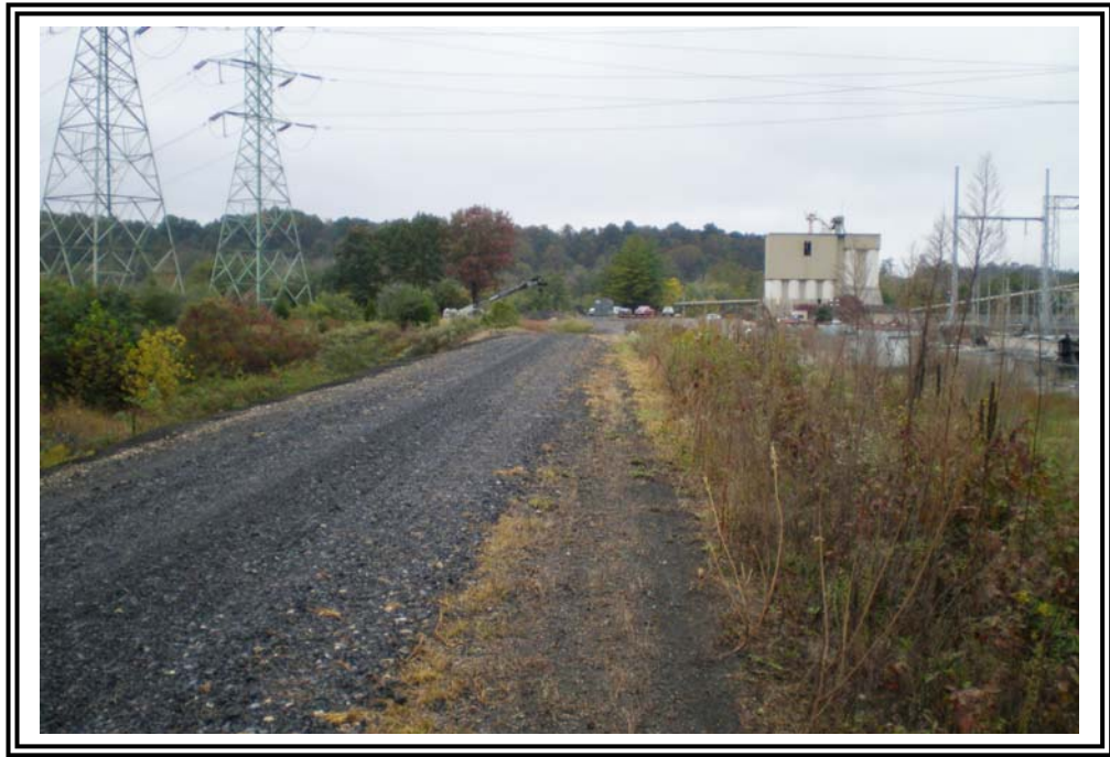
Crest of north dike, facing northwest.
