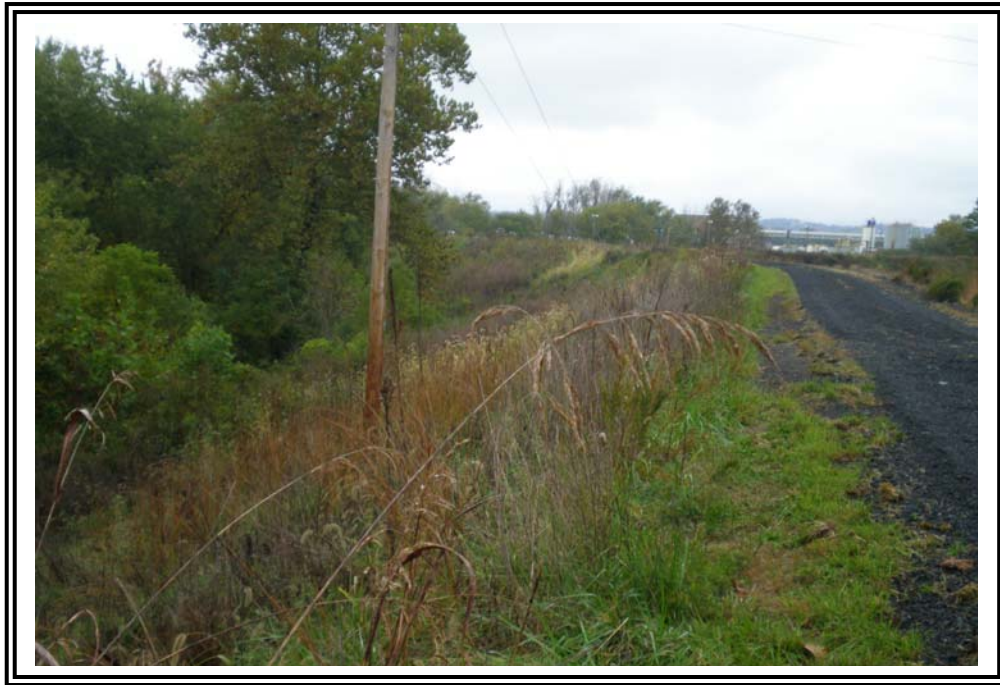
Exterior slope and crest of south dike, looking north.
