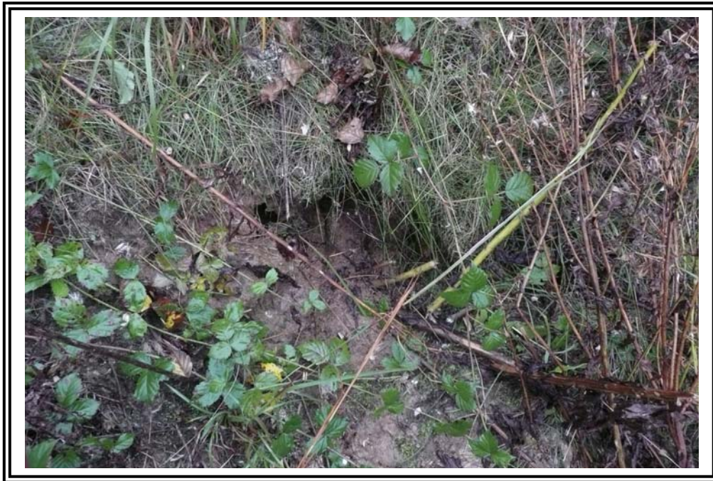
Possible animal burrow in west dike exterior slope.
