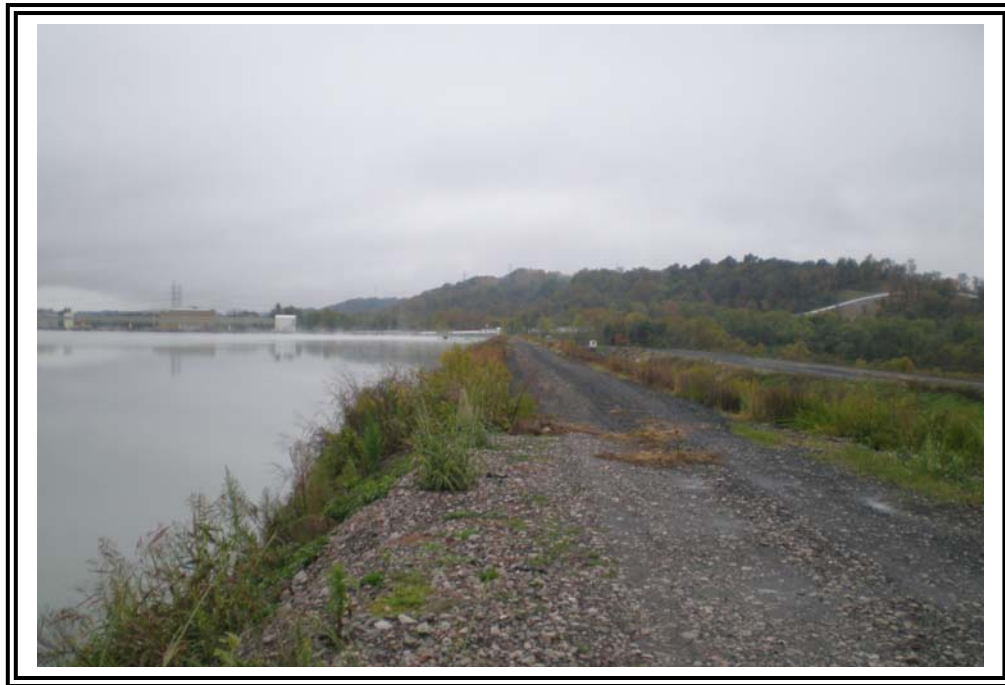
West dike crest and interior slope, looking south.
