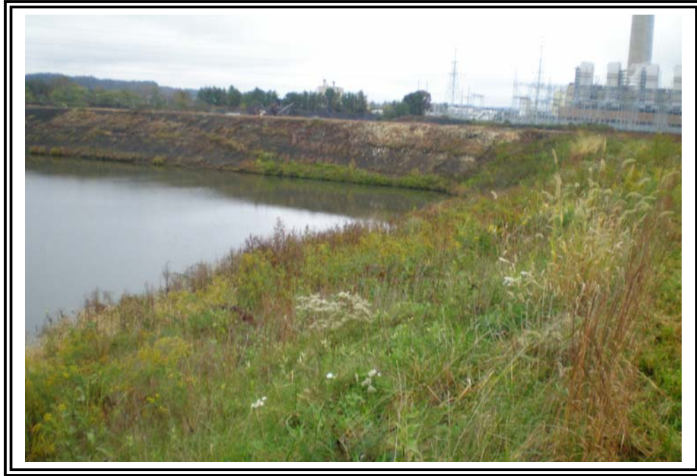
Interior slope of Clearwater Pond (south dike), looking northeast.
