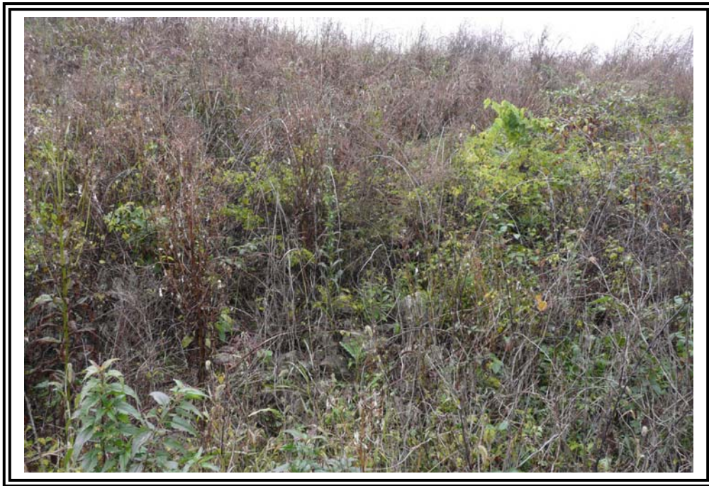
Area of rock slope protection/drain on exterior slope of east dike. Slope protection placed where slope steepened in area of transmission tower.
