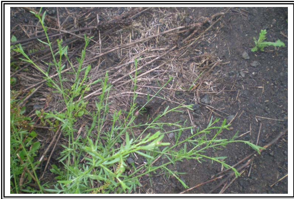
Small, isolated animal burrow on interior slope of the south dike.
