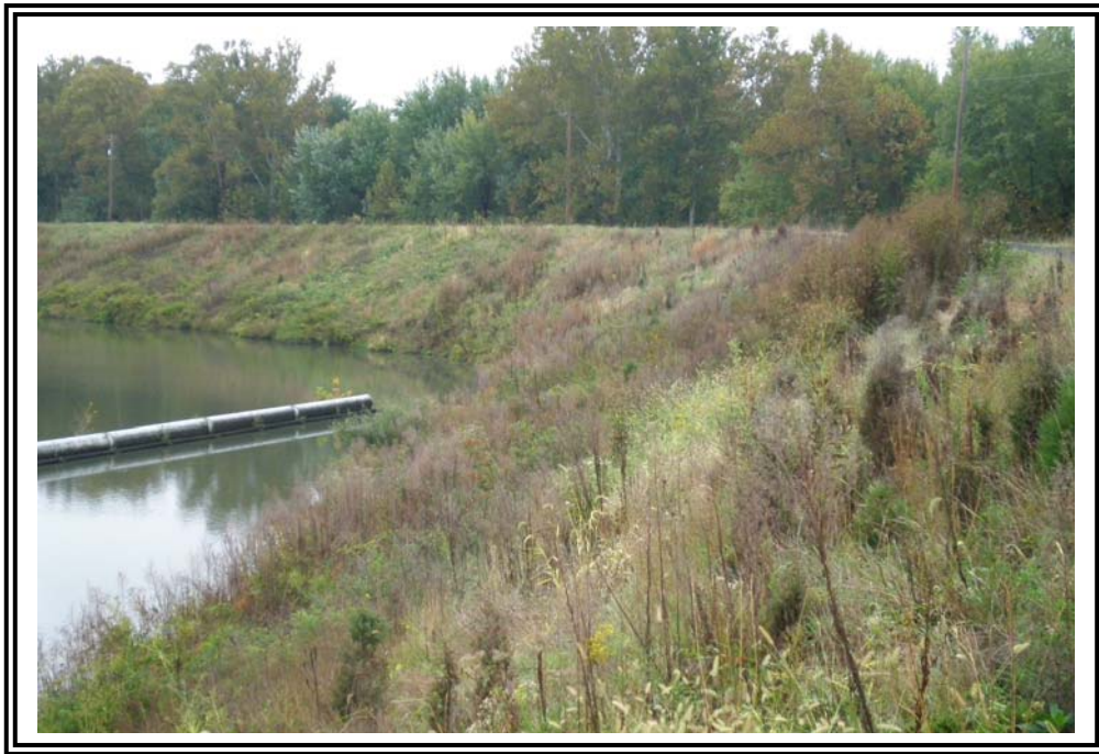
Interior slope of south dike, facing south.
