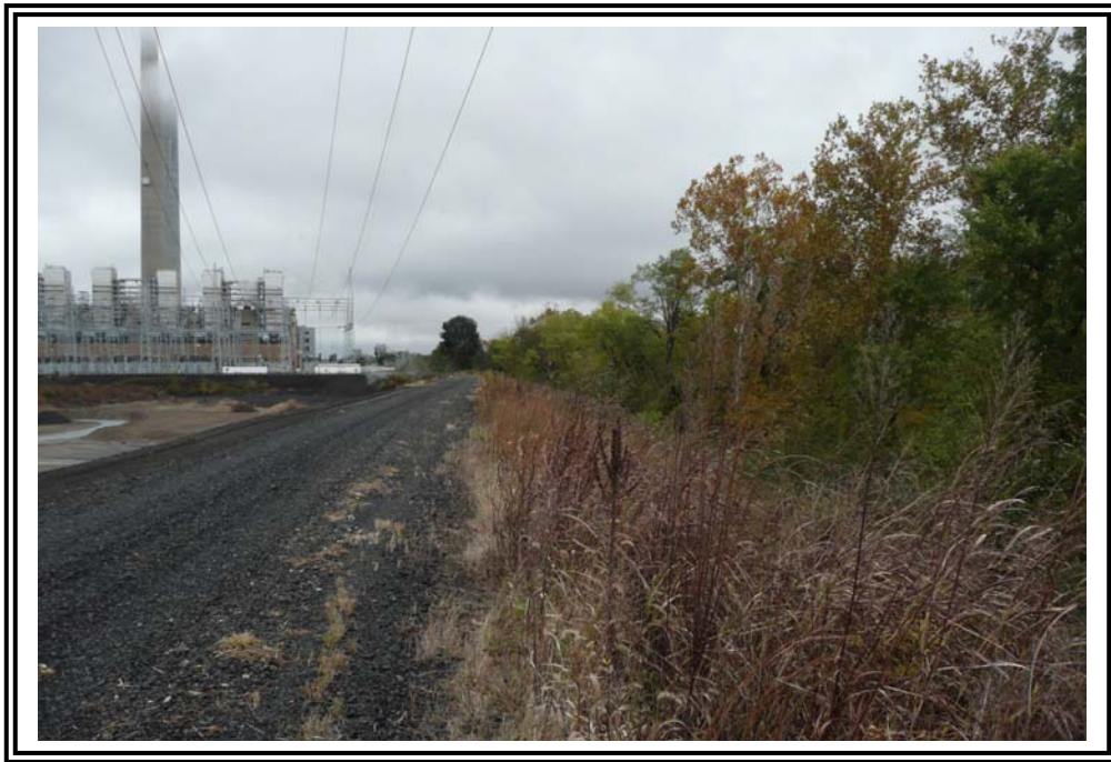
East dike crest and exterior slope, looking north.
