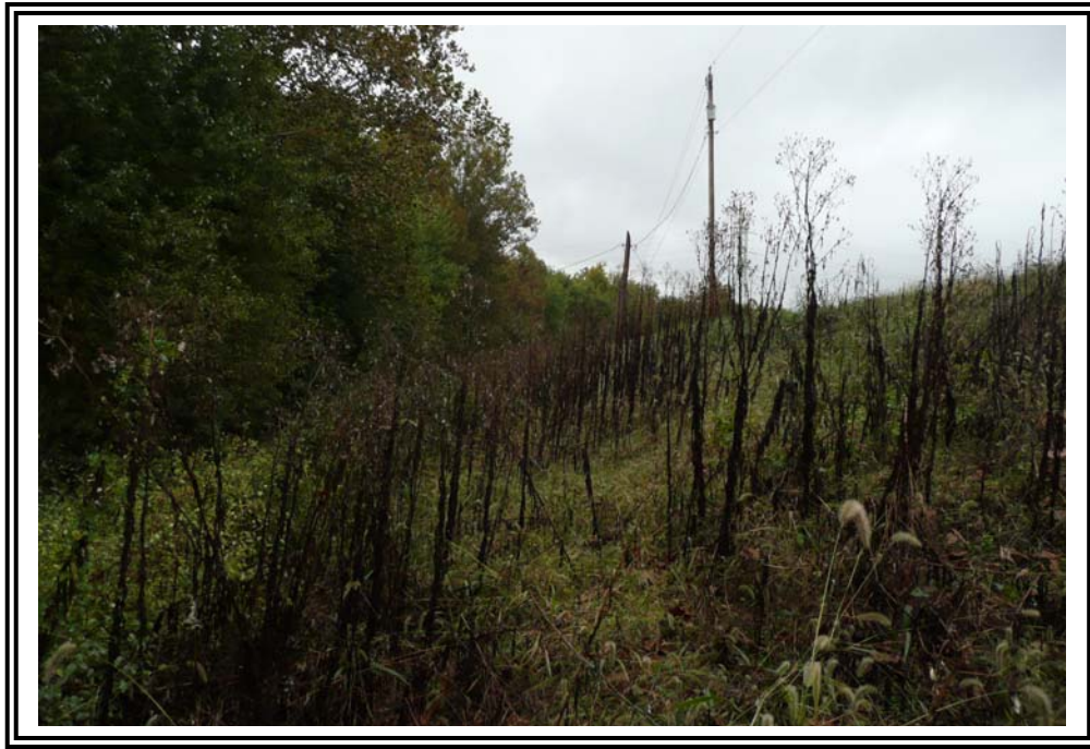
Exterior slope of south dike (Clearwater Pond section), looking west.
