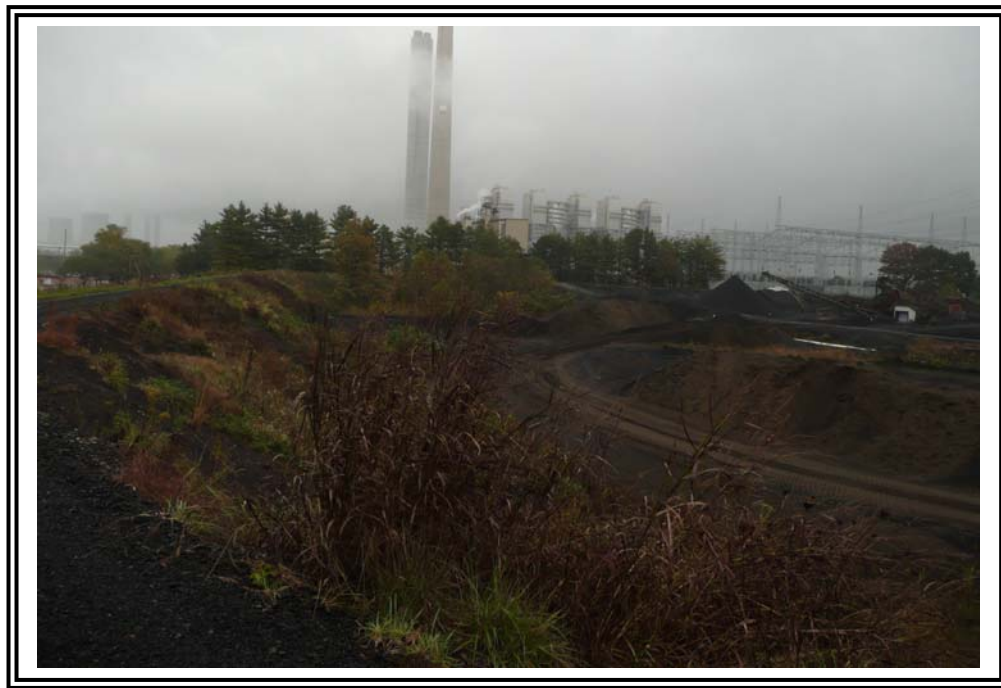
Interior slope of west dike and bottom ash processing area, looking north.
