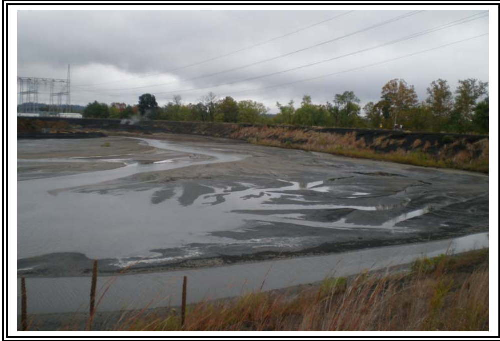
Looking west across Bottom Ash Pond at the east dike.
