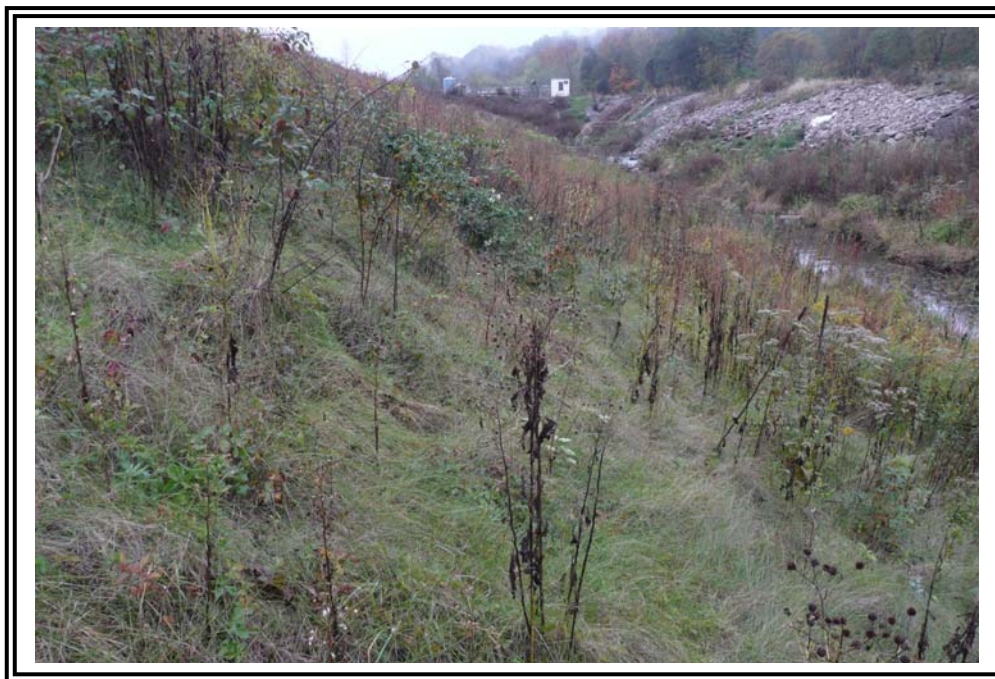
Exterior slope of west dike, looking south. Drainage feature at toe was collecting water during site visit.
