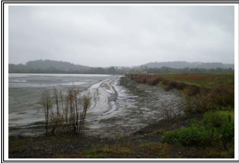
Interior slope of north dike, looking northwest.
