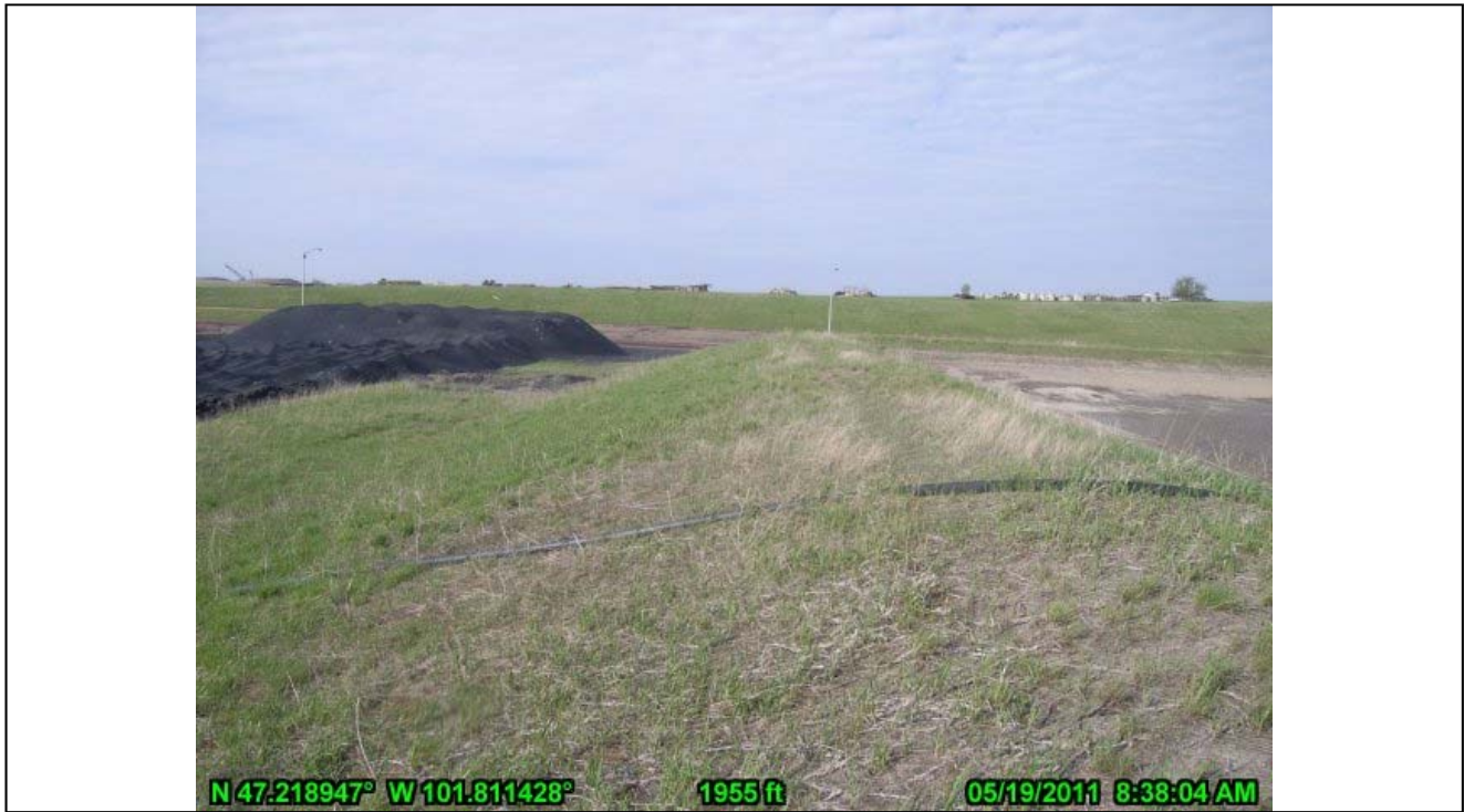
19-Nelsen Pond Southeast Landside Embankment (looking SW)
