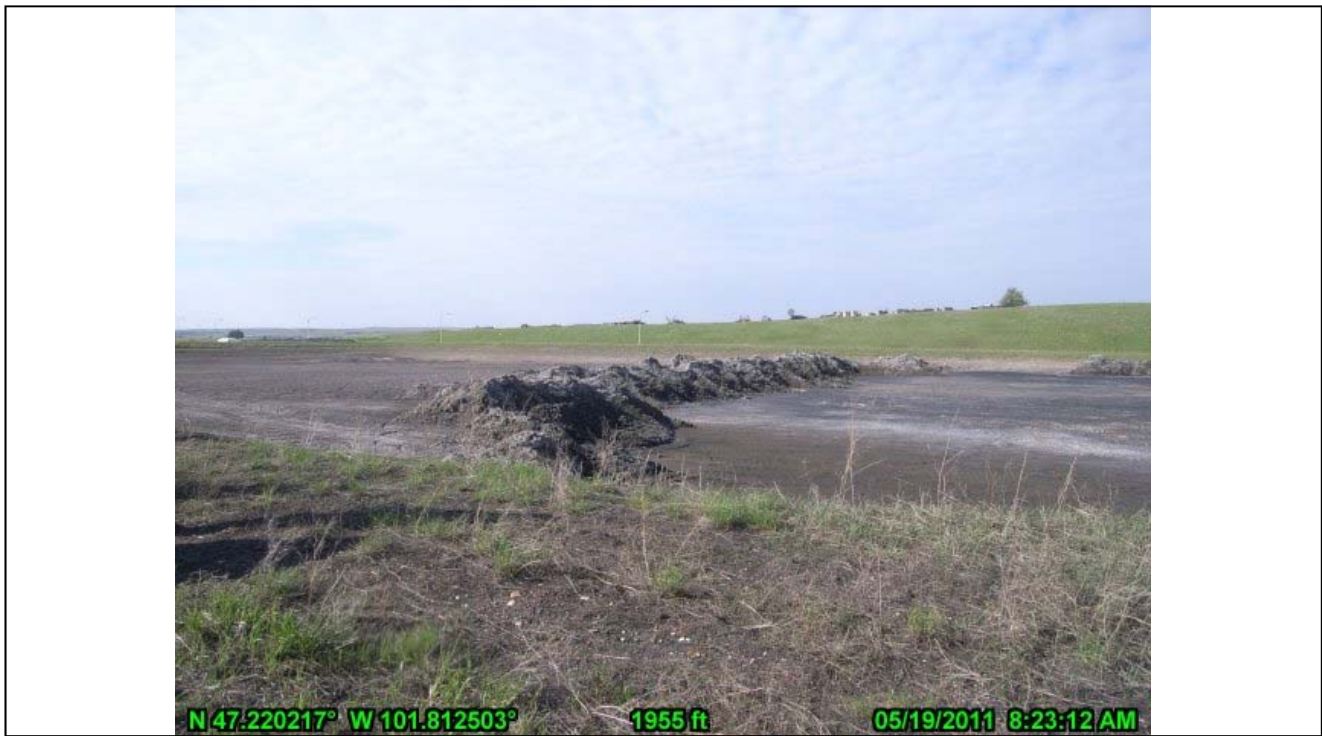
3-Nelsen Pond Dredging Activity (looking SW)
