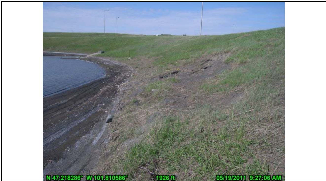
42-Ash Pond Northwest Waterside Embankment Scarping (looking SW)
