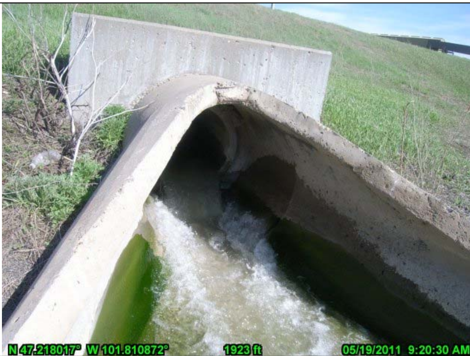
38-Ash Pond Inlet from the Sluice Pond
