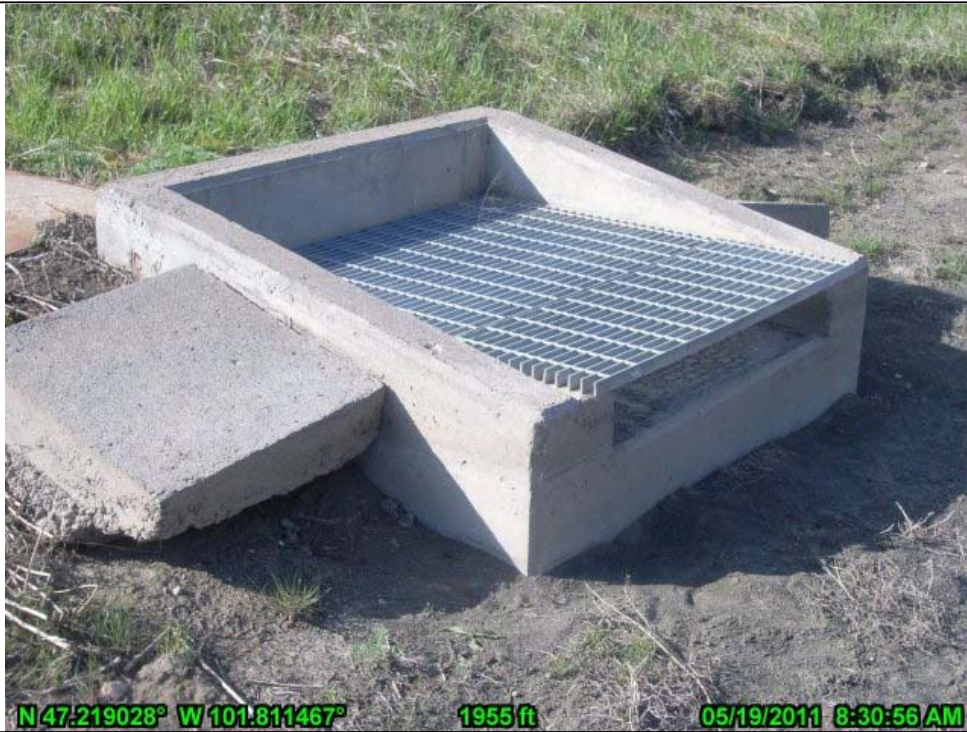
17-Nelsen Pond Overflow Inlet Structure
