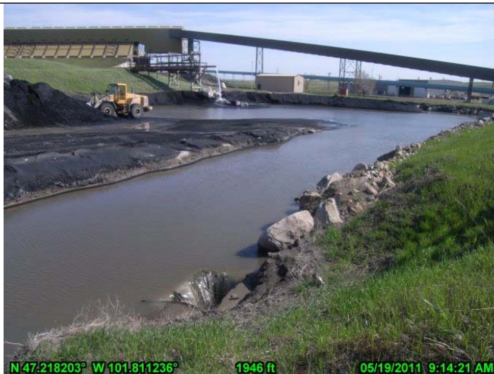
34-Sluice Pond 3'x4' Outlet Intake to Ash Pond without Trashrack (looking NE)
