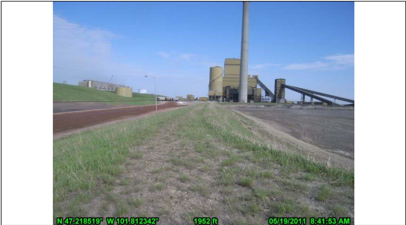
22-Nelsen Pond Southwest Embankment Crest (looking NW)
