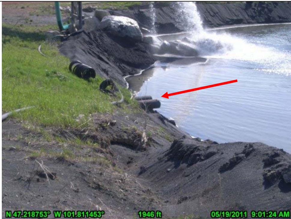
29-Outlet Pipes from Nelsen Pond (Steel Drain Pipe and Overflow Pipe)
