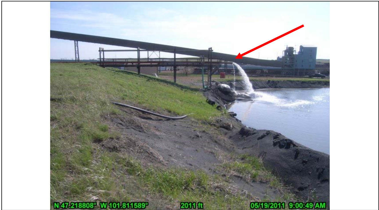
28-Sluice Pond Inlet and Northwest Waterside Embankment (looking NE)
