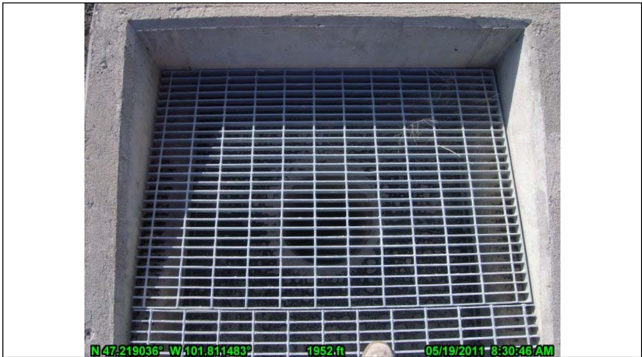
16-Nelsen Pond Overflow Structure and Trashrack
