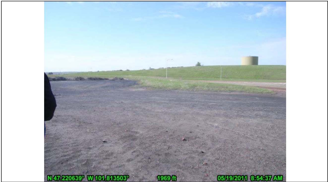
27-Nelsen Pond North Embankment and Dredging Ramp Entrance (looking W)
