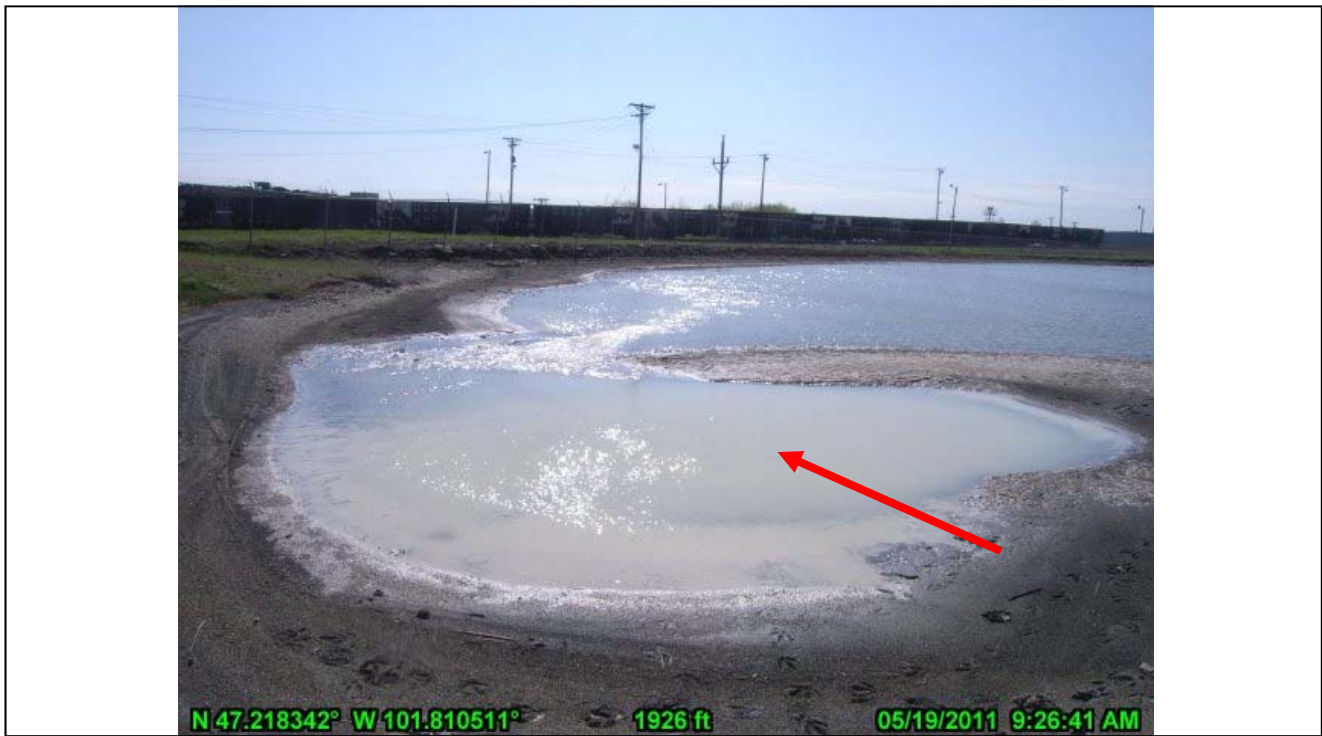
41-Ash Pond Inlet (underwater) from Plant Drains (looking SE)
