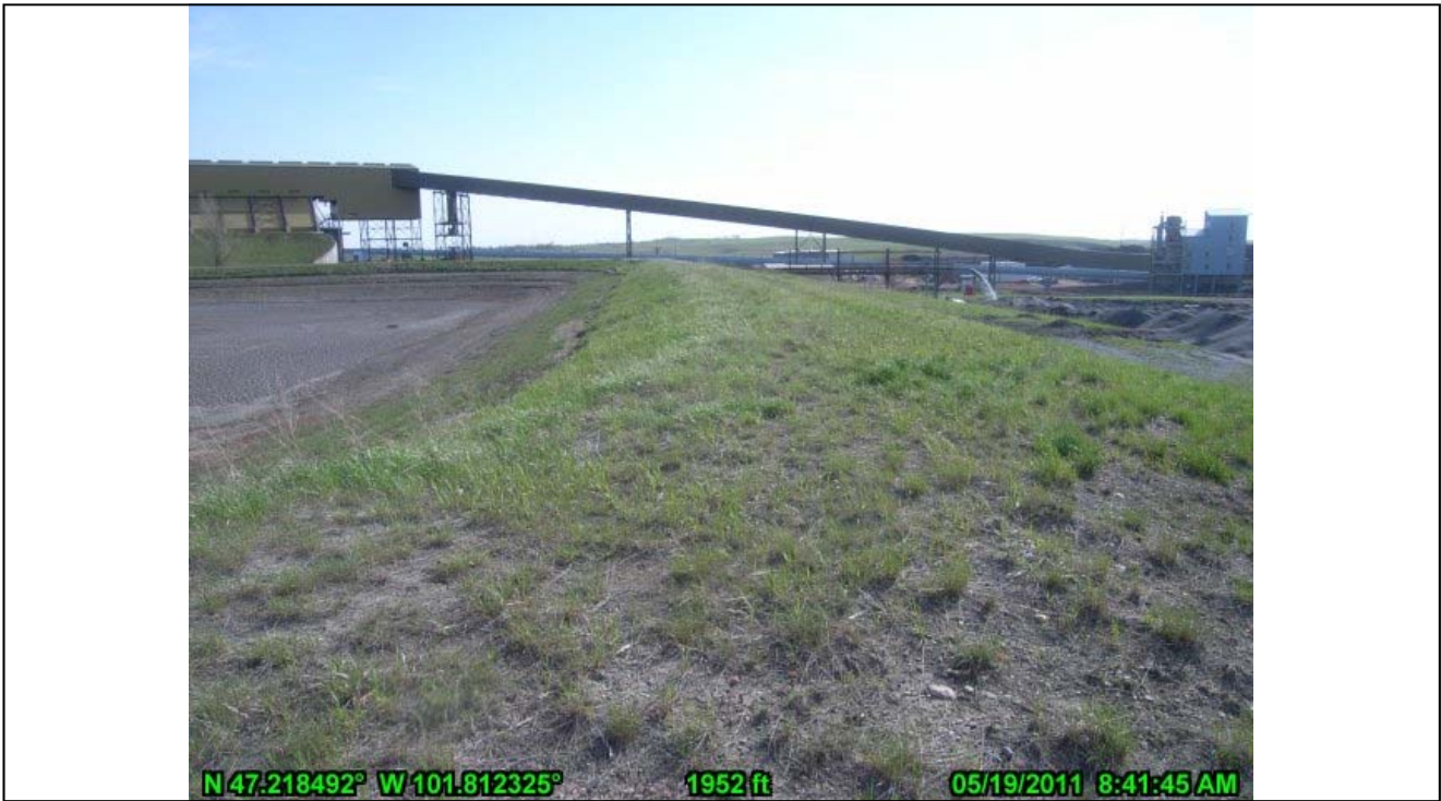
21-Nelsen Pond Southeast Waterside Embankment (looking NE)
