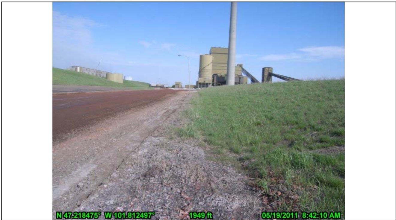
23-Nelsen Pond Southwest Landside Embankment (looking NW)
