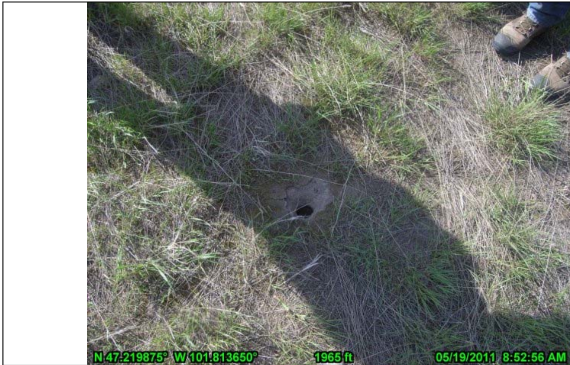
26-Nelsen Pond West Embankment Animal Burrow
