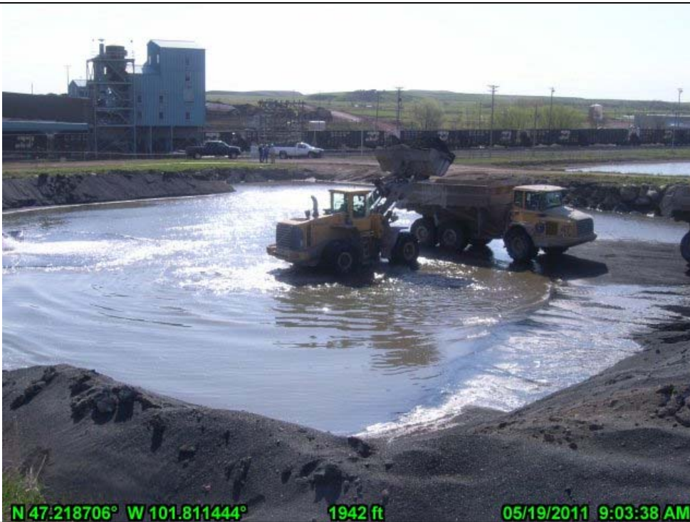
30-Slucice Pond Dredging (looking E)
