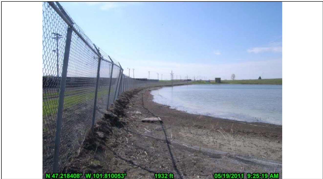
40-Ash Pond East Incised Embankment (looking S)
