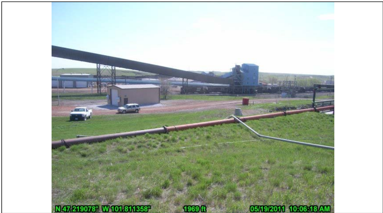
10-Down Gradient Area Adjacent to Max Height of Nelsen Pond (looking E)
