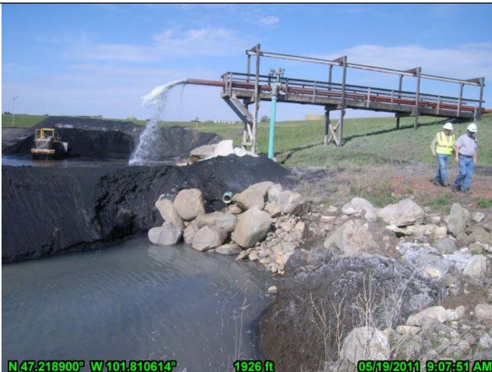
32-Sluice Pond Slag Inlet (red pipe) and Economizer Inlet (green pipe)
