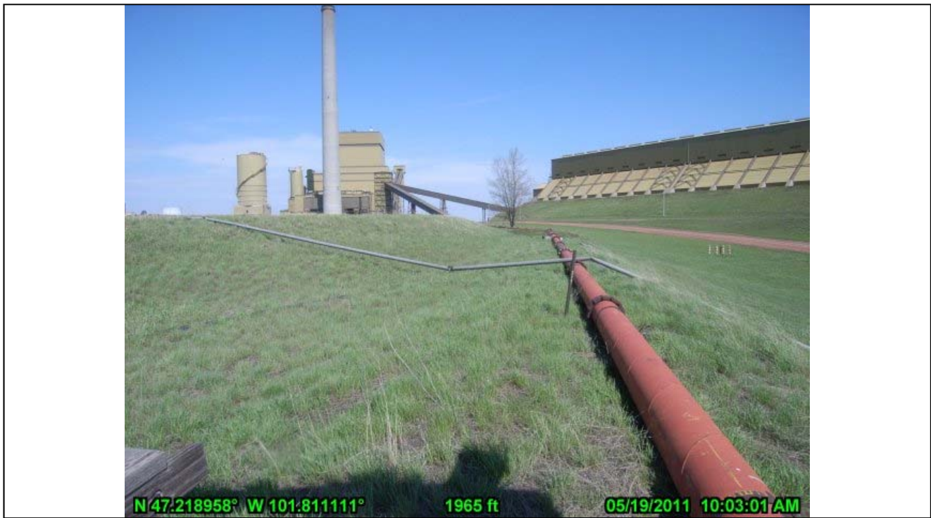
9-Nelsen Pond East Landside Embankment and Sluice Pipe (looking NW)
