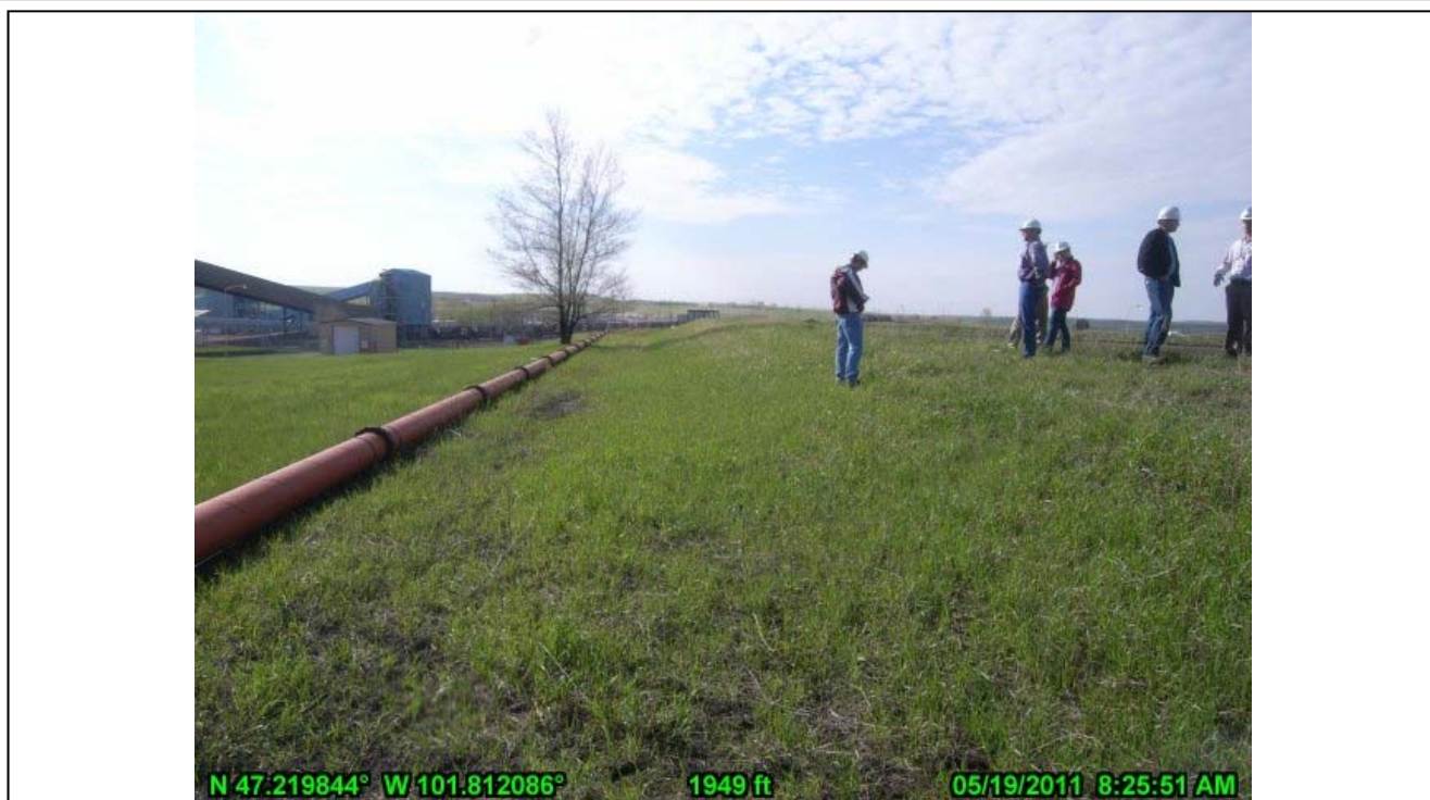
5-Nelson Pond Northeast Landside Embankment and Sluice Pipe (looking SE)
