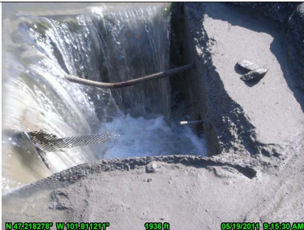
35-Sluice Pond 3'x4' Concrete Outlet Intake Structure to the Ash Pond without Trashrack
