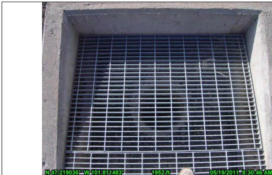
16-Nelson Pond Overflow Structure and Trashrack
