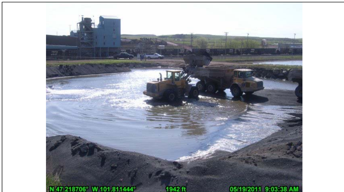
30-Sluice Pond Dredging (looking E)
