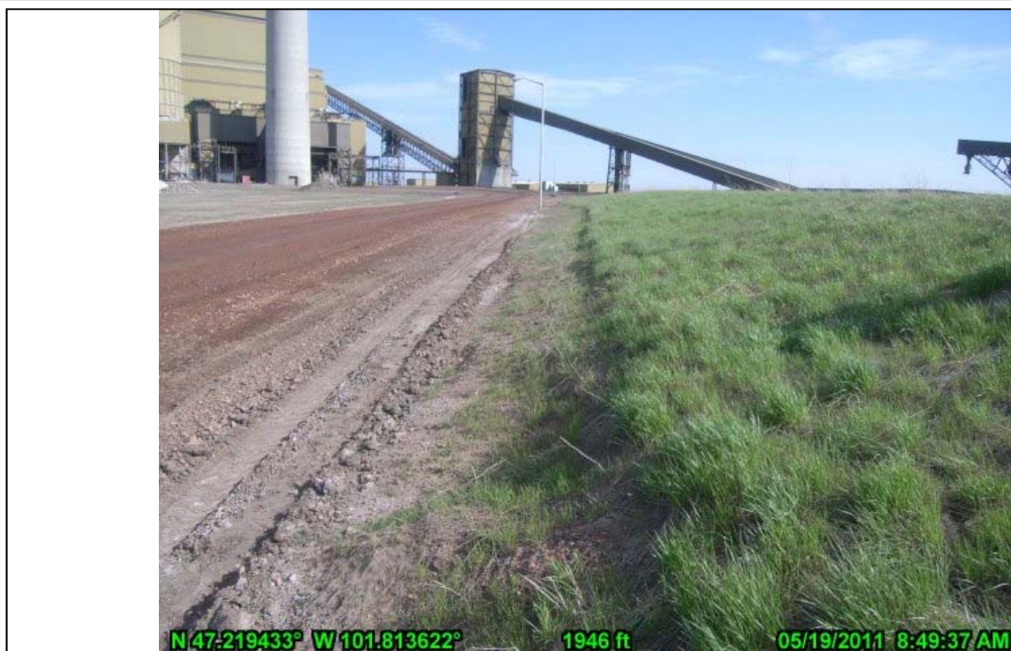
25-Nelson Pond West Landside Embankment Toe (looking N)
