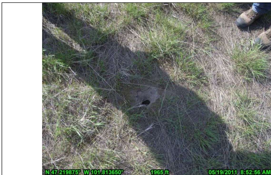
26-Nelson Pond West Embankment Animal Burrow
