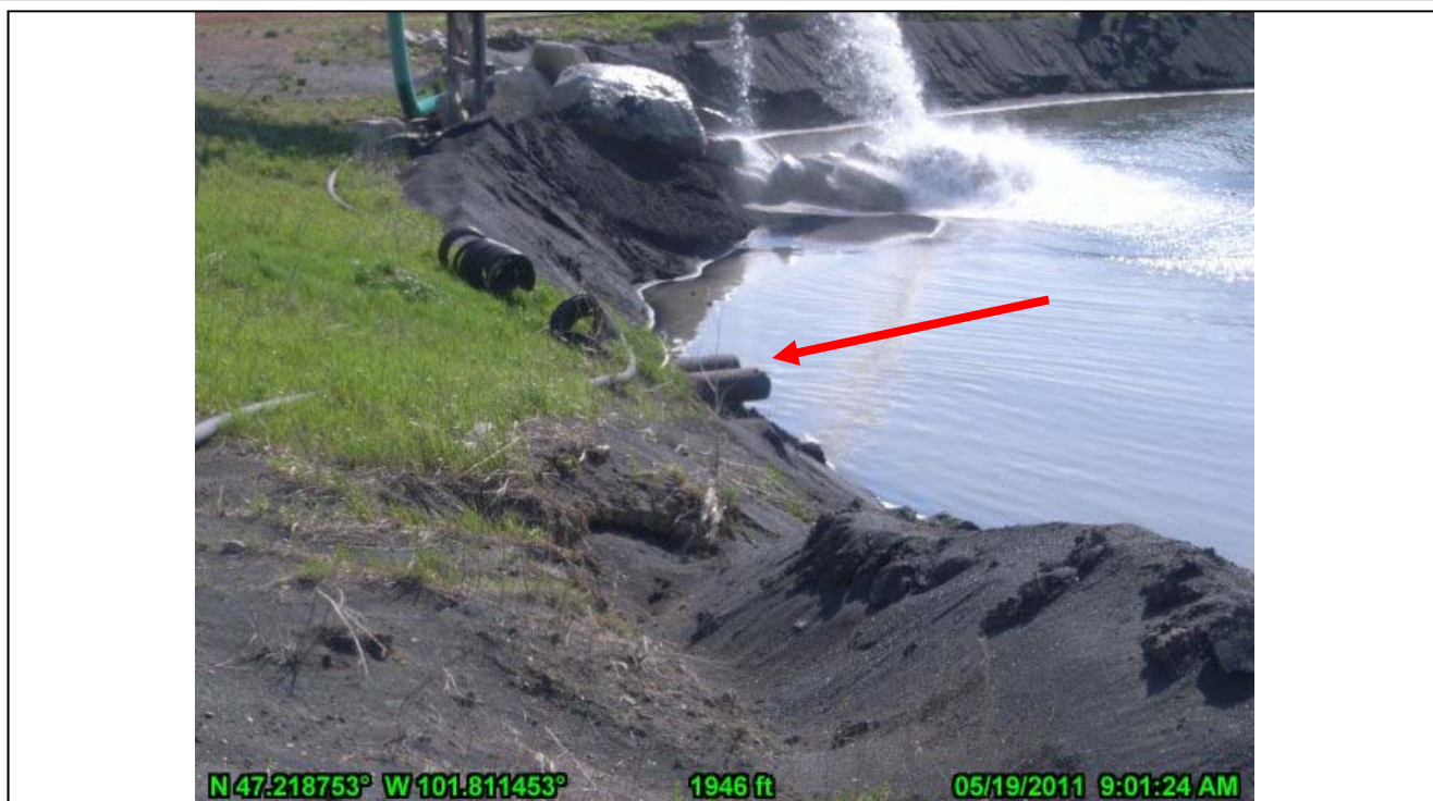
29-Outlet Pipes from Nelson Pond (Steel Drain Pipe and Overflow Pipe)
