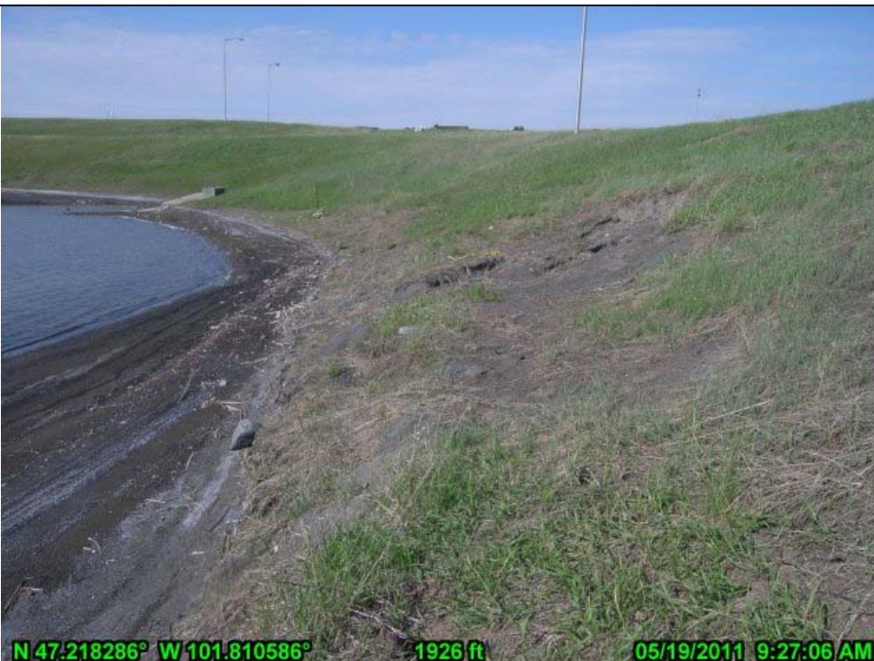
42-Ash Pond Northwest Waterside Embankment Scarping (looking SW)
