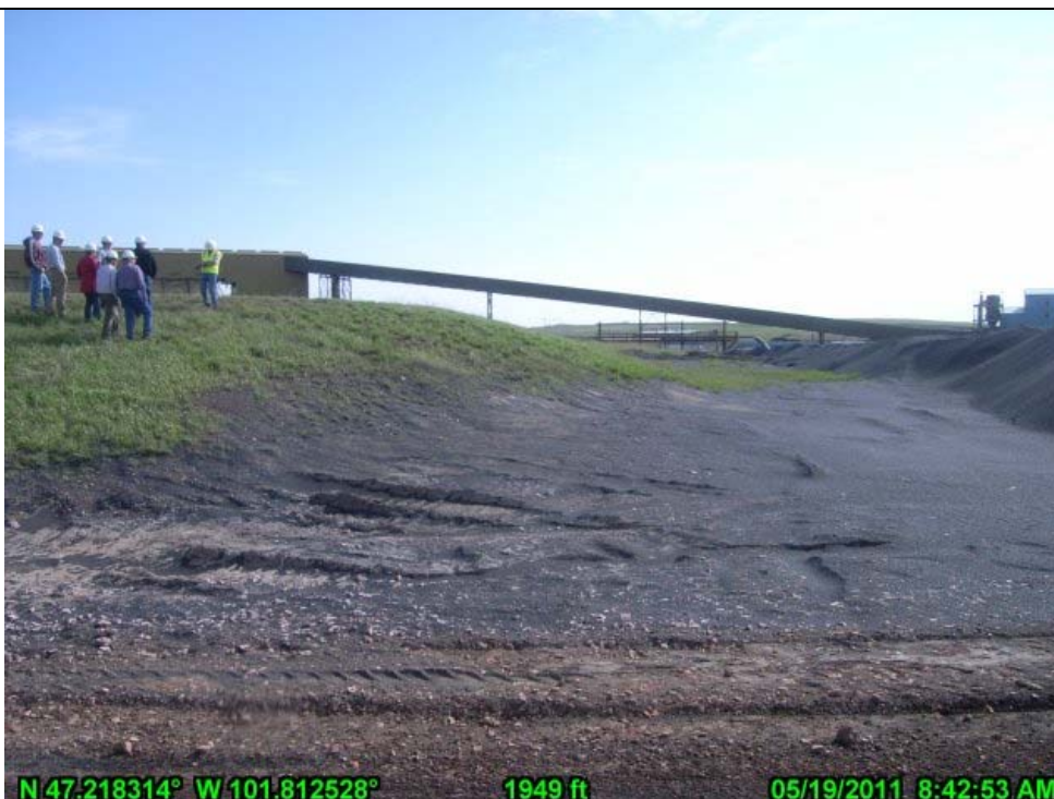
24-Nelson Pond Steepening of Southern Landside Embankment Corner (looking E)
