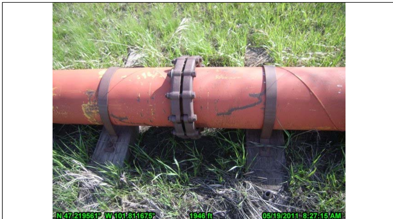
6-Sluice Pond Sluice Pipe
