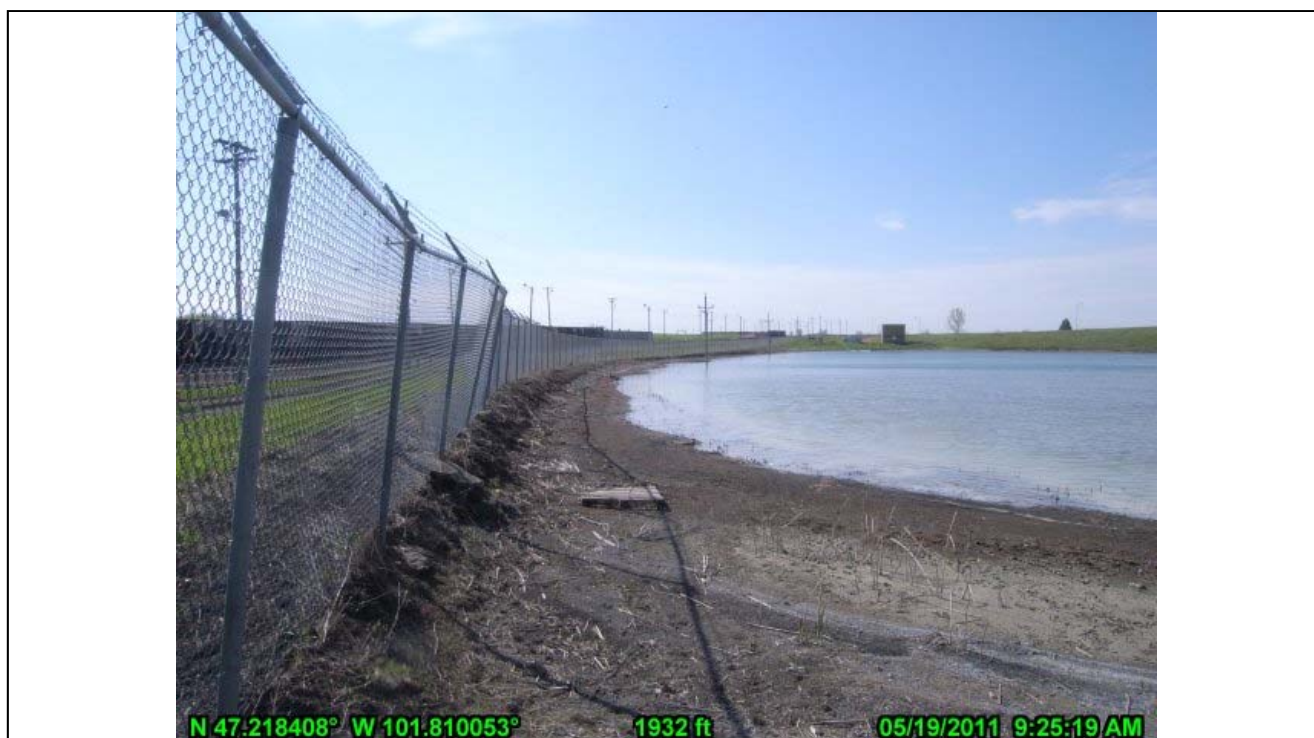
40-Ash Pond East Incised Embankment (looking S)
