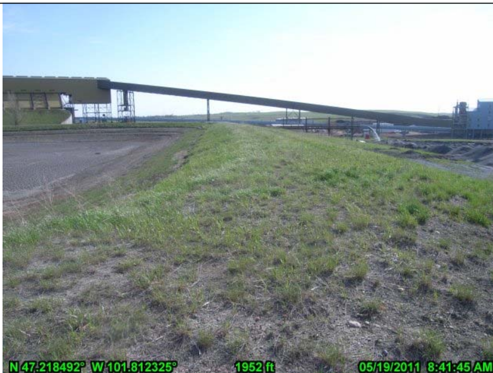
21-Nelson Pond Southeast Waterside Embankment (looking NE)
