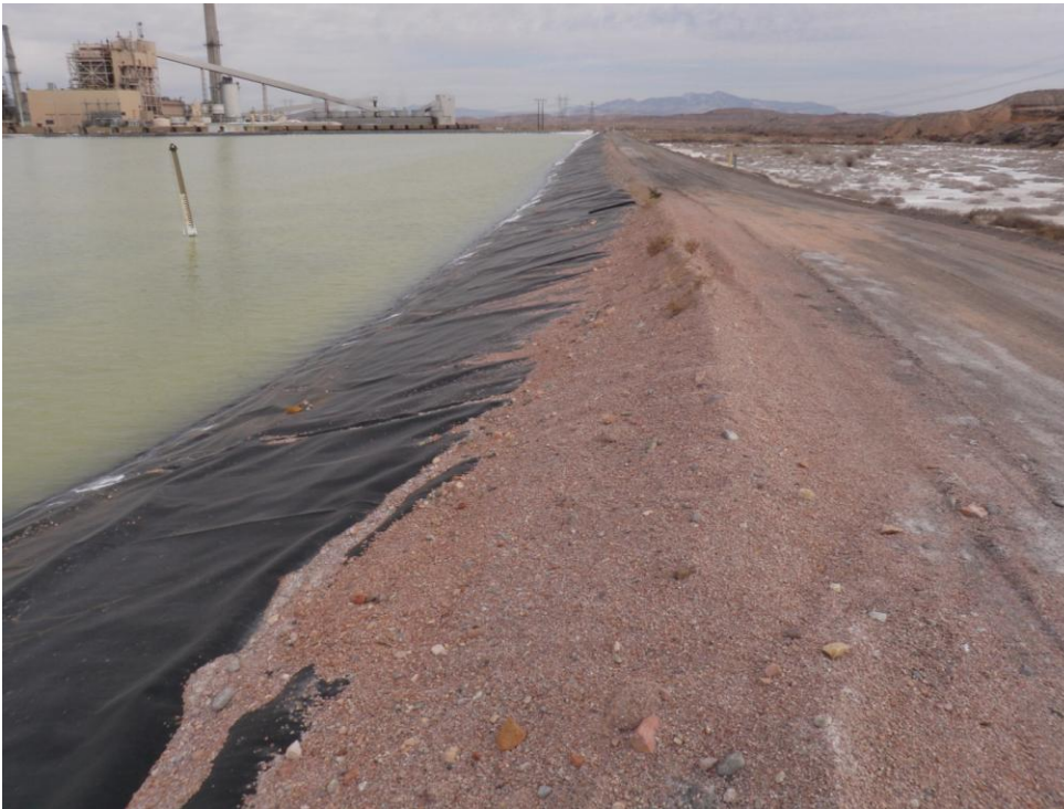
Photo 21: Looking east. Pond E1 south dike - HDPE liner and staff gage.
