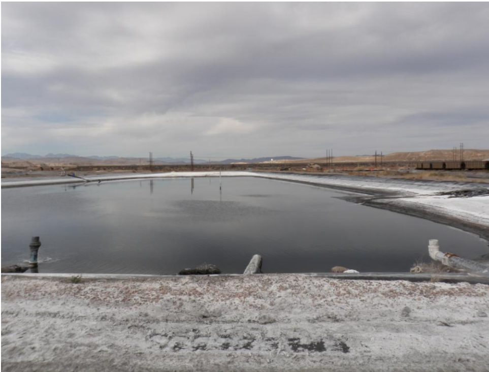
Photo 7: Looking northwest. Pond F from divider dike. Inlet on left.
