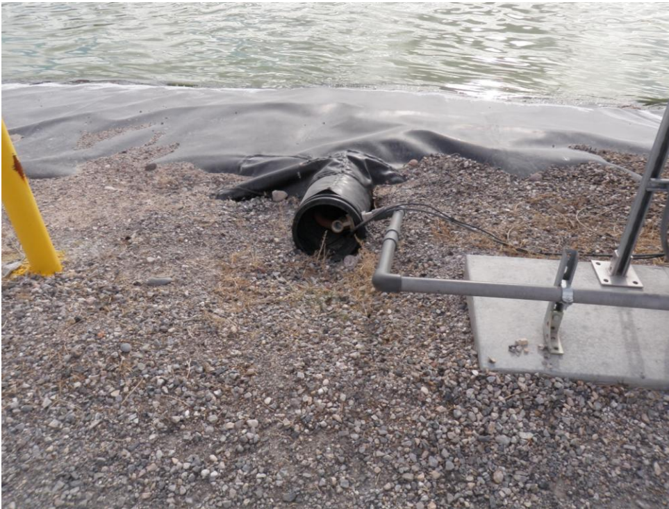
Photo 31: Typical interstitial drain.
