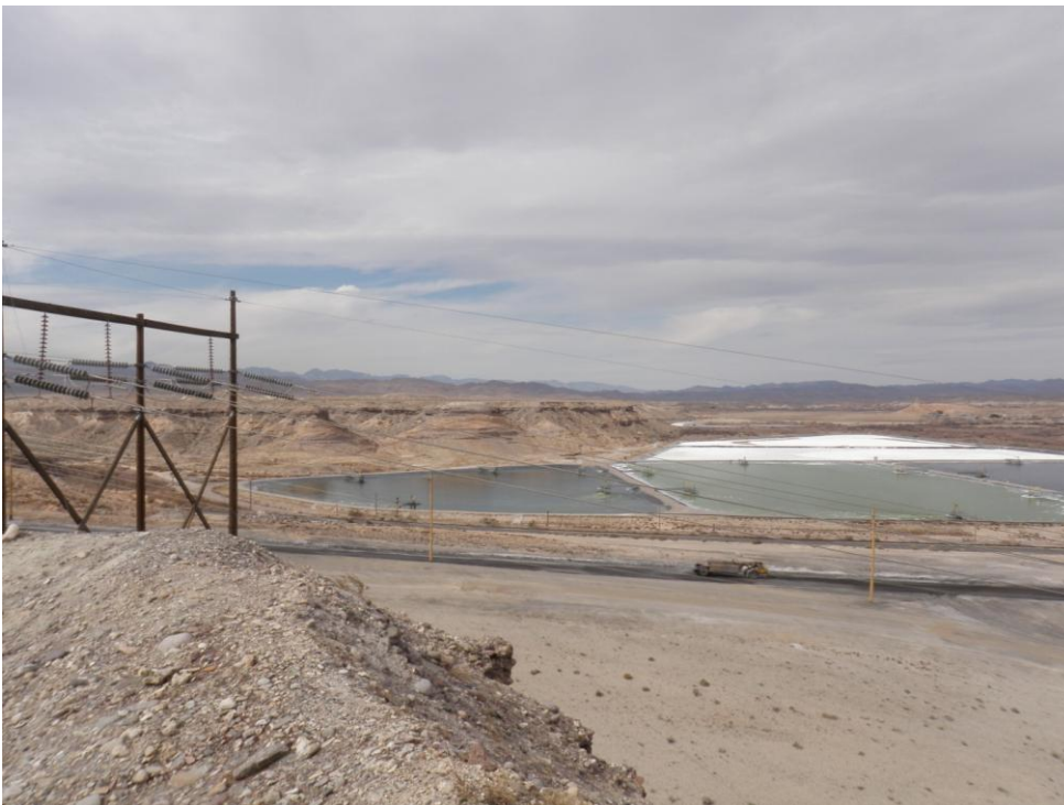
Photo 4: Site overview from Mesa Landfill Area. Looking west. From right to left, Pond B1 – B2 – B3. Ponds C1 and C2 in the background – white solids.
