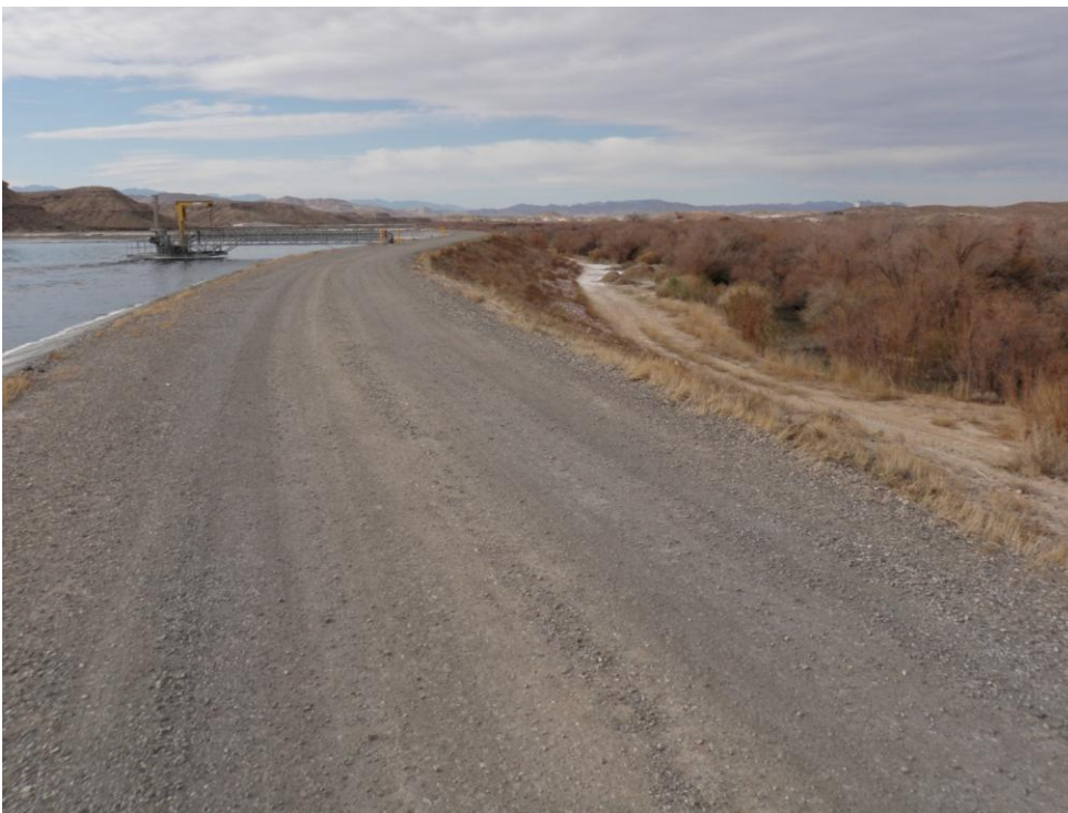
Photo 28: Looking northwest. Pond B1 north dike. Muddy River at right.
