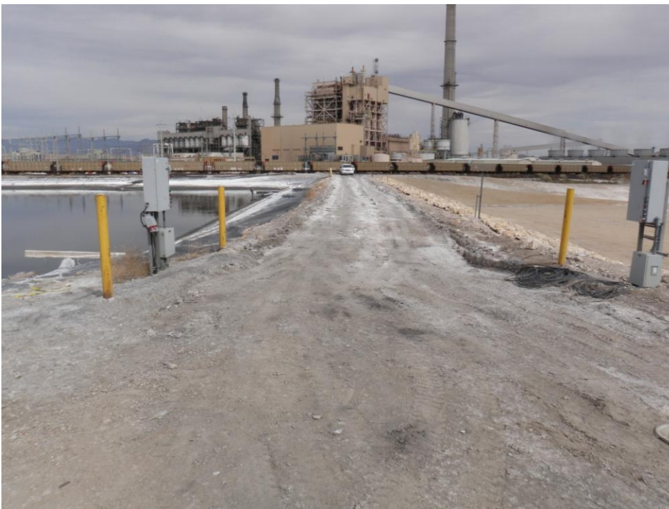
Photo 8: Looking northeast. Pond F on left. Former pond G on right.
