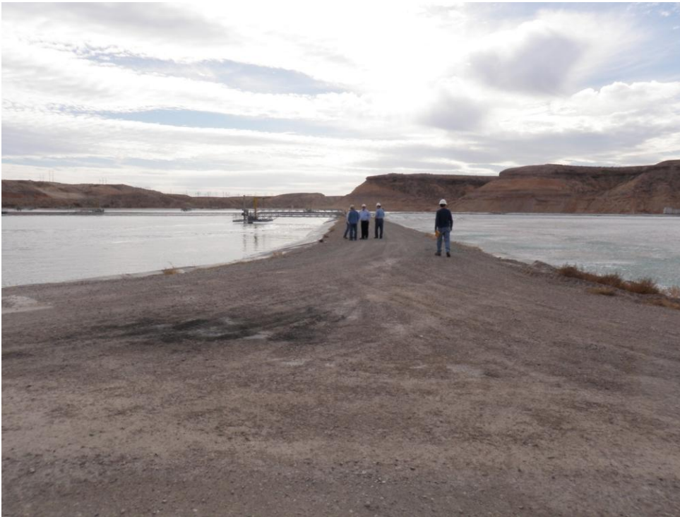
Photo 29: Looking southwest. Divider dike. Pond B1 on left. Pond C1 on right.
