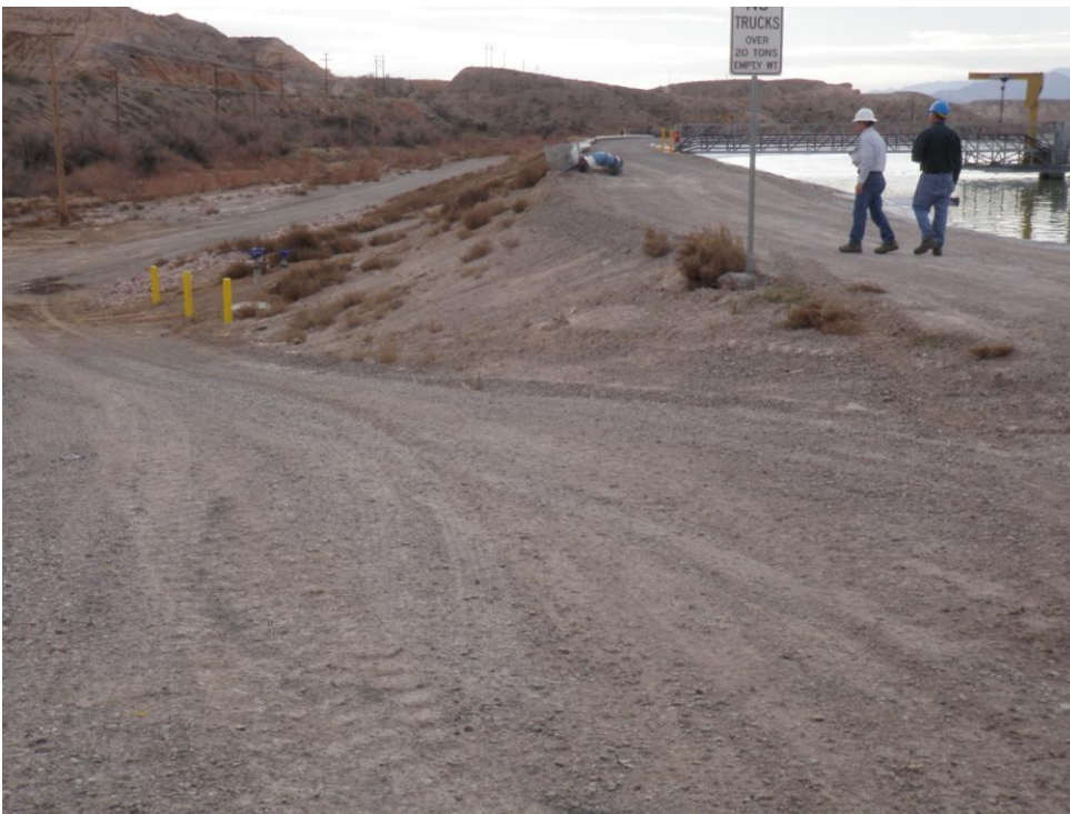
Photo 32: Looking southwest. Pond B2 east dike. Riprap at toe.
