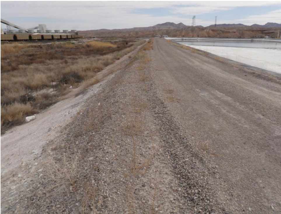
Photo 13: Looking southeast. North dike of Pond F. Typical soil cement slope protection. Muddy River located at left.
