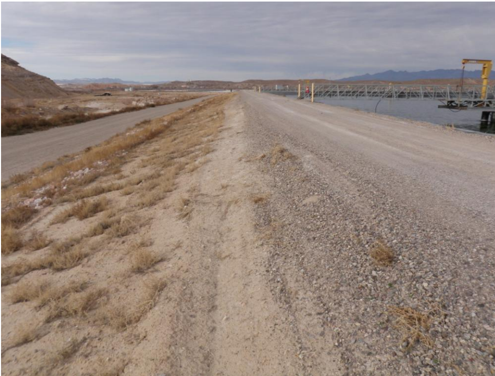
Photo 33: Looking north. Pond B3 west dike.
