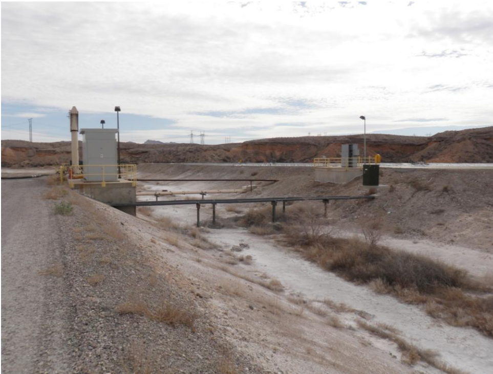
Photo 11: Looking east. From south dike of Pond F. Pumphouse at left and pipes to Ponds E1 and E2. The only pipes in service are the cream colored set in the background near the ground.
