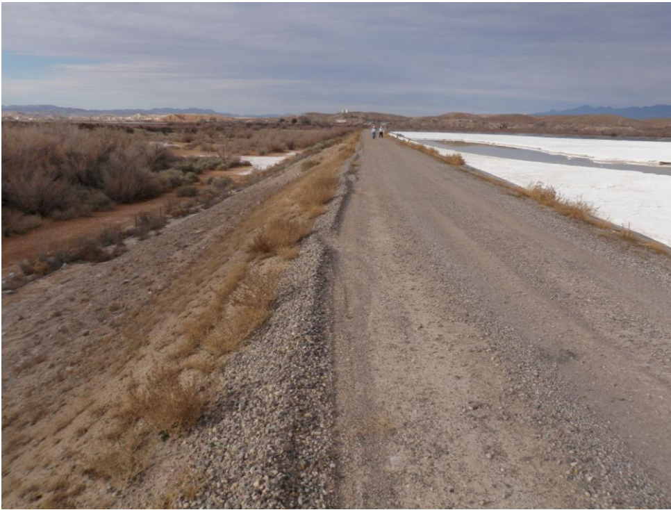
Photo 37: Looking north. Pond C2 west dike. Muddy River at left.
