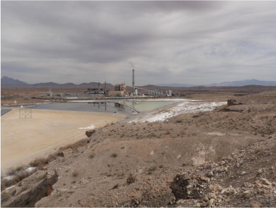
Photo 1: Site overview from Mesa Landfill Area. Looking northeast. Reid Gardner Generating Station in background. From right to left Pond E1 – E2 – former pond D.
