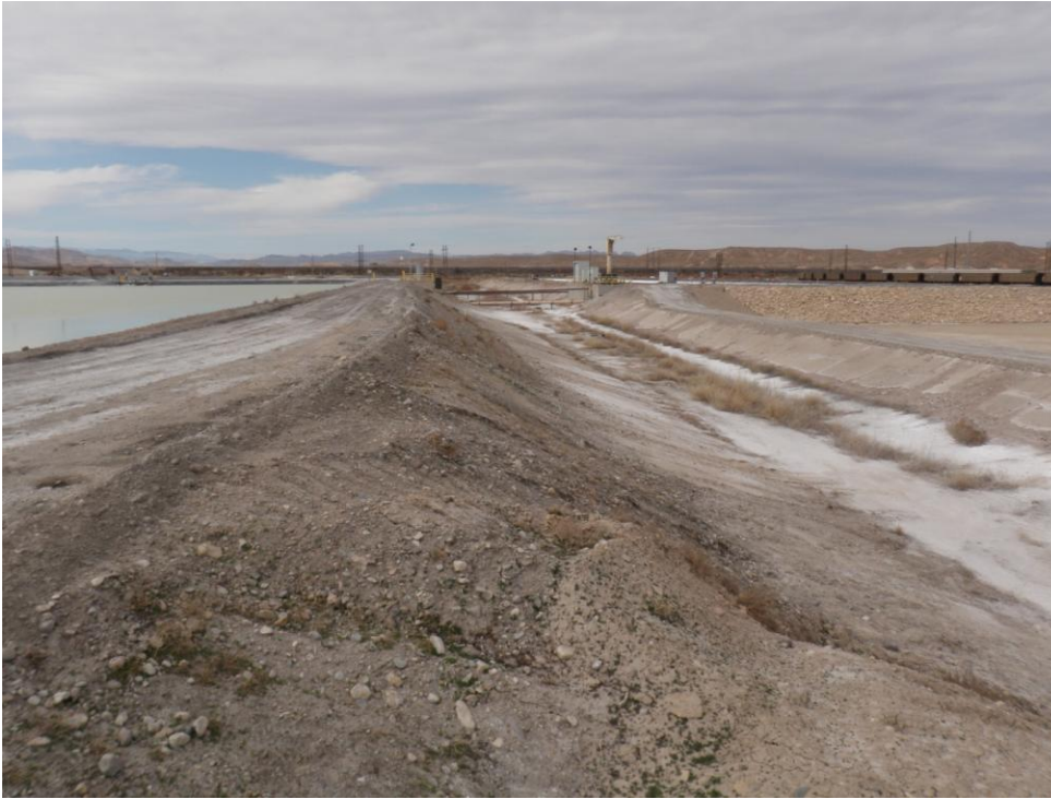
Photo 23: Looking northwest. Pond E1 east dike. Former Pond G on right with partially removed dike and rip rap slope protection on former divider dike with Pond F. Pipes connecting Pond F with Pond E1 in the center-background.
