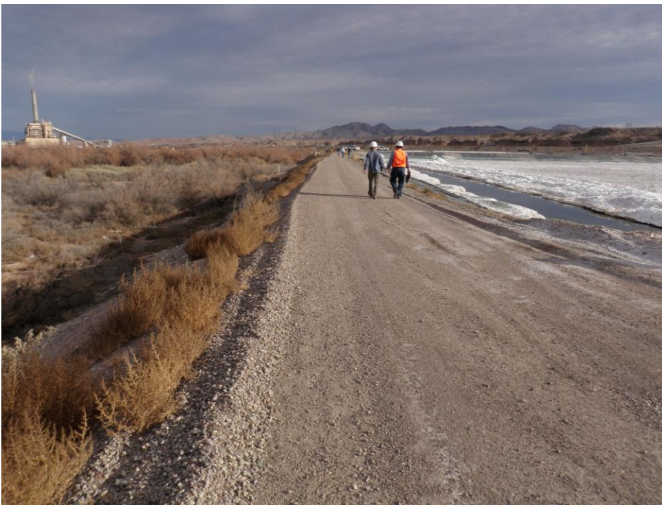
Photo 40: Looking southeast. Pond C1 north dike.
