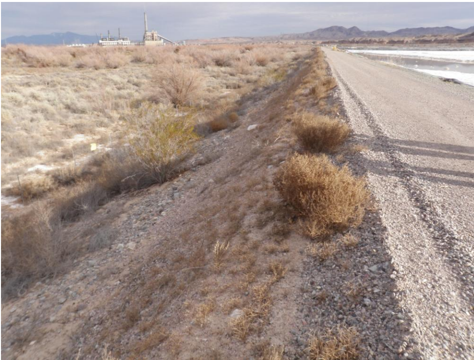
Photo 38: Looking southeast. Pond C2 north dike. Shrub growing on slope near toe.
