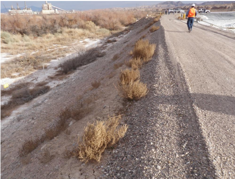
Photo 42: Looking southeast. Pond C1 north dike.
