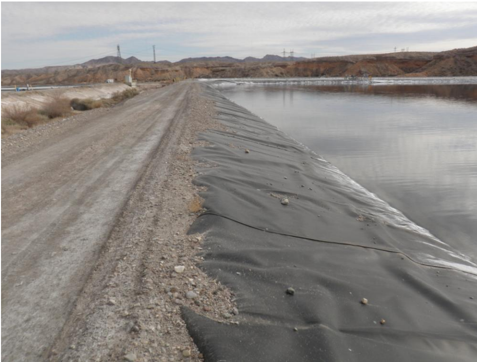
Photo 27: Looking southeast. Pond E2 east dike.
