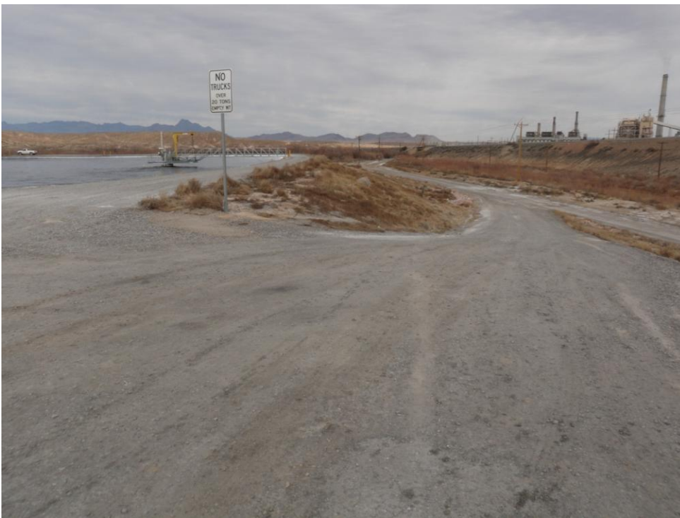
Photo 30: Looking northeast. Pond B1 east dike.
