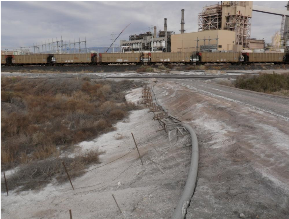
Photo 16: Looking northeast. Piping from Reid Gardner Station to Pond F.
