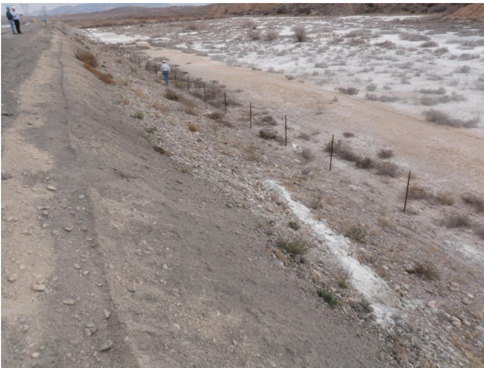
Photo 22: Looking east. Pond E1 south dike.
