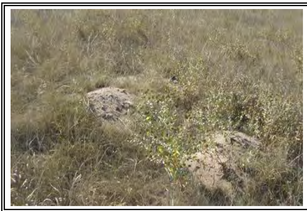
Animal burrows on downstream embankment of North Dam.
