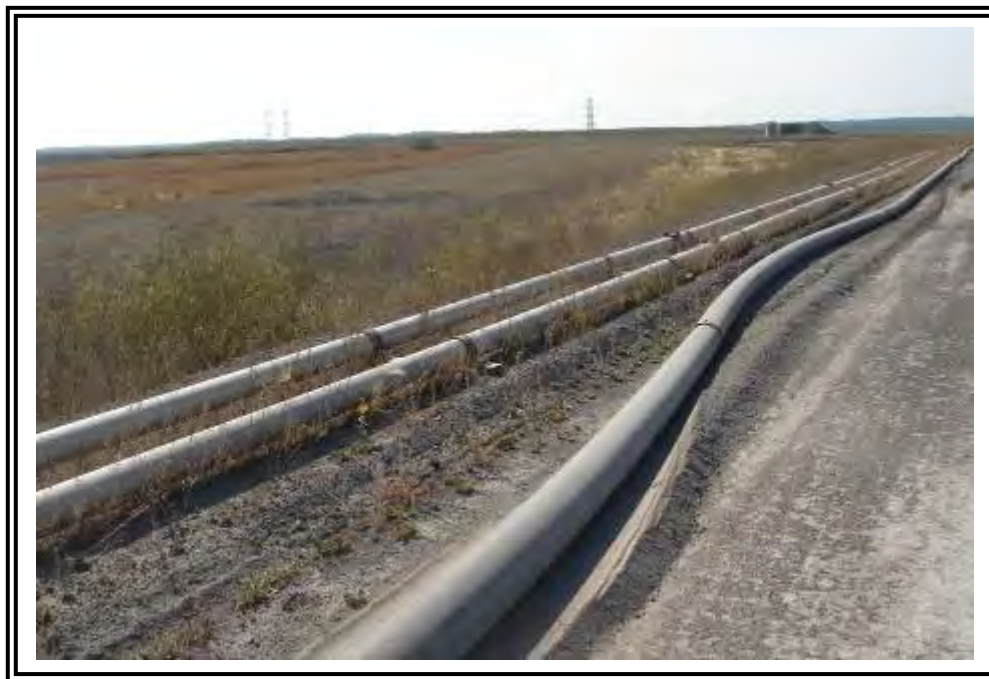
Partially filled portion of Pond 2, facing southwest.
