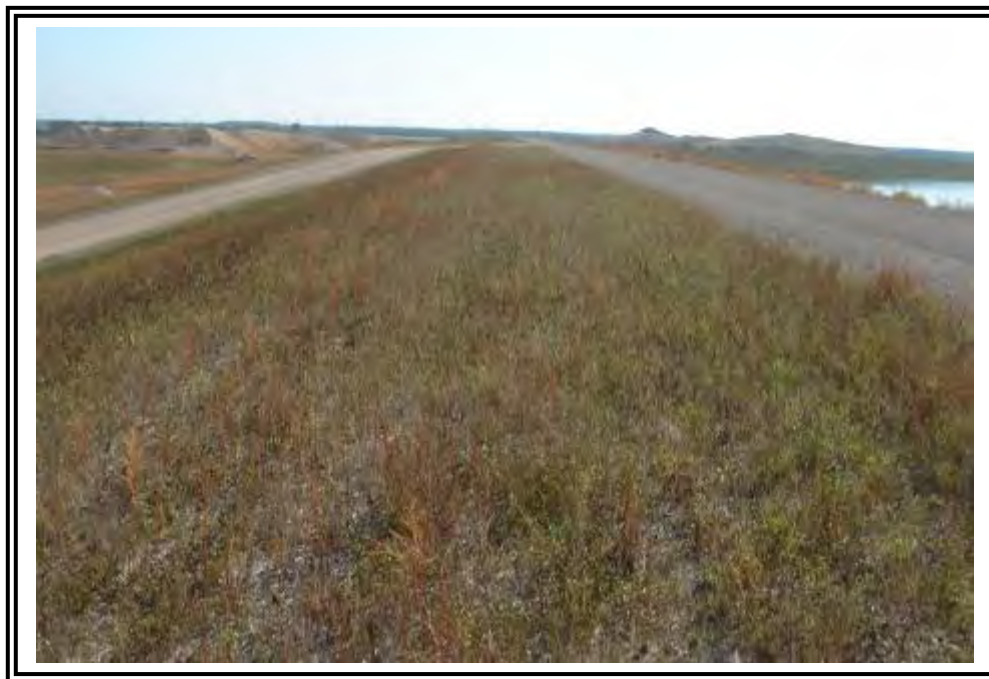
Downstream slope of East Embankment, looking south.
