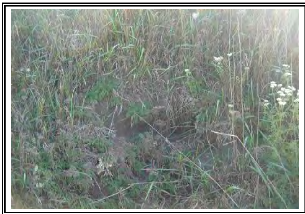
Erosion observed at mid-height on downstream embankment slope of the West Dam.
