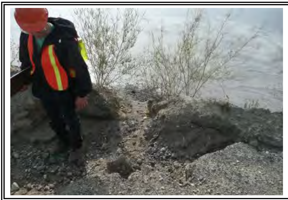
Erosion of Pond No. 2 upstream embankment, facing west.
