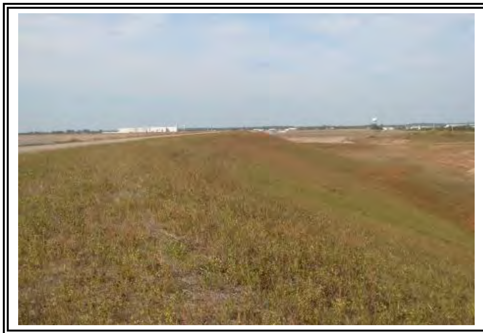
Downstream slope of East Embankment, facing north.
