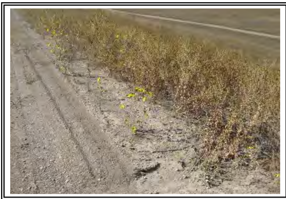
Minor erosion at top of downstream embankment of North Dam, facing northwest.
