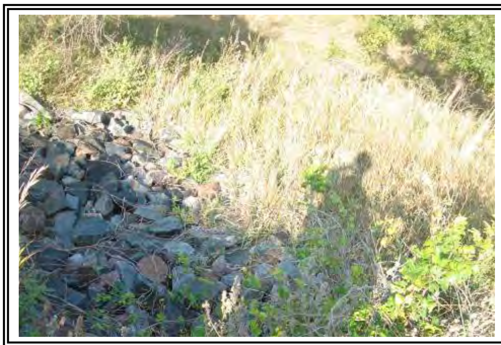
Drainage along downstream embankment slope of South Dam.
