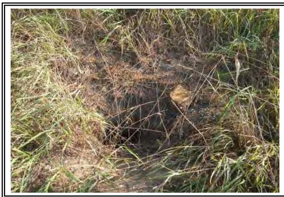
Animal burrow on embankment slope of South Dam.
