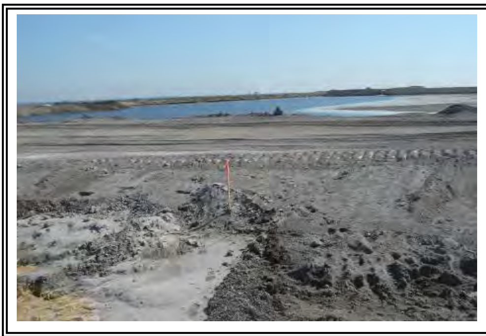
Active portion of pond, facing south.
