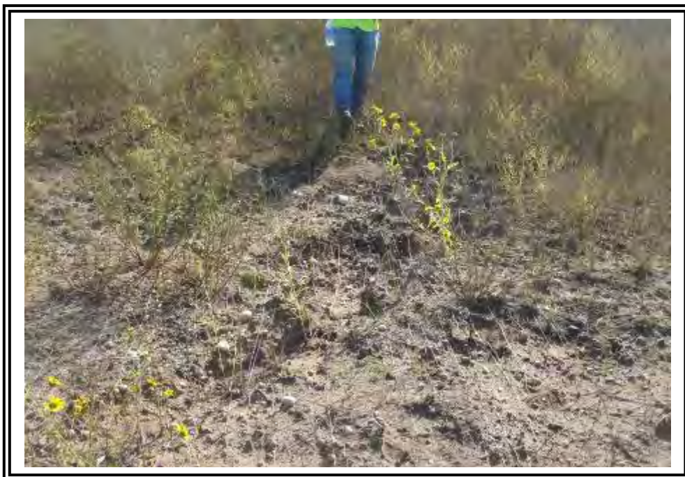
Minor erosion on downstream embankment slope of North Dam.
