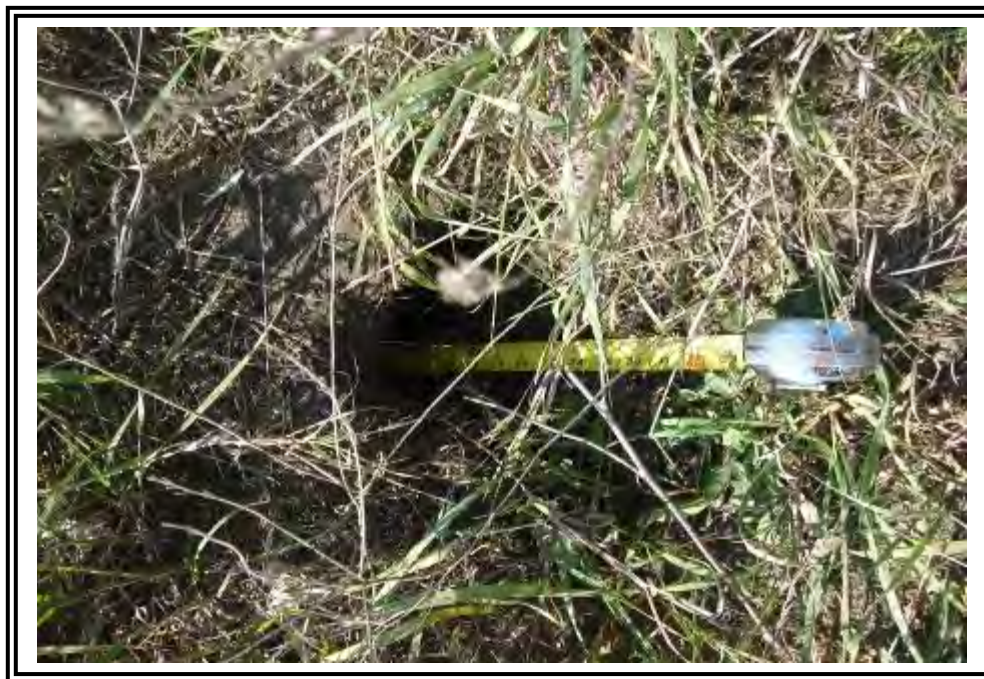
Animal burrow in East Dam near groin. Burrow was measured to be approximately 2'-4" deep from the ground surface.
