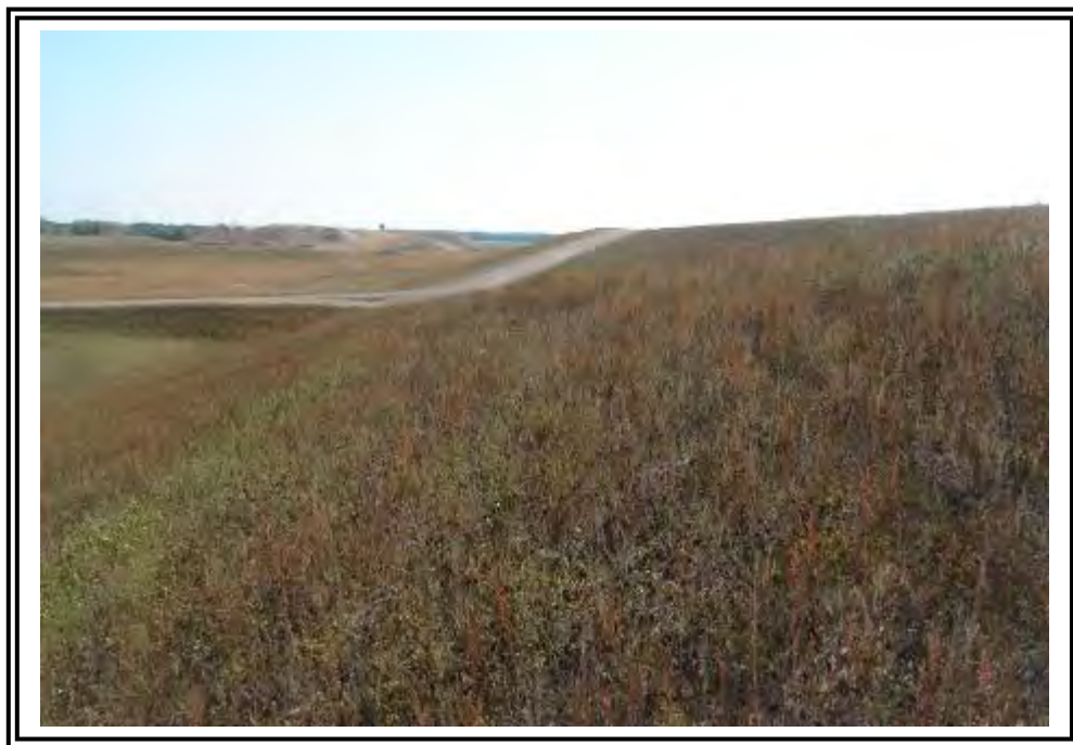
Downstream slope of East Embankment, facing south.
