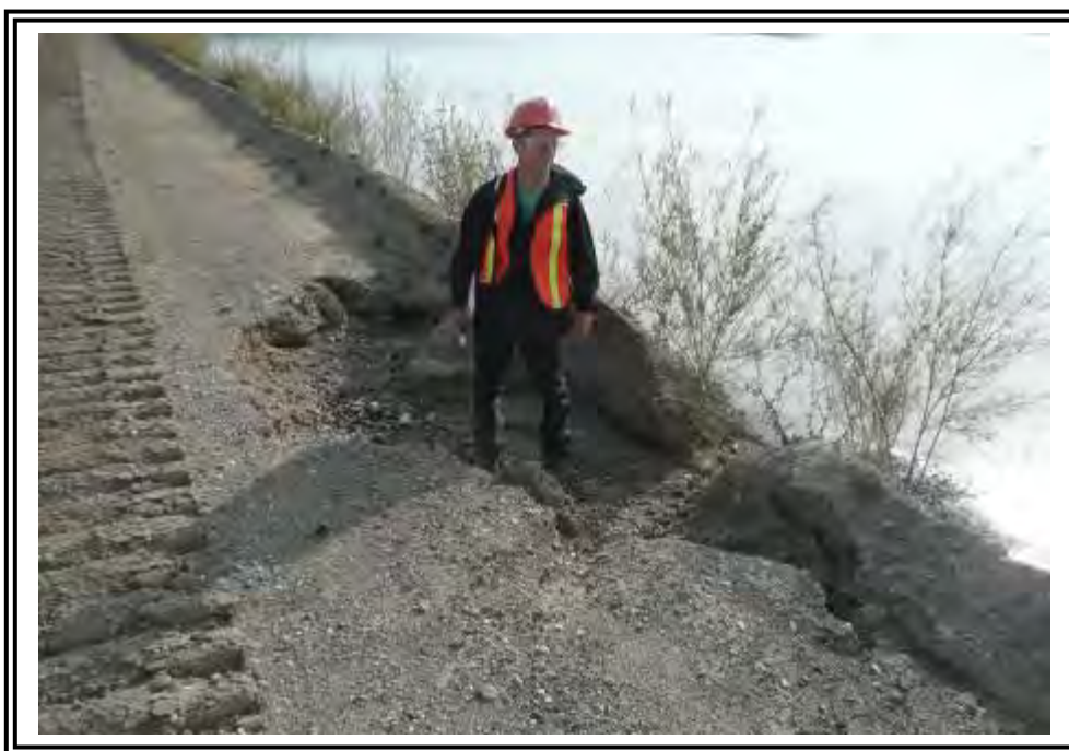
Erosion of Pond No. 2 upstream embankment, facing south west.
