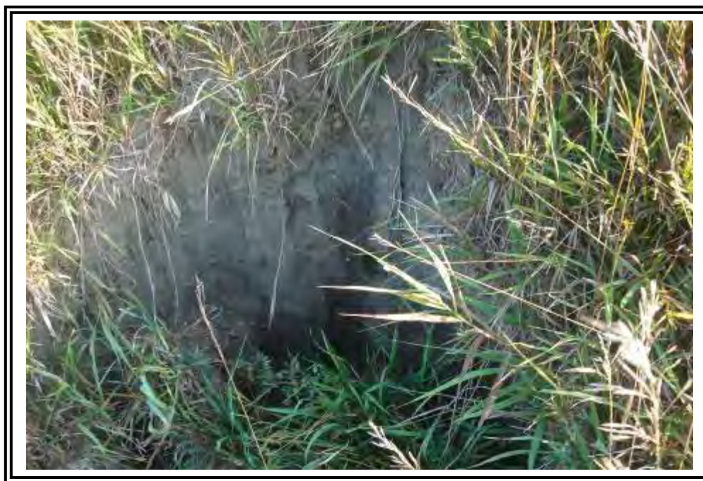
48-inch diameter, 3-foot deep sink hole near crest of South Dam.
