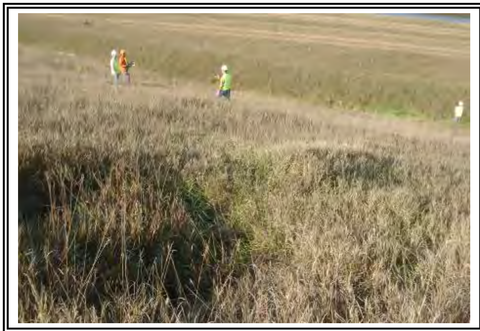
Downstream embankment slope of West Dam, facing west. Note surface undulations observed.
