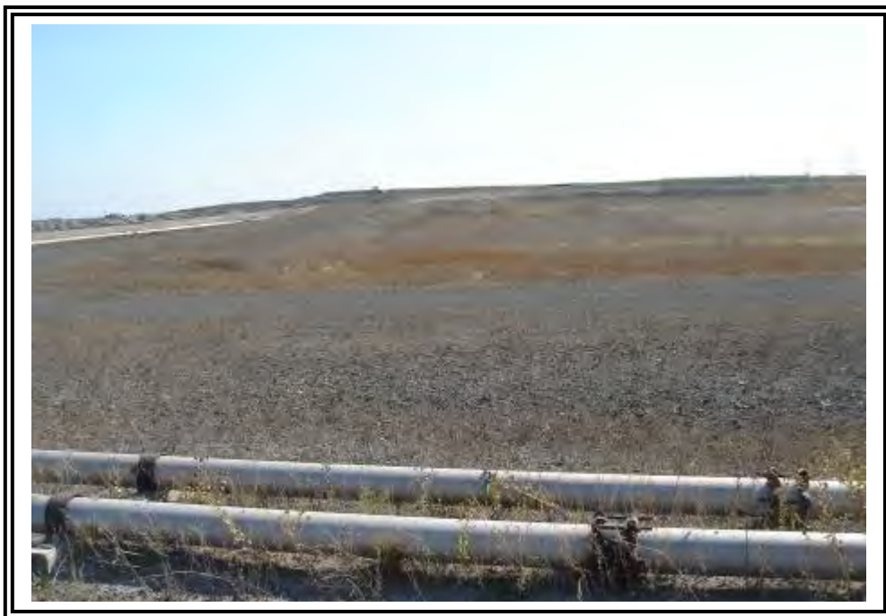
Partially filled portion of Pond 2, facing south.
