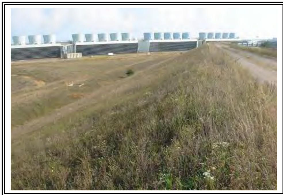
Downstream embankment slope West Dam, facing northeast.
