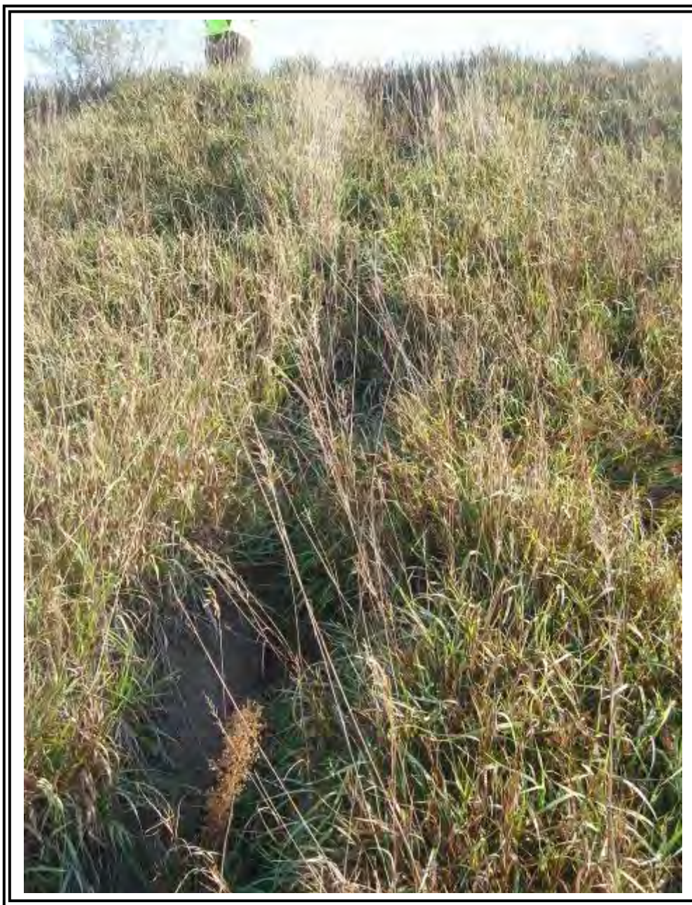
Erosion observed on downstream embankment slope of South Dam.
