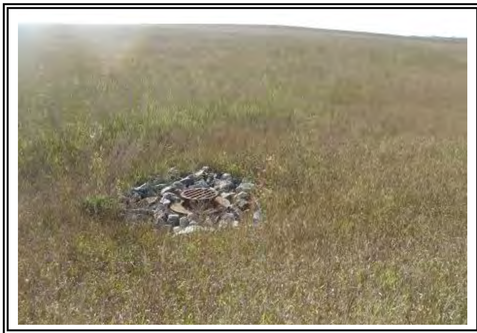
Drainage inlet in Pond 1 cap, looking east.
