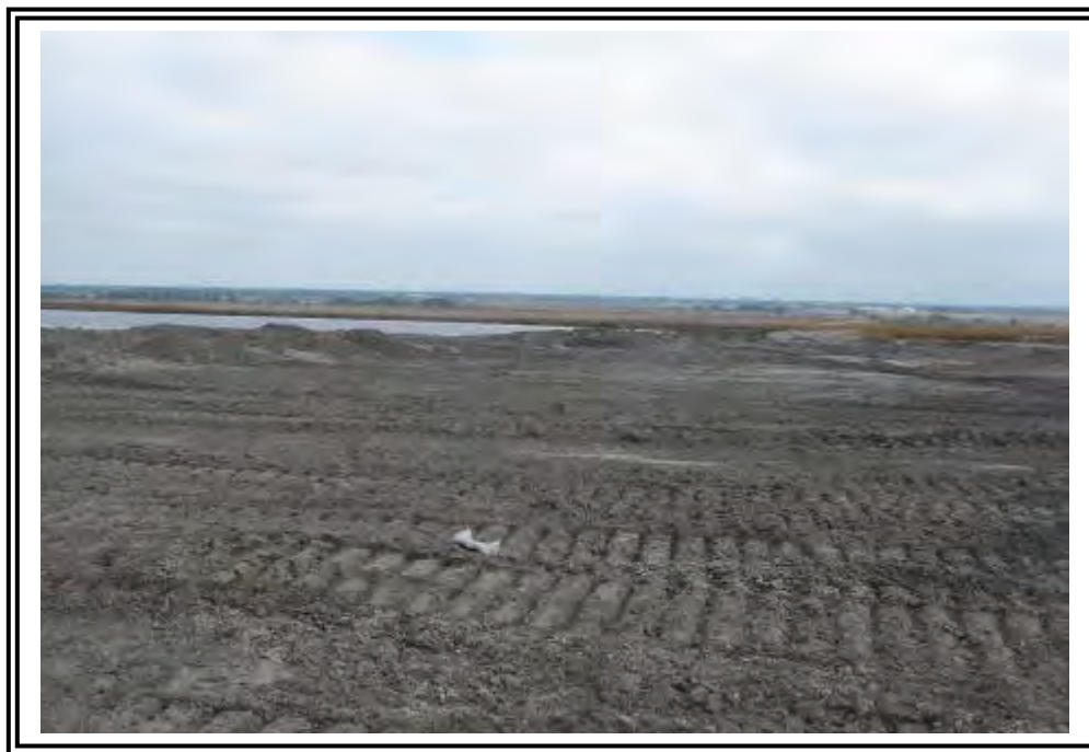
Pond 2 filling operations, facing northeast.
