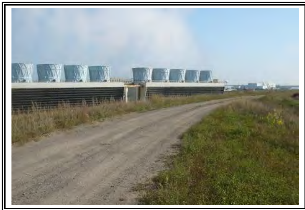
Crest of North Dam, facing east.
