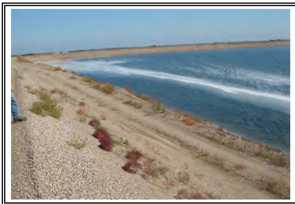
Upstream slope of North Embankment, facing east.
