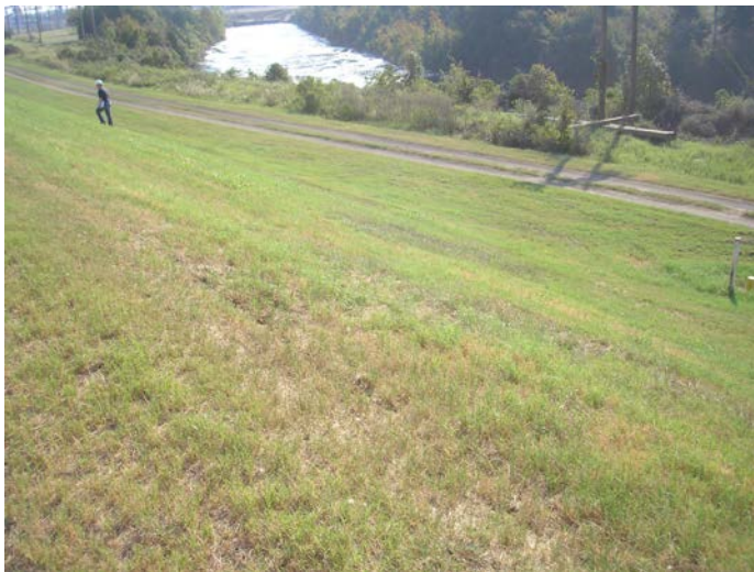
Figure 5.2.3-2 Plant Cooling Water Discharge Canal near Bottom Ash Pond North Embankment
