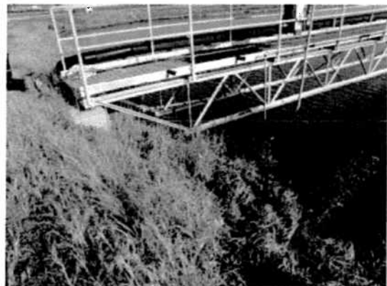
Figure 9: Bush Growing South Pond Embankment
