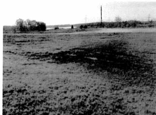
Figure 17: South Pond Standing Water at Toe
