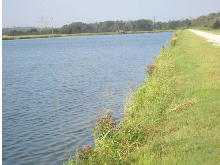
Figure 5.2.2-1 Interior Slope South Embankment
