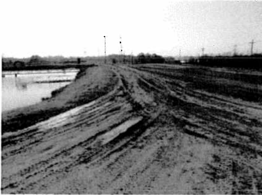
Figure 4: Crest Rutting North Pond
