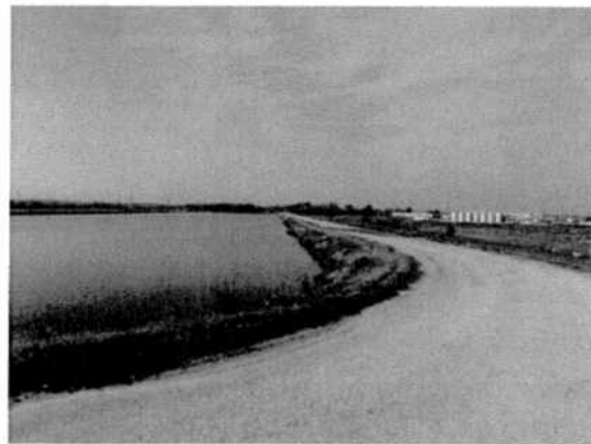
Figure 3: Crest of North Impoundment
