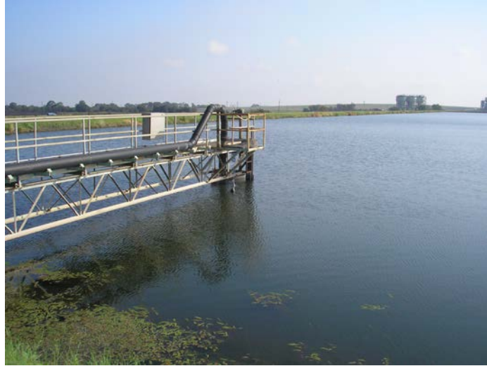
Figure 5.3.3-1: Access Bridge to Riser Structure; Bottom Ash Pond South Cell
