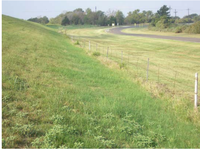
Figure 5.2.3-1 North Embankment Outside Slope and Toe
