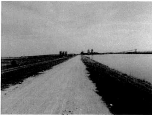
Figure 2: Crest of North Impoundment
