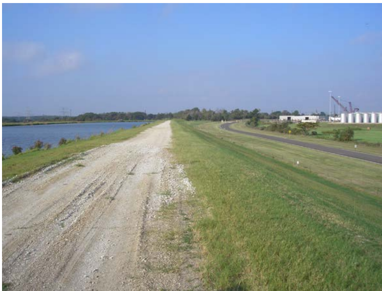
Figure 5.2.1-1 North Dike Crest View West Along Bottom Ash Pond
