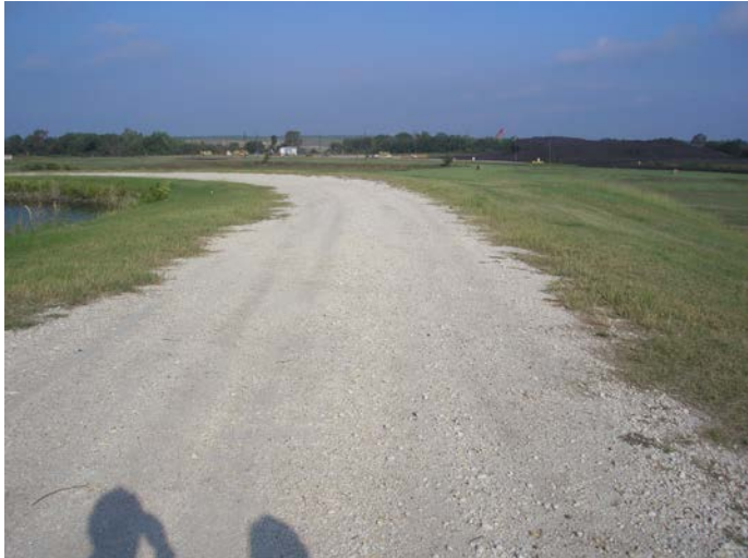
Figure 5.2.4-1: Bottom Ash Pond Northeast Groin
