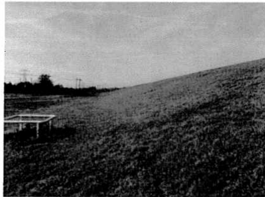
Figure 11: Downstream Embankment South Pond
