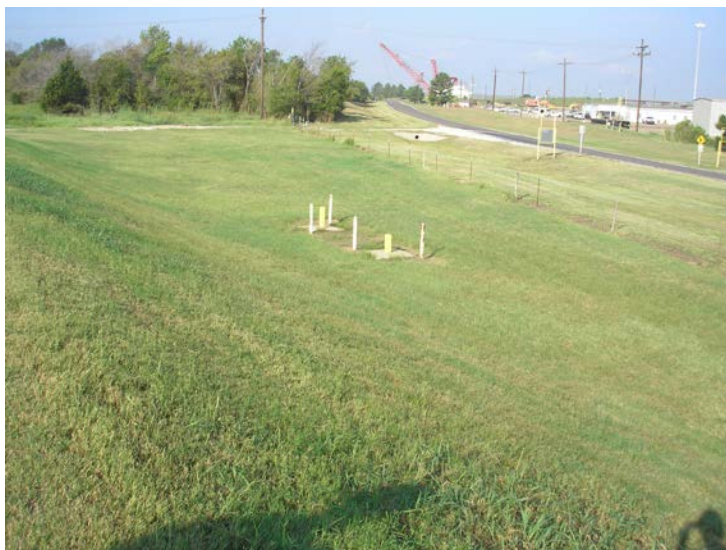
Figure 9.2-1: Piezometer near Embankment Toe – Northwest Groin
