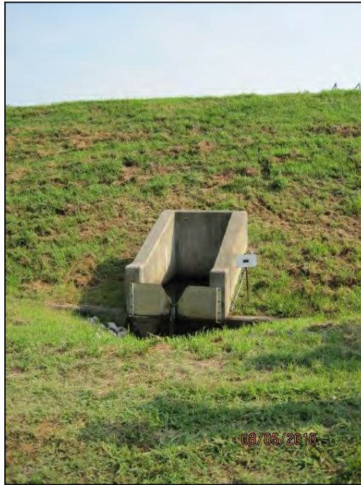
POND OUTLET AND KPDES OUTFALL 001 AT TOE OF SOUTH DIKE
