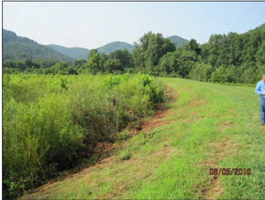
1-1 SOUTHWEST INTERIOR SLOPE AND CREST
