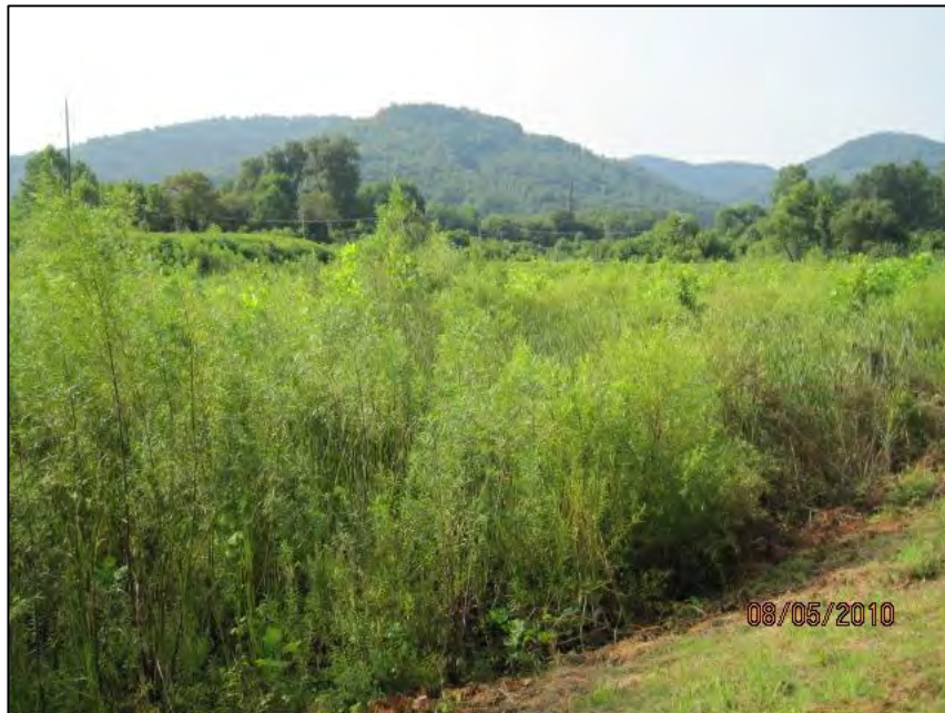
1-2 FROM SOUTHWEST DIKE LOOKING SOUTHEAST AT POND INTERIOR
