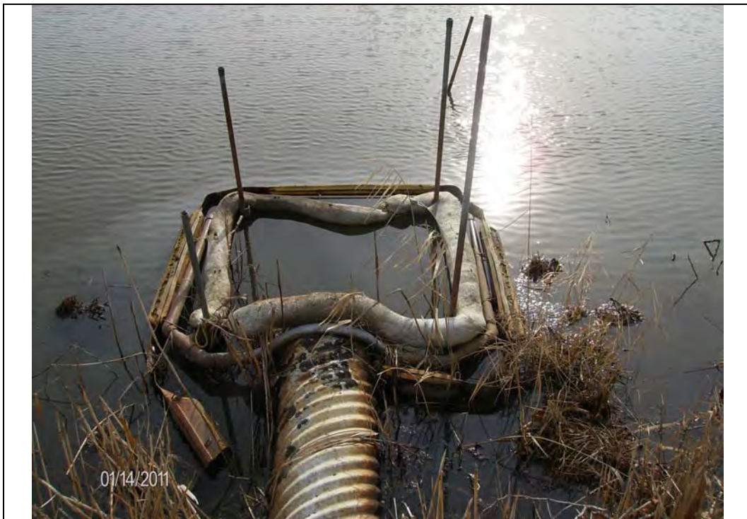
Photo #2: Principal Spillway inlet
