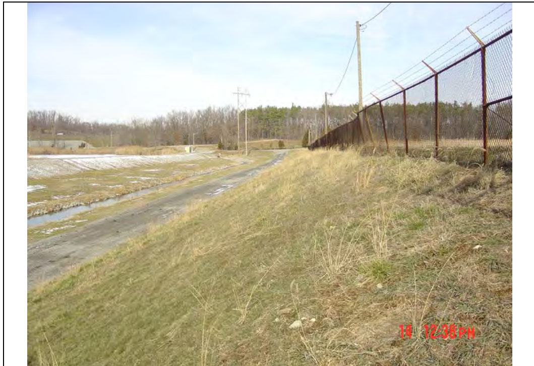
Photo #5: West embankment, exterior slope, looking north
