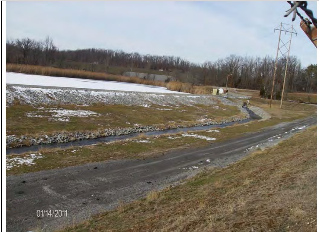
Photo #5: East embankment, downstream slope and toe, looking northwest
