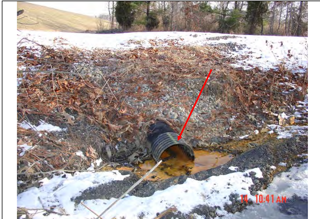
Photo #6: Drainage pipe at west end of south embankment, looking NE Note: Ponded water in outlet pipe
