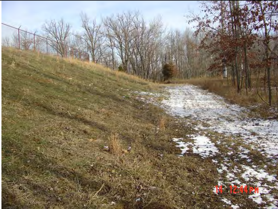
Photo #1: Exterior slope toe, south embankment east side, looking NW
