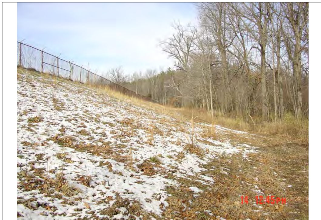
Photo #6: East embankment, exterior slope and toe, looking north
