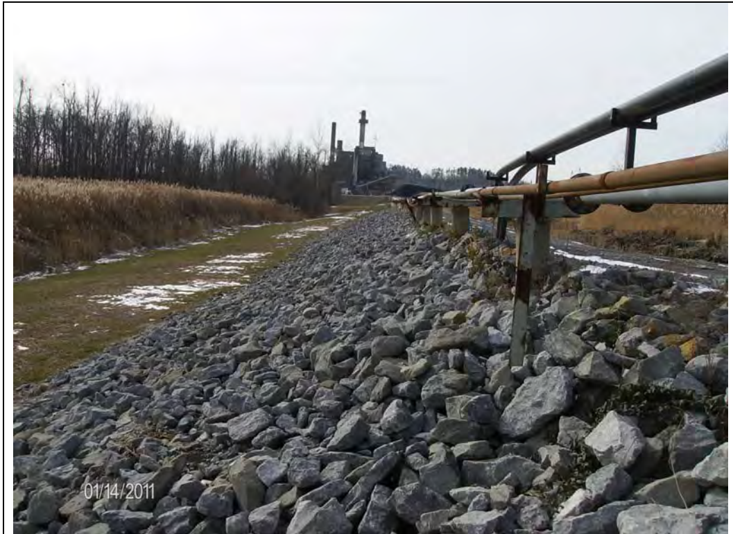
Photo #7: South embankment, downstream slope, southwest
