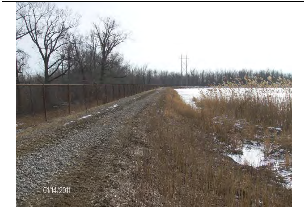
Photo #3: East embankment, interior slope, looking south
