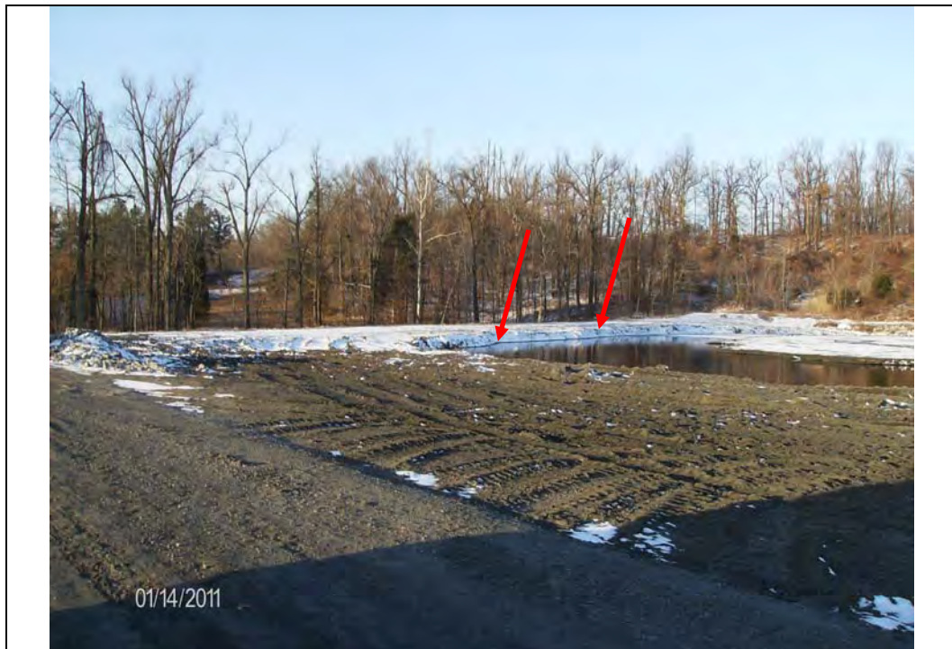
Photo #5: Interior slope of west embankment, looking west
