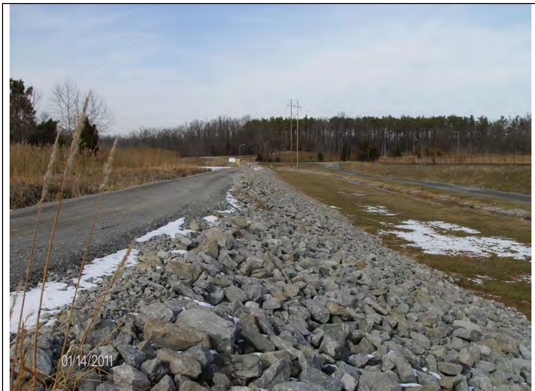
Photo #6: East embankment crest and downstream slope, looking north
