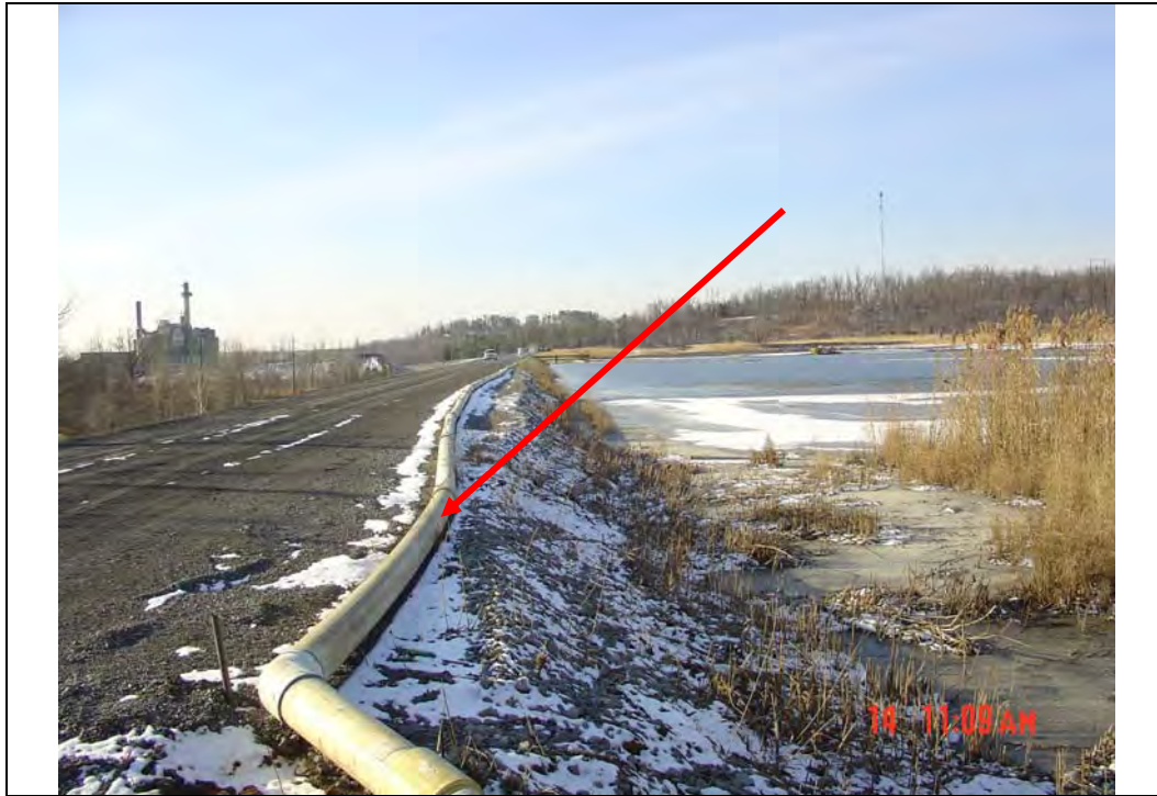
Photo #15: East end of south embankment, interior slope and crest, looking west Note: Ash discharge line
