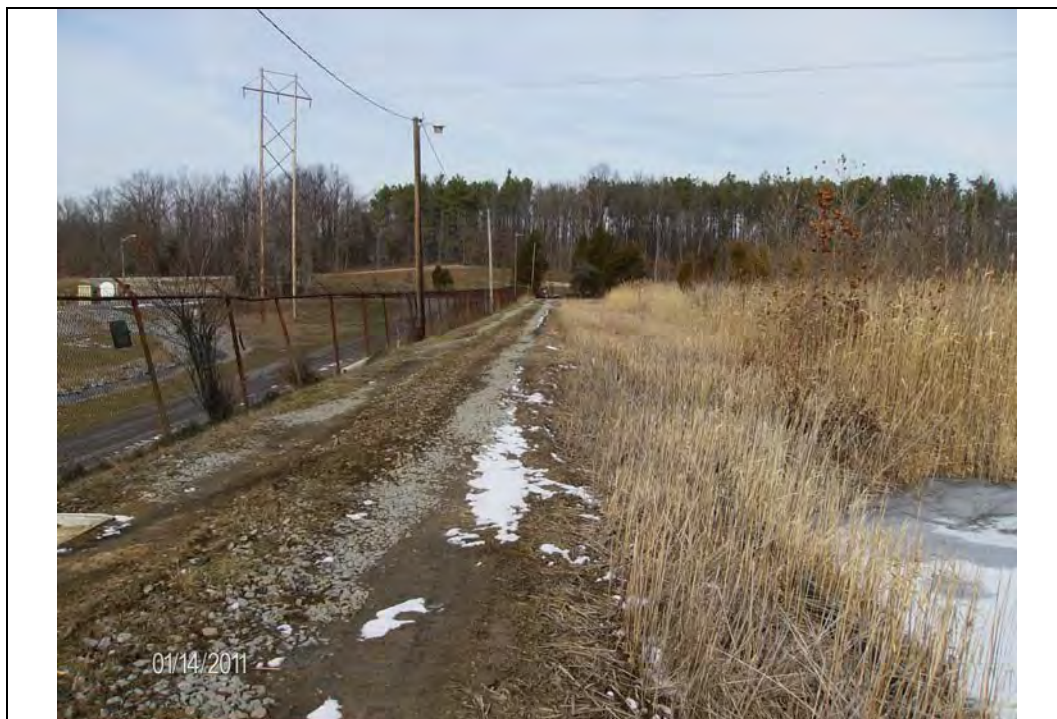
Photo #4: West embankment, crest and interior slope, looking north
