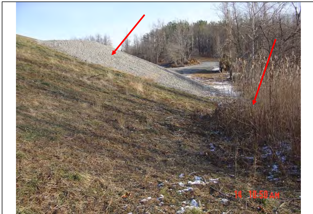
Photo #11: Toe of south exterior slope, looking NE
