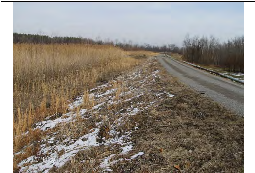
Photo #5: South embankment, interior slope, looking east Note: Sparse vegetation
