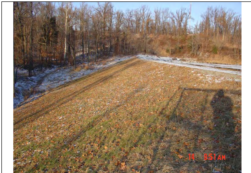
Photo #10: Exterior slope of west embankment, east
