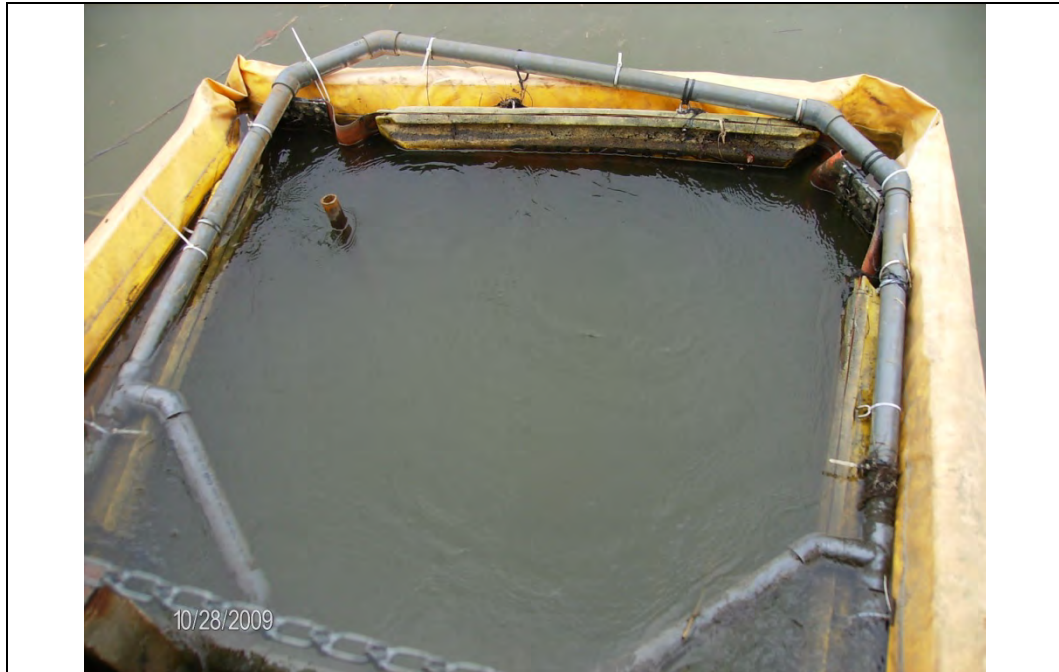
Photo #3: Principal Spillway Inlet
