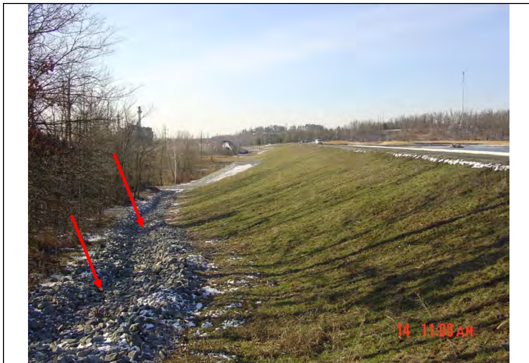
Photo #12: East end of south embankment, exterior slope, looking south
