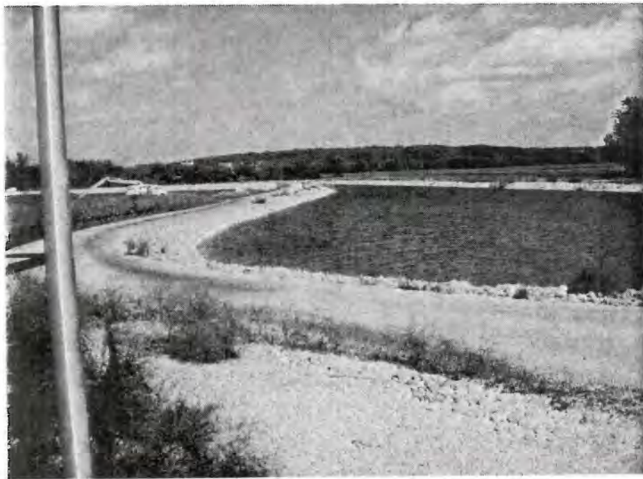
Figure 8.1-1: Photo of dike dividing ash pond from clear water pond.
