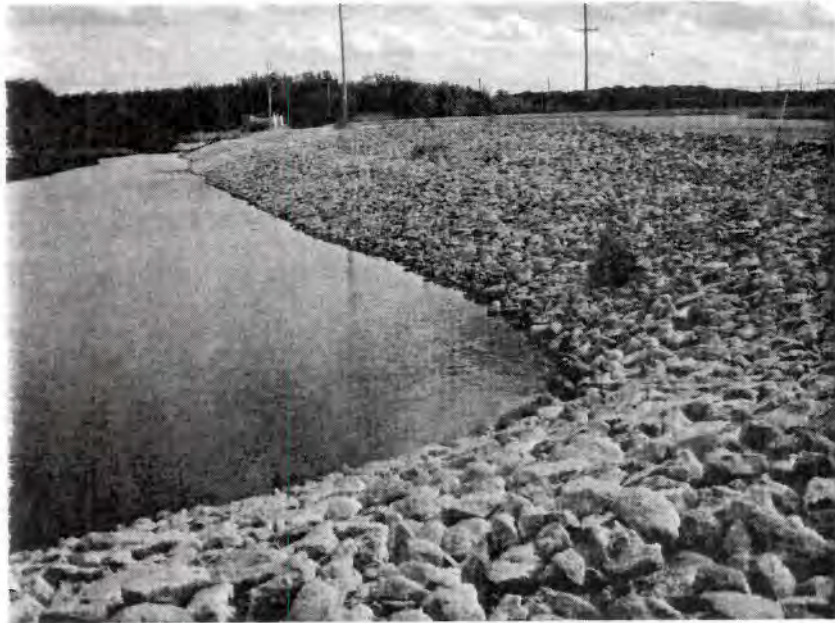
Figure 5.2.4-1: Photo of Interior Groin at Northwest Corner of Impoundment. Note that the dike in upper right hand corner also serves as the flood prevention dike for the plant.
