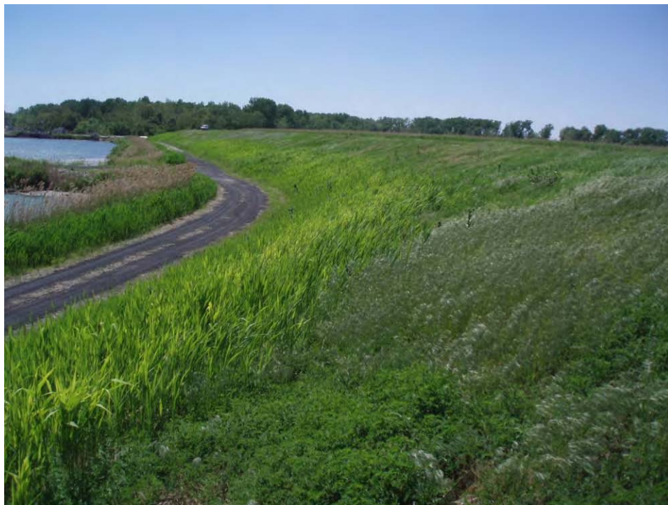
59. Pond B - South embankment exterior slope, looking west. Note change in vegetation at mid slope and stabilized FGD material is very soft.
