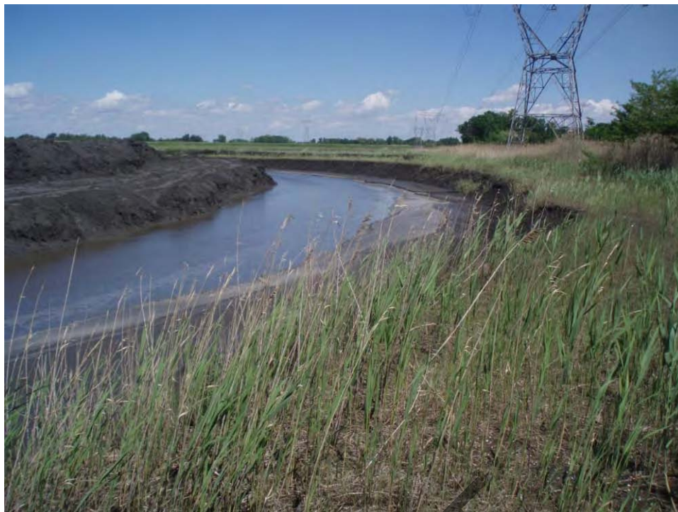
5. Pond A rim ditch, looking north.
