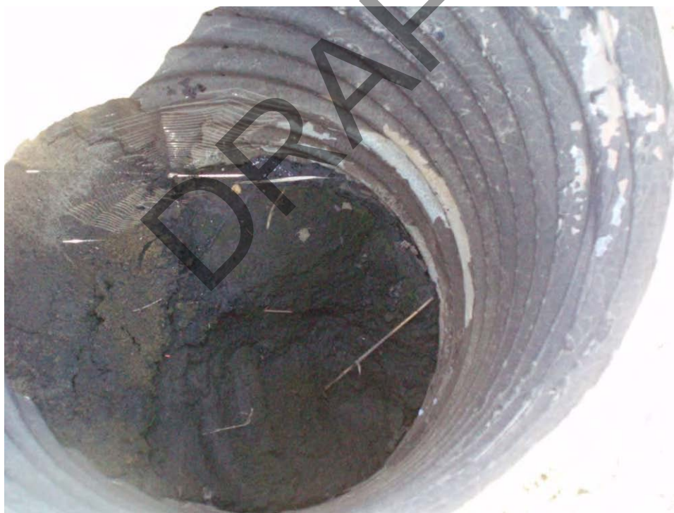
142. Inside of equalizer pipe at Pond C. Note approximately half of the pipe is filled ash.
