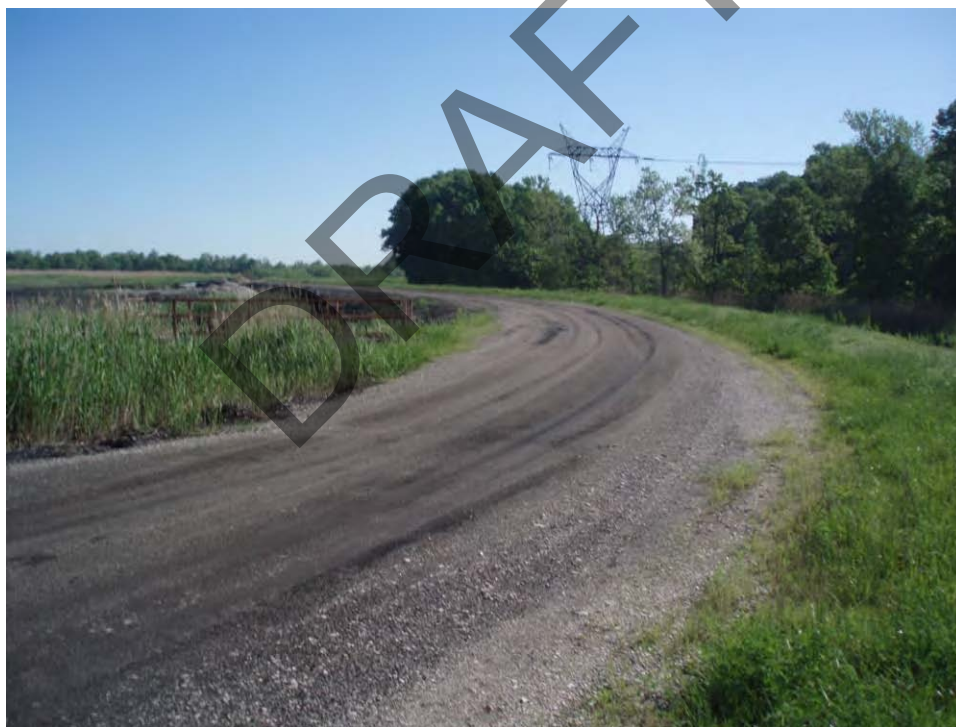
136. Pond C - East embankment crest, looking northeast.
