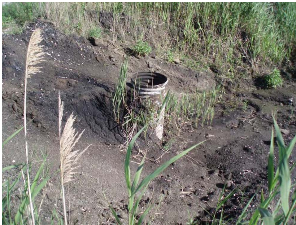
141. 24-inch-diameter CMP equalizer pipe from Pond C to Pond B. Note inlet has a T connection on the end of the pipe.
