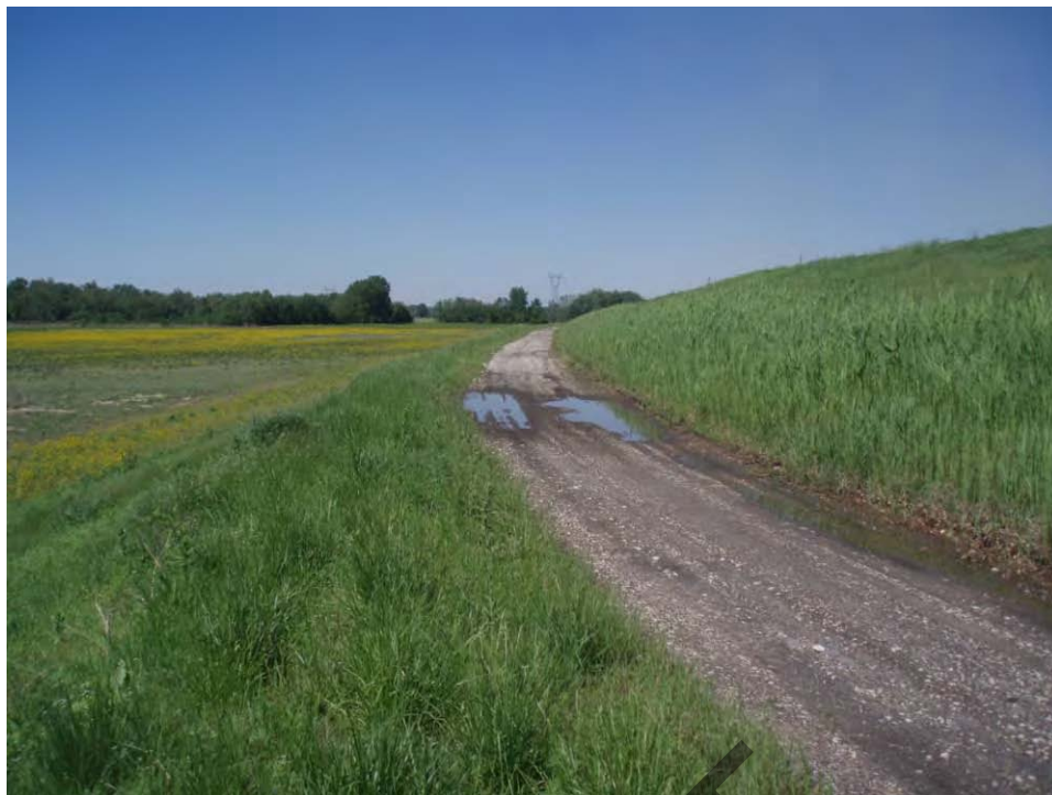
75. Pond B - West embankment bench, looking north. Note inside of bench is wet from recent storm events.
