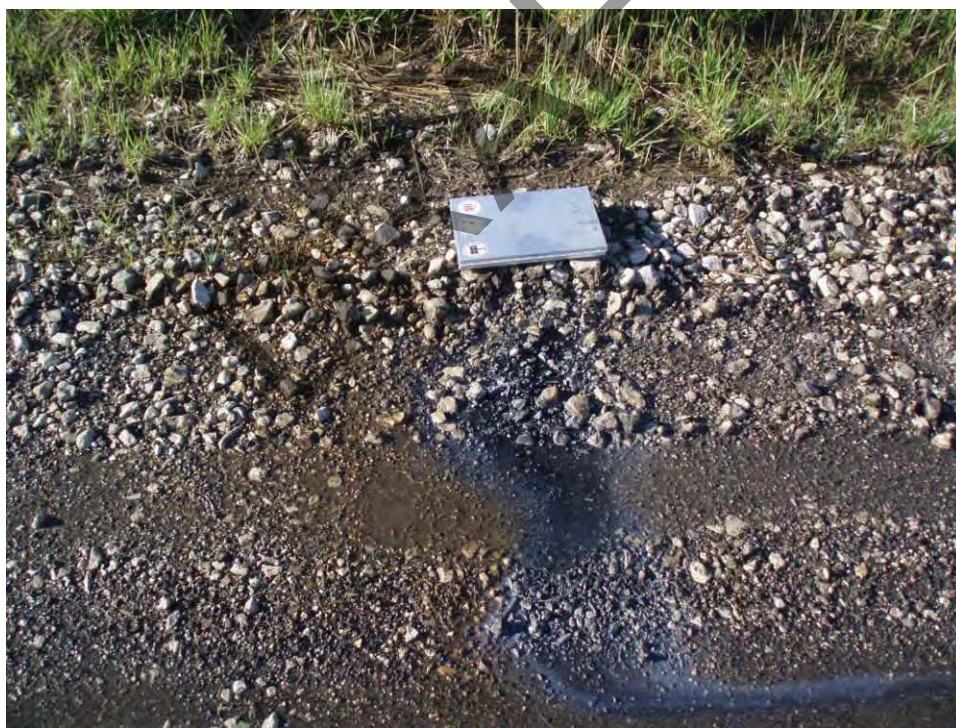
116. Pond C - West embankment bench, looking at active seepage located at toe of upper exterior slope. Note the white and black sheen in the water.
