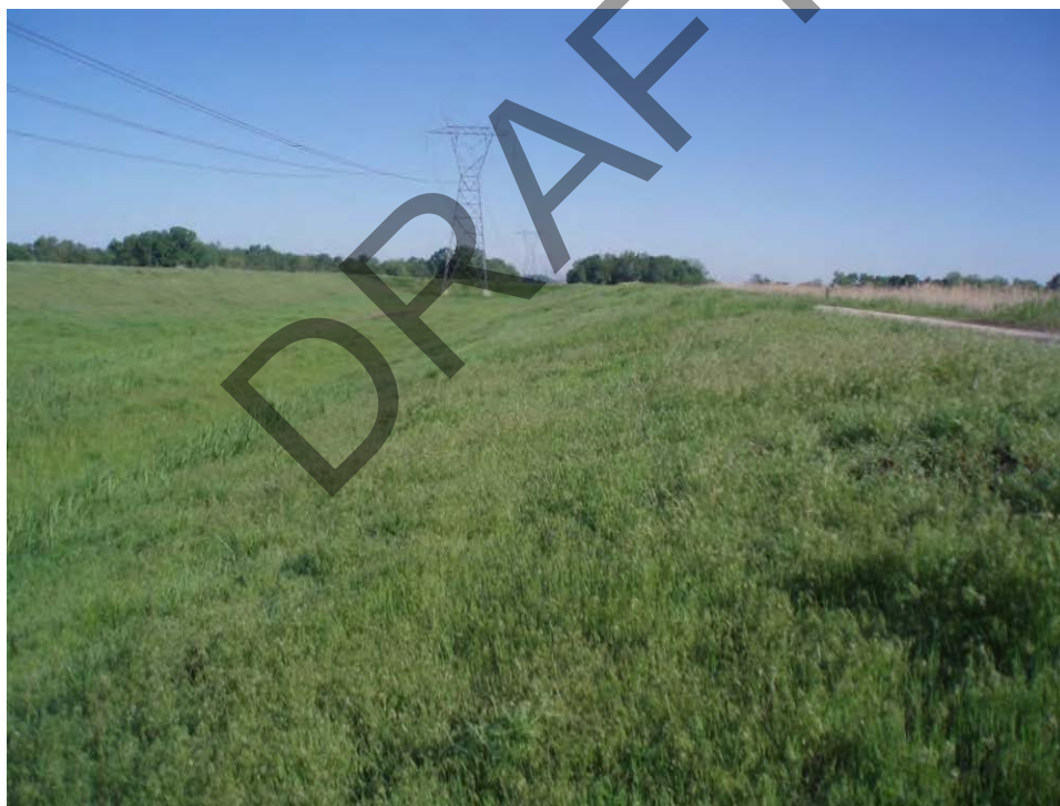
138. Pond C - South embankment exterior slope, looking northwest at area between Pond B and Pond C.
