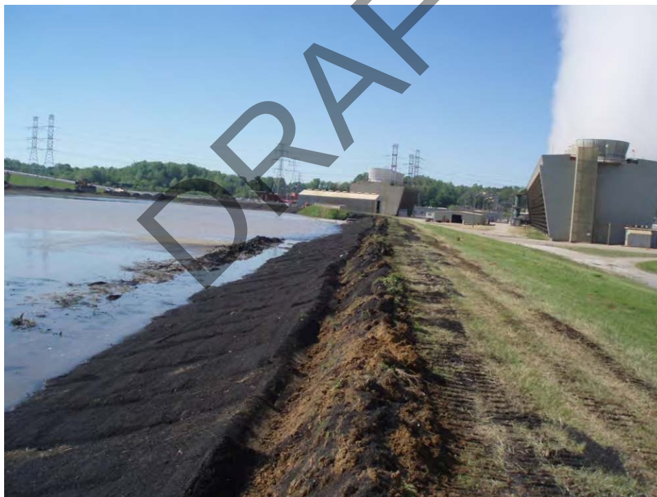
32. Pond A - West embankment interior slope, looking south at rough embankment grading
