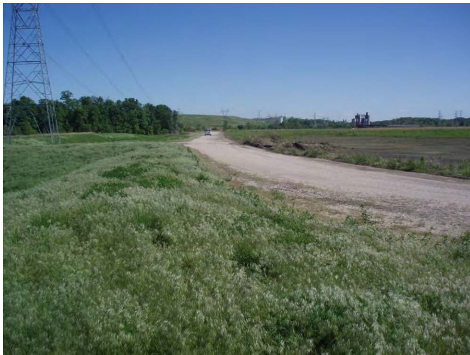
93. Pond B - North embankment crest, looking southeast.
