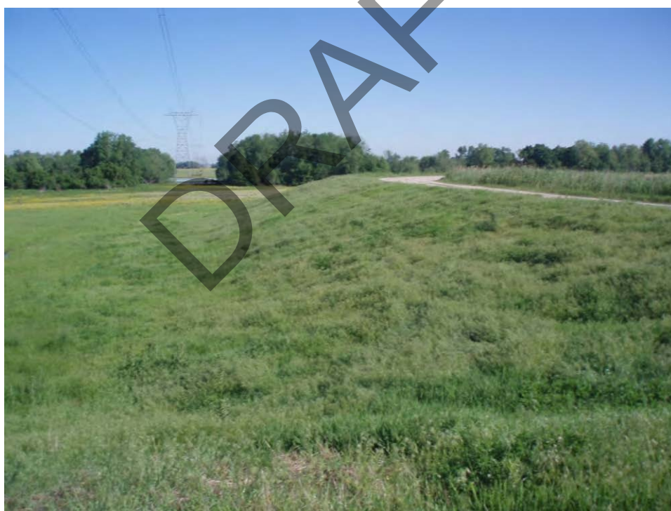
140. Pond C - South embankment exterior slope, looking northwest.
