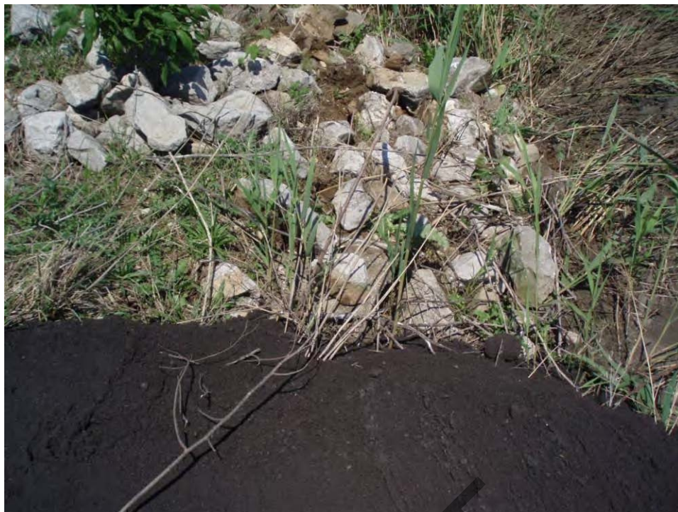
33. Pond A - 24-inch-diameter RC pipe being covered by ash.
