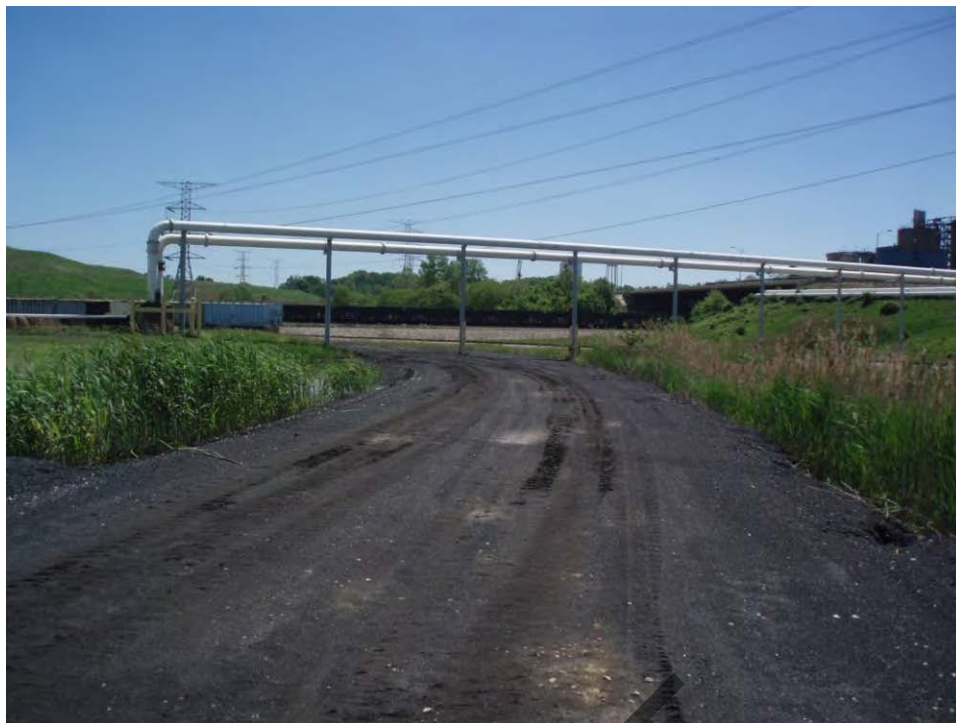
11. Pond A - South embankment looking southeast.
