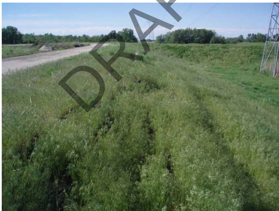
96. Pond B – North embankment exterior slope looking northwest at tractor ruts, bare spots, very soft stabilized FGD.
