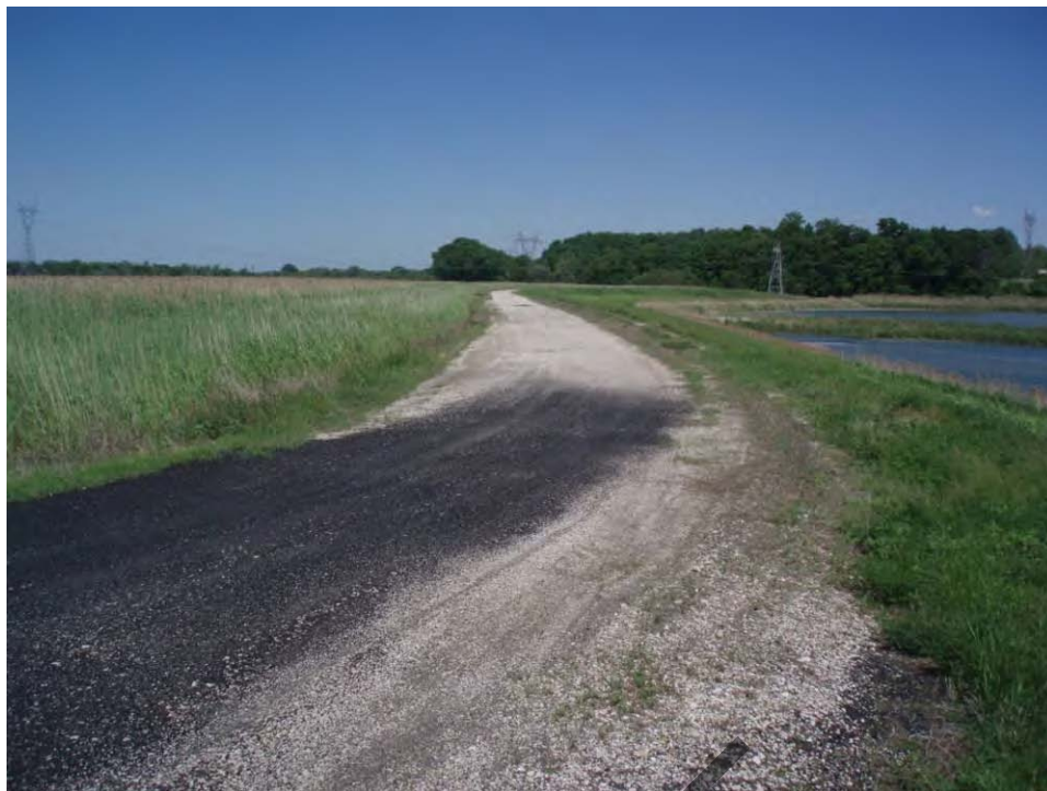
67. Pond B - South embankment crest, looking northeast.
