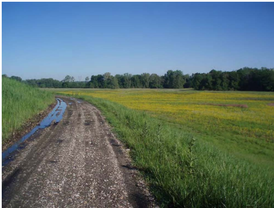
123. Pond C - North embankment bench, looking northwest.
