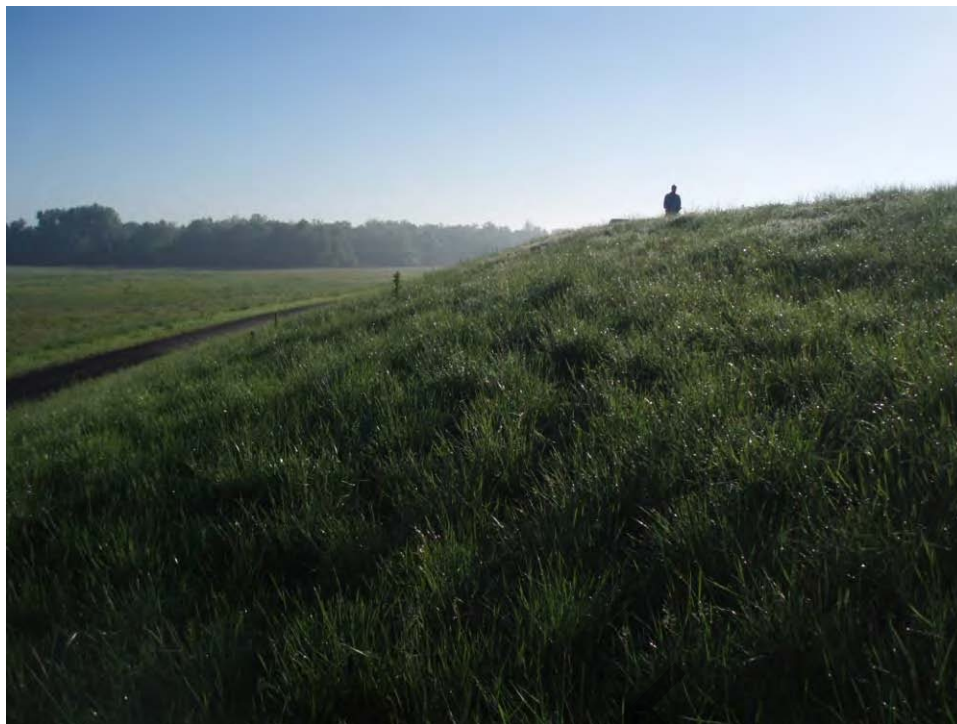
101. Pond C - West embankment upper exterior slope, looking northeast.
