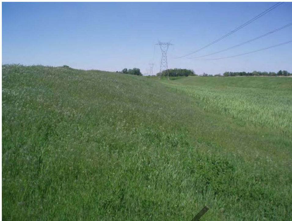
55. Pond B - East embankment exterior slope, looking north.
