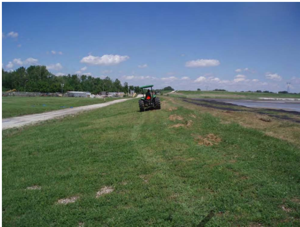
19. Pond A - West embankment exterior slope, looking north at mowing operation.
