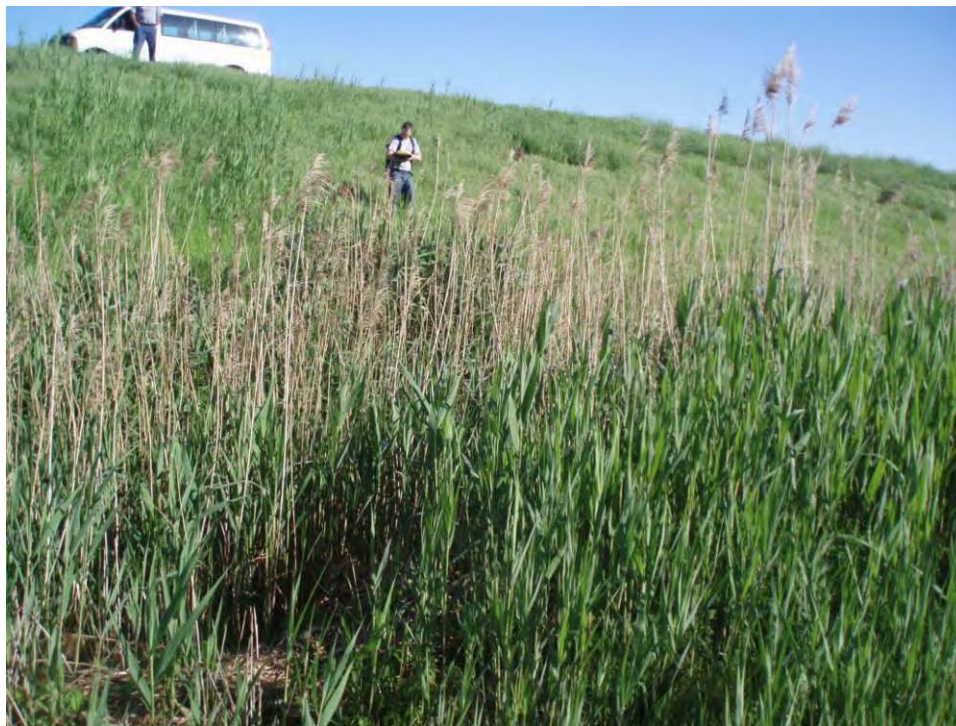
129. Pond C - East embankment exterior slope, looking at area of outlet pipe from outlet structure. Note water was flowing from outlet pipe into drainage ditch.
