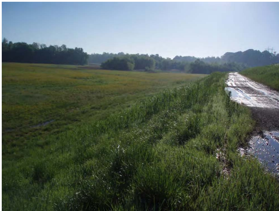
113. Pond C - West embankment bench, looking east.
