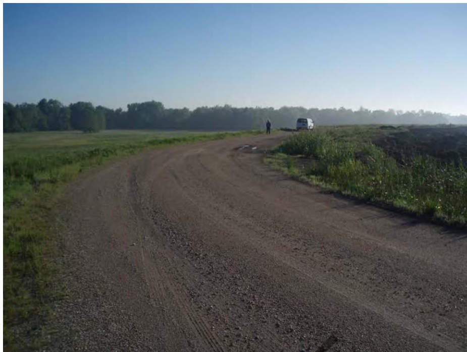
99. Pond C - West embankment crest, looking northeast.
