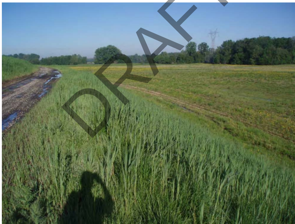
114. Pond C - West embankment bench, looking west.
