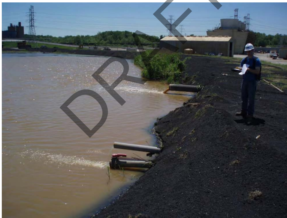
20. Pond A - West embankment interior slope, looking south at one (1) 12-inch-diameter DI pipe and two (2) 8-inch-diameter steel pipes from plant.
