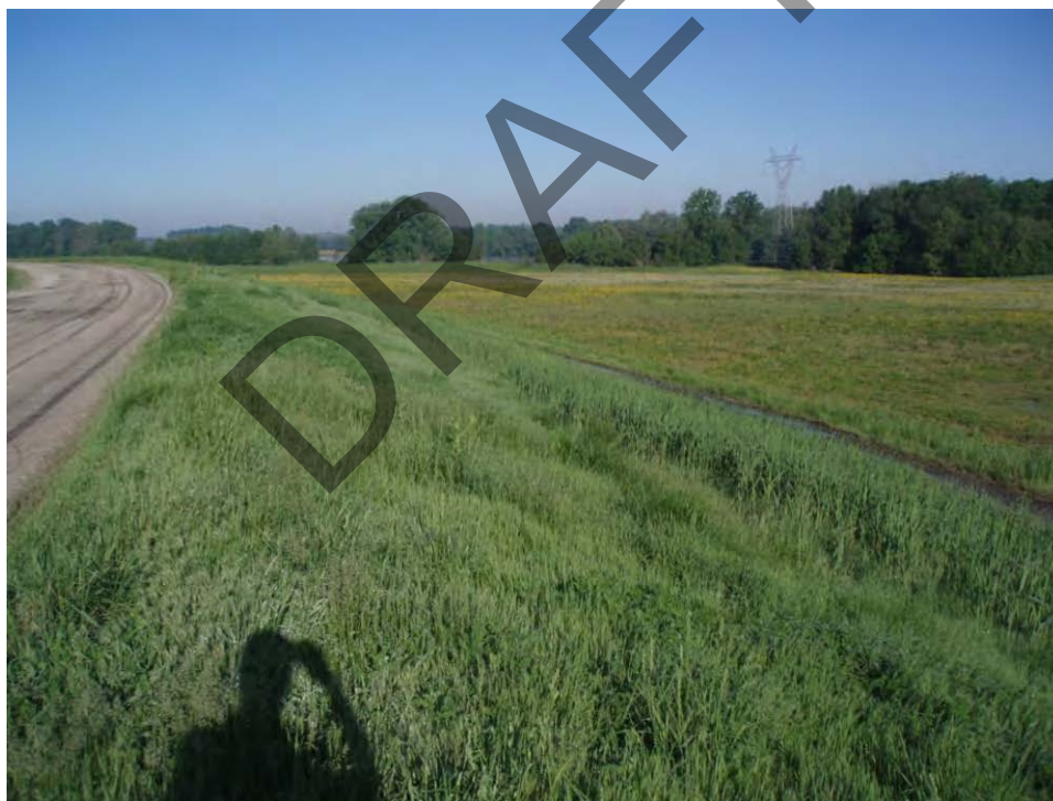
112. Pond C - West embankment crest, looking west.
