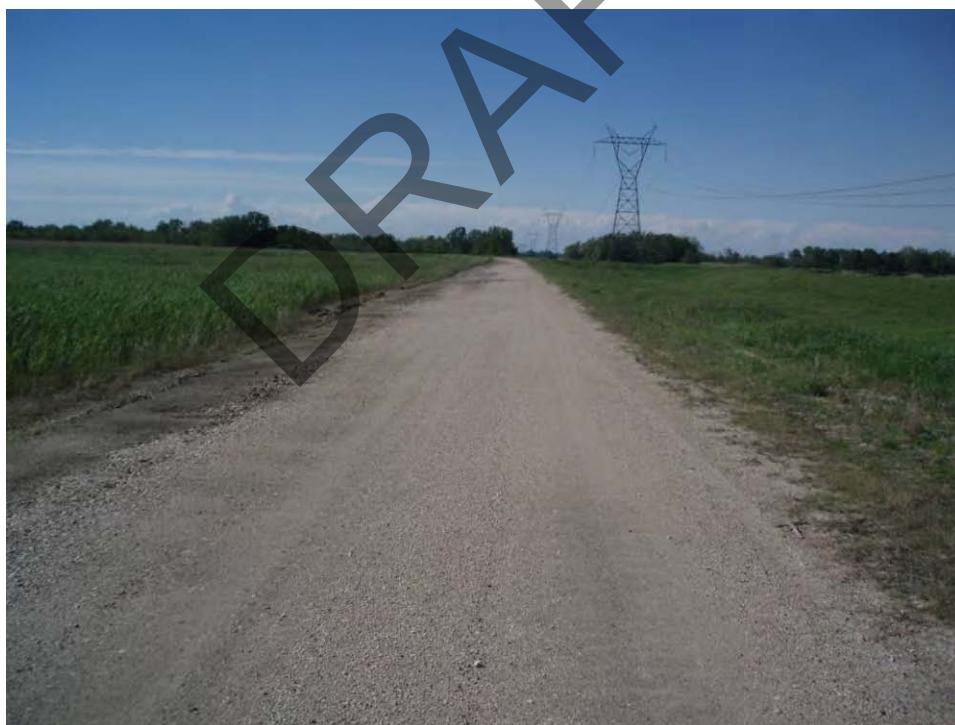
98. Pond B - North embankment crest, looking northwest.
