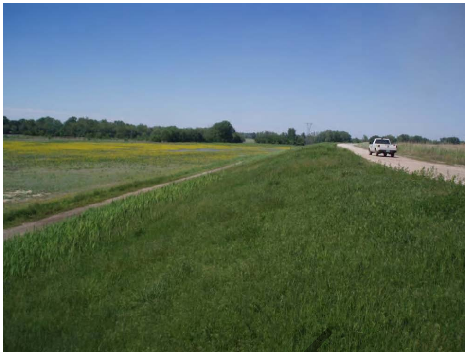
77. Pond B - West embankment upper exterior slope, looking north.
