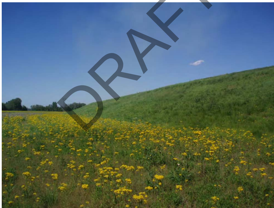
74. Pond B - West embankment, looking north at downstream area in flood plain. Note field area is saturated and wet from recent storm events.
