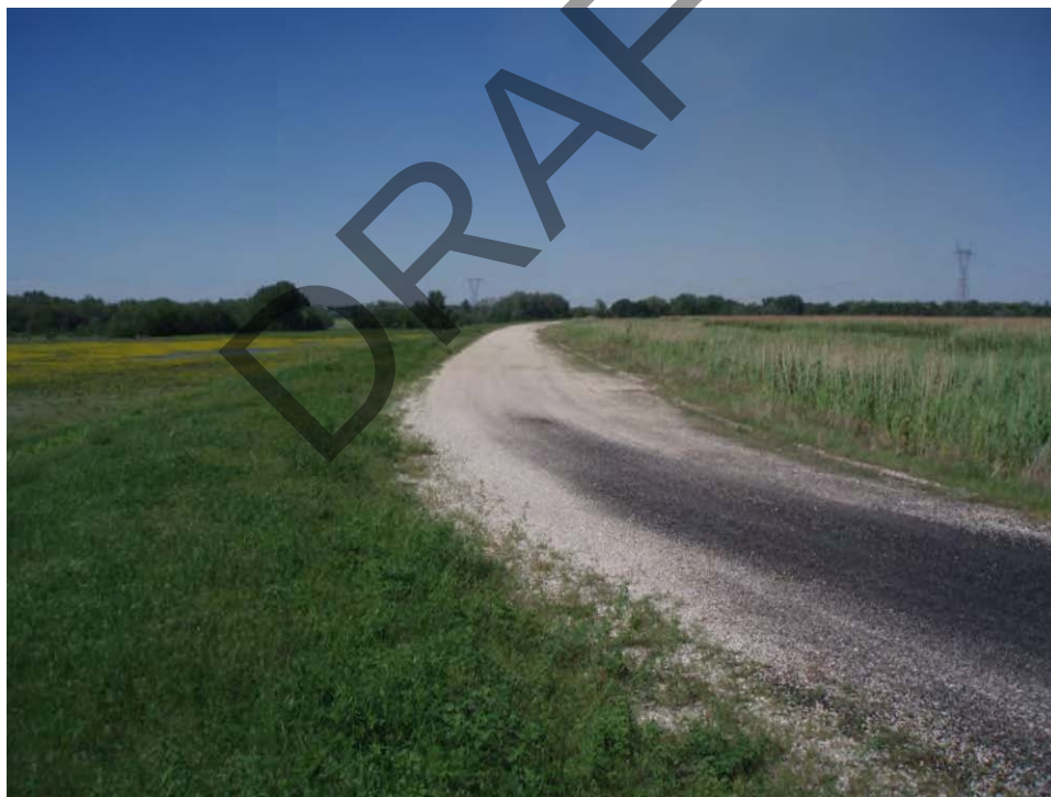
76. Pond B - West embankment crest, looking north.
