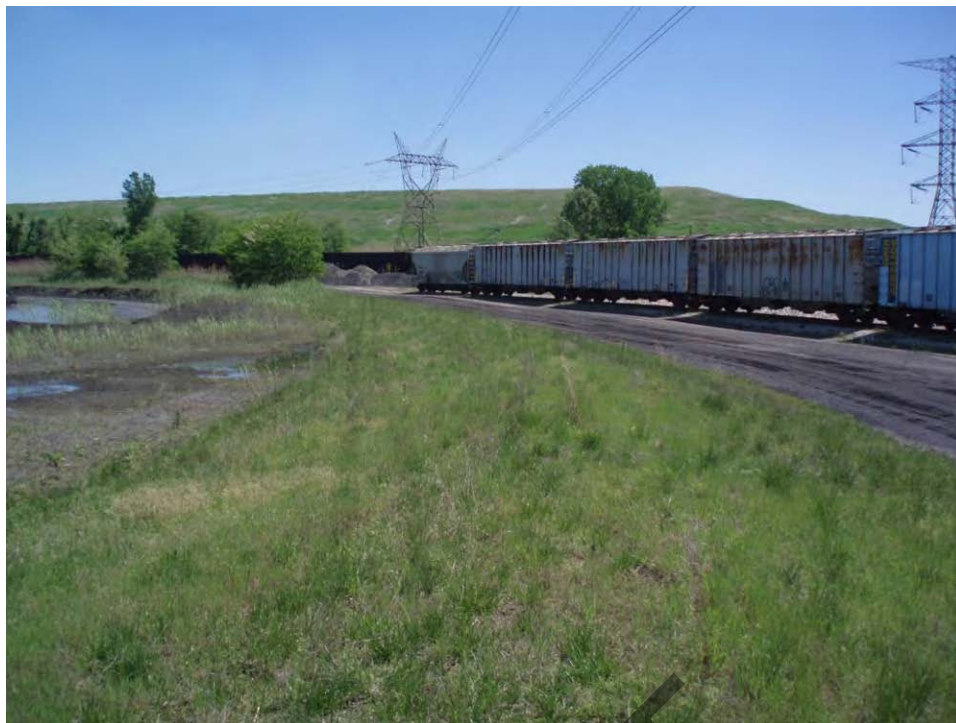
9. Pond A - South embankment crest, looking east.
