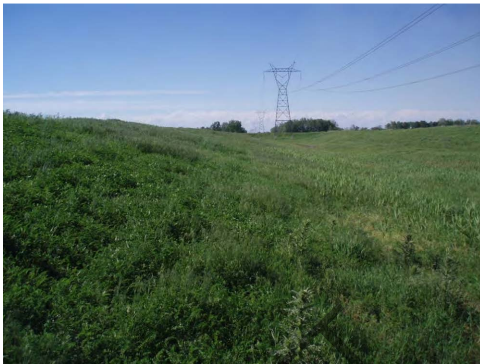
97. Pond B - North embankment exterior slope, looking northwest.
