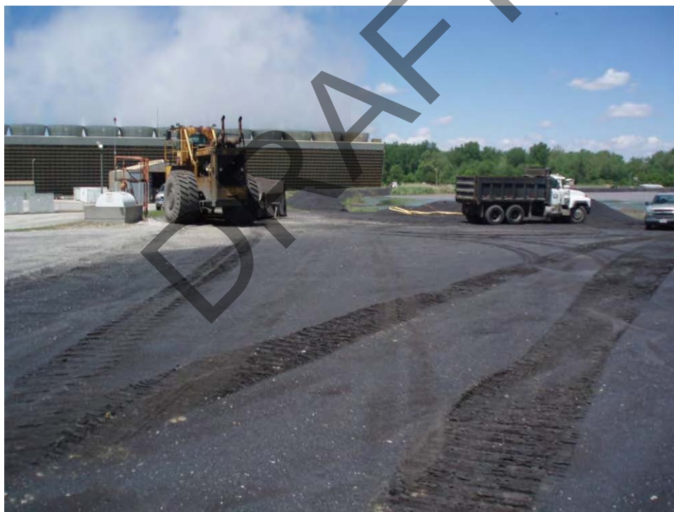
14. Pond A - South embankment crest, looking northwest.
