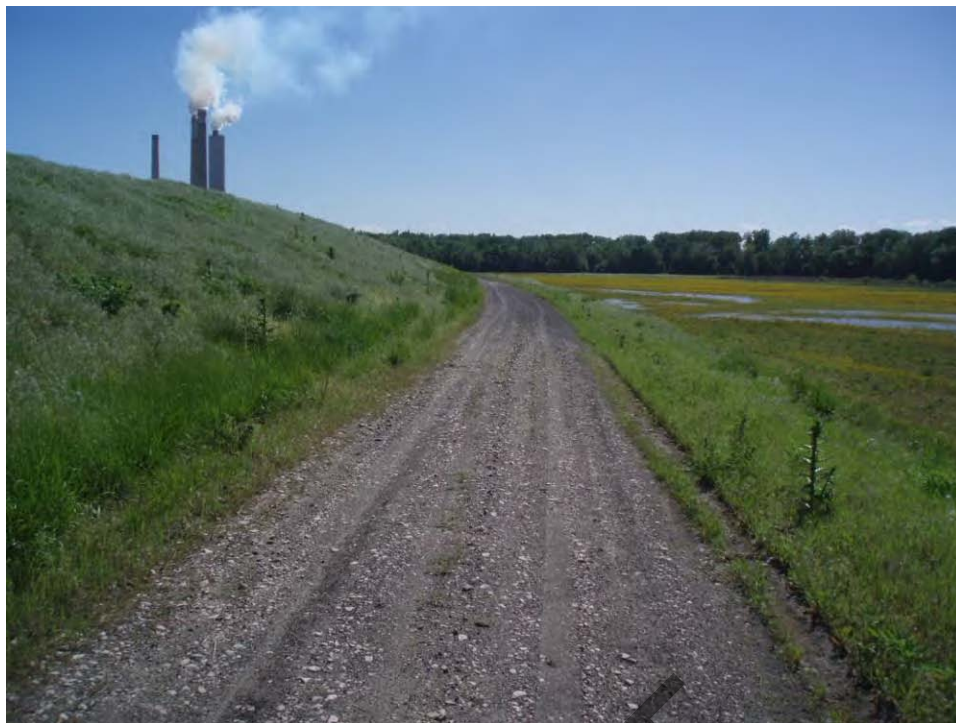
89. Pond B - West embankment bench, looking southwest.
