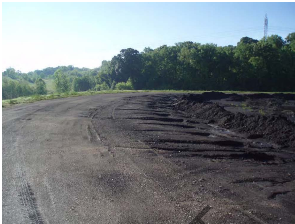
121. Pond C - North embankment crest, looking southeast.
