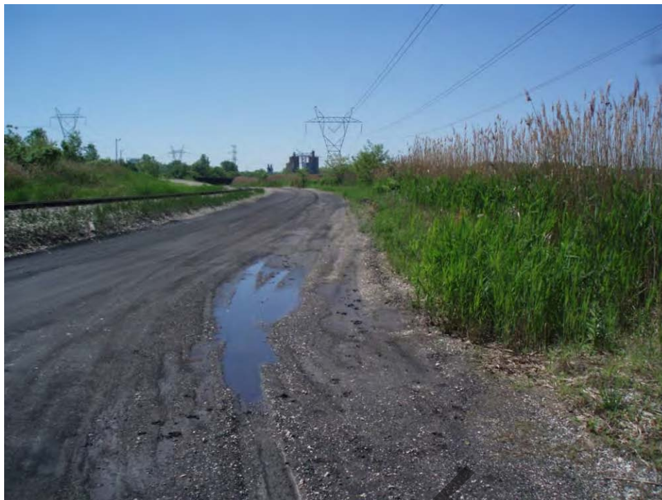
1. Pond A - East embankment crest, looking south.
