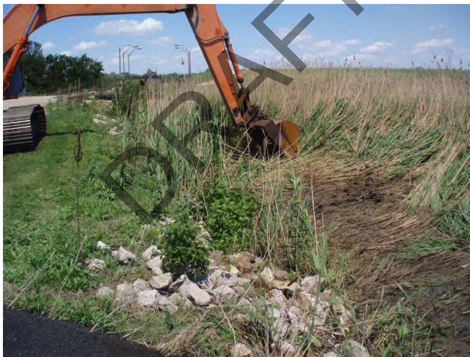
30. Pond A - West embankment interior slope, looking north at excavator flattening vegetation before placing ash material. Note an unknown 24-inch-diameter RC pipe in the embankment was being covered with ash.
