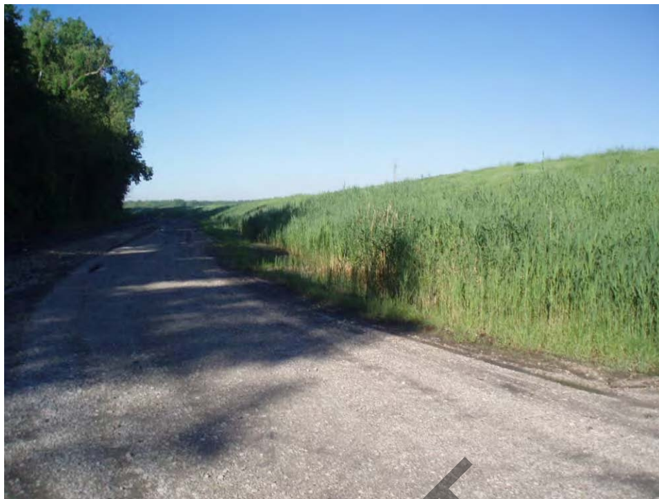
127. Pond C - East embankment exterior slope and drainage ditch, looking southwest. Note water level in drainage ditch approximately 1.5' below roadway and 5'-8' tall vegetation on lower portion of the slope extending from northern corner to access ramp. Slope at drainage ditch is over-steepened.
