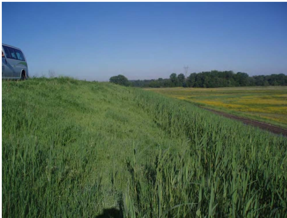
119. Pond C - West embankment upper exterior slope, looking west.
