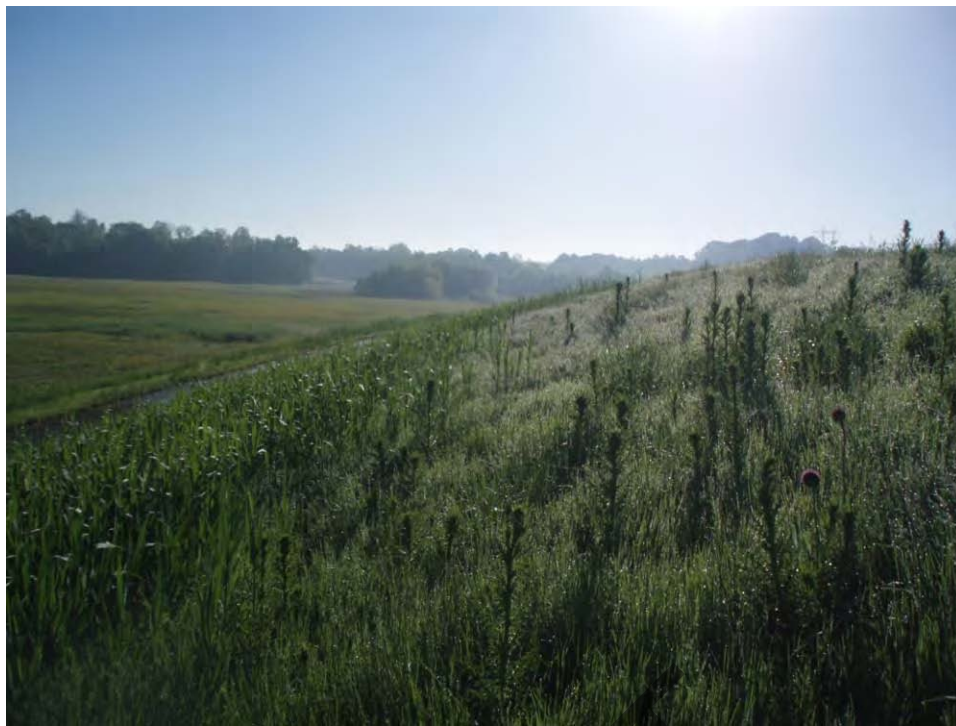
109. Pond C - West embankment upper exterior slope, looking northeast.
