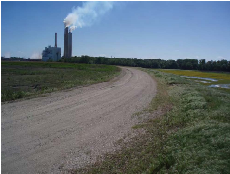
91. Pond B - West embankment crest, looking southwest.
