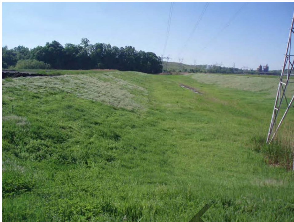
139. Pond C - South embankment exterior slope, looking southeast at area between Pond B and Pond C.
