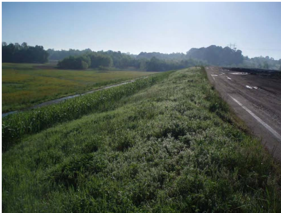
111. Pond C - West embankment crest, looking east.
