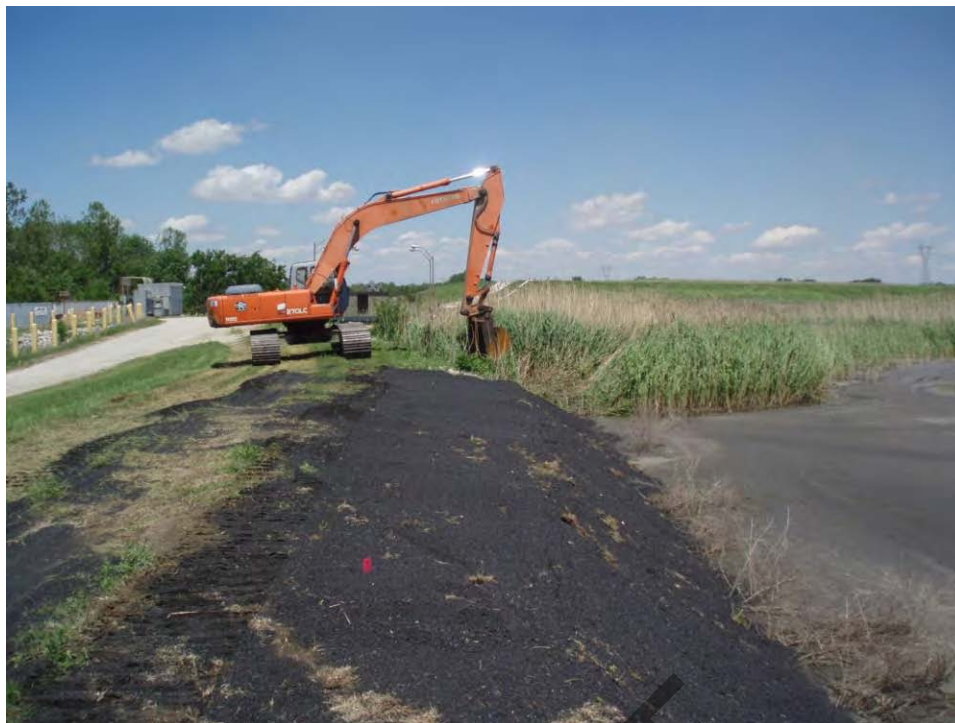
29. Pond A - West embankment interior slope looking north at embankment work.
