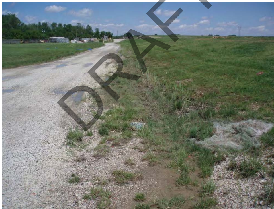
24. Drainage ditch at toe of Pond A west embankment. Note ditch has sparse vegetation.
