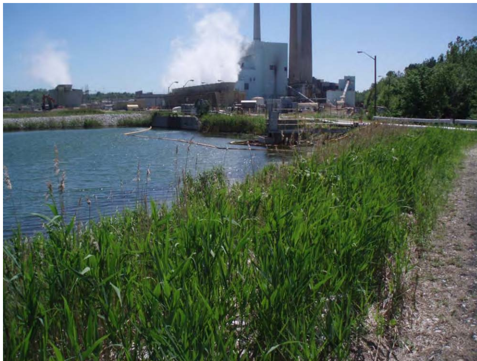
65. Pond A - Discharge, looking southwest at outlet structure and recycle pump station.
