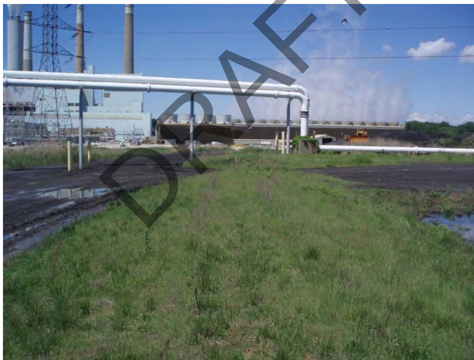
10. Pond A - South embankment crest, looking west. Note access ramp excavated in crest to access the sluice pipes.
