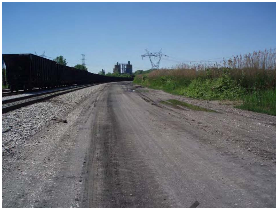
3. Pond A – East embankment crest, looking south.
