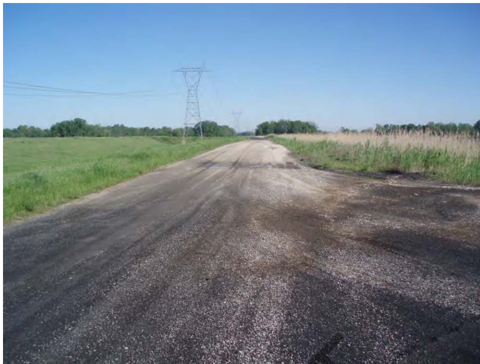
137. Pond C - South embankment crest, looking northwest.
