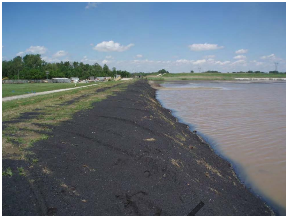
21. Pond A - West embankment interior slope and crest, looking north
