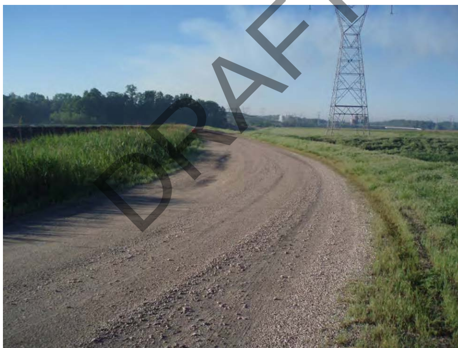
100. Pond C - South embankment crest, looking southeast.
