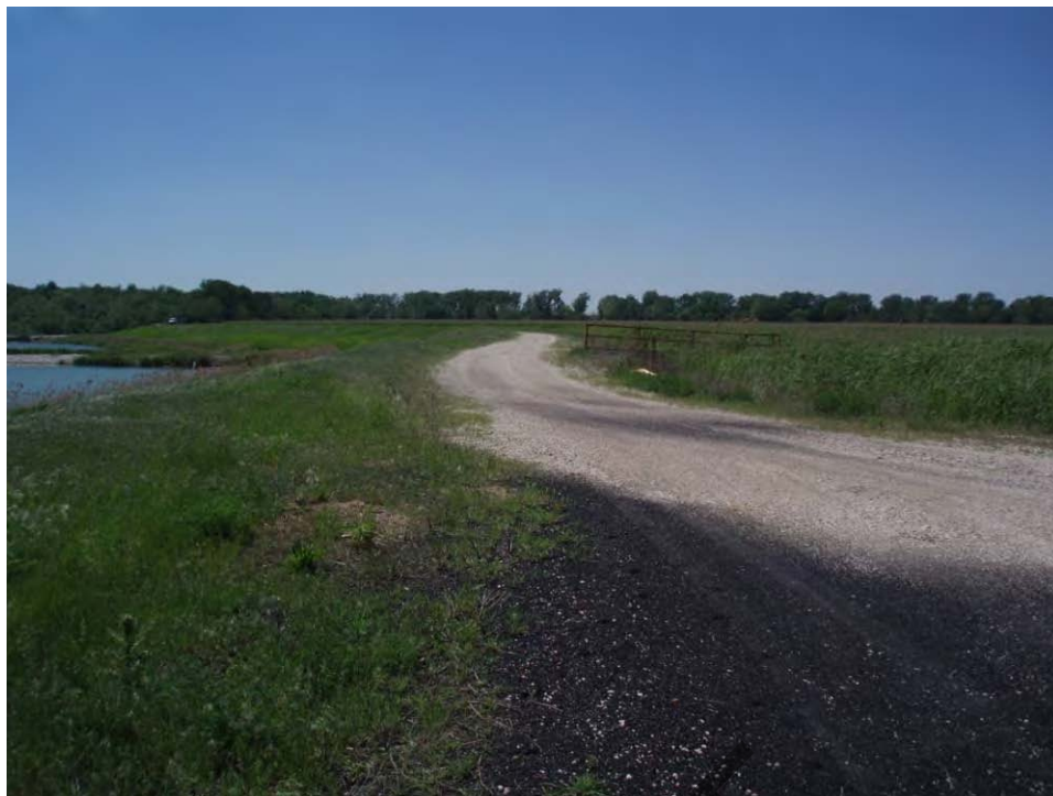
53. Pond B - South embankment crest, looking west.
