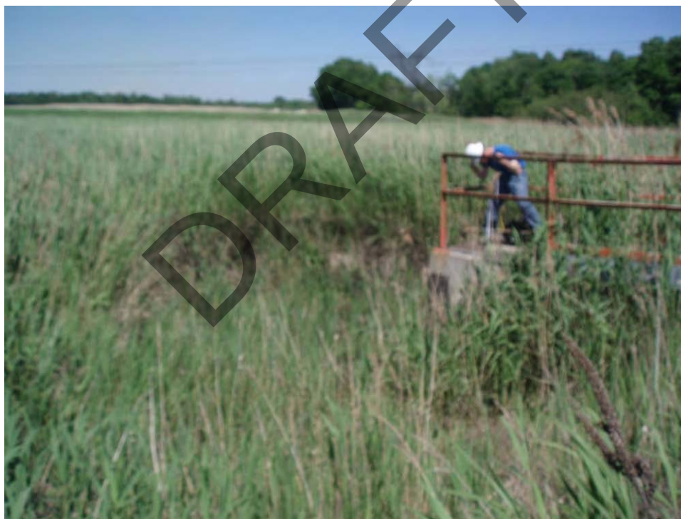
56. Pond B - Overview of outlet control structure with stoplogs, looking east.
