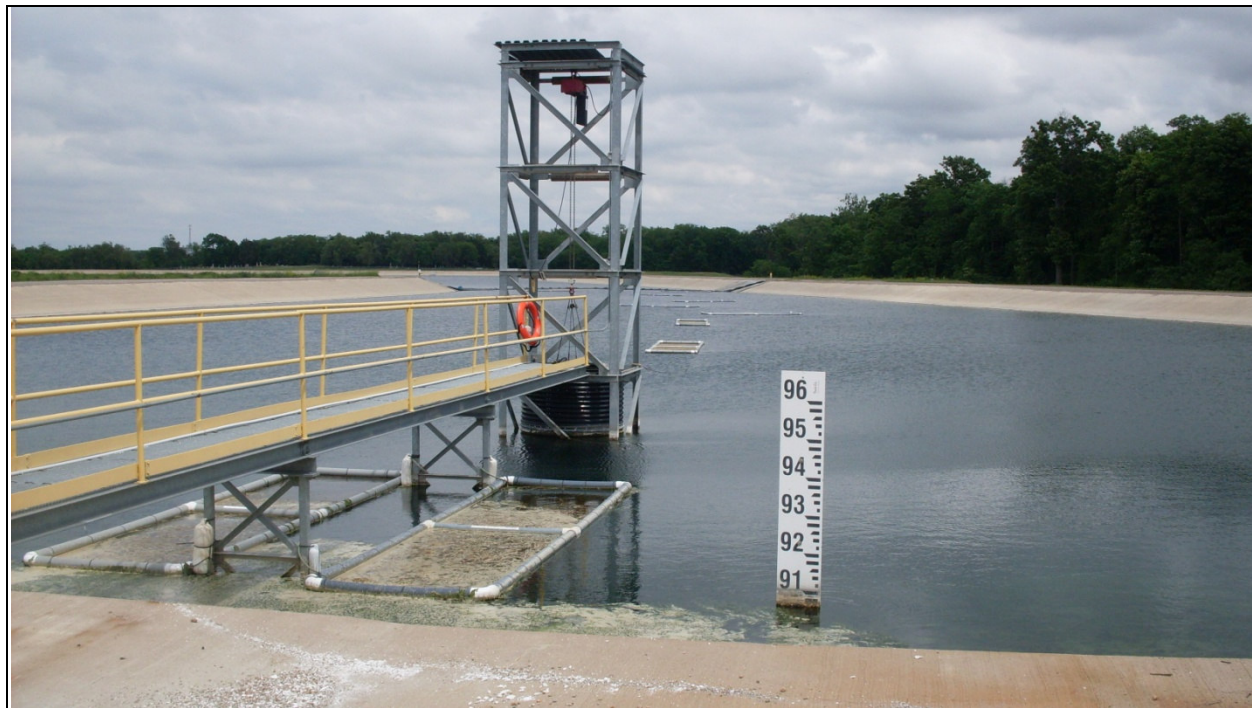
Photo 53: (EAPS) Cell 3, Staff Gage and Primary Spillway, Havana Power Plant, Havana, IL, 05.27.09
