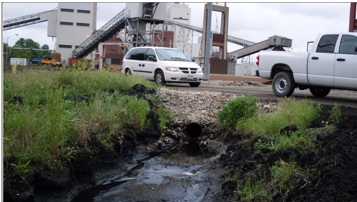
Photo 66: (NAPS) Coal Runoff (culvert connecting two NAPS cells), Havana Power Plant, Havana, IL, 05.27.09
