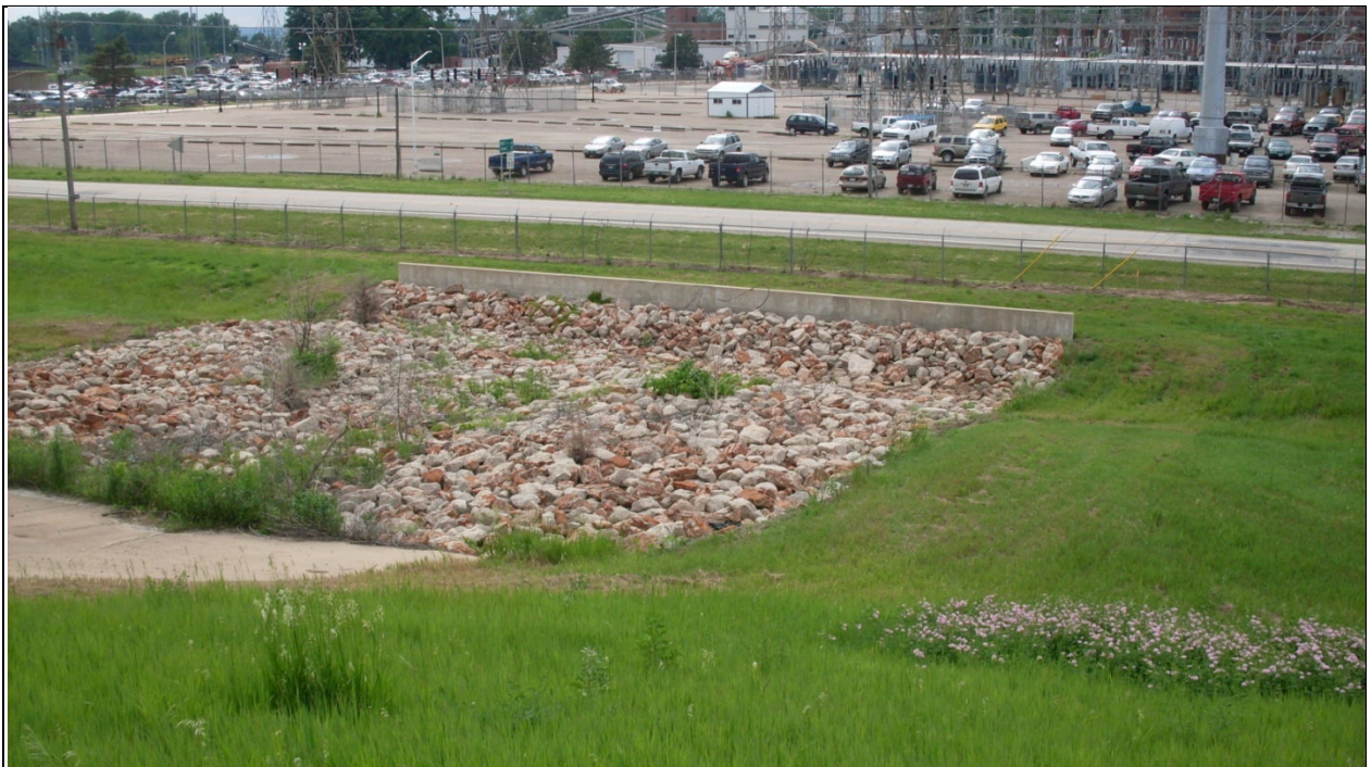
Photo 16: (EAPS) Cell 4, W Edge (energy dissipater of emergency spillway), Havana Power Plant, Havana, IL, 05.27.09
