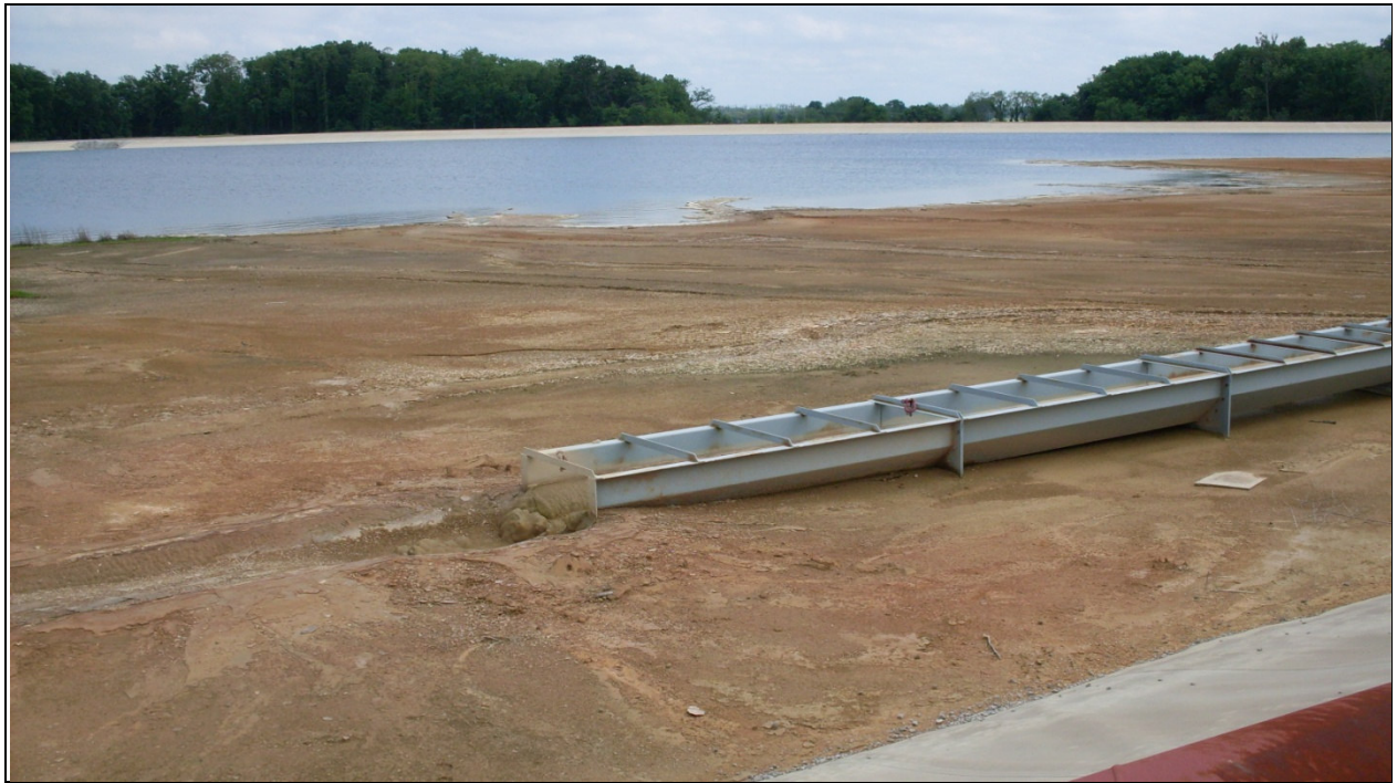
Photo 37: (EAPS) Cell 3, Open Trough Fly Ash Discharge, Havana Power Plant, Havana, IL, 05.27.09
