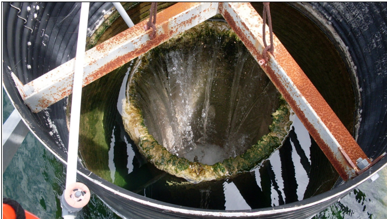
Photo 39: (EAPS) Cell 4, Primary Spillway from Cell 4 to River, Havana Power Plant, Havana, IL, 05.27.09
