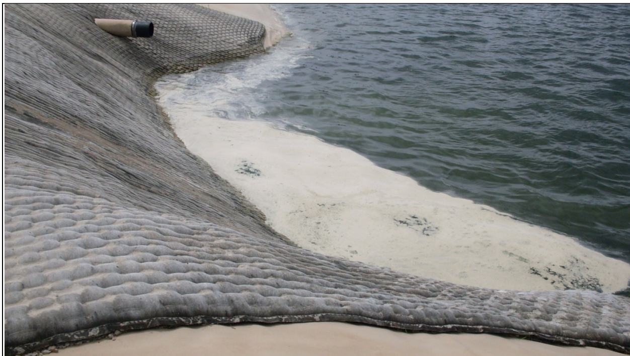
Photo 40: (EAPS) Cell 3, Pipe at SE of Cell 3 (fabrication over synthetic liner), Havana Power Plant, Havana, IL, 05.27.09
