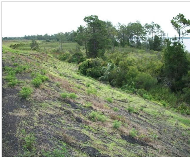
Photo 20b South embankment near center
