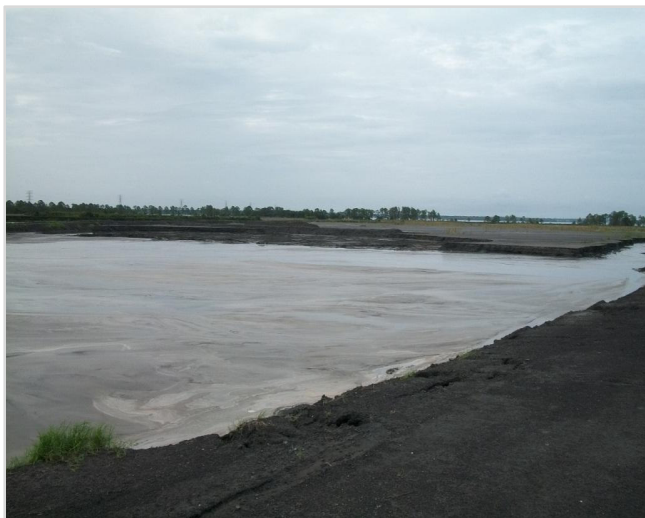
Photo 1 Ash Pond near North West Access Road - looking South East
