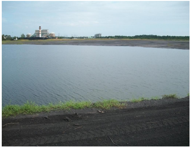
Photo 18 Ash Pond at internal dike on South embankment - looking North West
