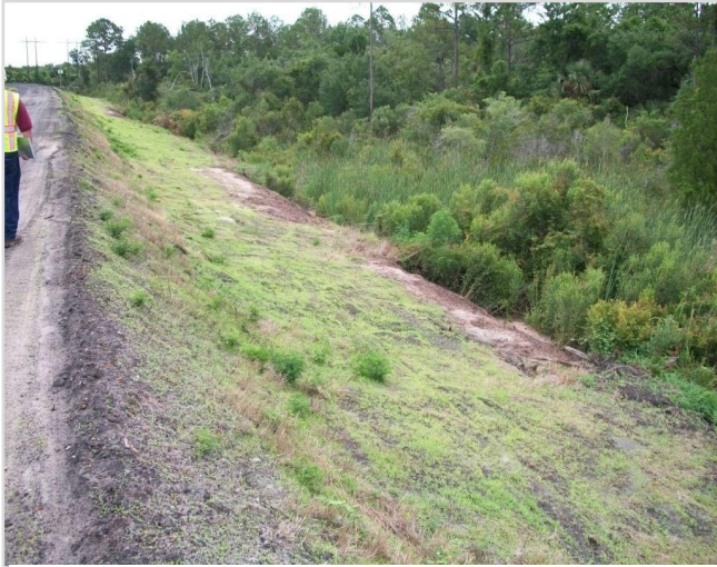
Photo 22 South embankment – looking East
