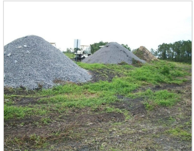
Photo 14 Emergency repair stockpile at South West corner of pond
