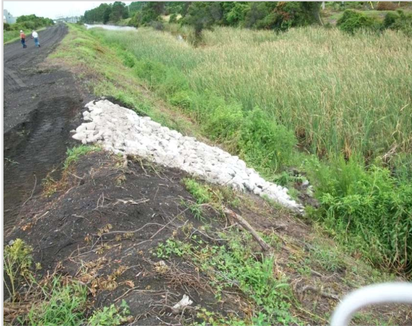
Fig. 5.2.3-2. Rip rap repair on downstream slope of north embankment.
