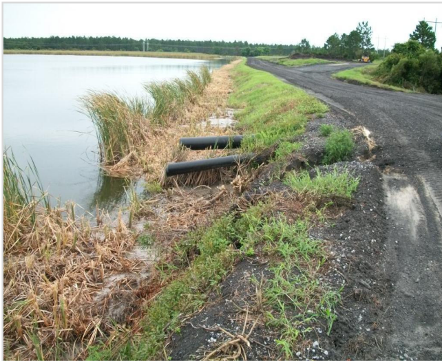
Photo 24 East embankment – looking North - note inflow pipe from stormwater management facility
