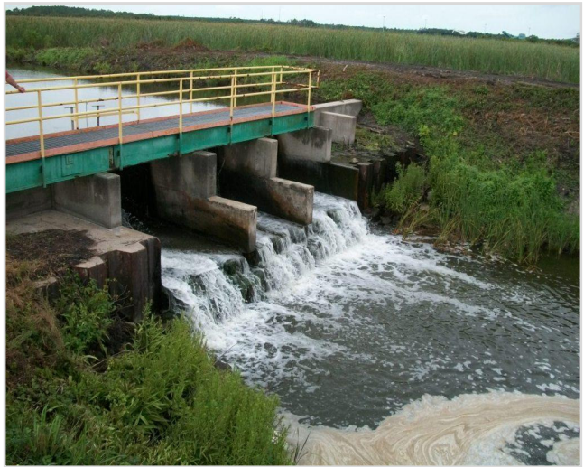
Photo 27 Ash Pond outfall weir
