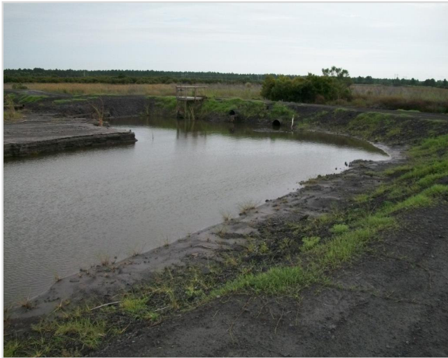
Photo 19 Internal drainage near center of South embankment
