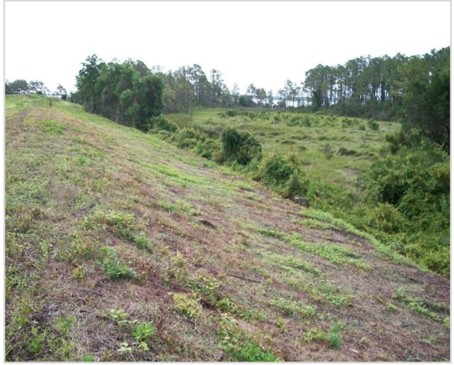
Photo 16 South embankment - looking East
