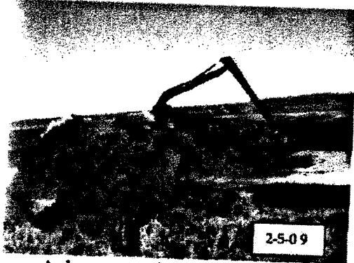
Ash removal maintenance operations and dewatering in ponds
