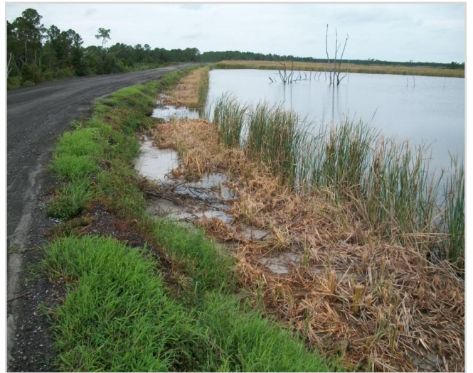
Photo 25 South embankment – looking West
