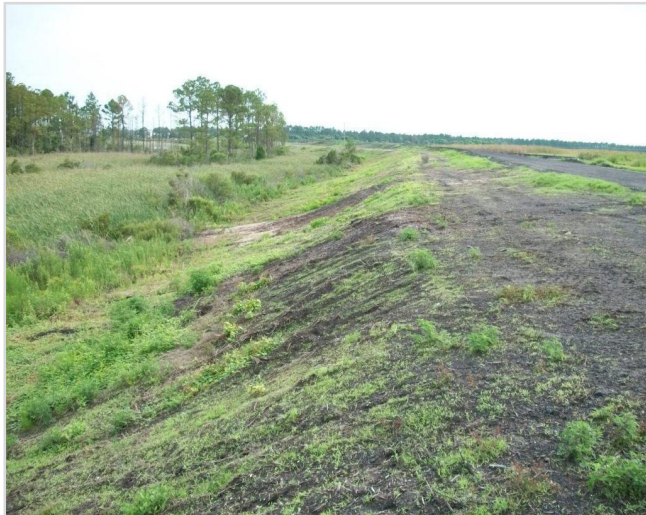
Photo 13 West embankment at South West corner – looking North note slope rilling
