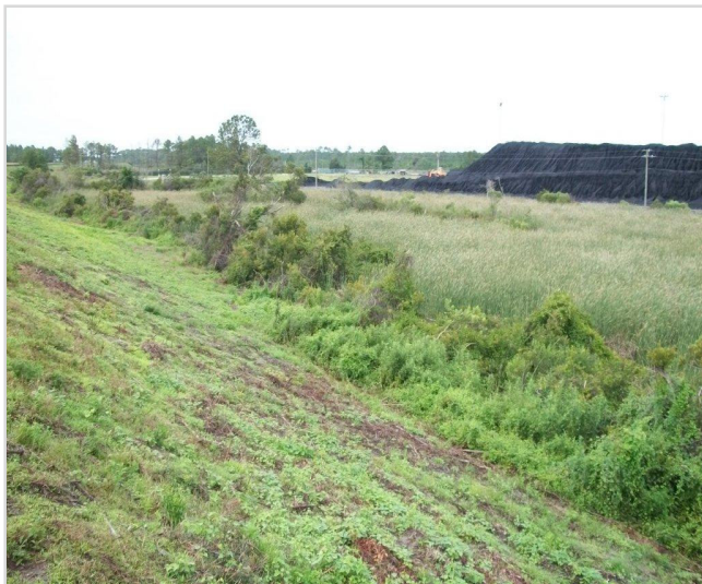
Photo 5 Slope of West Embankment
