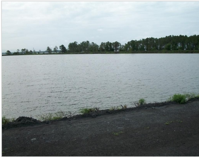
Photo 11 Ash Pond at South West corner – looking South East
