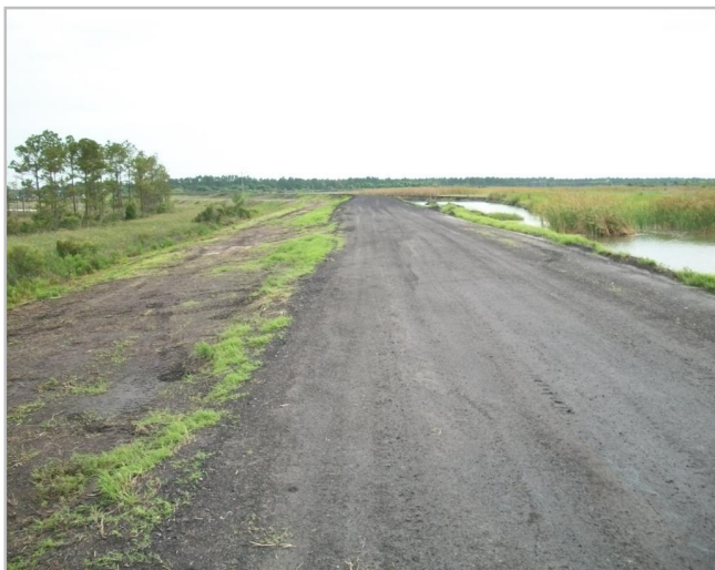
Photo 9 West embankment at South West corner of Ash Pond – looking North
