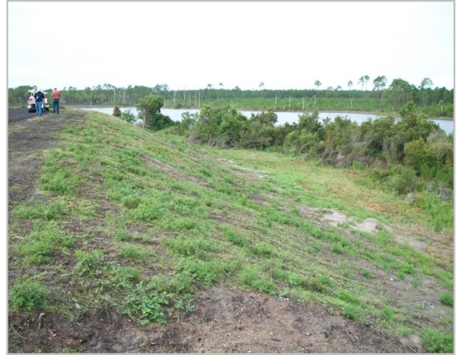
Photo 12 West embankment looking South
