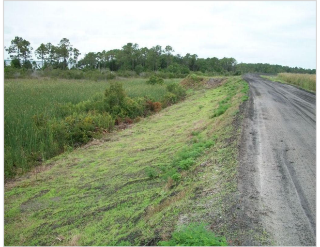
Photo 23 South embankment – looking West
