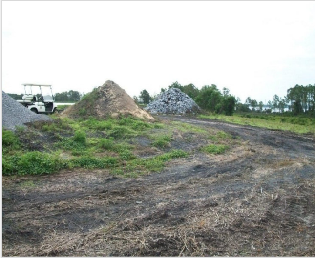
Photo 15 Emergency repair stockpile at South West corner of pond
