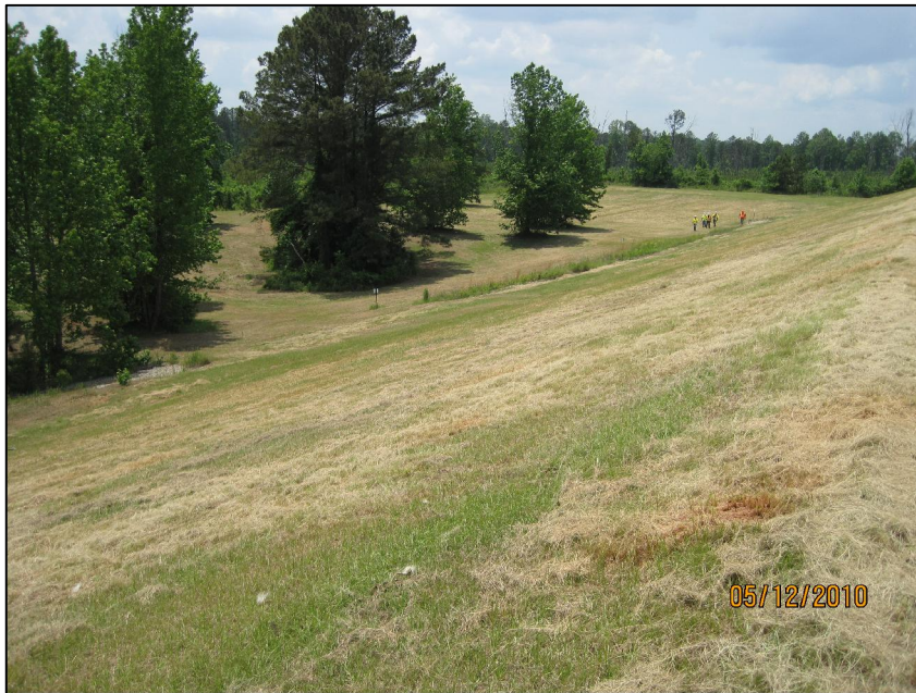
CREST OF SETTLING POND, LOOKING SOUTHWEST AT BLANKET DRAIN AND GROIN AREA OF RIGHT ABUTMENT
