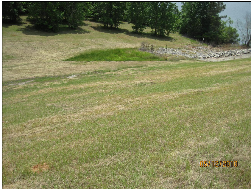
CREST OF SETTLING POND, LOOKING SOUTH AT TOE OF GROIN AREA AT LEFT ABUTMENT, OBSERVED LARGE ANIMAL BURROW AT TOE OF DOWNSTREAM SLOPE IN THIS AREA
