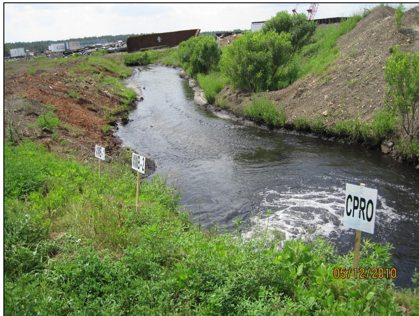
AP-42 SOUTH DIKE, WASTEWATER BASIN (WWB1 AND WWB2) AND COAL PILE RUNOFF OUTLET PIPES
