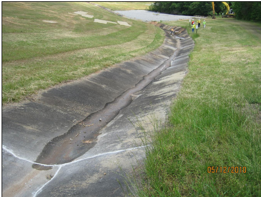
DOWNSTREAM SLOPE OF EAST DIKE, LOOKING NORTH, WATER SEEPING INTO AND BACK OUT OF DITCH AT JOINTS
