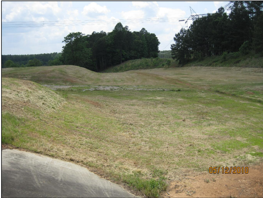
AP-39 LOOKING SOUTH THROUGH EMERGENCY SPILLWAY
