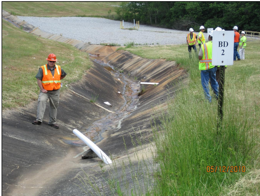
DOWNSTREAM SLOPE OF EAST DIKE, LOOKING NORTH, WATER ENTERING CONCRETE DITCH FROM BD-2 AND BD-3
