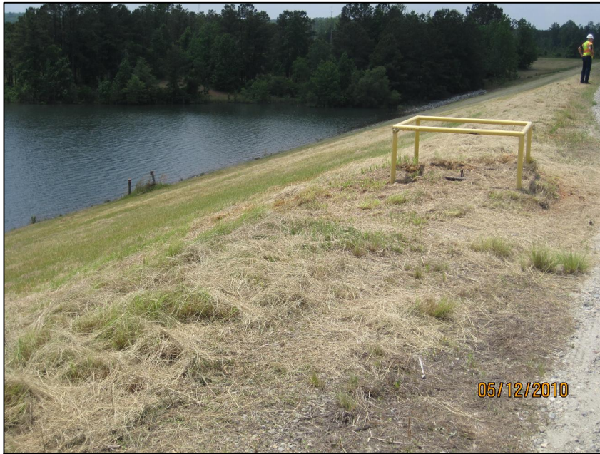
CREST OF SETTLING POND, LOOKING SOUTHWEST AT SETTLEMENT MONUMENT ON CREST AND PZ'S AT DOWNSTREAM TOE (LAKE JULIETTE)
