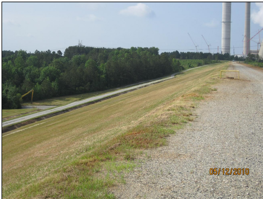
CREST OF EAST DIKE, LOOKING SOUTH (SETTLEMENT MONUMENT #6) REPAIRED SURFACE EROSION AREA (RESEEDED AND MATTED) ON DOWNSTREAM SLOPE AT FAR LEFT OF PHOTO
