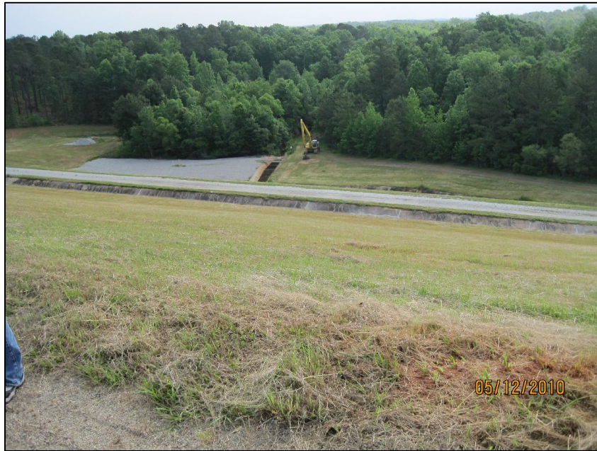
AP-3 CREST OF EAST DIKE, LOOKING EAST AT TOE DRAIN OUTLET
