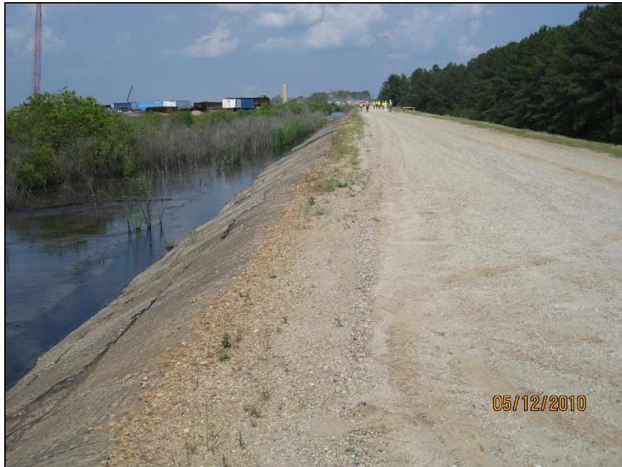
AP-50 SOUTH DIKE, UPSTREAM FABRIFORM SLOPE OF SOUTH DIKE
