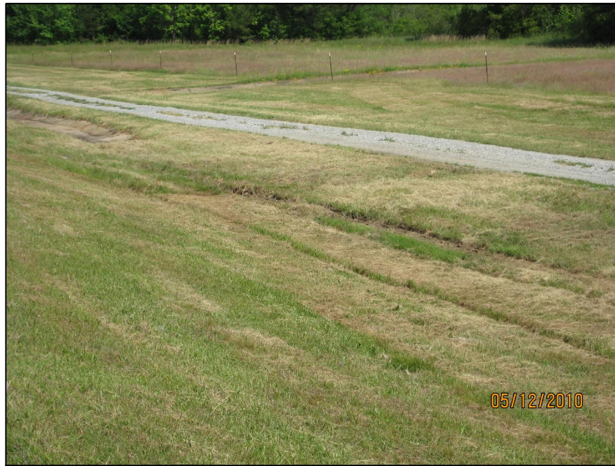
DOWNSTREAM TOE OF NORTH DIKE, APPROX. 125 FEET LONG WET SURFACE AREA AT EAST END OF CONCRETE DITCH
