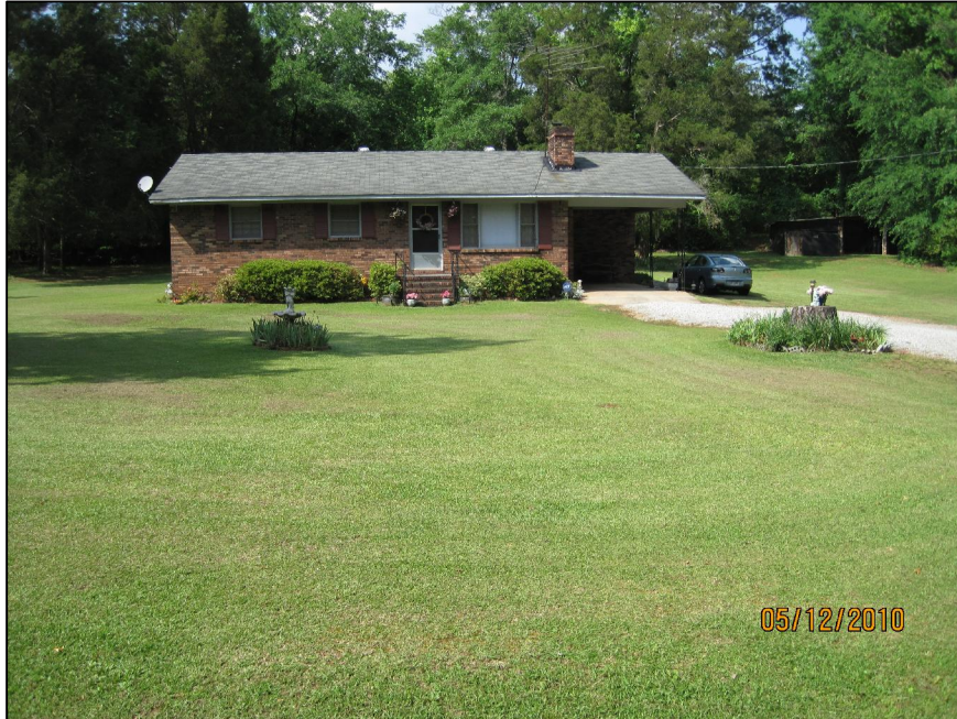
AP-53 LOOKING NORTHEAST AT 2136 LUTHER SMITH ROAD
