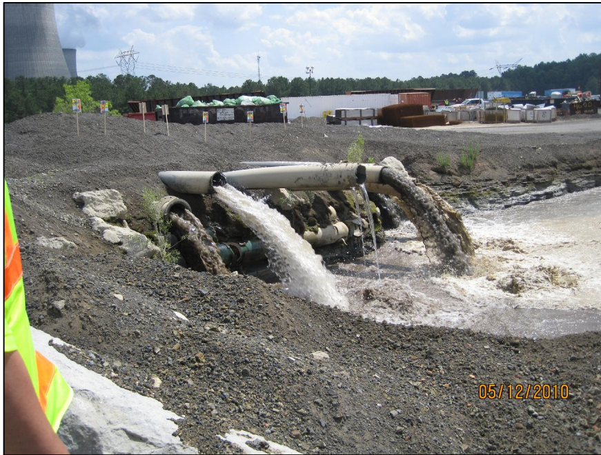
AP-43 SOUTH DIKE, BOTTOM AND TOP ASH SLURRY LINE OUTLET PIPES
