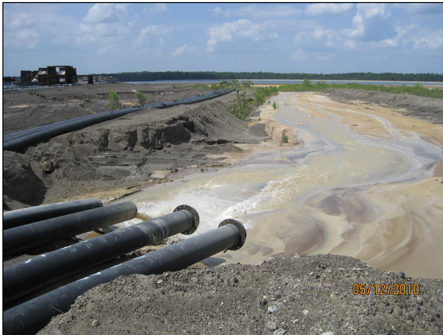
AP-44 SOUTH DIKE, UNITS 1 AND 2 TOP ASH SLURRY LINE OUTLET PIPES
