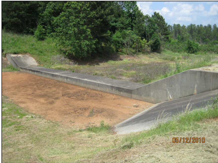
AP-38 EMERGENCY SPILLWAY
