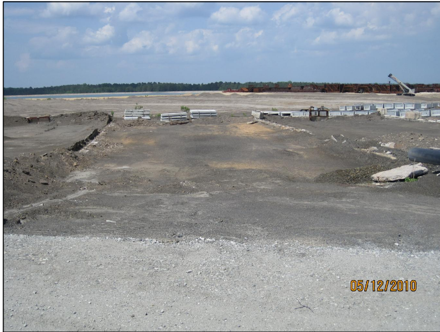
AP-45 SOUTH DIKE, LOOKING NORTH AT ASH POND
