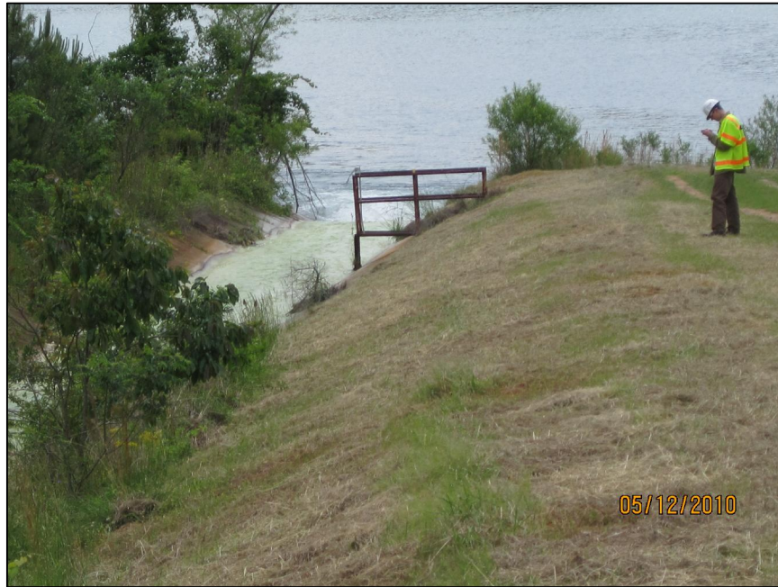
AP-41 LOOKING SOUTH AT ASH POND OUTLET TO SETTLING BASIN
