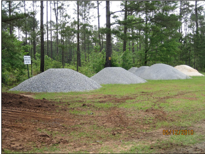
AP-23 EAST OF DOWNSTREAM TOE OF EAST DIKE, EMERGENCY SUPPLIES
