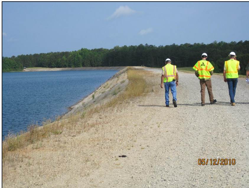
INTERSECTION OF CREST OF EAST AND NORTH DIKE LOOKING NORTHWEST, LEFT: UPSTREAM FABRIFORM SLOPE OF NORTH DIKE, FAR LEFT: NORTH DIKE ABUTMENT TIE-IN
