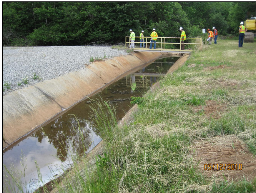
AP-29 DOWNSTREAM TOE OF EAST DIKE, LOOKING EAST, BLANKET DRAIN OUTLET
