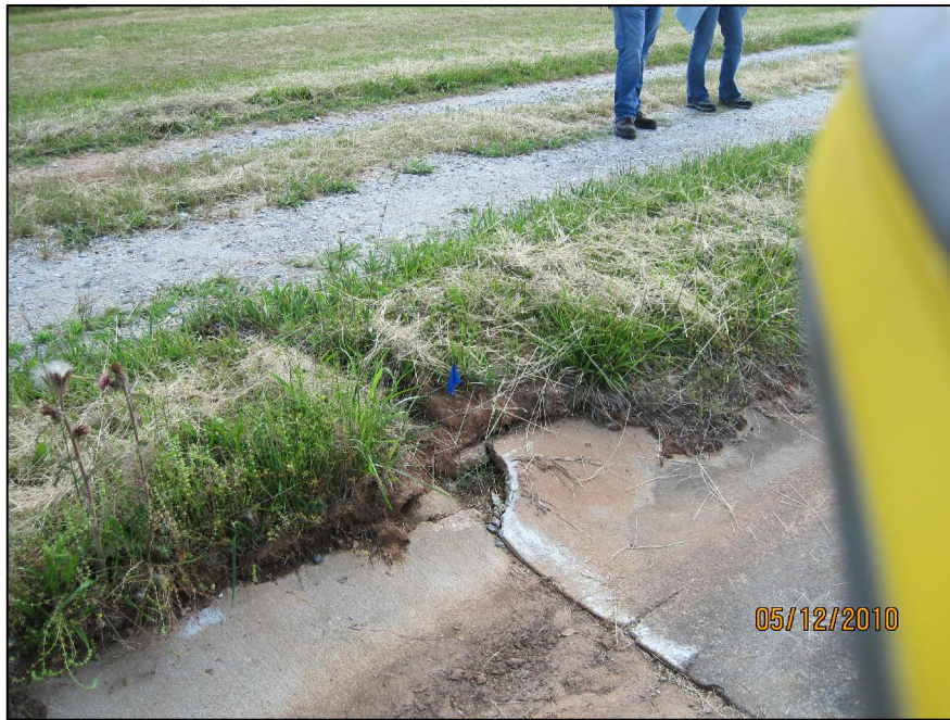
DOWNSTREAM TOE OF NORTH DIKE, MINOR EROSION AND BROKEN CONCRETE DITCH
