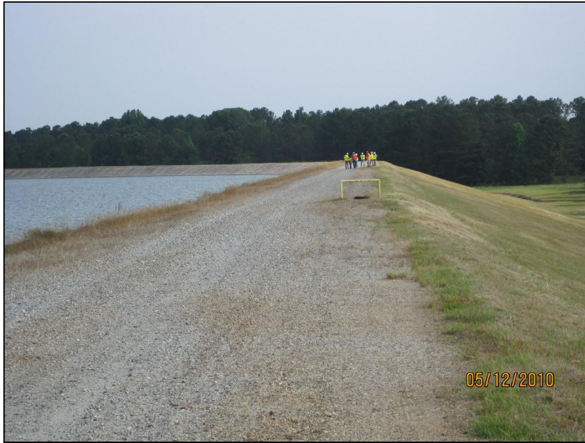
CREST OF EAST DIKE, LOOKING NORTH AT SETTLEMENT MONUMENT #6 AND #7) LEFT:UPSTREAM FABRIFORM SLOPE OF SOUTH END OF NORTH DIKE, RIGHT:DOWNSTREAM SLOPE OF NORTH END OF EAST DIKE
