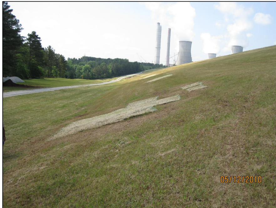
DOWNSTREAM SLOPE OF EAST DIKE, LOOKING SOUTH AT REPAIRED AREAS ON SLOPE
