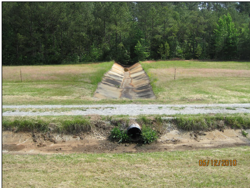
DOWNSTREAM TOE OF NORTH DIKE, LOOKING NORTHEAST AT TOE DRAIN OUTLET
