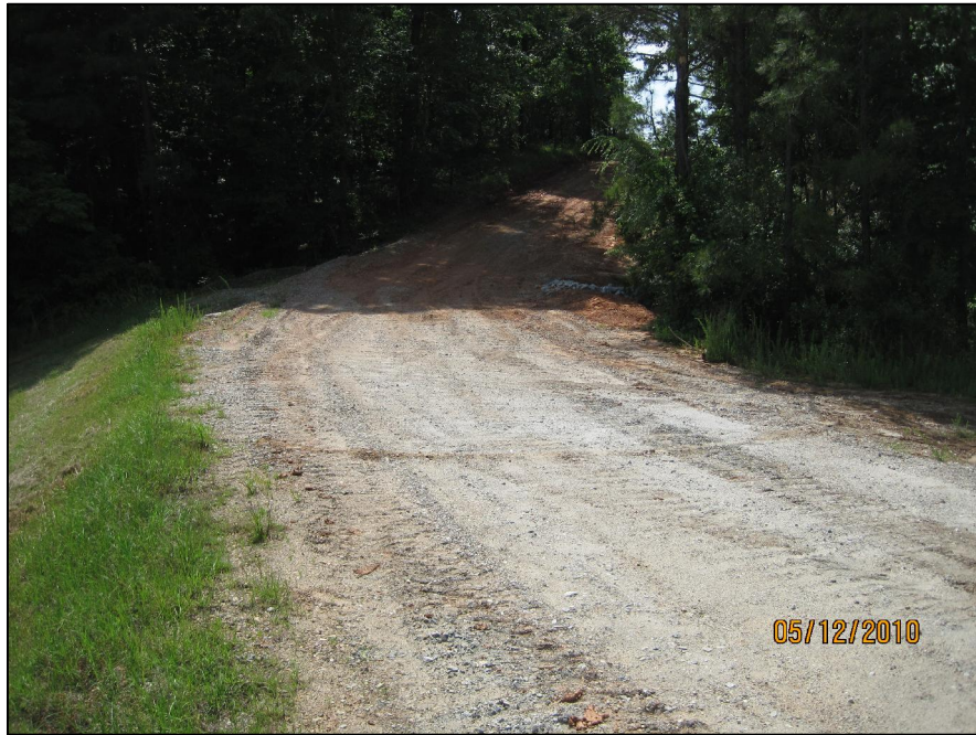
AP-49 SOUTH DIKE, TIE-IN OF RIGHT ABUTMENT
