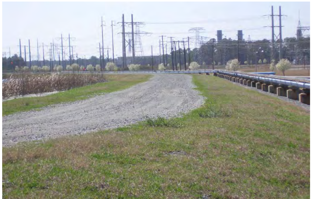
Figure 5.2.1-1 – West Embankment Crest
