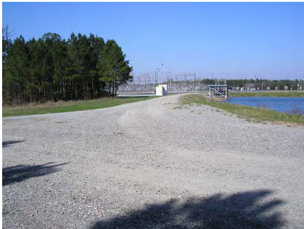
Figure 5.4.1-1 – South Embankment Crest at East End
