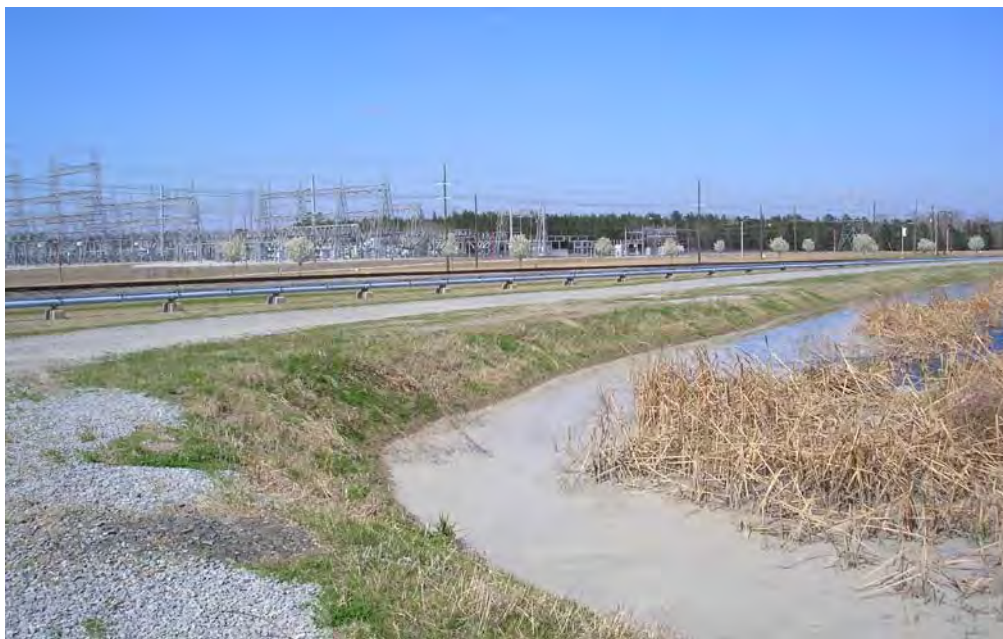
Figure 5.2.2-1 – Inside Slope of West Embankment at South Groin
