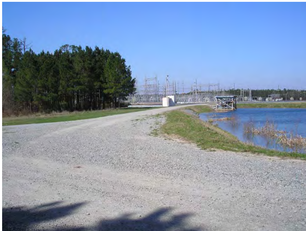
Figure 5.4.3-1 – South Embankment Downstream Slope (Left Side of Gravel Surfaced Crest).
