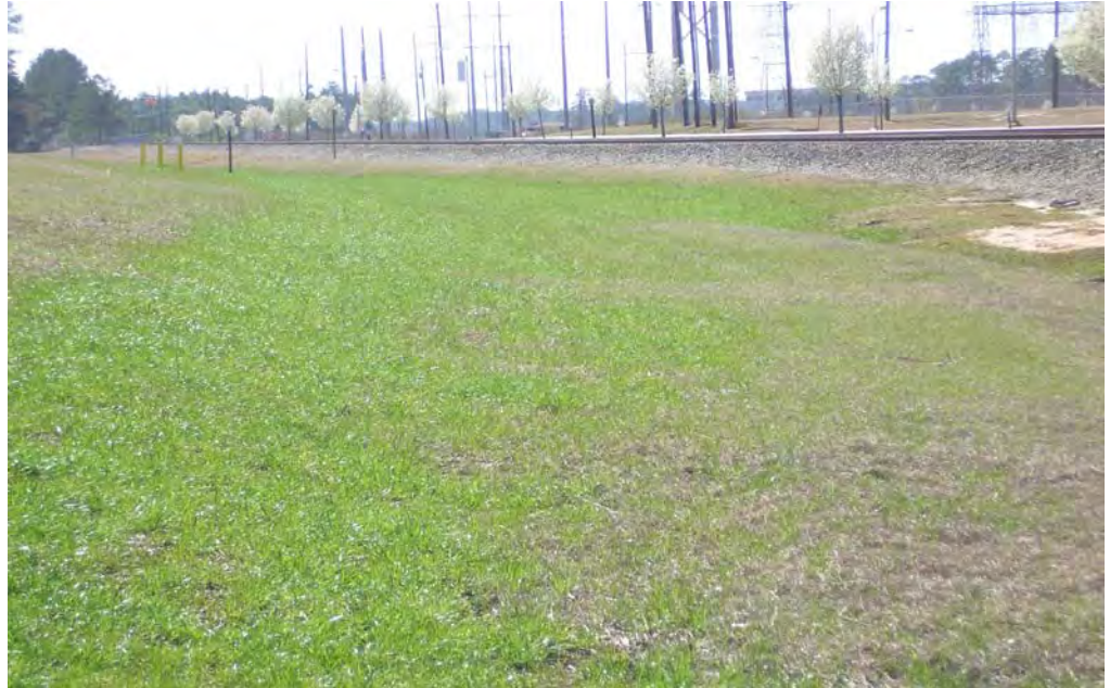
Figure 5.2.3-1 – West Embankment Outside Slope
