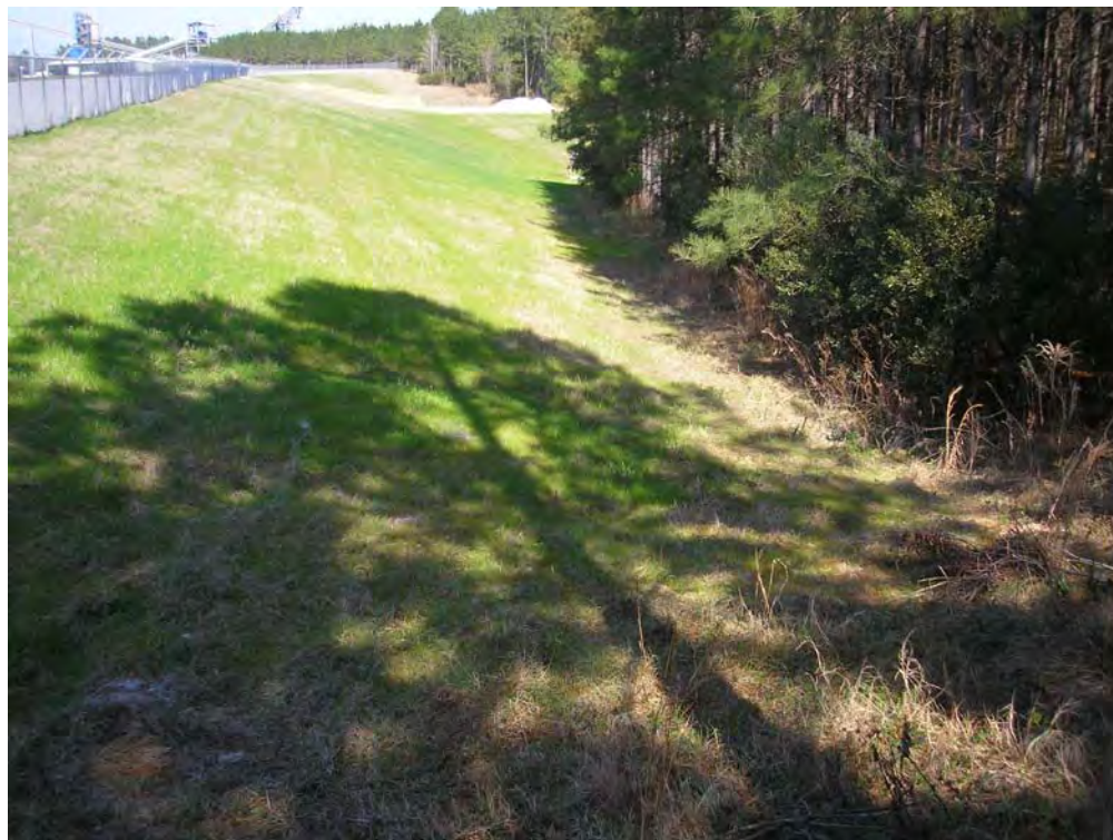
Figure 5.3.3-1 – East Embankment Outside Slope
