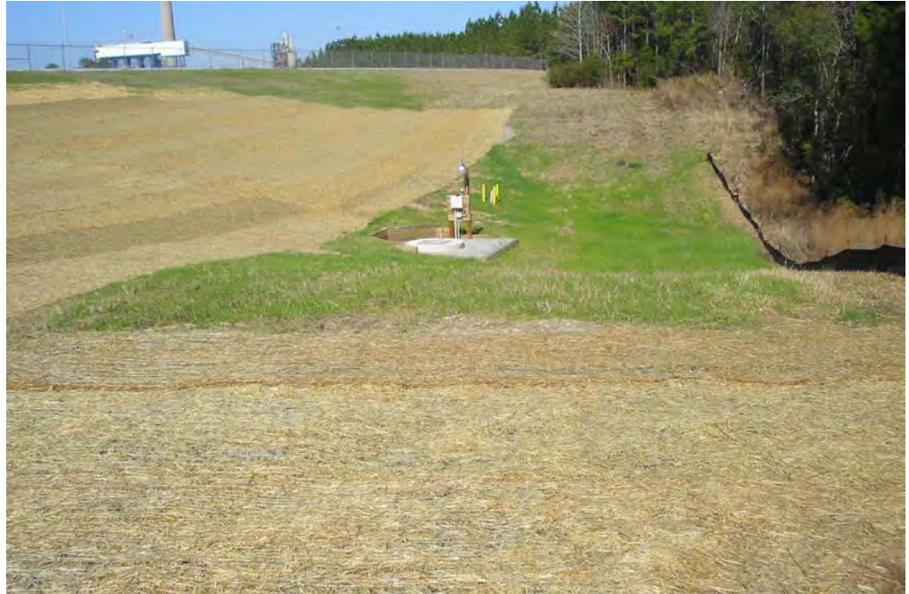
Figure 5.3.3-2 East Embankment Area of New Subsurface Drainage System
