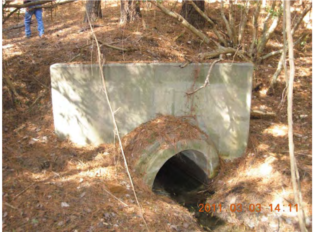
Figure 5.6.2-1 – Primary Spillway Outlet Conduit Discharge
