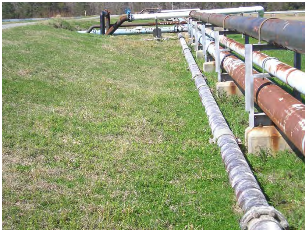
Figure 5.5.3-1 – North Embankment Outside Slope.
