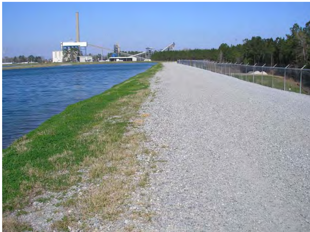
Figure 5.3.1-1 – Crest of East Embankment near South End
