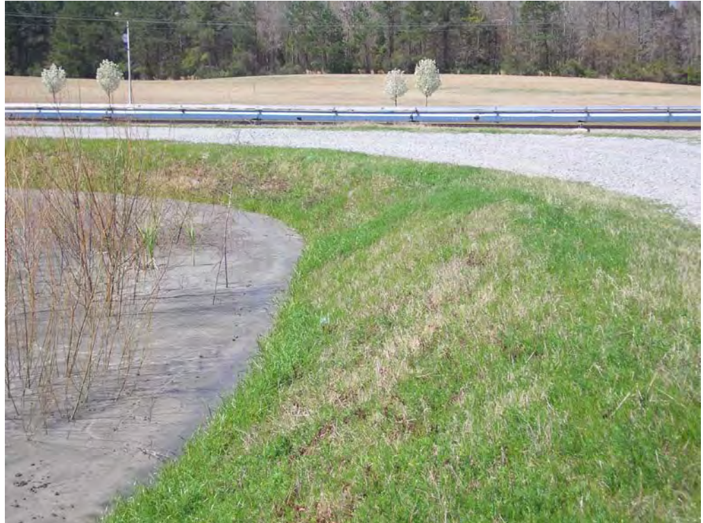
Figure 5.2.4-1 – West Embankment Inside Groin at North End
