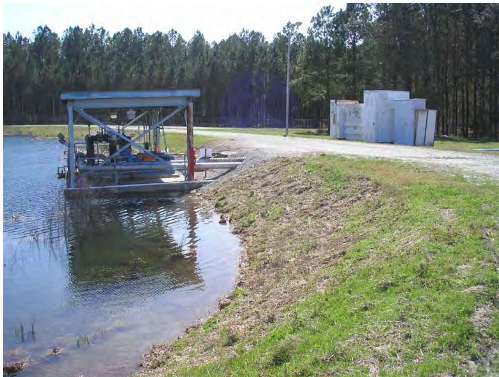
Figure 5.4.2-1: South Embankment Inside Slope
