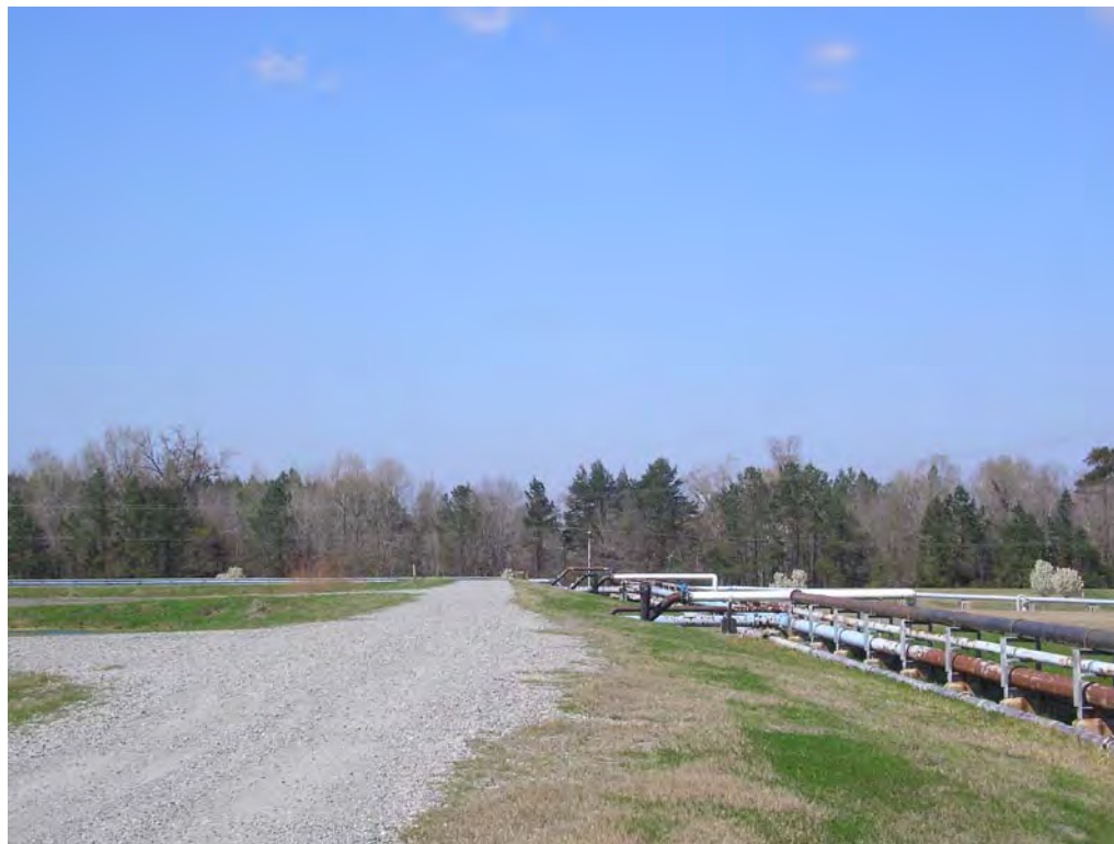
Figure 5.5.1-1 – North Embankment Crest and Outside Slope
