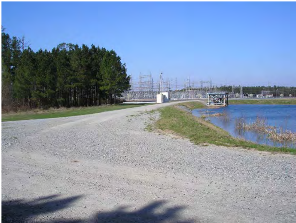
Figure 5.3.4-1 East Embankment Inside Groin at South End (East Embankment on Right Side of Photograph)
