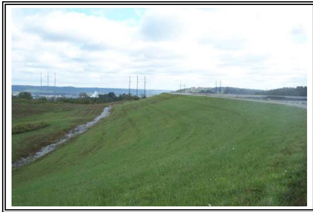
Downstream slope of ATB #2 looking east.
