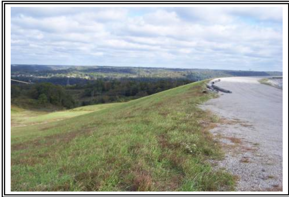
Downstream slope from access road looking northeast.
