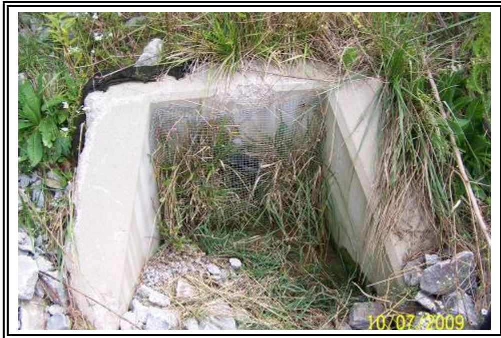
Toe drain at base of main fill.
