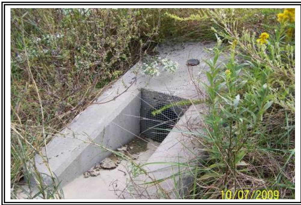
Upper toe drain at east side of main drainage fill (dry).
