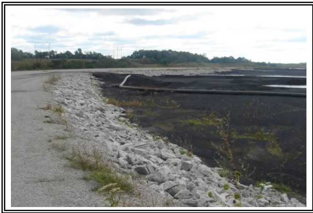
Upstream slope of ATB #2 looking southeast towards east abutment.
