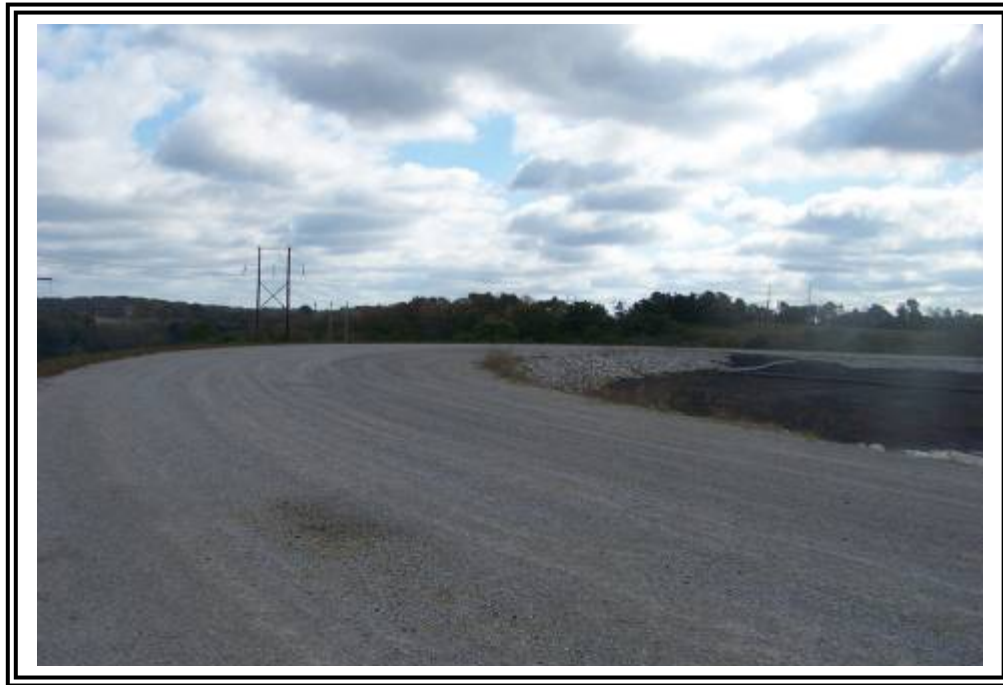
Crest of ATB #2 looking southeast.
