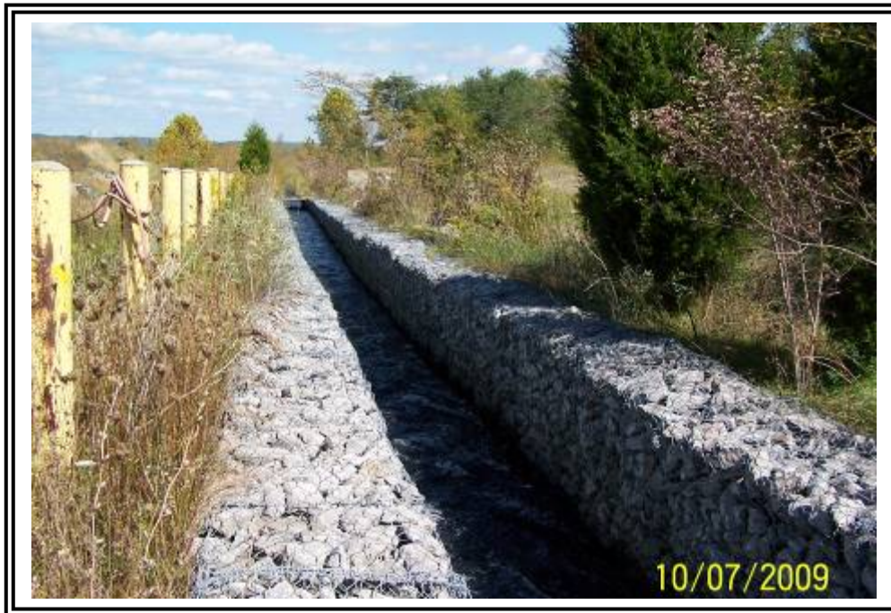
Sluiceway from ATB #2 discharge into ATB #1.
