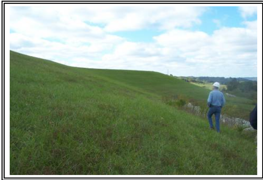
Downstream slope of ATB #2 looking west from northeast corner of dike.
