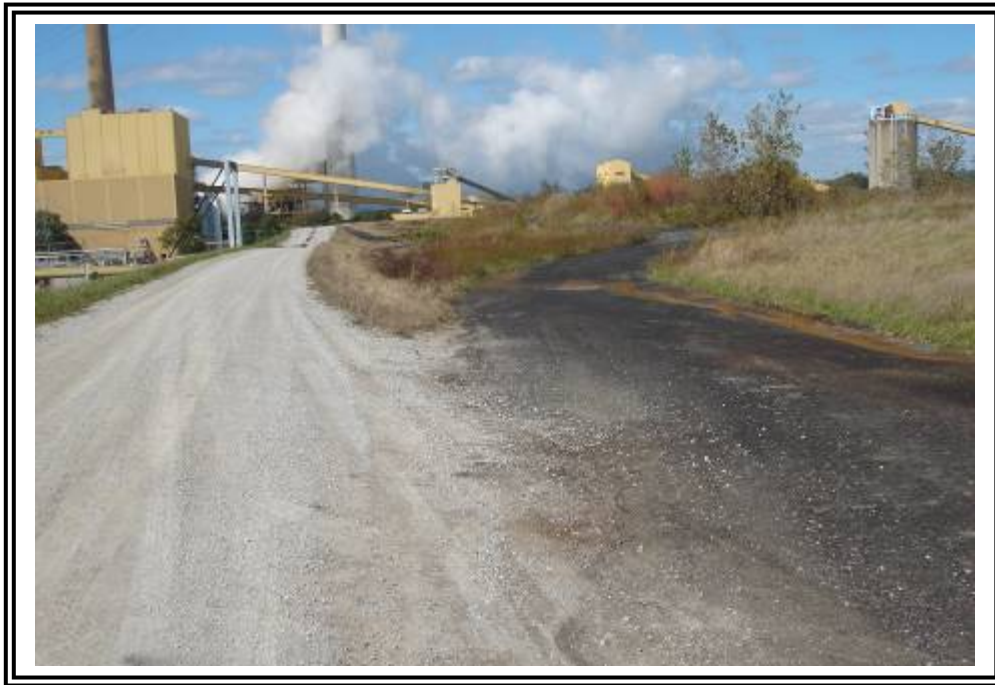
“Upstream” end of ATB #1 at west dike/abutment, looking north.
