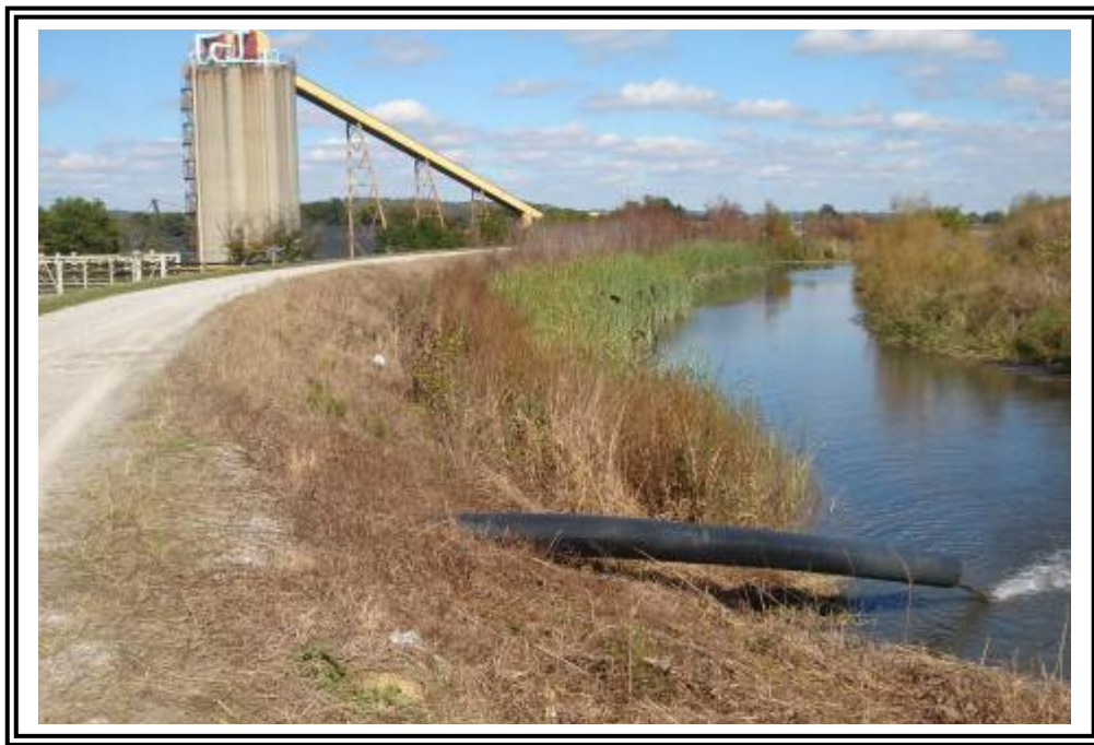
Upstream slope at northwest corner of ATB #1 looking northeast.
