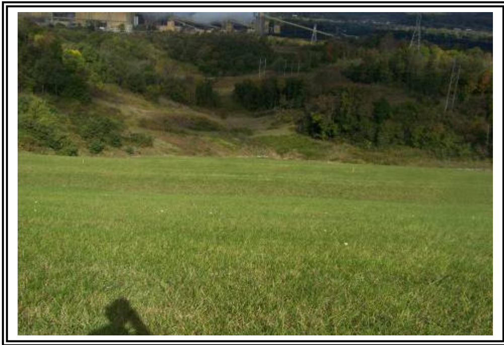
Downstream slope of ATB #2 at the maximum height section looking north.
