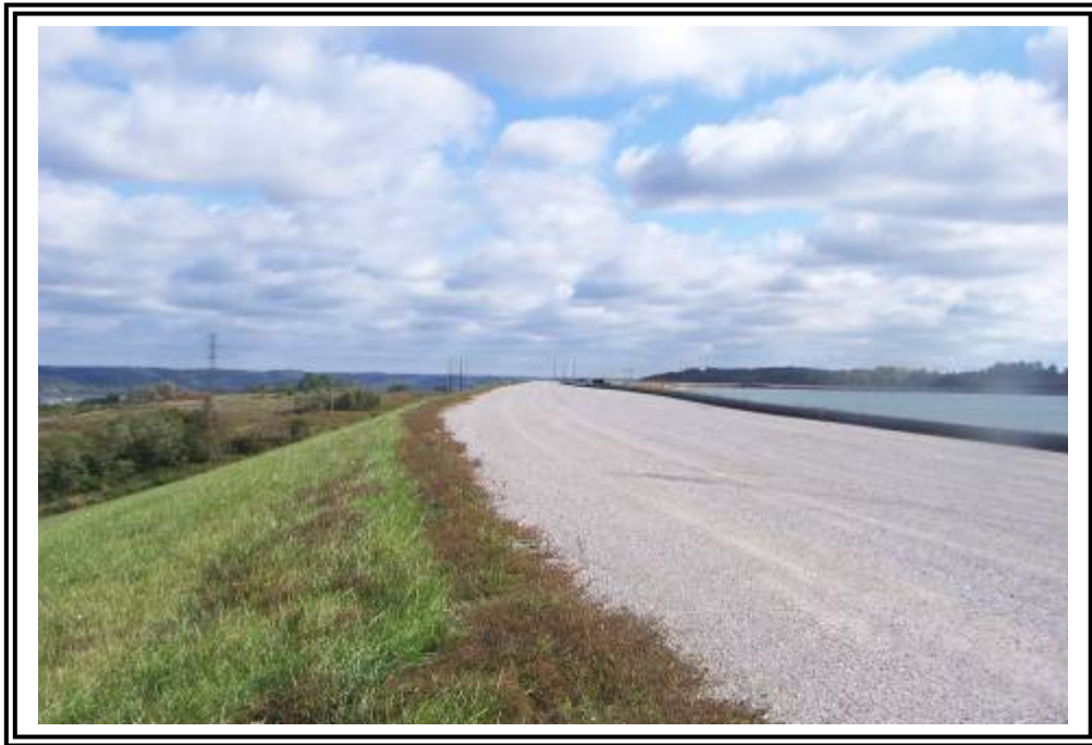
Crest of ATB #2 looking east.
