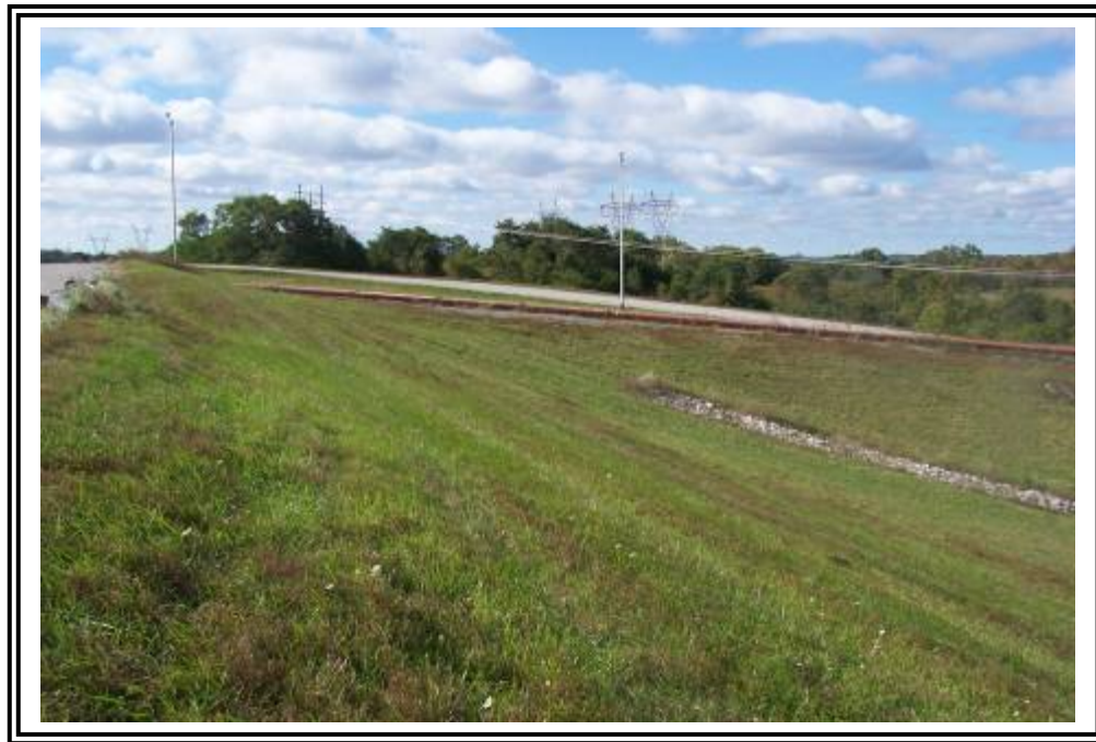
Downstream slope looking west toward access road.
