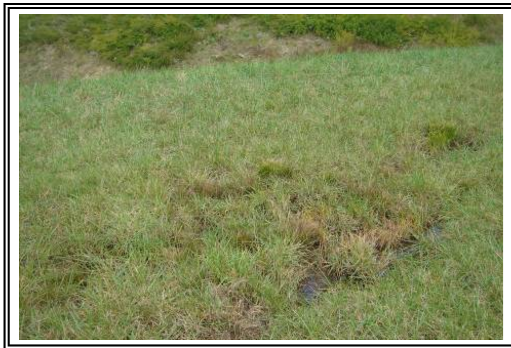
Close up of standing water on upper bench. Soil firm when probed.
