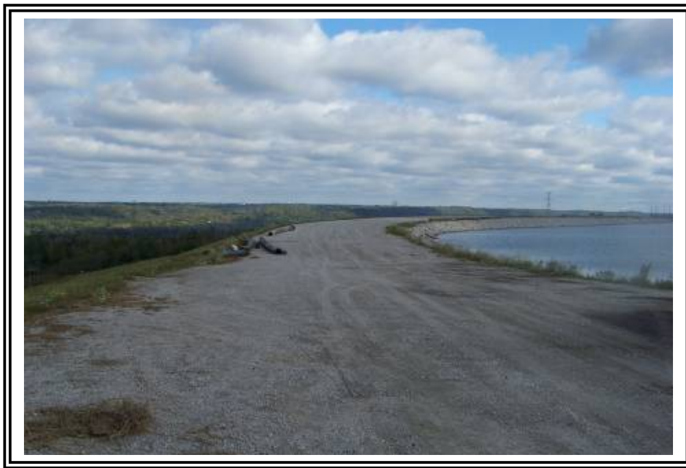
Crest of ATB #2 from access to decant structure looking east.
