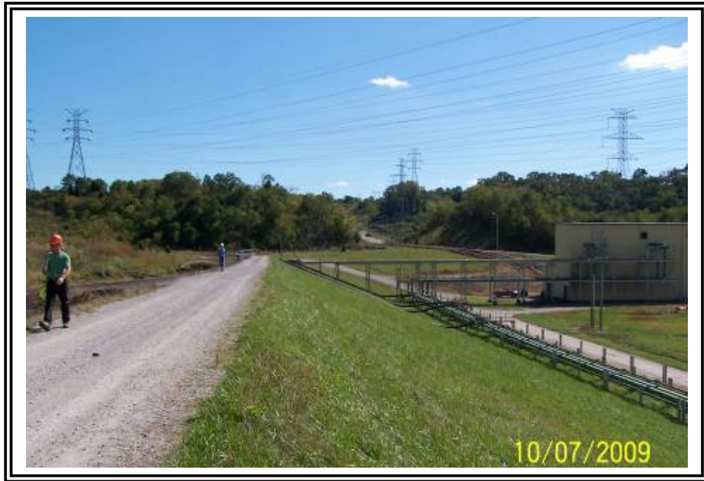
Downstream slope ATB #1 west dike looking south.
