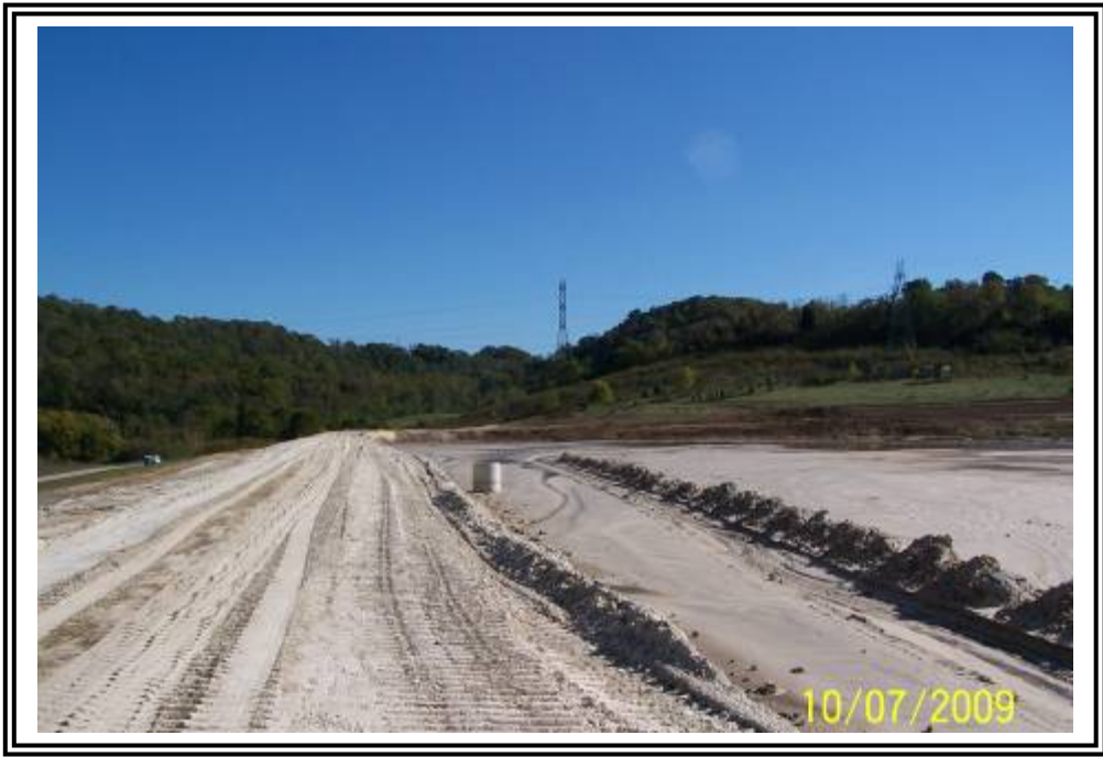
Crest of gypsum stacking facility dike east side, looking south.
