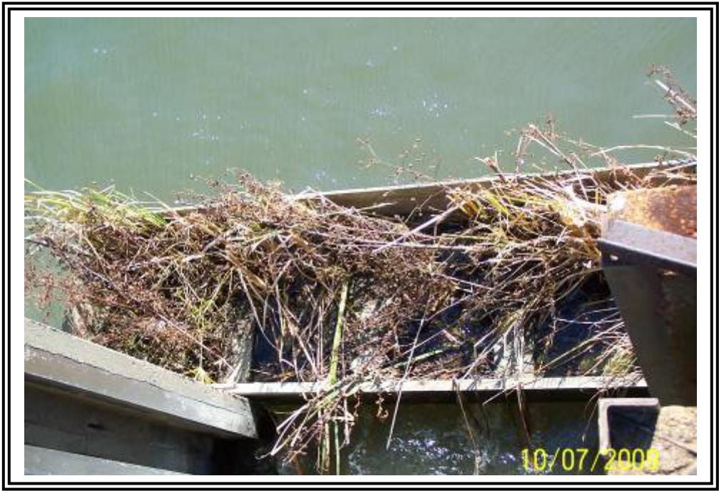
Decant structure in ATB #1.
