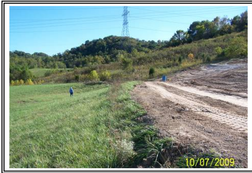
East abutment of gypsum starter dike, looking south.
