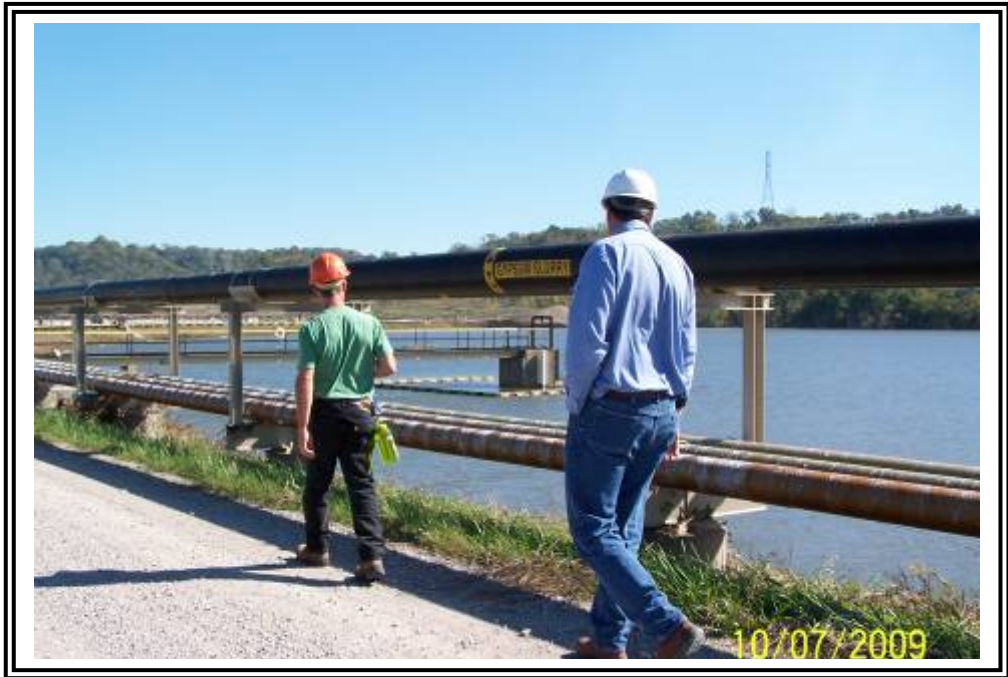
Outlet structure in ATB #1.
