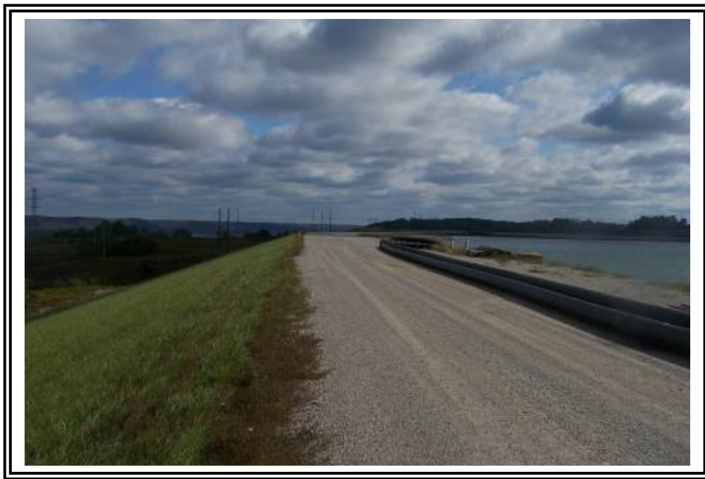
Crest of ATB #2 looking east.
