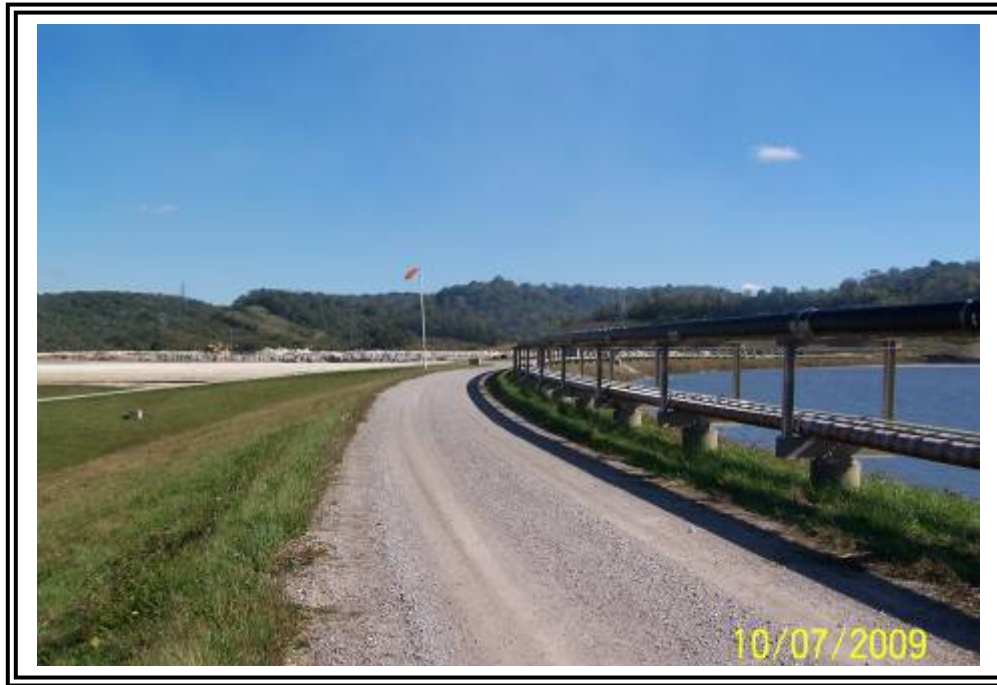
ATB #1 dike crest at northeast corner, looking southeast.
