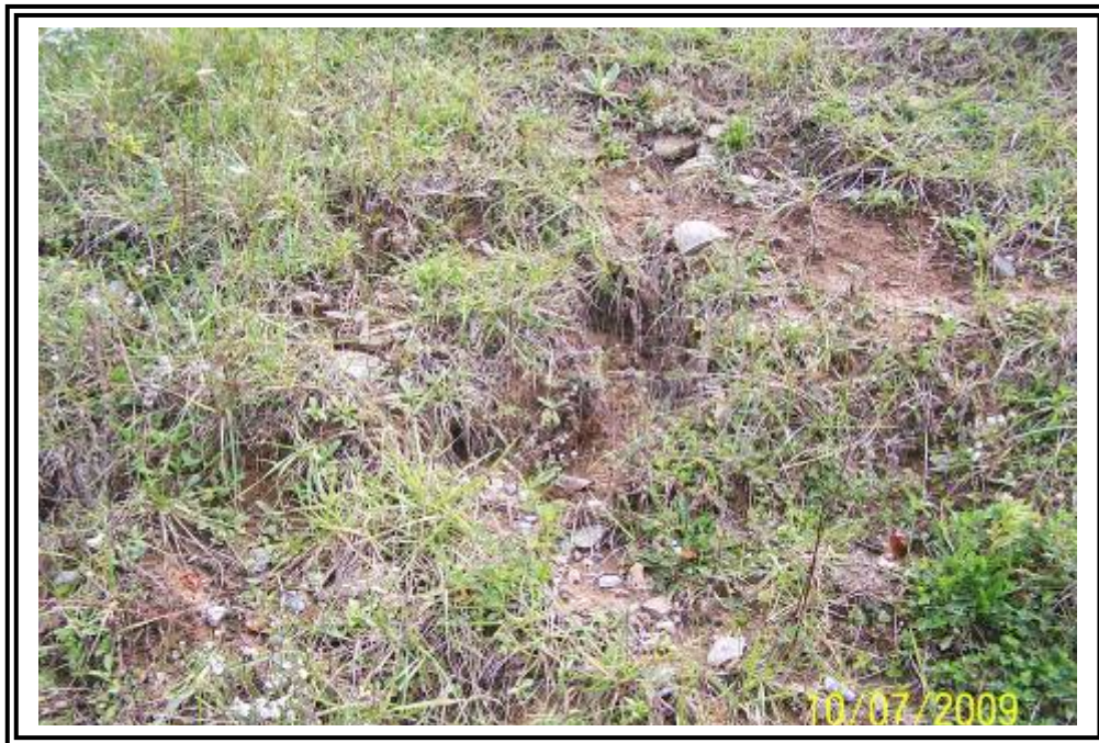
Erosion at occasional locations appears related to turning mowers.
