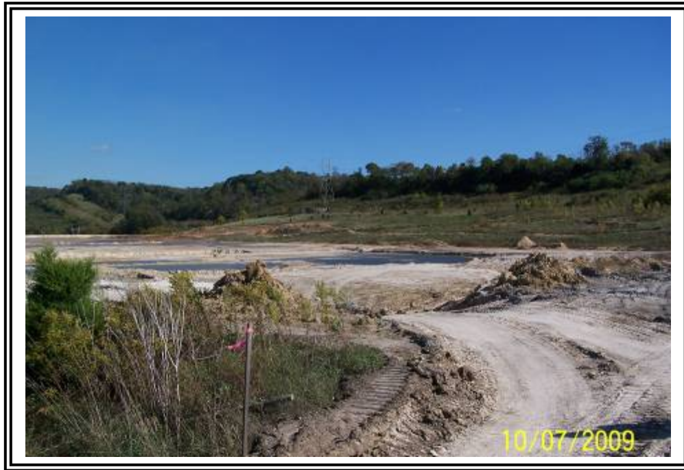
South end of gypsum stacking facility looking southeast.
