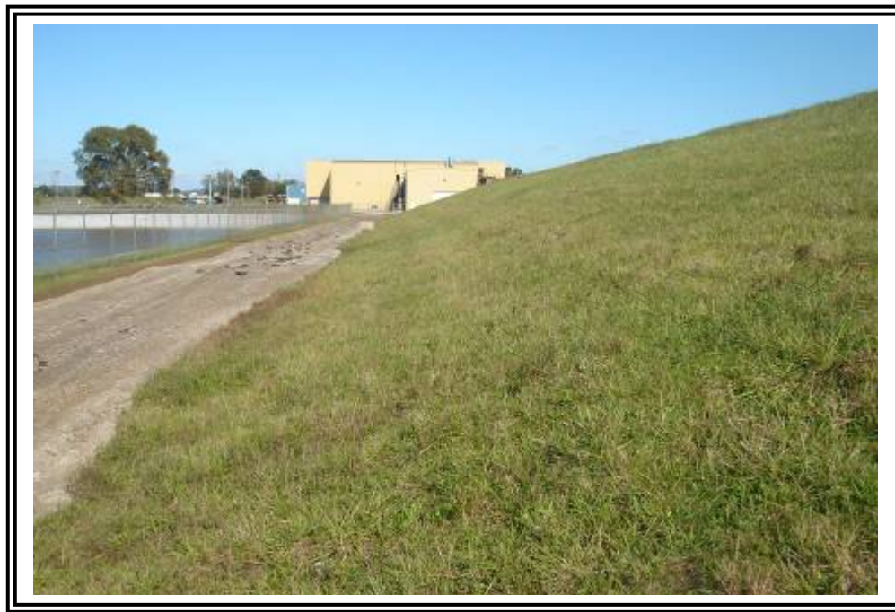
Downstream slope of north side of gypsum stacking facility starter dike (compacted soil), looking east.
