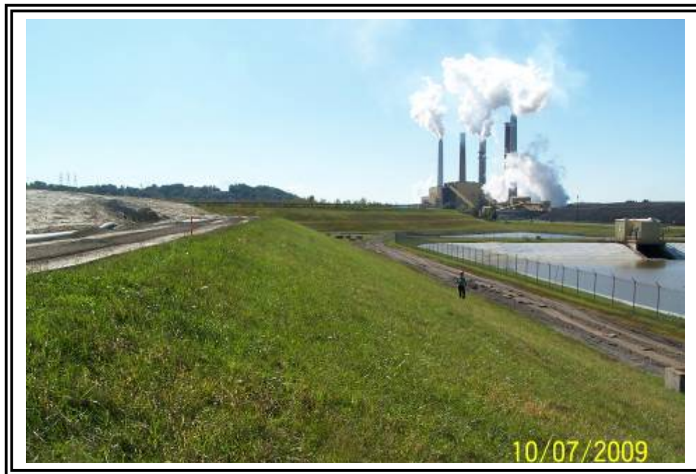
Downstream slope of gypsum stacking facility starter dike at the northeast corner looking west.
