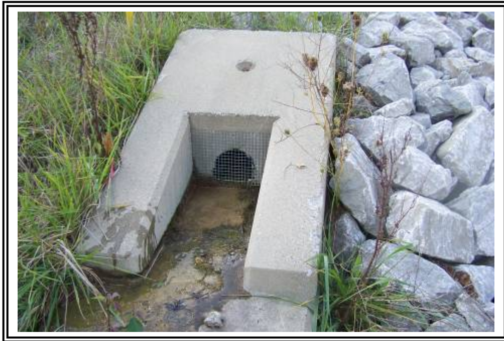
Toe drain on east of ATB #2. Flow clear/immeasurable.
