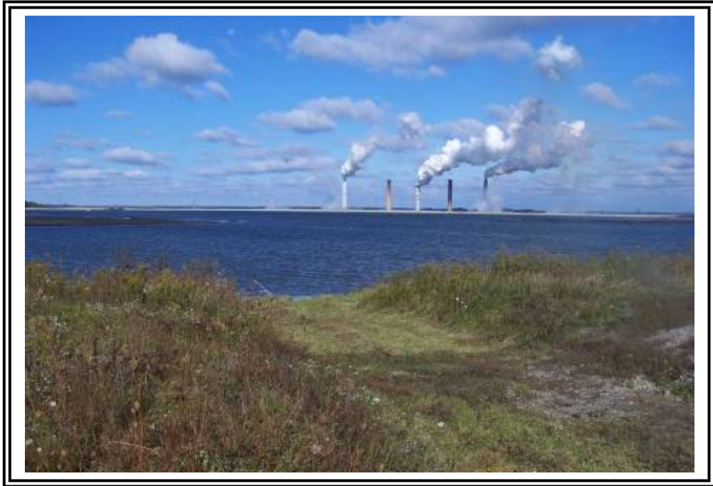
Emergency spillway from south side of ATB #2 looking north.
