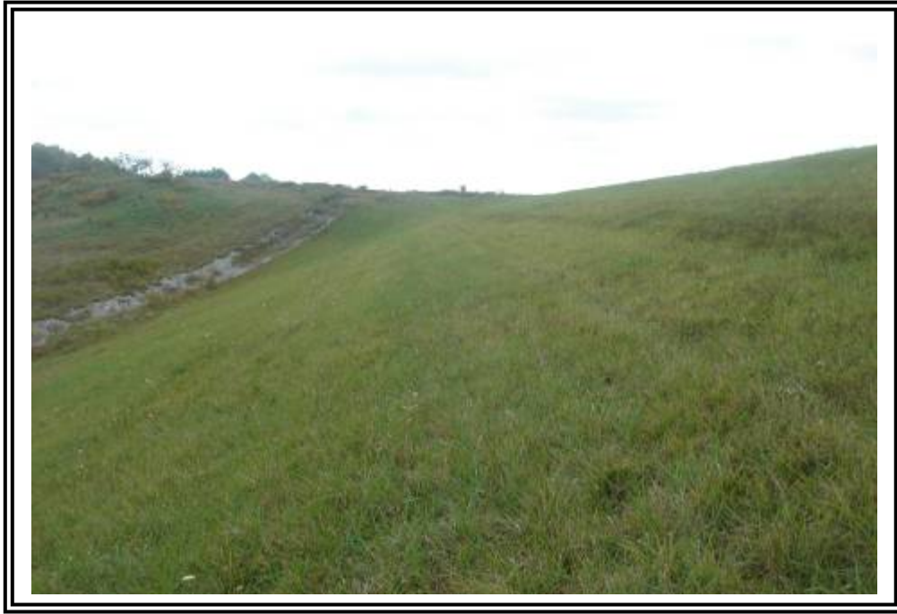
East abutment of ATB #2 looking south.
