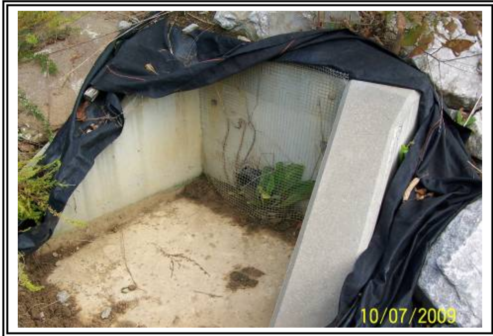
Toe drain above lowest bench of main fill.
