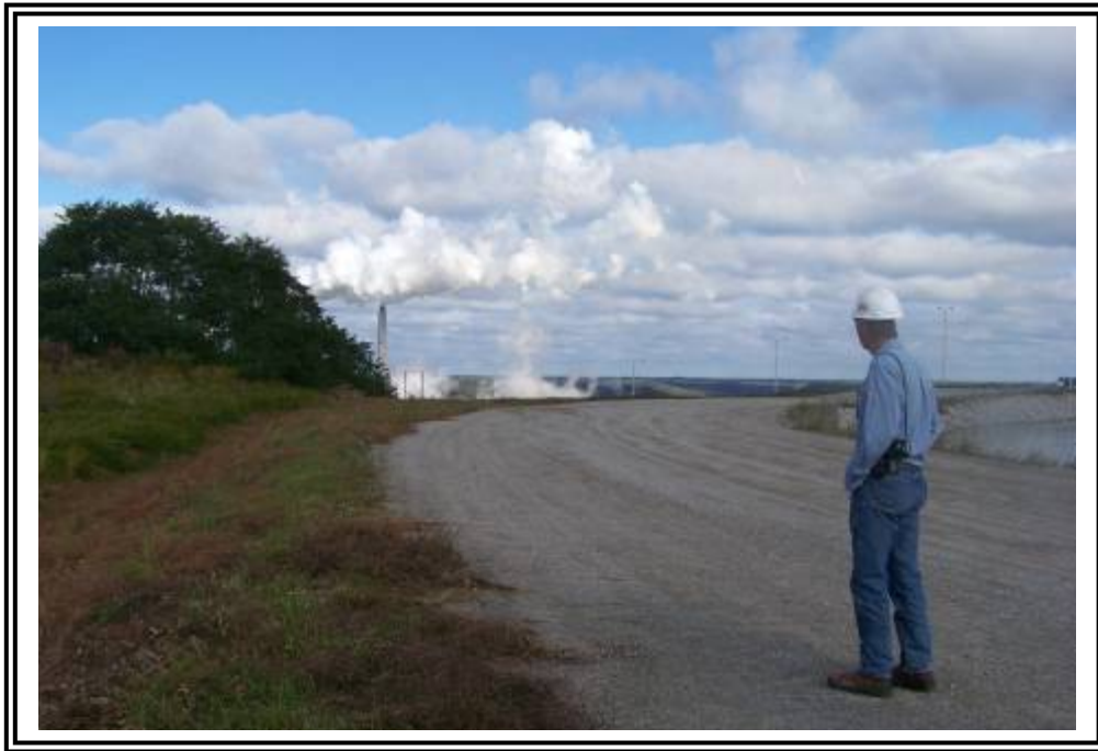
Crest of ATB #2 at west end looking northeast.
