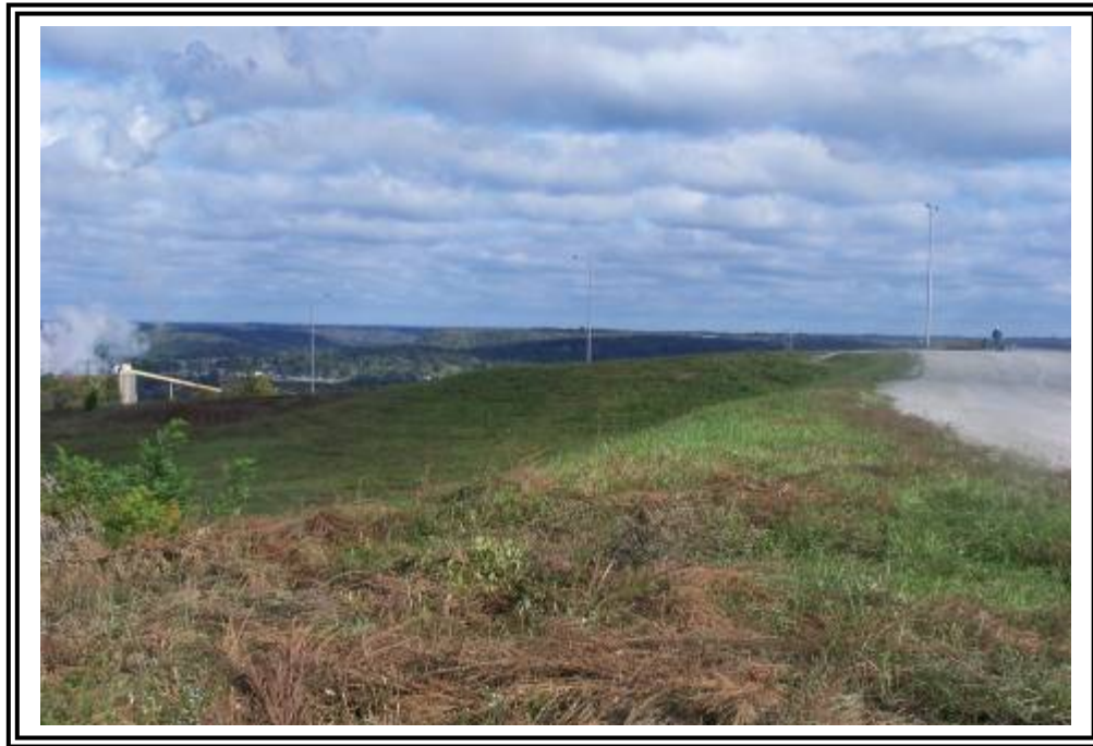
Western knoll looking east toward access road at downstream slope.
