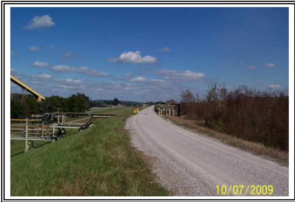
Crest of ATB #1 north dike looking east. Note trees are growing in deposited ash.
