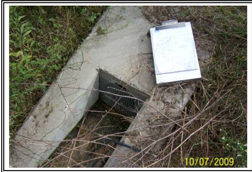
East toe drain at west of main fill.
