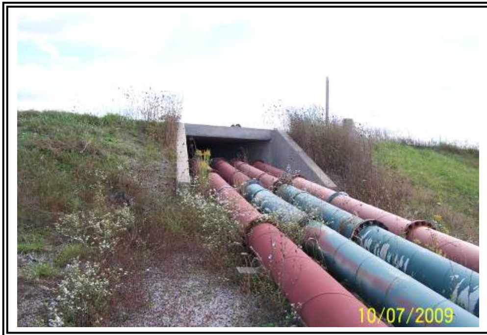
Utilidor of sluice lines at dam crest. Crest slightly higher at this location.
