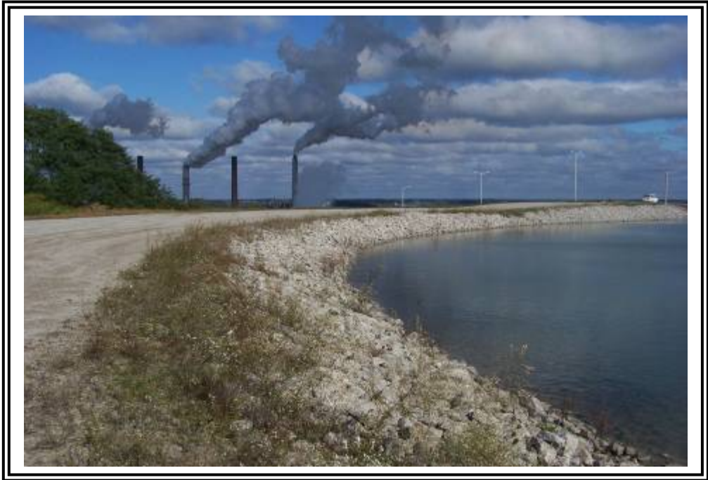
Upstream slope of ATB #2 looking north.
