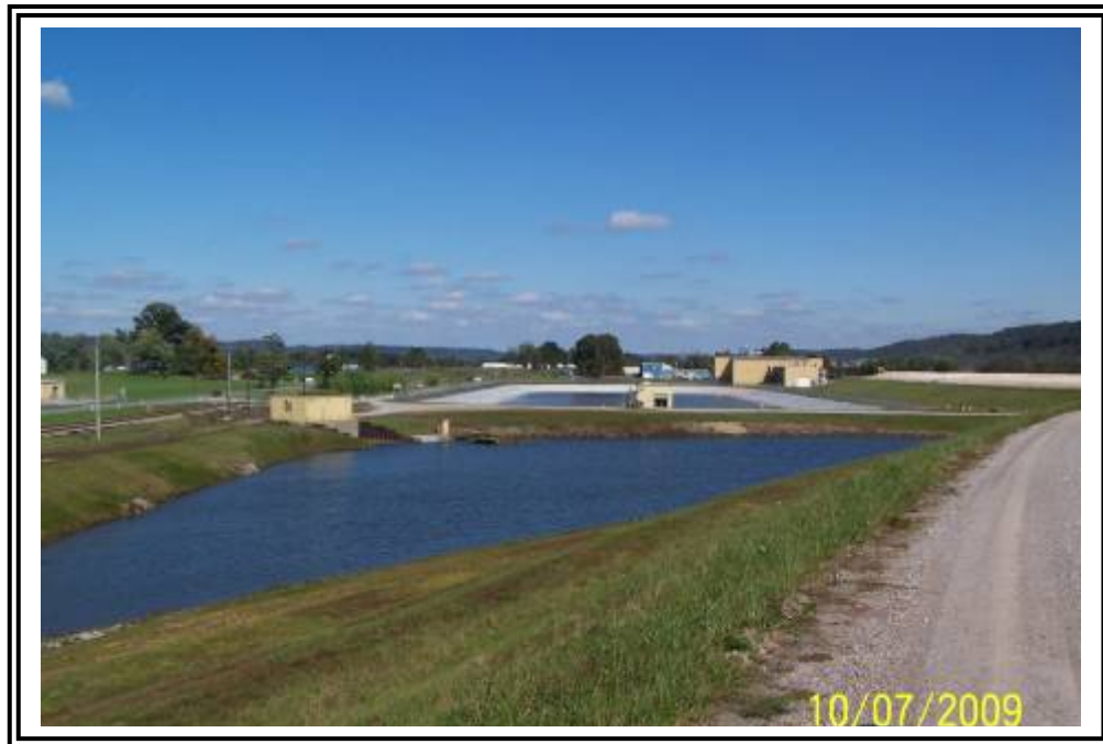
Secondary Ash Treatment basin (foreground) and gypsum stack surge pond (beyond) are incised ponds.
