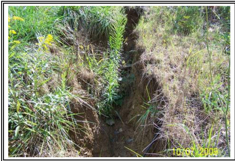
Erosion cut gully in west side of main fill about midway up slope from the base. About 2 feet deep.
