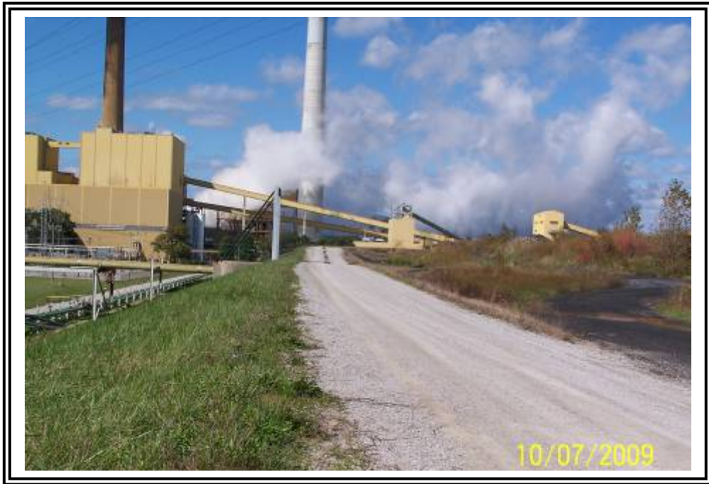
Crest of west dike ATB #1 looking north, "bumpiness" from buried sluice pipe crossing.
