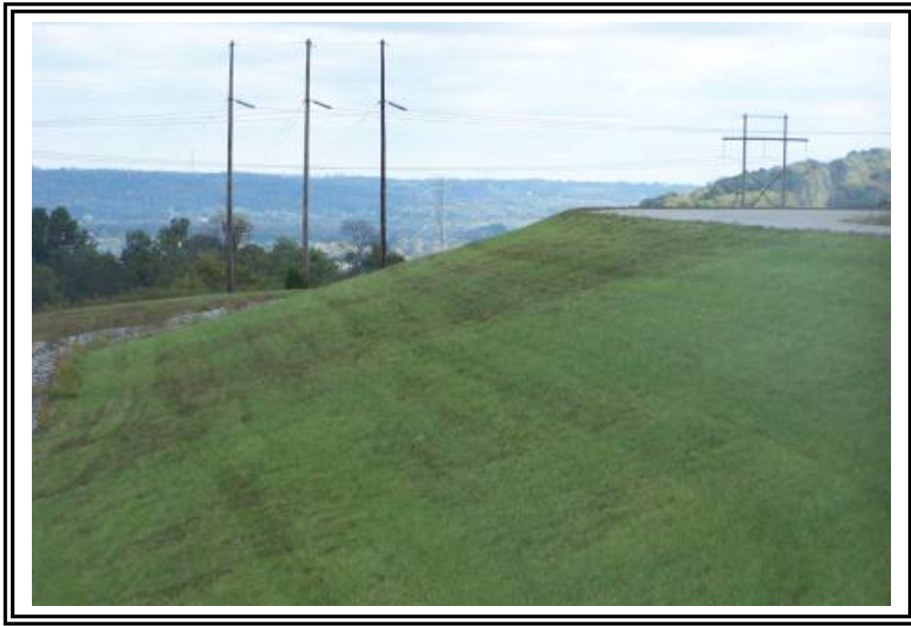
Downstream slope of east end of ATB #2 dike looking northeast.
