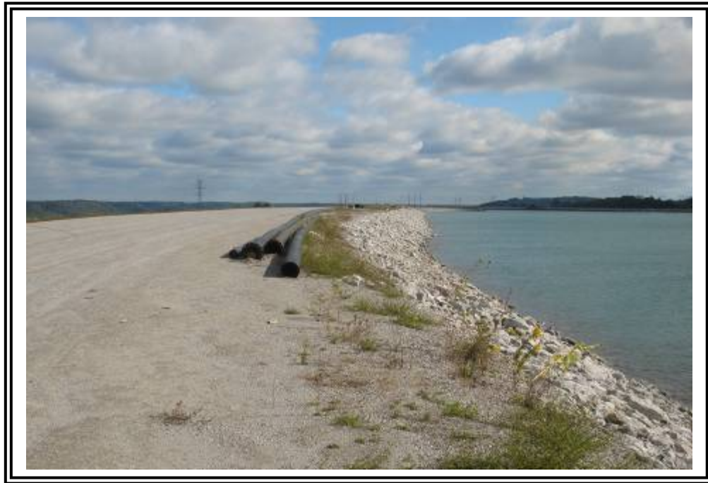
Upstream slope of ATB #2 looking east.
