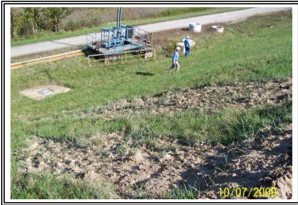
Runoff from gypsum stacking facility east dike under construction.
