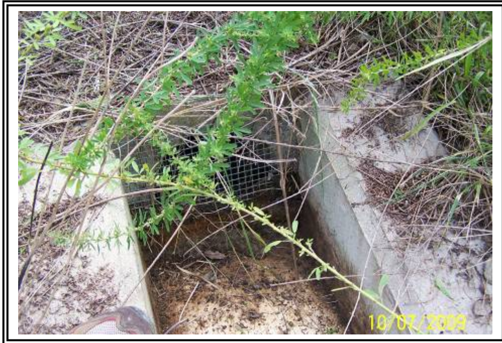
West toe drain at west of main fill.
