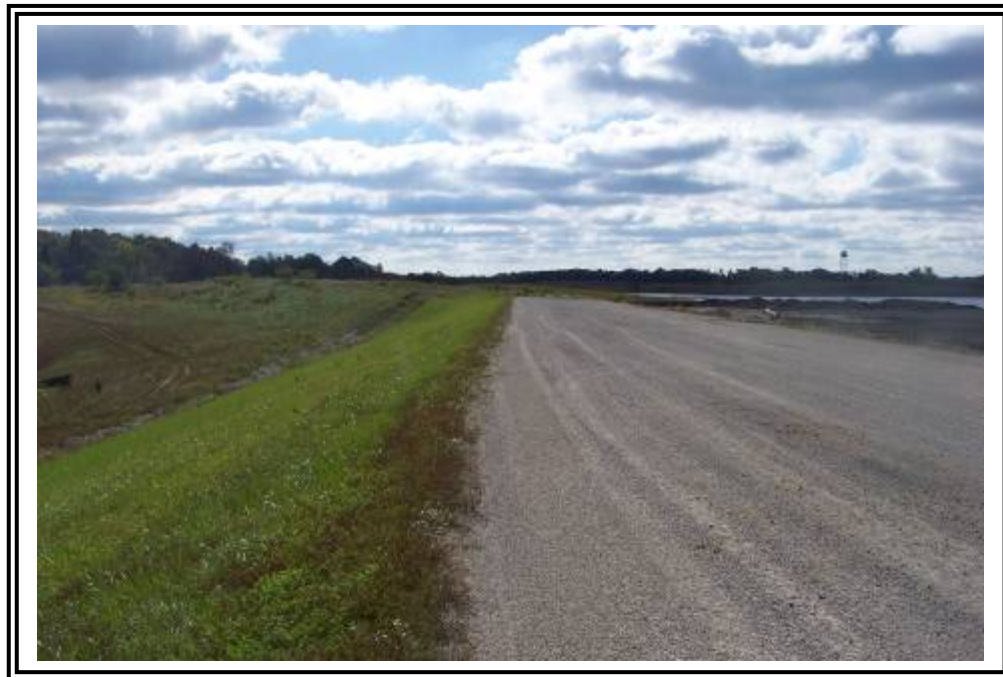
Crest of ATB #2 looking south toward the east abutment.
