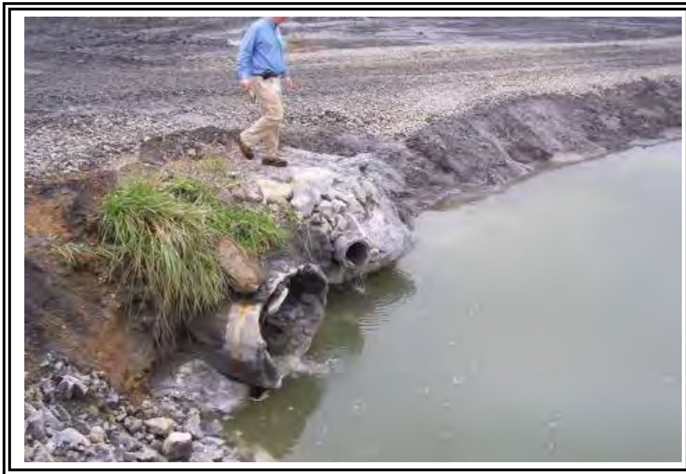
Stormwater flows from landfill (capped and uncapped) areas and discharges into E-Pond within the ATB.
