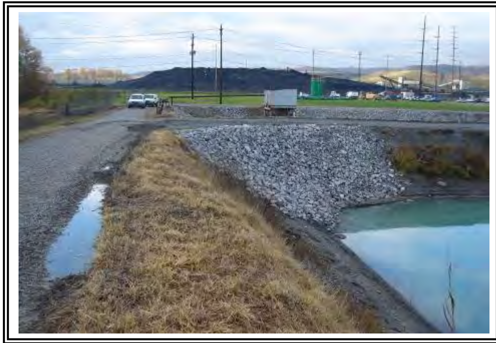
Standing water on east dike at Basin/ Dead Storage Pond looking south.
