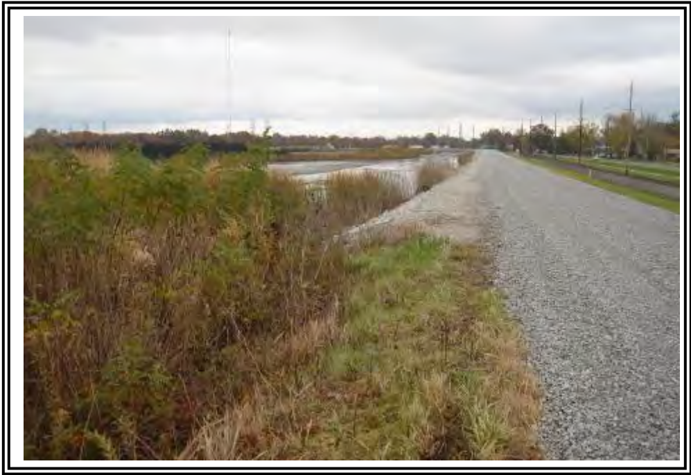
Crest of ATB south dike looking east.
