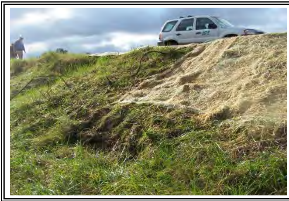
Irregularity on north dike at Basin/ Dead Storage Pond. Combination of surface slumps, erosion rills, etc. Probes soft to about 9" then firm.
