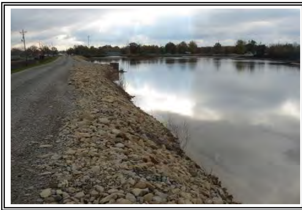
Upstream slope and crest of ATB north dike looking east.
