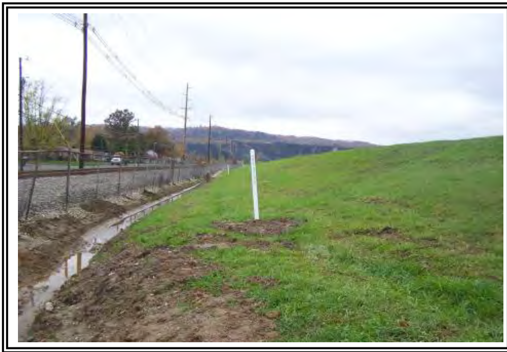
Downstream slope of ATB south dike looking west.
