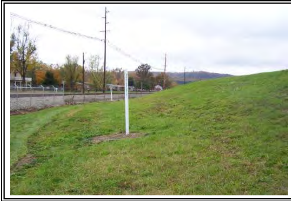
Downstream slope of ATB east dike at southwest corner. White markers indicate the location of a high pressure gas line installed in 2005.
