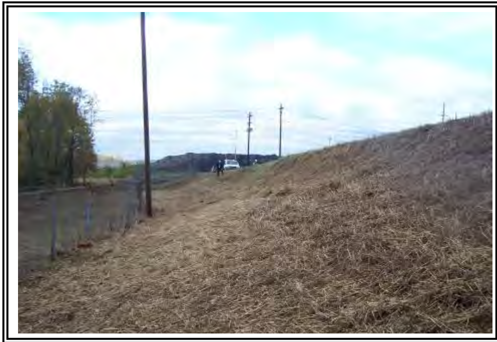
Downstream slope of east dike at Basin/ Dead Storage Pond looking south. Note steepness of the embankment and irregularity of grading. January 2010 survey showed the upper portion of the slope to be 1.7H:1V flattening to 2.8H:1V at the toe.
