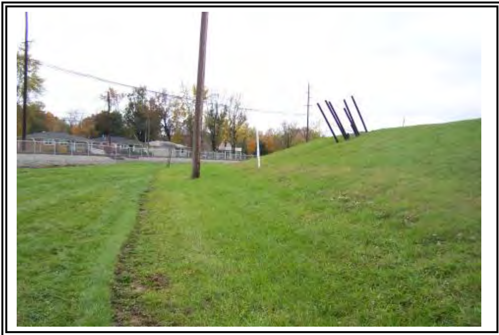
Downstream slope of ATB east dike looking south. White markers indicate the location of a high pressure gas line installed in 2005.
