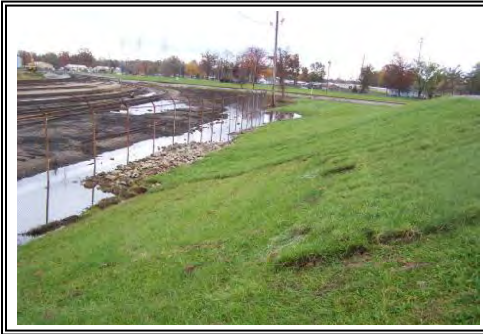
East end of ATB north dike has been regraded and had sod placed to address drainage problems. E.ON U.S elected to place new sod rather than seed because of this year's excessive rain.
