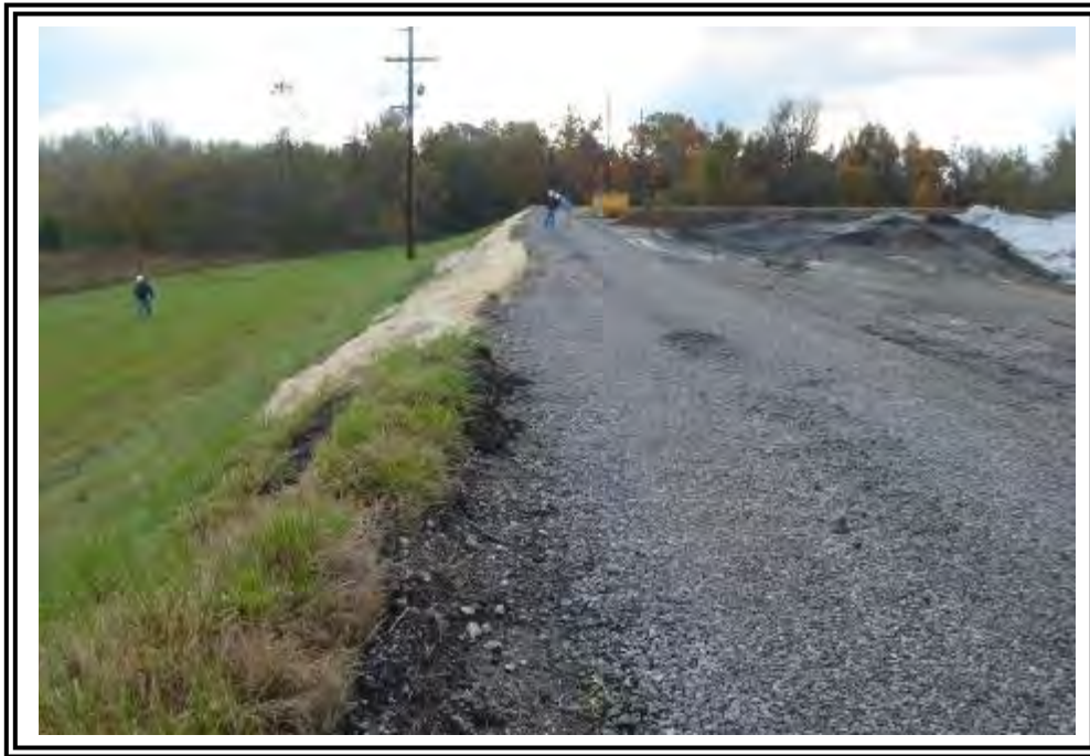
Crest of Basin/ Dead Storage Pond north dike looking east.
