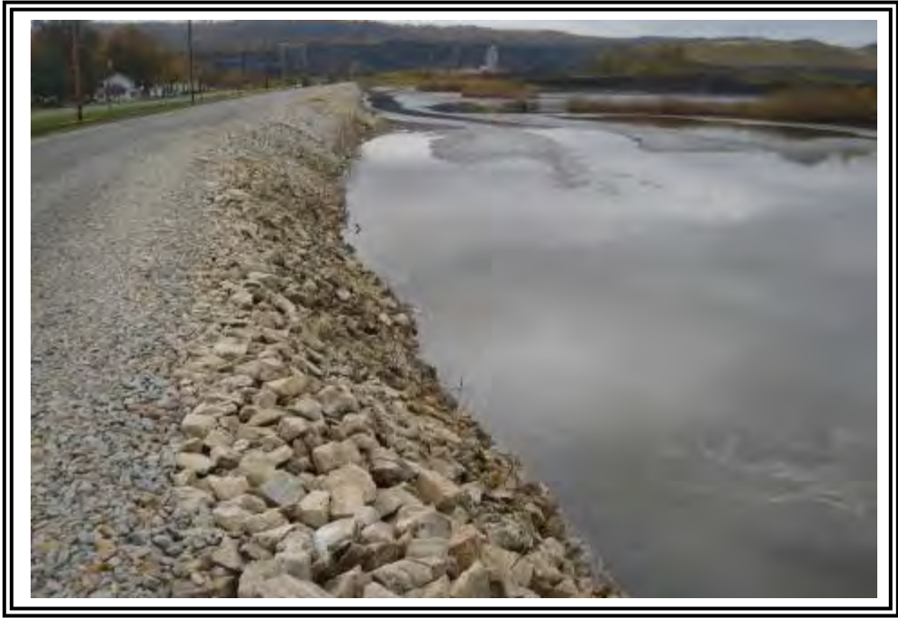
Upstream slope of ATB south dike looking west.
