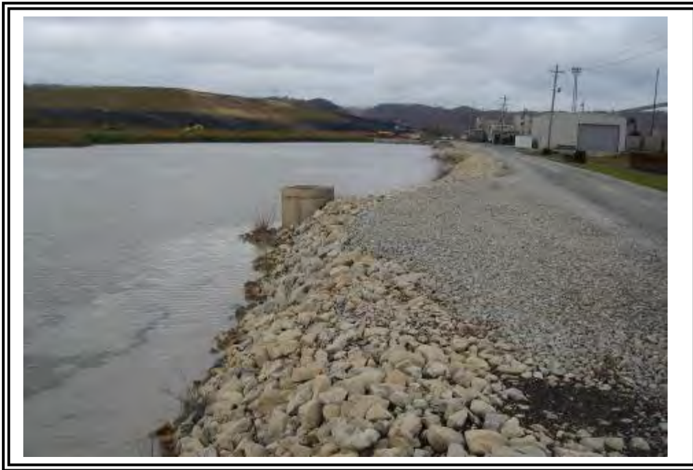
Upstream slope and crest of ATB north dike looking west.
