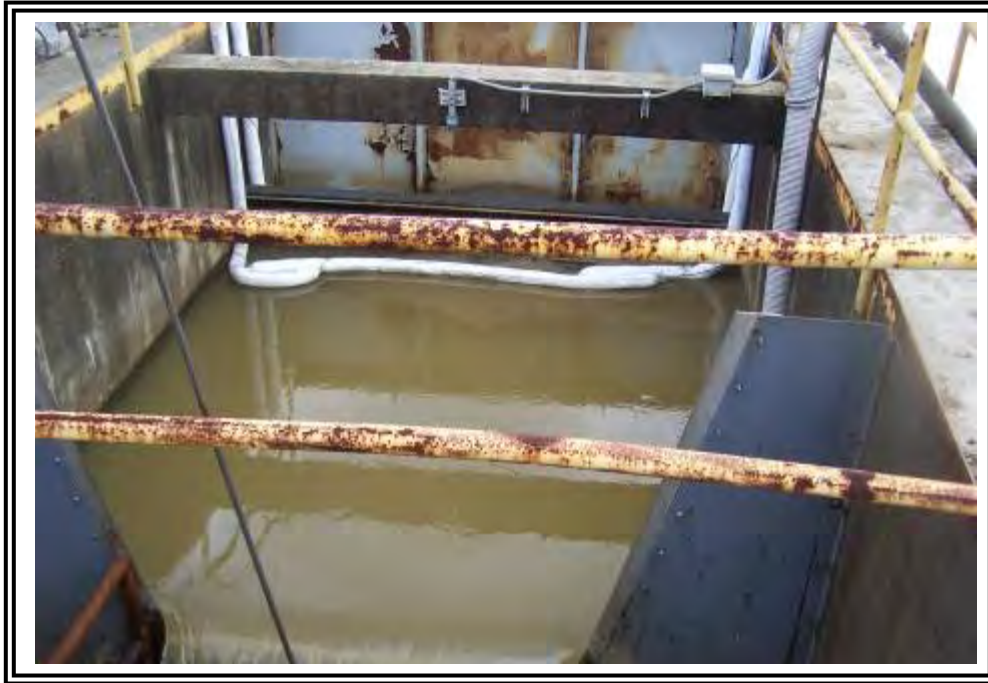
ATB discharge structure.
