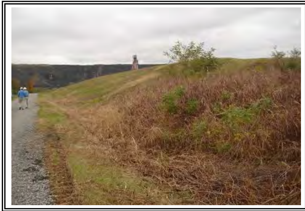
Stockpiled material for use at the landfill adjacent to ATB south dike looking west.
