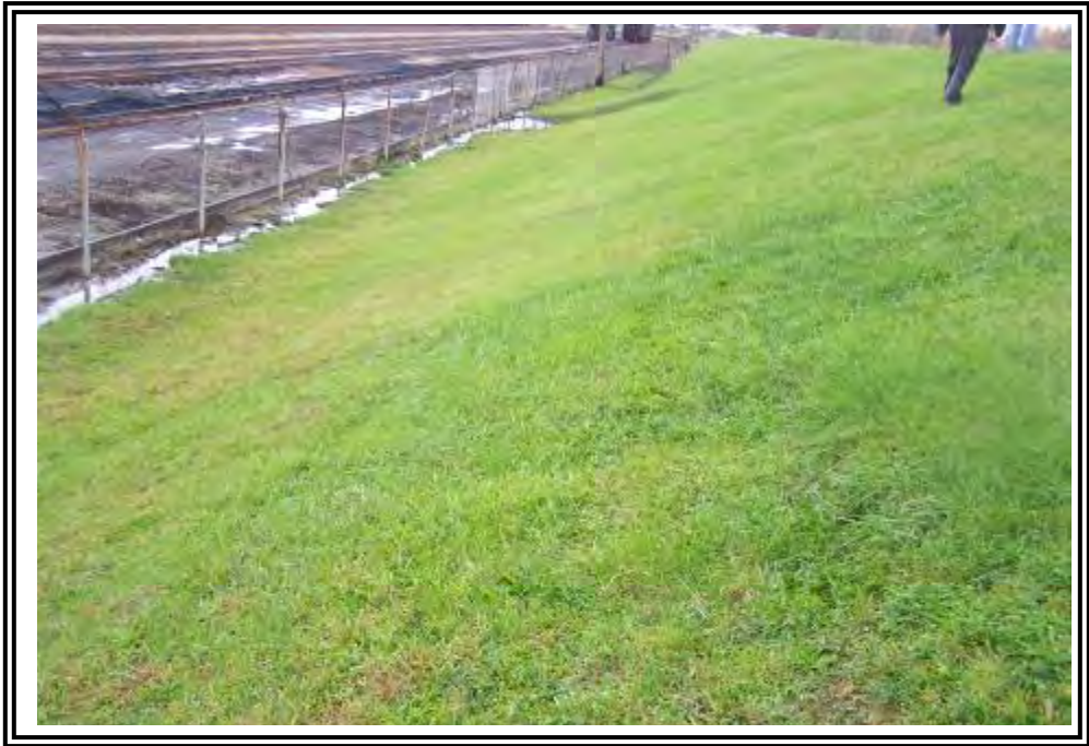
Downstream slope of north dike at ATB looking east. Slight irregularity in slope grading difficult to distinguish as an “as constructed” condition or soil creep.
