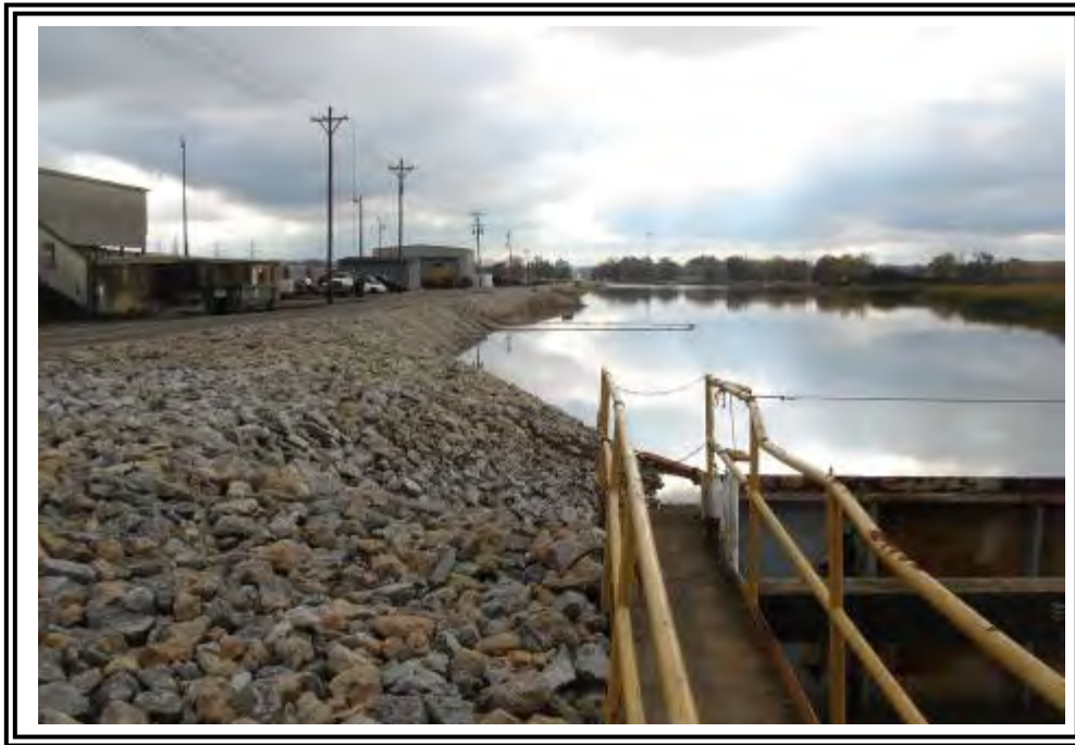
Upstream slope of ATB north dike looking east from outlet structure.
