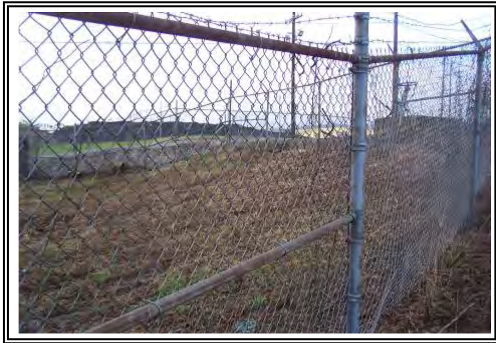
Looking towards south abutment at Basin/ Dead Storage Pond.
