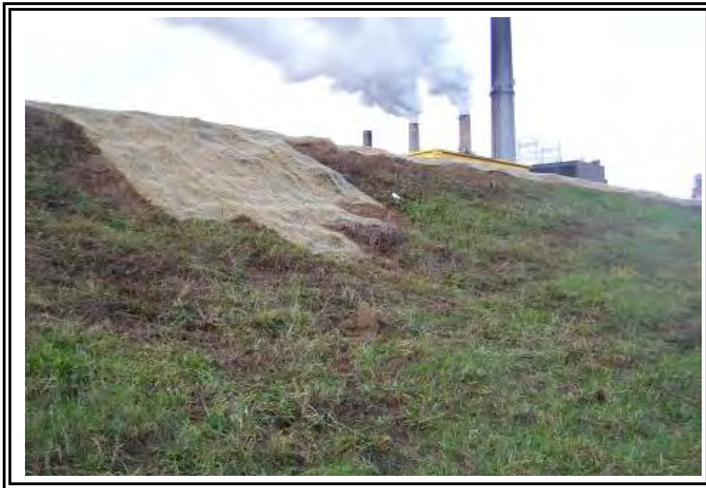
Recent patchwork repair along crest of north dike at Basin/ Dead Storage Pond.
