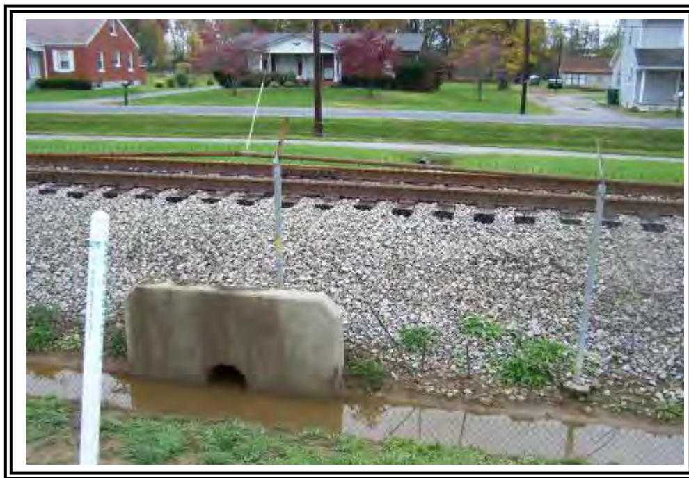
Drainage swale outlet along ATB south dike looking south.
