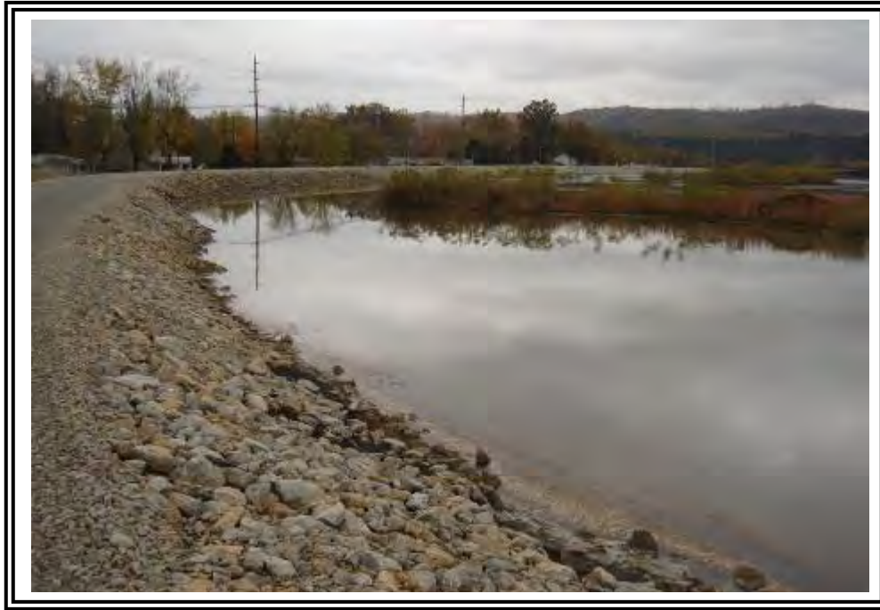
Upstream slope of ATB east dike looking south.
