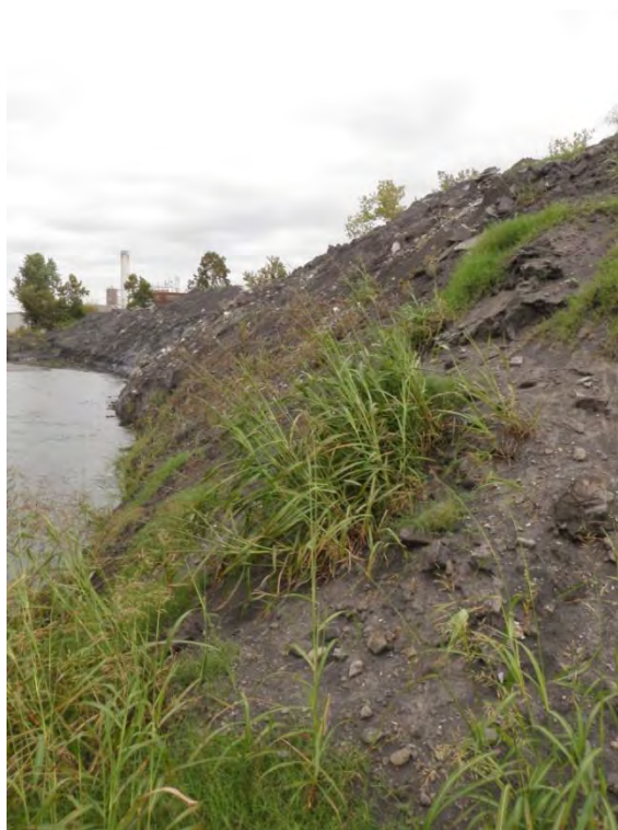
Photo 4: View of inside slope of ash piles in East Cell.
