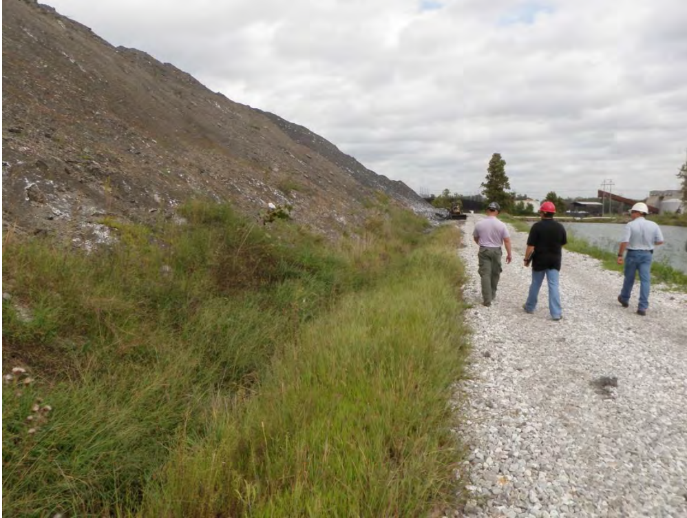
Photo 11: View of ash in the West Cell, looking north along the dike between the East and West Cells.
