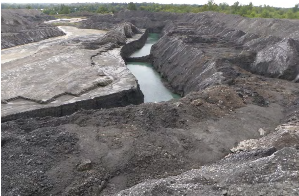
Photo 12: Excavation in West Cell showing how sluiced ash is conveyed through cell, looking south.
