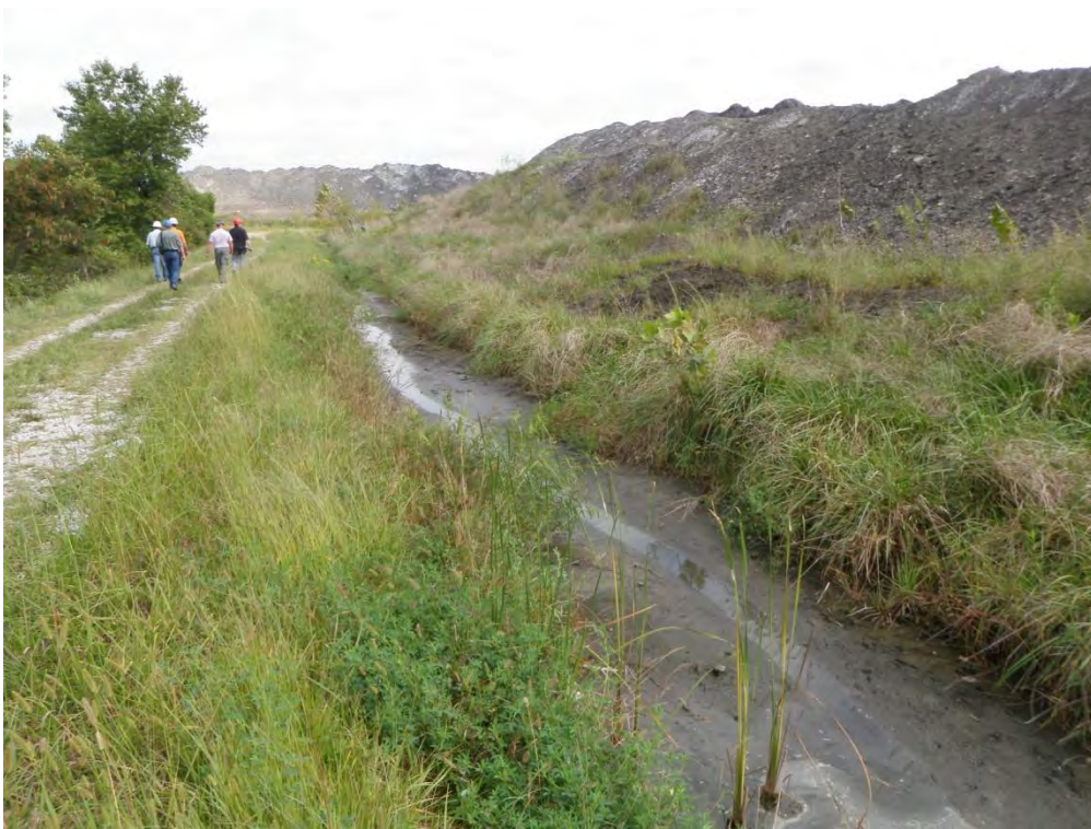
Photo 8: West perimeter dike showing interior drainage ditch and ash piles in East Cell.
