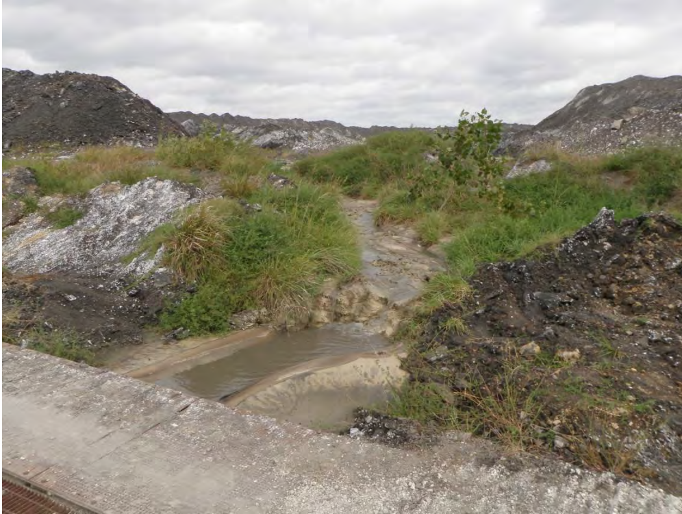
Photo 9: View of West Cell looking northwest from bridge over spillway between the East and West Cells.
