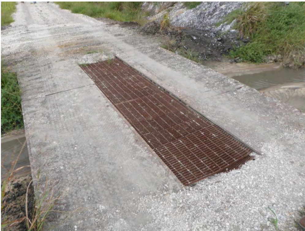
Photo 10: Bridge spanning spillway between the East and West Cells.
