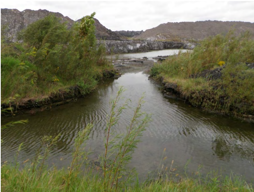
Photo 6: Inlet for perimeter dike drain connection to East Cell pond (dike drain ditch in foreground).
