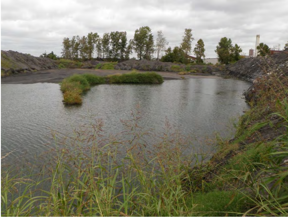
Photo 5: East Cell, looking northwest toward the location of the outlet pipe.
