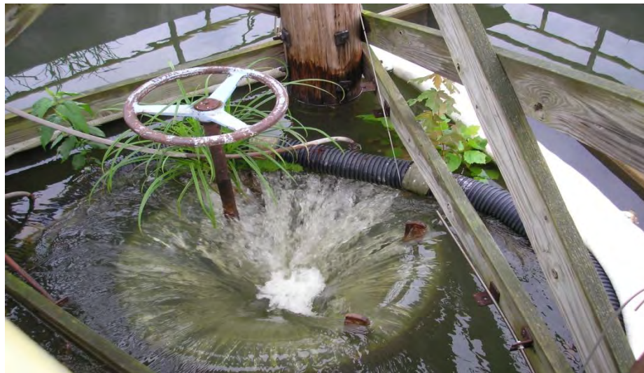
Figure 5.3.2-2: Photo of Primary Spillway Pipe Invert
