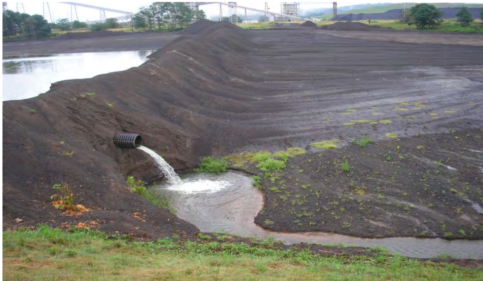
Figure 8.1-1: Photo of Decant Water from West to East Sections of Impoundment
