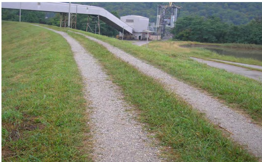
Figure 5.2.1-1: Photograph of Impoundment Dike Crest View to East
