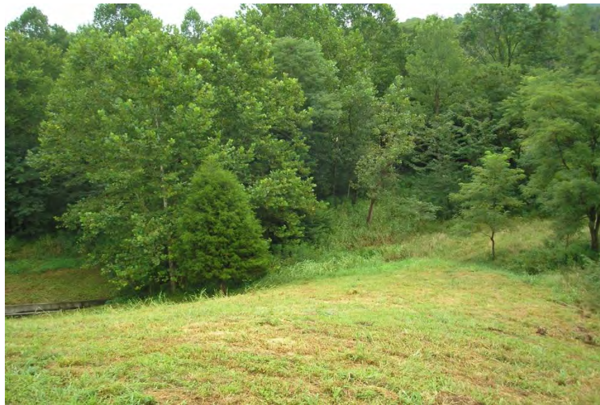
Figure 5.2.4-1: Photo of Embankment Crest at Northeast Corner Abutment
