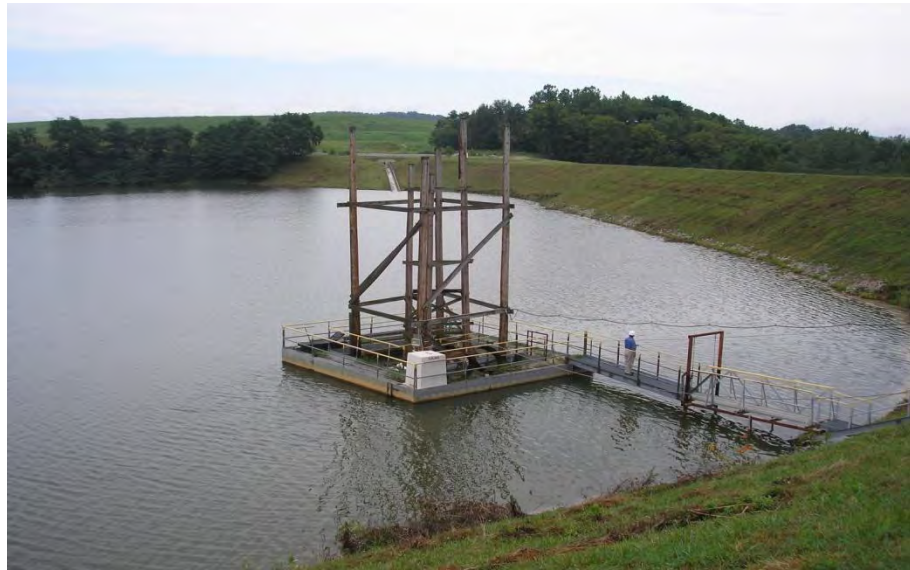
Figure 5.3.1-1: Photo of Primary Spillway Riser Structure
