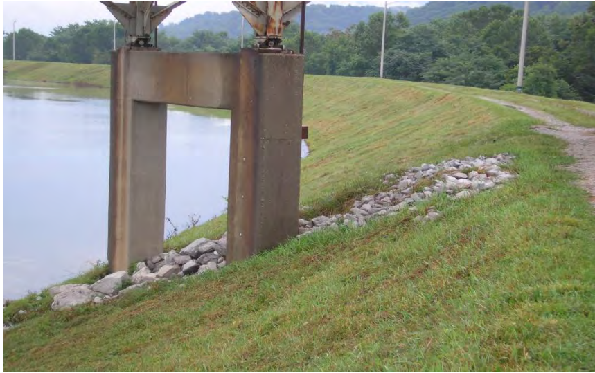
Figure 5.2.2-4: Erosion Repairs beneath Coal Conveyor Structure
