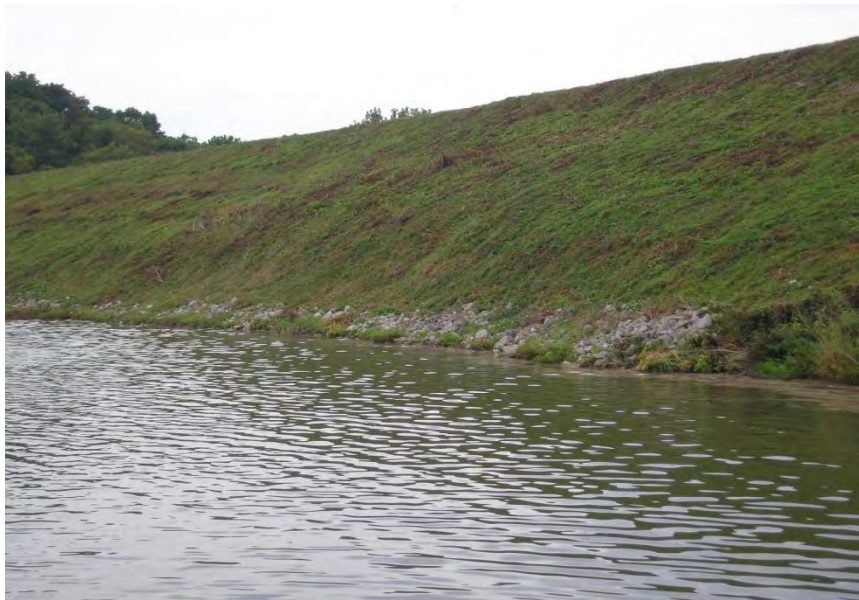
Figure 5.2.2-5: Rip Rap Armoring to Protect against Wave Erosion
