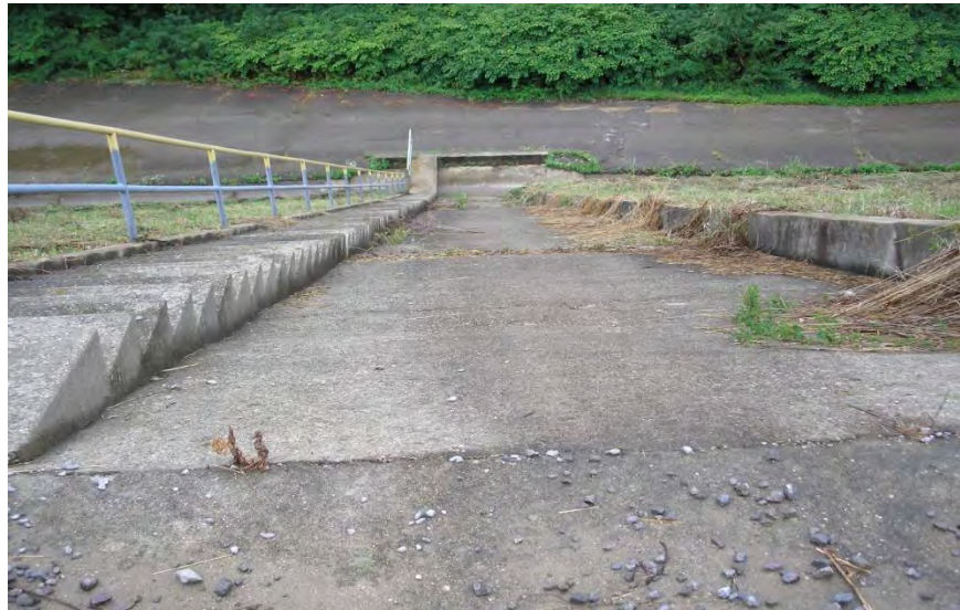
Figure 5.3.3-2: Photo of Emergency Spillway on Down-gradient Slope of Embankment
