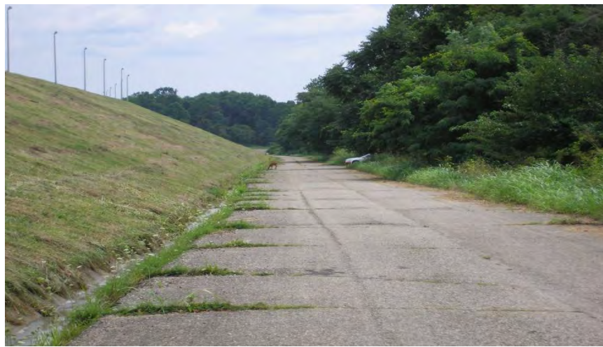
Figure 5.2.3-4: Photo of Down-gradient Embankment Toe with Drainage Ditch and Adjacent Pavement
