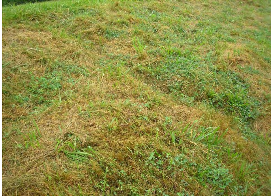
Figure 5.2.2-2: Photo of Small Erosion Rill on Up-gradient Slope
