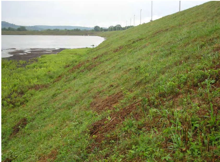
Figure 5.2.2-1: Photo of Embankment Up-gradient Slope View to East
