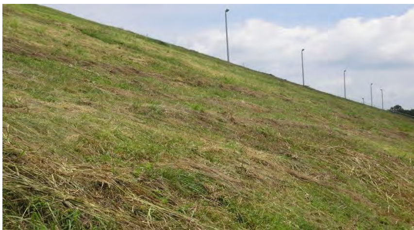
Figure 5.2.3-1: Photo of Embankment Down-gradient Slope View to East
