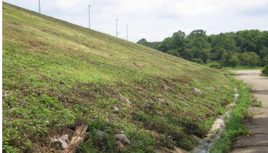
Figure 5.2.3-2: Rip-Rap Protection at Bottom of Down-gradient Slope
