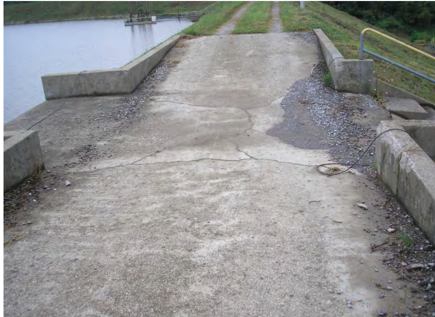
Figure 5.3.3-1: Photo of Emergency Spillway Invert.
