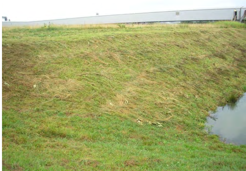
Figure 5.2.4-1: Photo of Interior Groin at Southwest Corner of Impoundment
