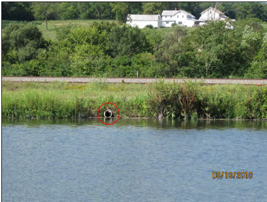
EMERGENCY OVERFLOW BETWEEN WEST PRIMARY SETTLING POND AND EAST PRIMARY SETTLING POND
