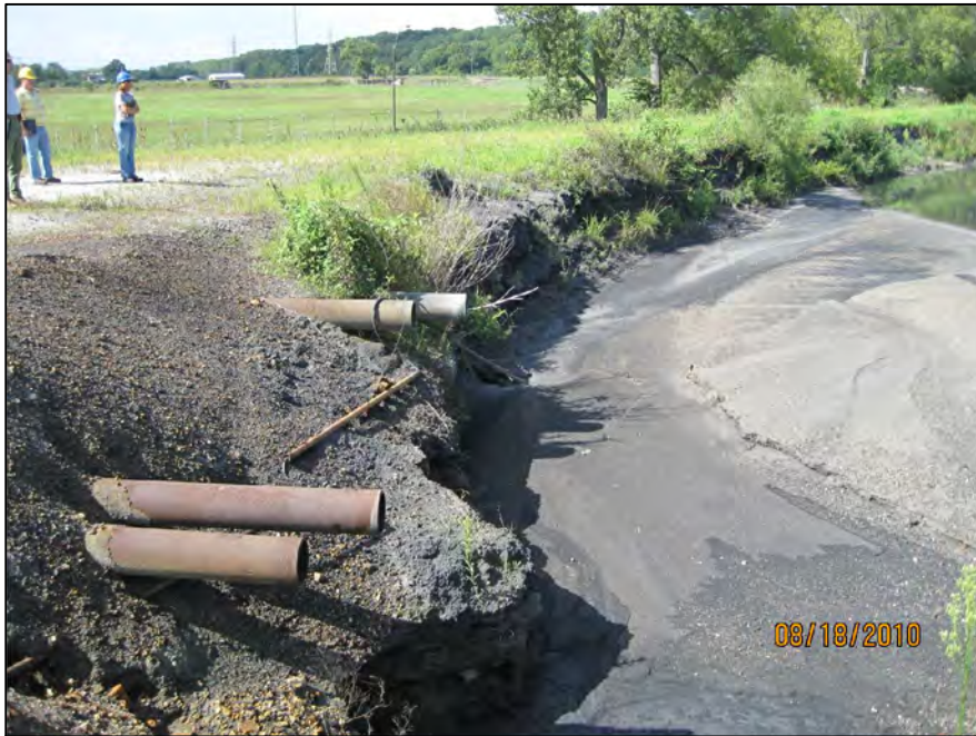
INLET PIPES FROM PLANT TO WEST PRIMARY SETTLING POND LOCATED AT SOUTHEAST CORNER OF POND
