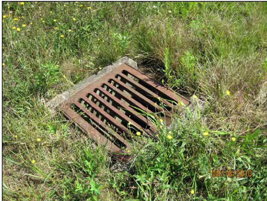
STORM DRAIN ALONG SOUTHERN DOWNSTREAM TOE
