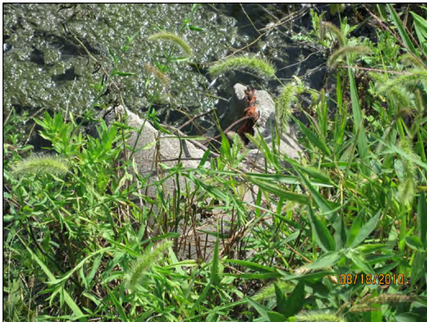
E-18 EMERGENCY OVERFLOW BETWEEN WEST PRIMARY SETTLING POND AND EAST PRIMARY SETTLING POND
