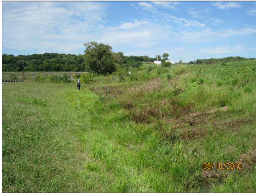
WET AREA ALONG SOUTHERN DOWNSTREAM TOE
