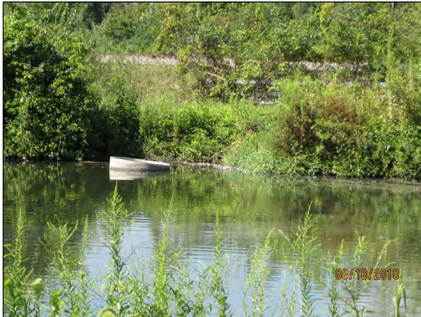
E-6 FROM NORTHERN CREST LOOKING WEST TOWARDS VERTICAL DISCHARGE STRUCTURE
