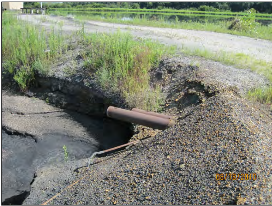
INLET PIPES FROM PLANT TO WEST PRIMARY SETTLING POND LOCATED AT SOUTHEAST CORNER OF POND
