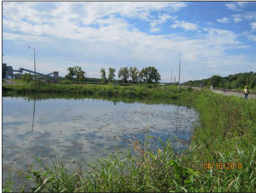
S-1 FROM NORTHERN DIKE LOOKING SOUTH
