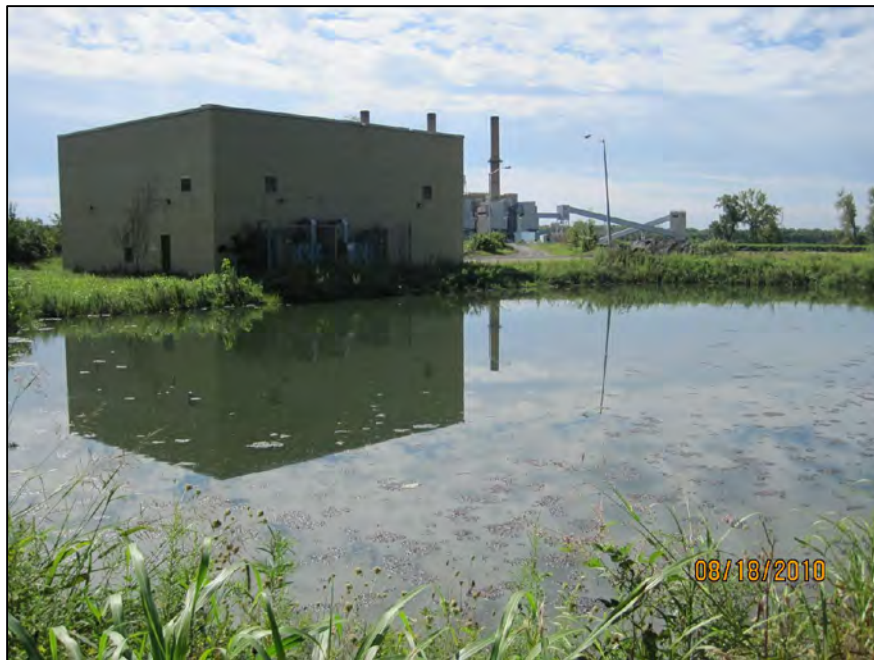
S-2 FROM NORTHERN DIKE LOOKING SOUTHEAST TO TREATMENT FACILITY
