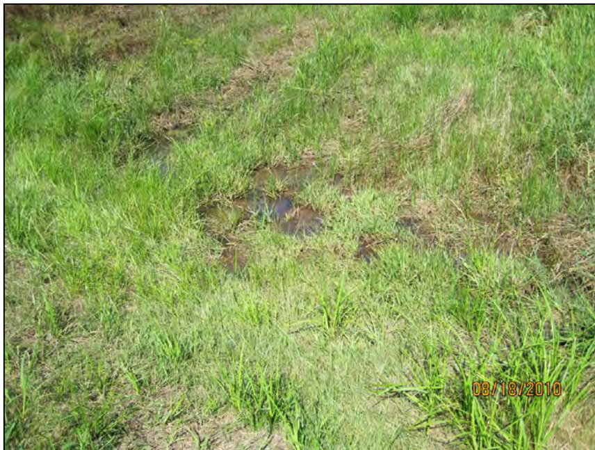
E-12 WET AREA ALONG SOUTHERN DOWNSTREAM TOE
