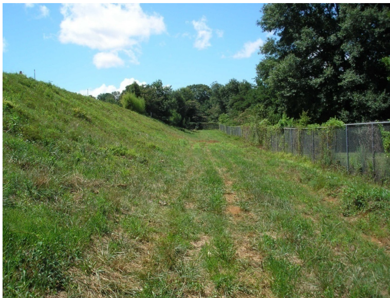
Photograph 23: West Dike Central Section View South, 6/23/2010
