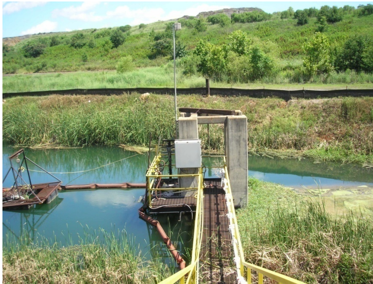
Photograph 28: Primary Riser Spillway, 6/23/2010
