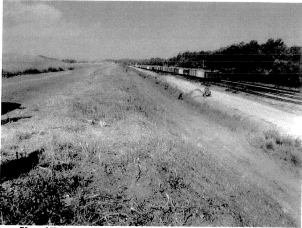
Photo SU-1: Condition of Vegetation on North Dike After Clearing
