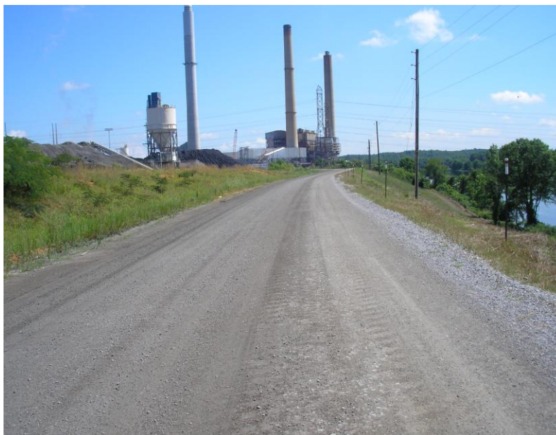
Figure 5.2.1.1. Photo Showing Crest of East Dike
