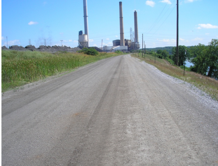
Photograph 1: Crest of East Dike View North, 6/23/2010
