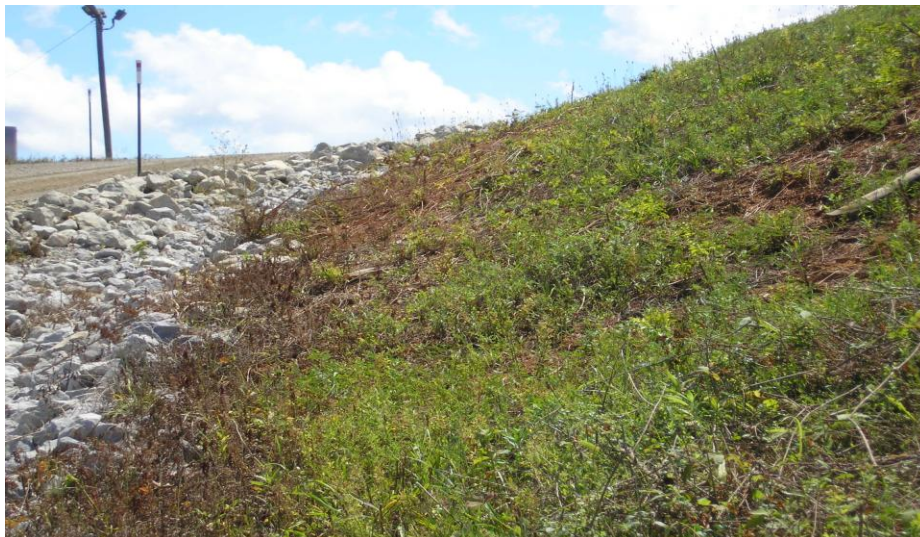
Figure 5.2.3-8 Photo Showing West End of North Embankment Downstream Slope
