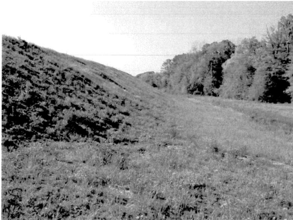
Photo 5 – Typical Condition of West Dike, From Toe
