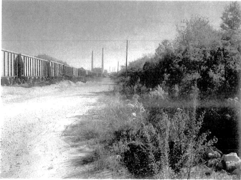
Photo 1: Toe of North Dike, Looking East
