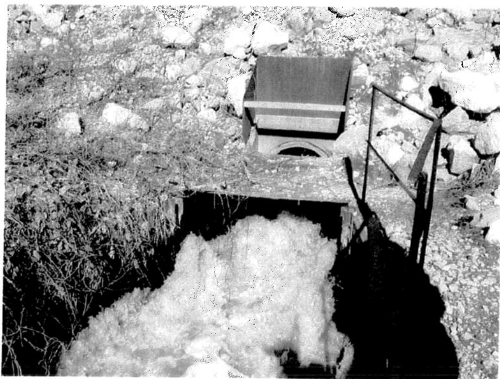
Photo IN-8: Discharge Outlet Structure
