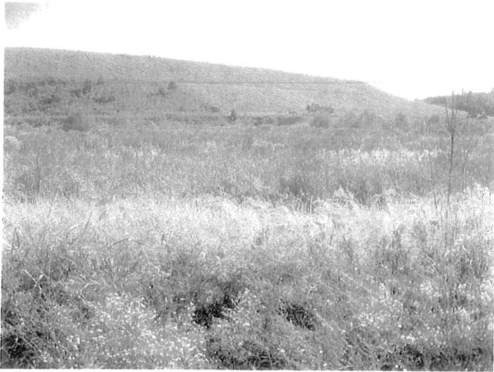
Photo 3: Gaston Ash Pond Near Mid-Point of West Dike, Looking East
