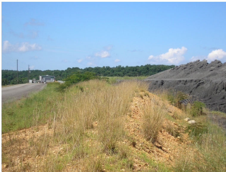
Photograph 2: East Dike Crest & Upstream East Dike View to South, 6/23/2010
