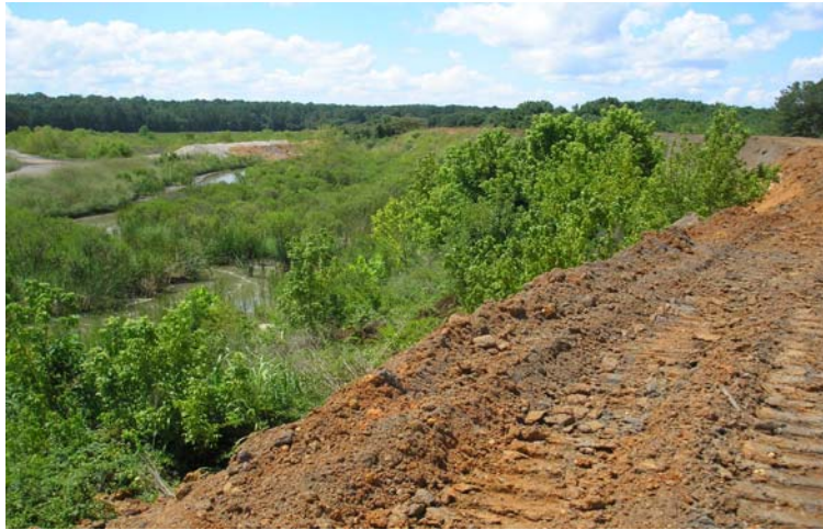
Photograph 7: West Dike Spoil Pile at Upstream Slope, 6/23/2010
