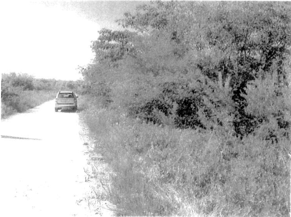
Photo 2: Crest of West Dike, Looking South
