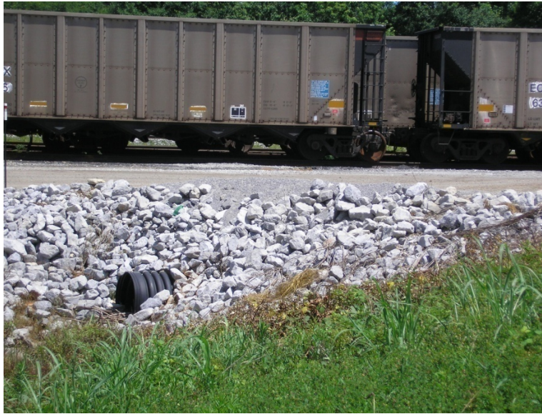
Photograph 27: West Dike Rail Drain at Toe North Abutment, 6/23/2010
