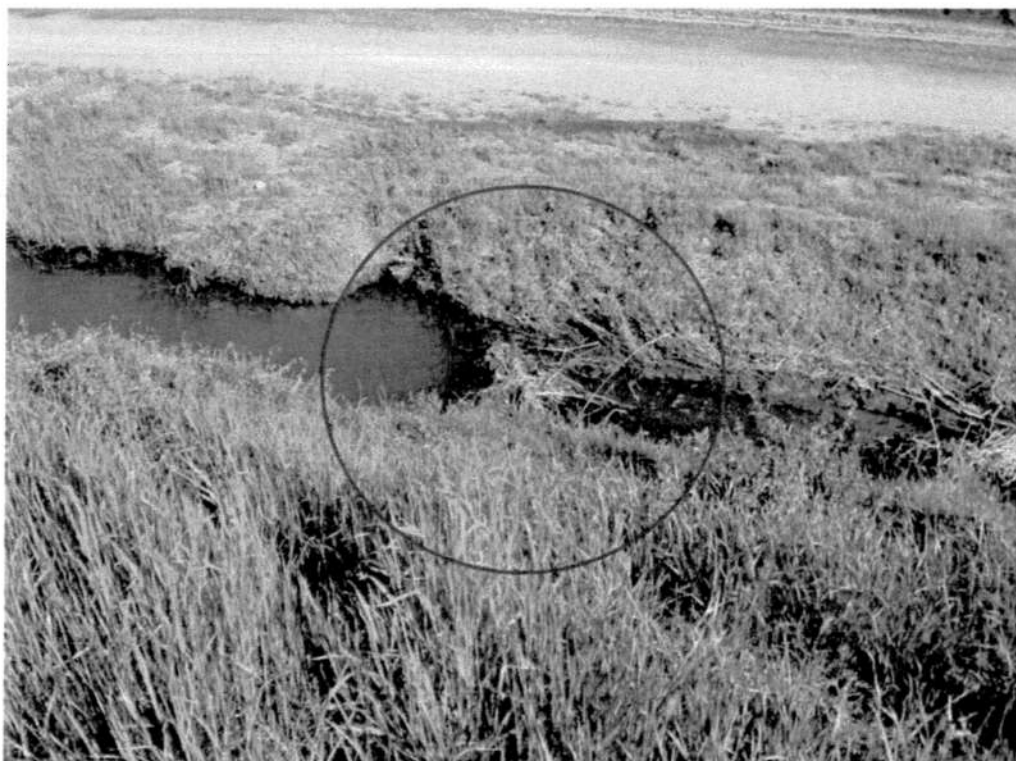
Photo 3 – Typical Beaver Dam in North Dike Toe Ditch
