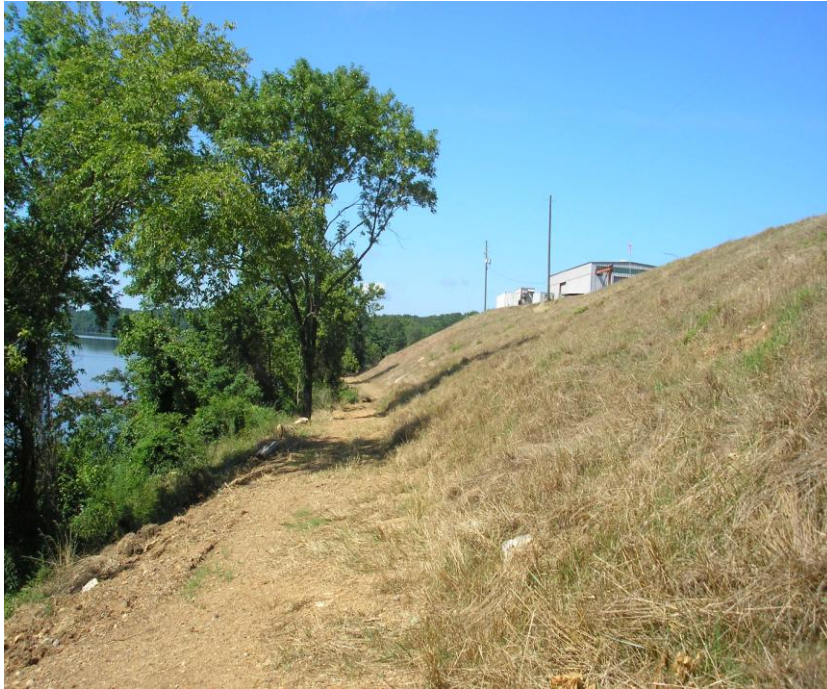
Figure 5.2.3-4 Photo Showing Toe of East Dike Downstream Slope
