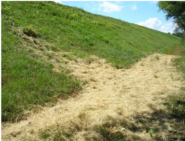
Photograph 20: West Dike Erosion Maintenance, 6/23/2010
