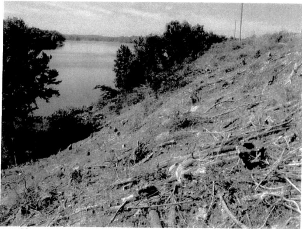
Photo SU-2: Condition of Vegetation on South Dike After Clearing
