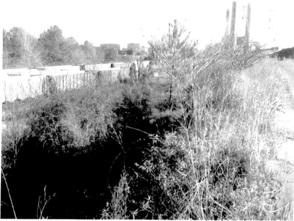
Photo IN-1: Typical Vegetation on North Dike – Initial Inspection
