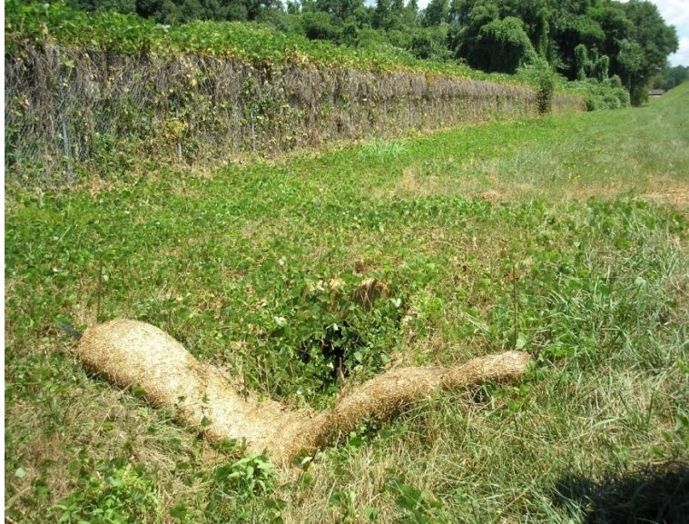
Photograph 22 West Dike - Surface Drain Near Dike Toe, 6/23/2010
