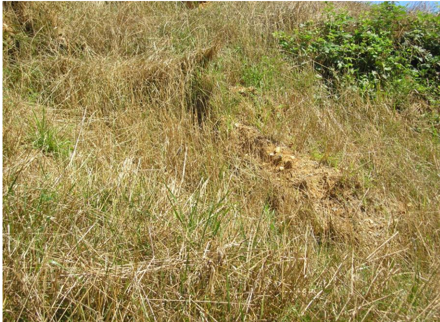
Figure 5.2.3-3 Photo Showing Small Erosion Rill East Dike Downstream Slope
