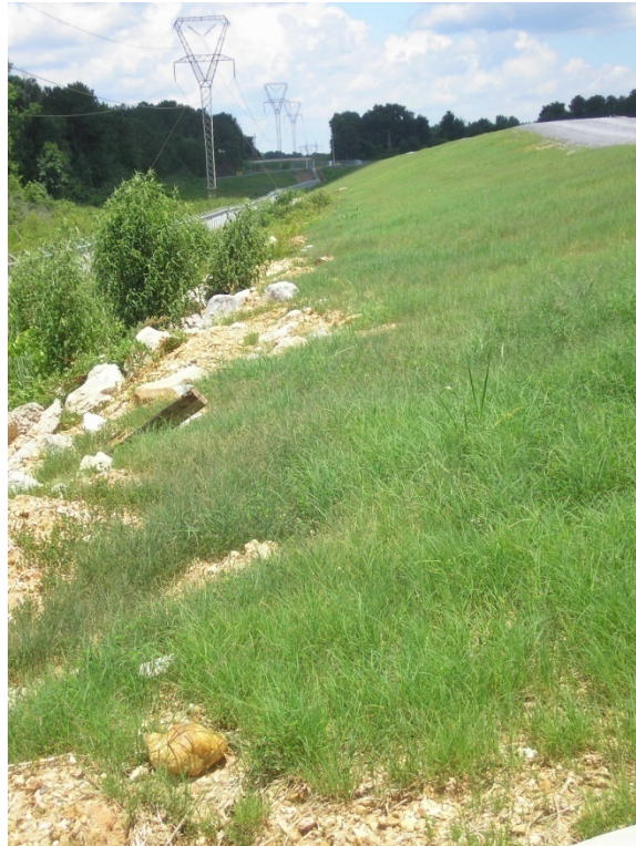
Photograph 19: West Dike Downstream Slope, 6/23/2010
