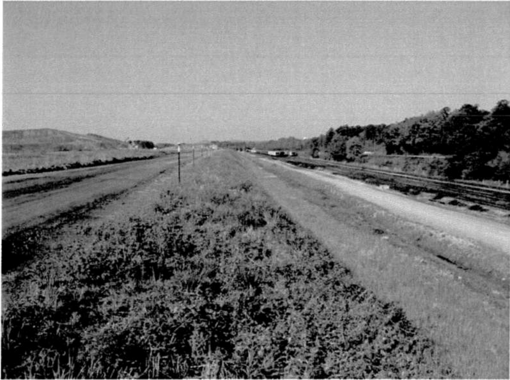
Photo 1 – Typical Condition of North Dike Embankment, From Crest
