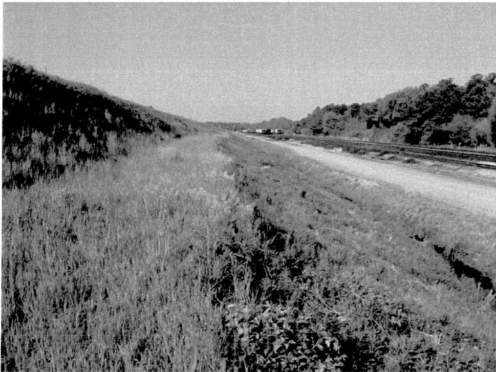
Photo 2 – Typical Condition of Midslope Access Road on North Dike
