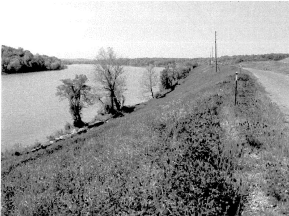
Photo 8 – Condition of East Dike, From Crest
