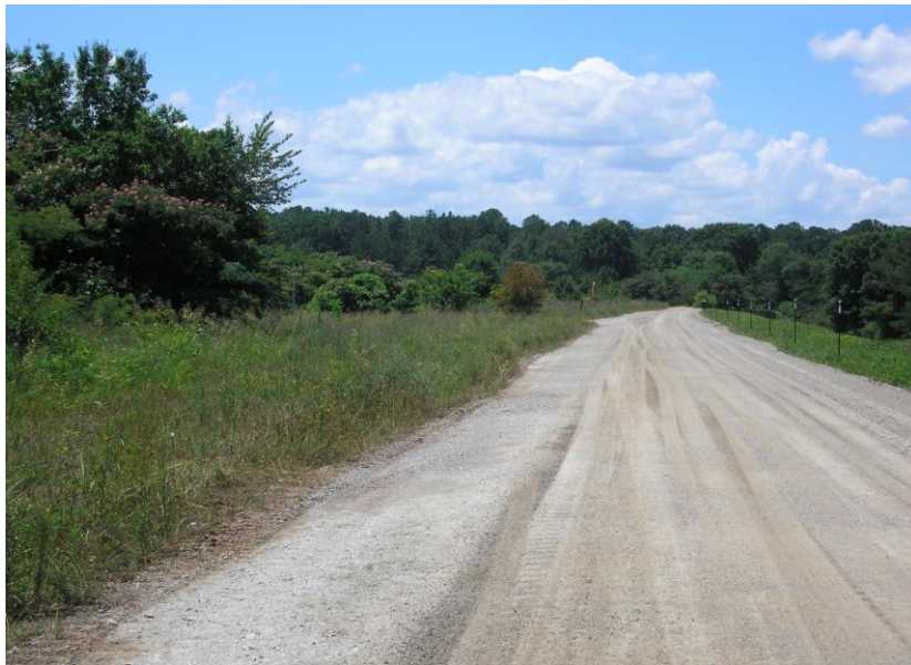
Figure 5.2.1-2 Photo Showing Dam Crest of West Dike (Upstream/Interior on Left)
