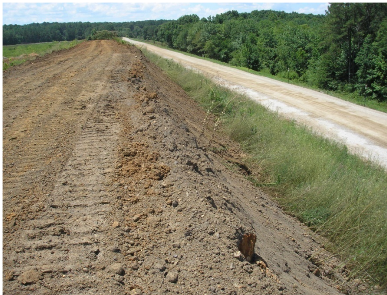
Photograph 4: West Dike Crest (Right Side) Central Section, 6/23/2010
