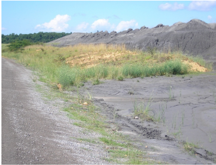
Photograph 3: Crest - East Dike View to South, 6/23/2010
