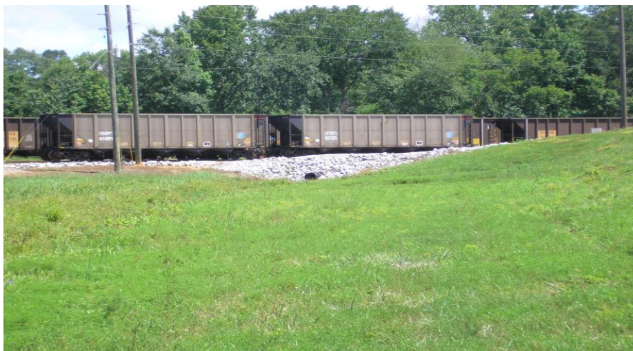
Figure 5.2.4-1 Photo Showing North End Groin Area of West Dike,
