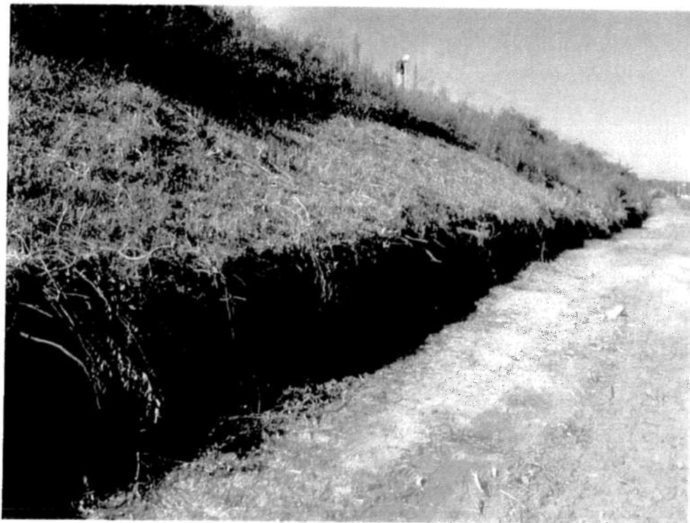
Photo SU-4: Access Road Cut into North Dike Embankment
