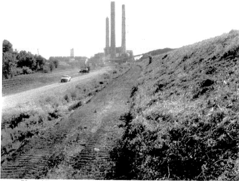
Photo SU-3: Midslope Access Road on North Dike Embankment
