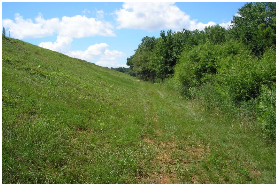
Figure 5.2.3-5 Photo Showing West Bank Downstream Slope
