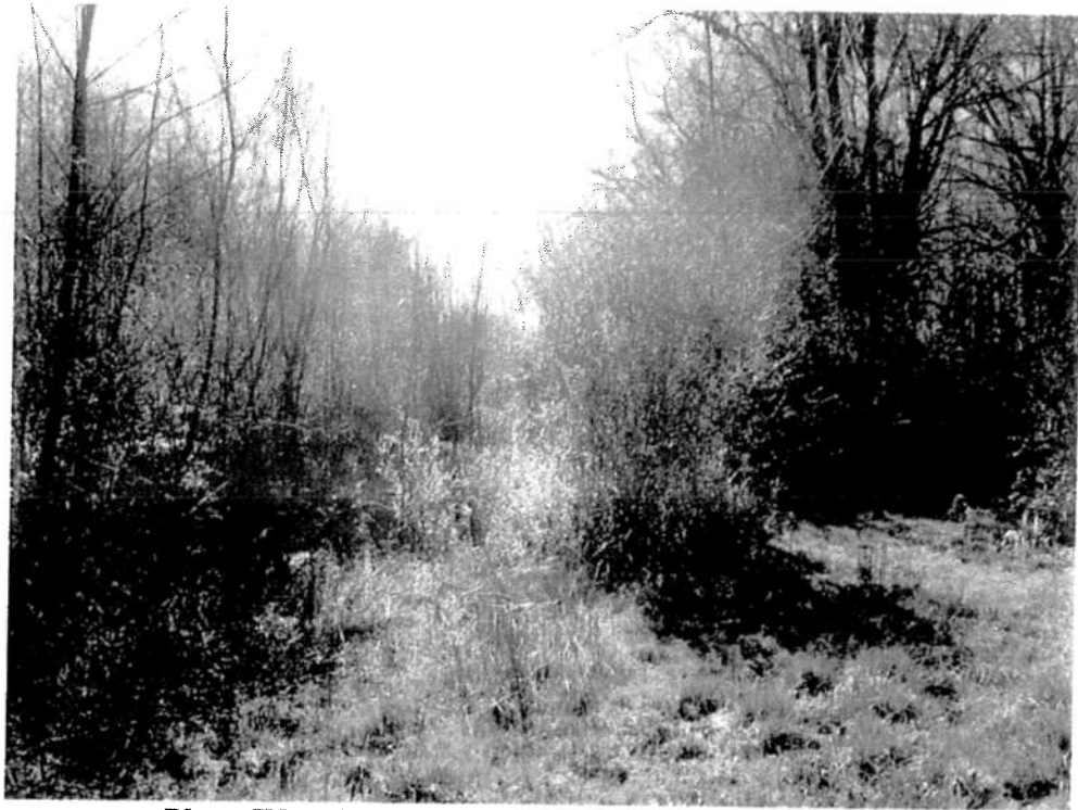
Photo IN-5: Dense Vegetation Along Toe of West Dike
