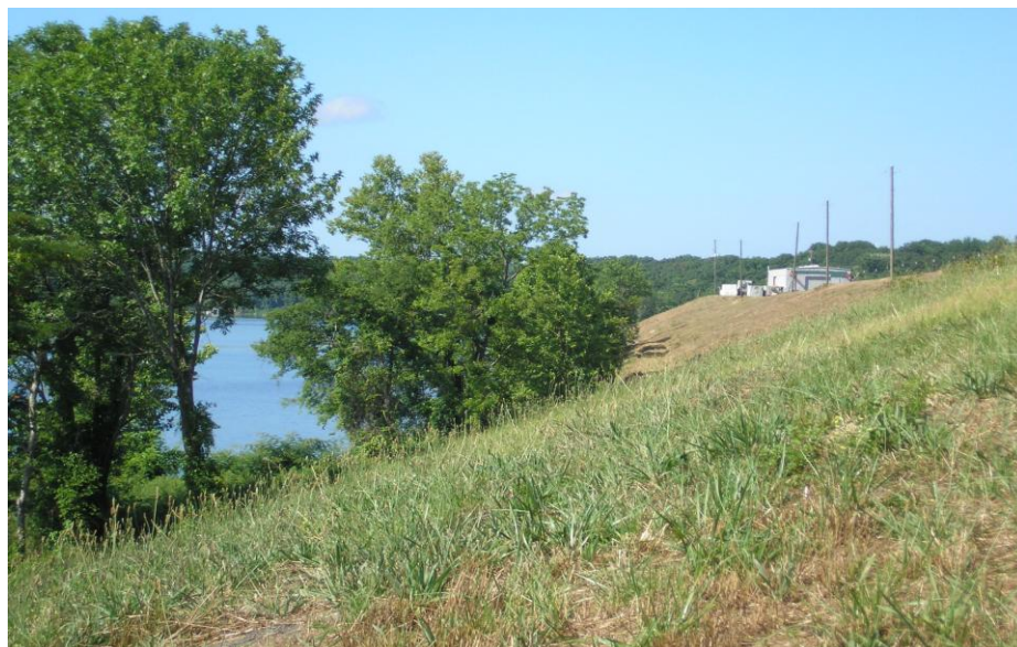
Figure 5.2.3 -1 Photo Showing Downstream Slope of East Dike.
