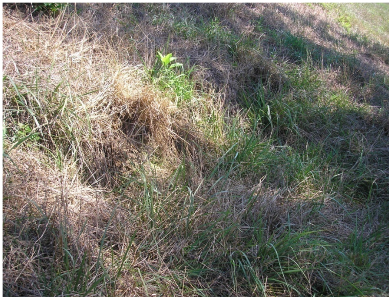
Photograph 14: Side Scarp of Slump - East Dike, 6/23/2010
