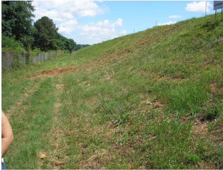
Photograph 21: West Dike South End View North, 6/23/2010
