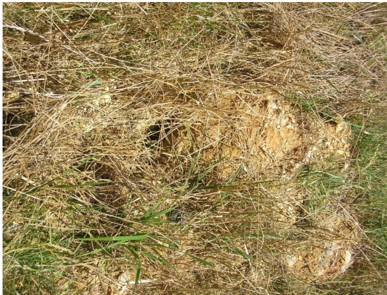
Photograph 10: Animal Burrow at East Dike Downstream Slope, 6/23/2010
