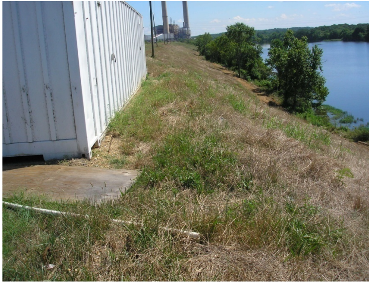
Photograph 17: Storage Container at Top East Dike South End, 6/23/2010
