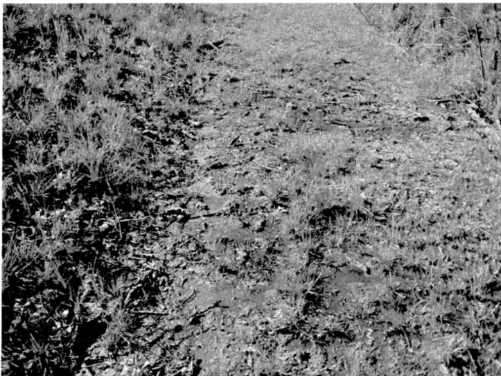
Photo 6 – Small Wet Zone on Toe of West Dike
