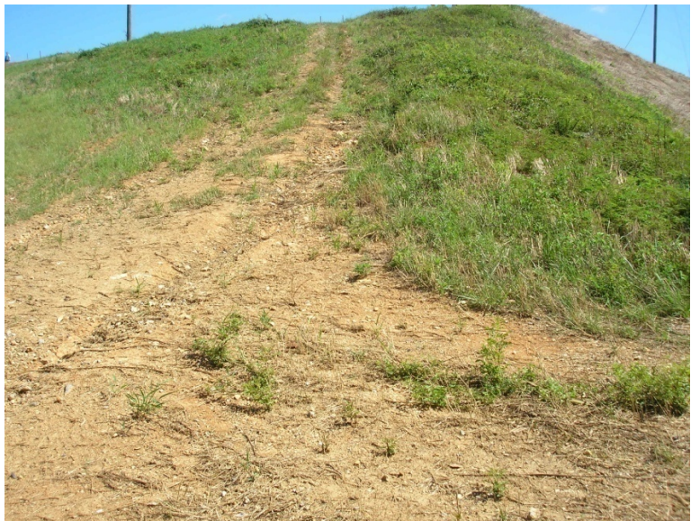
Photograph 16: South End - East Dike, 6/23/2010
