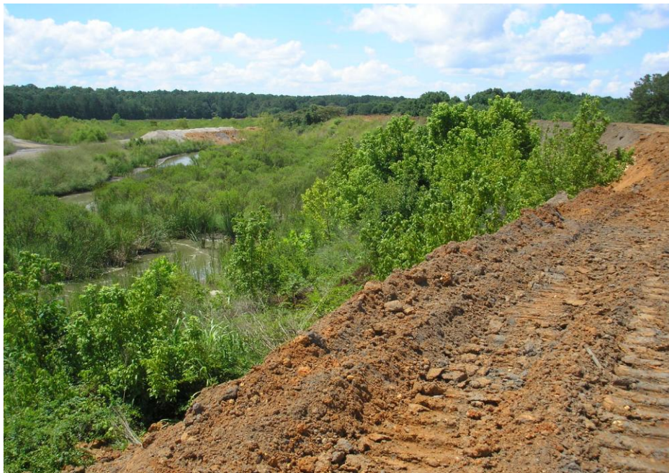
Figure 5.2.2-2 Photo Showing Upstream/Interior of West Dike
