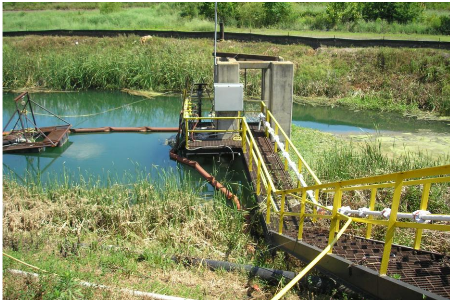
Figure 5.3.1-1 Photo Showing Overflow Riser
