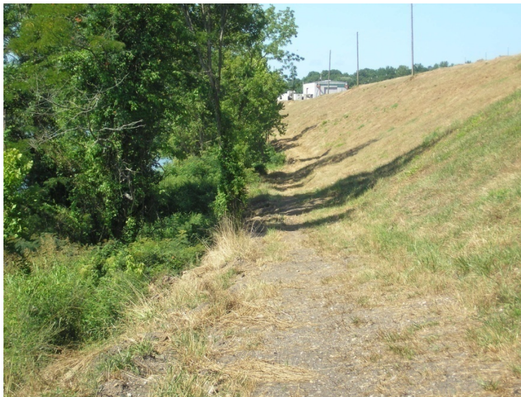
Photograph 18: Toe of East Dike, 6/23/2010
