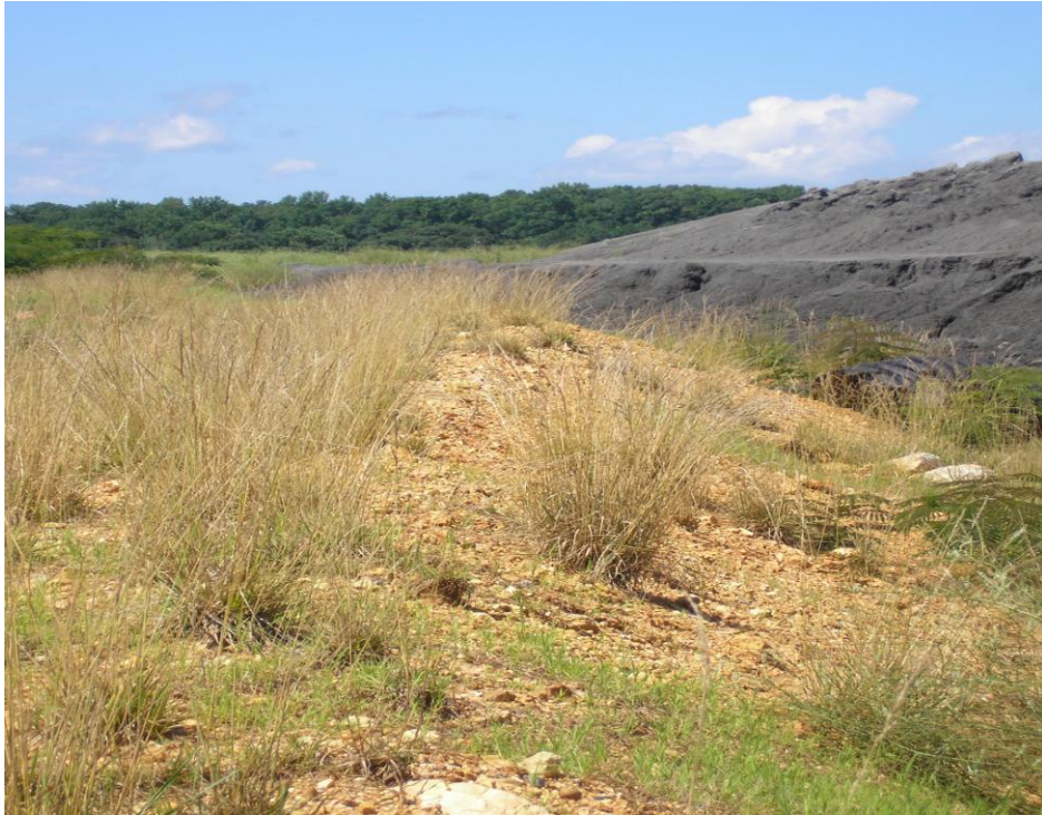
Figure 5.2.2-1 Photo Showing Upstream/Interior Slope of East Dike.
