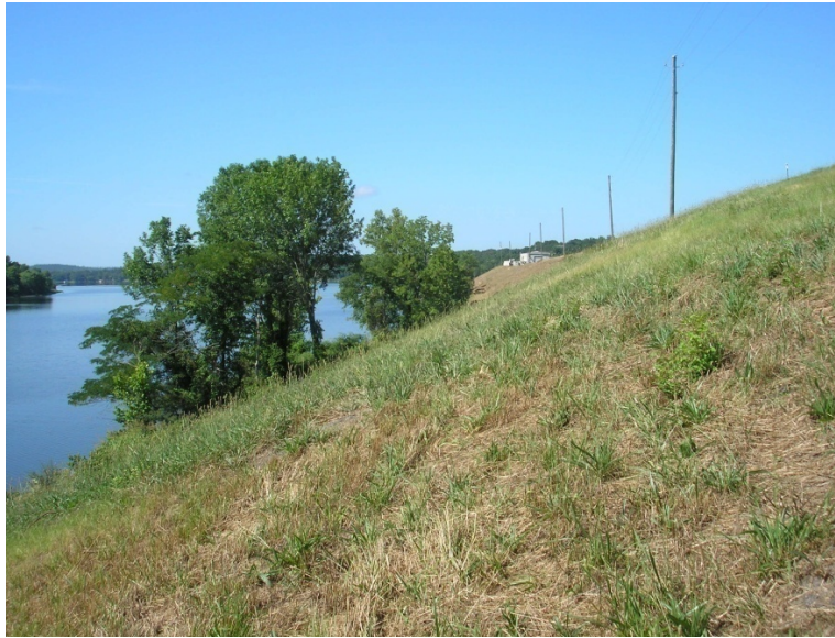
Photograph 13: East Dike - Downstream Slope View South, 6/23/2010
