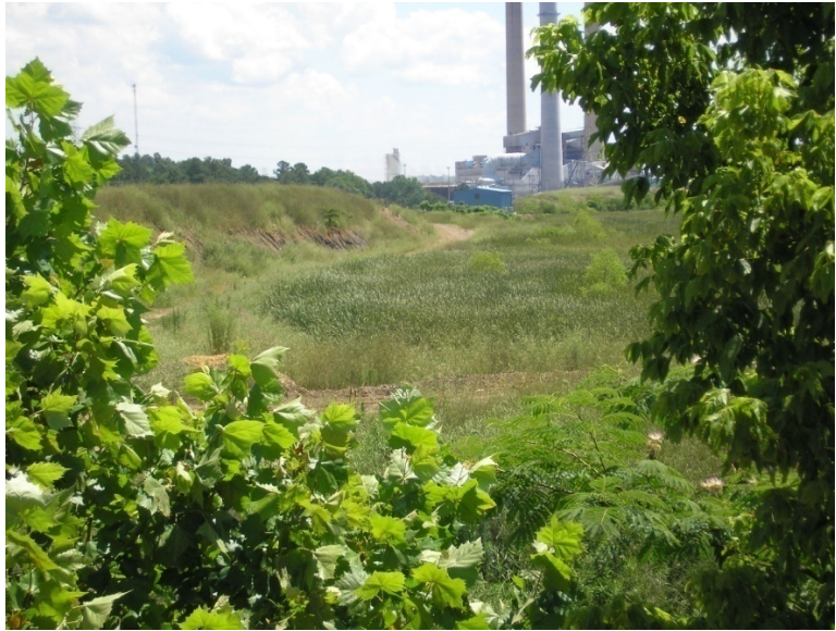
Photograph 11: East Dike North End, 6/23/2010
