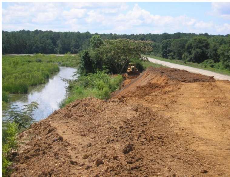
Photograph 8: West Embankment Interior Slope North End, 6/23/2010
