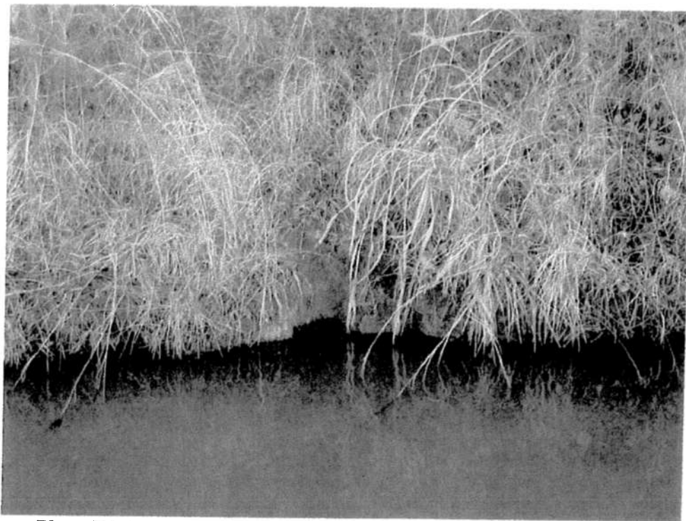
Photo IN-4: Typical Erosion Noted in Drain Along Toe of North Dike
