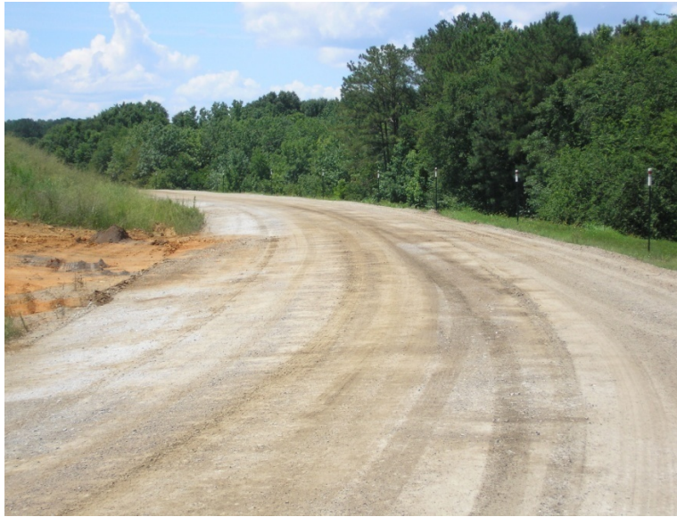
Photograph 5: West Dike Crest North End View South, 6/23/2010
