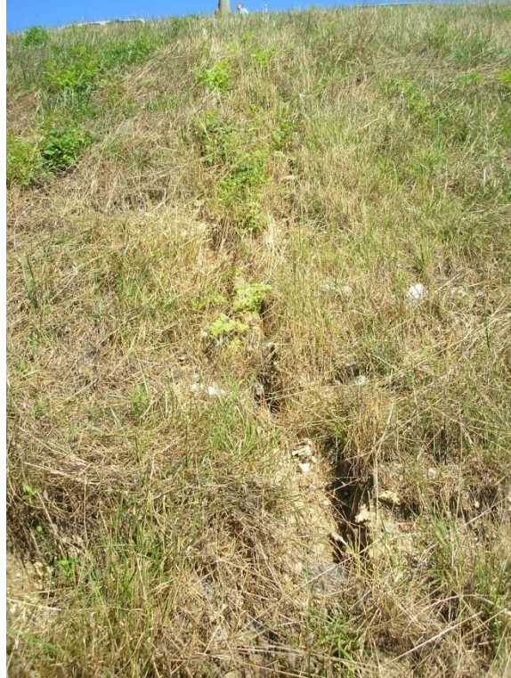
Photograph 10: Animal Burrow at East Dike Downstream Slope, 6/23/2010
