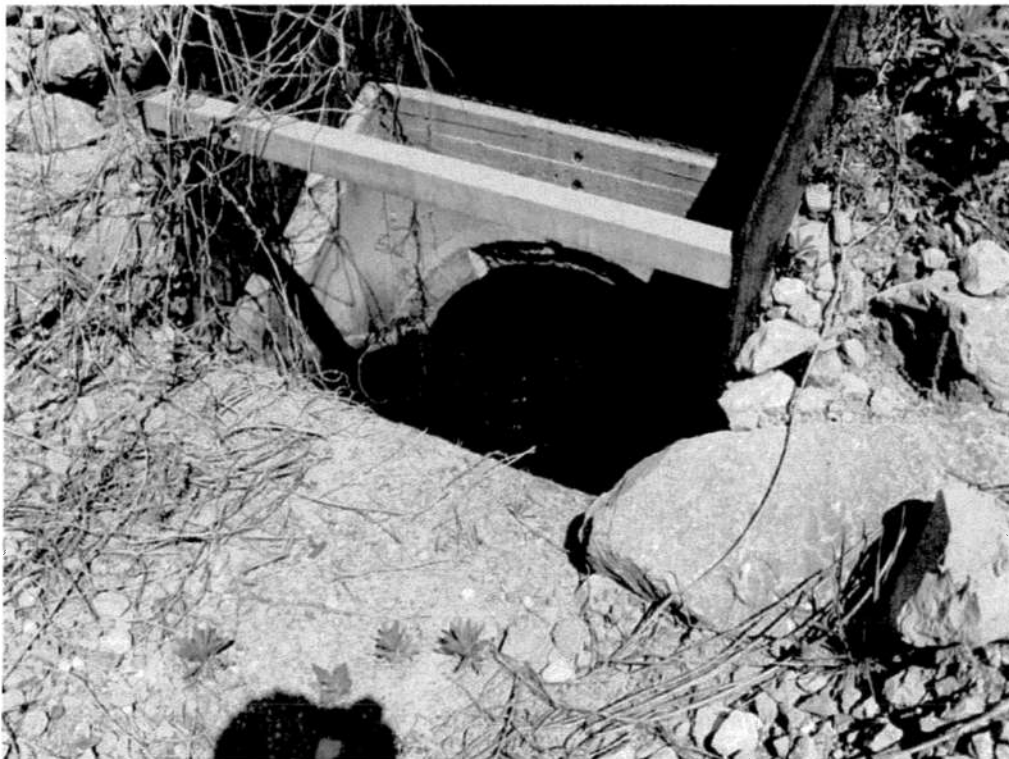
Photo 10 – Discharge Outlet Structure
