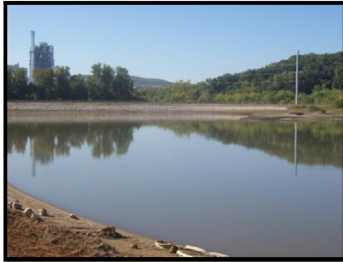
Figure 5.2.2-1: Riprap armored interior slopes of ash pond protected against wave action erosion, Southwest.
