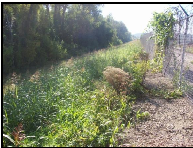
Figure 5.2.3-2: Ash pond external embankment with medium to heavy vegetative cover, Southeast.
