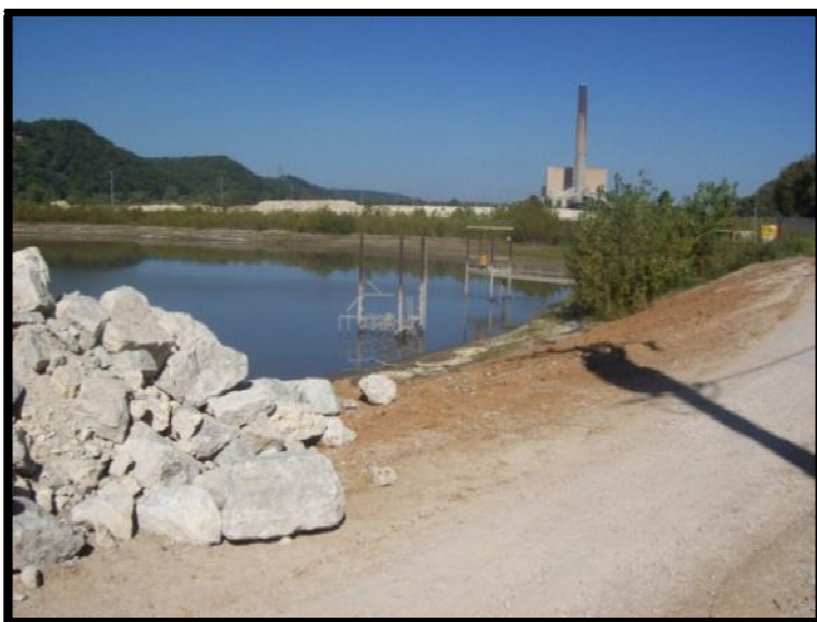
Figure 5.3.1-1: Ash pond inactive (left) and active (right) overflow structures, Northwest.
