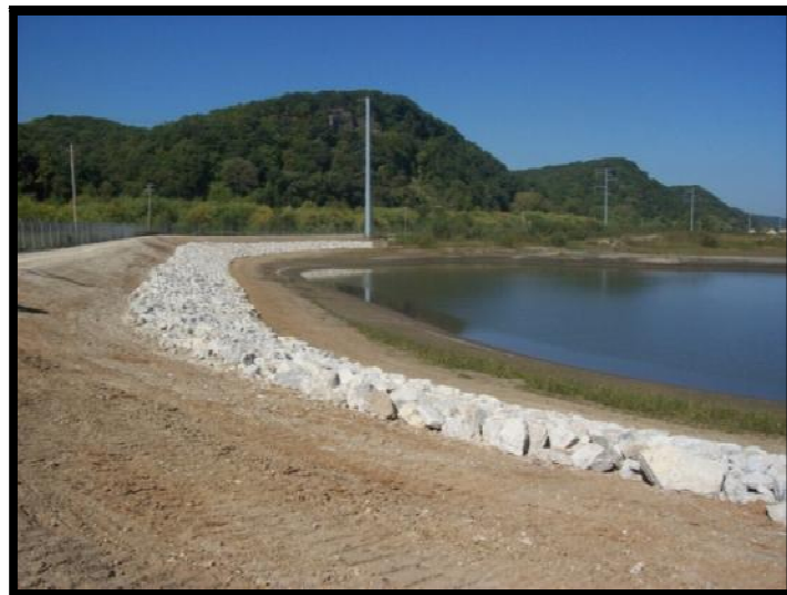
Figure 5.2.2-2: Riprap armored interior slope of ash pond.
