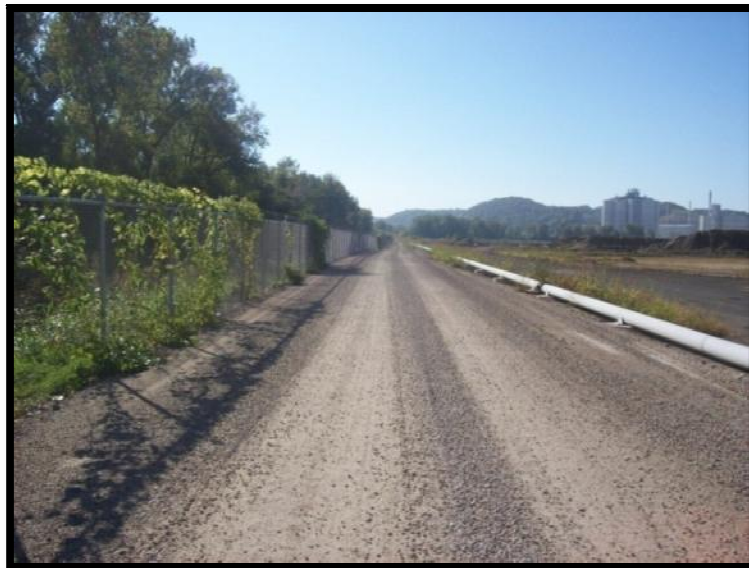
Figure 5.2.1-1: Typical crest condition of embankment, South.
