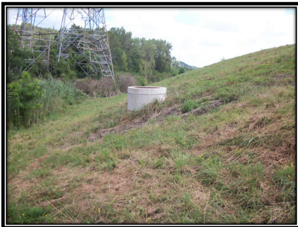
Photo 30 – Waste Water Sewer Line Manhole in Downstream Slope with Erosion Present
