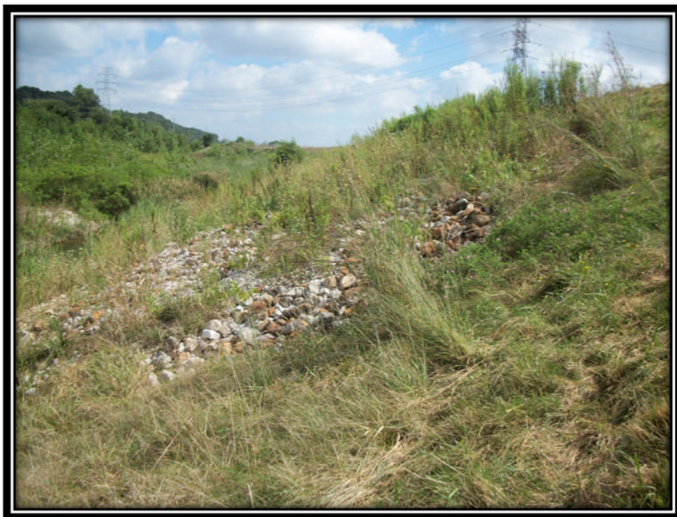
Photo 40 – Scarp that has Been Repaired on Western Pond 1 Downstream Slope
