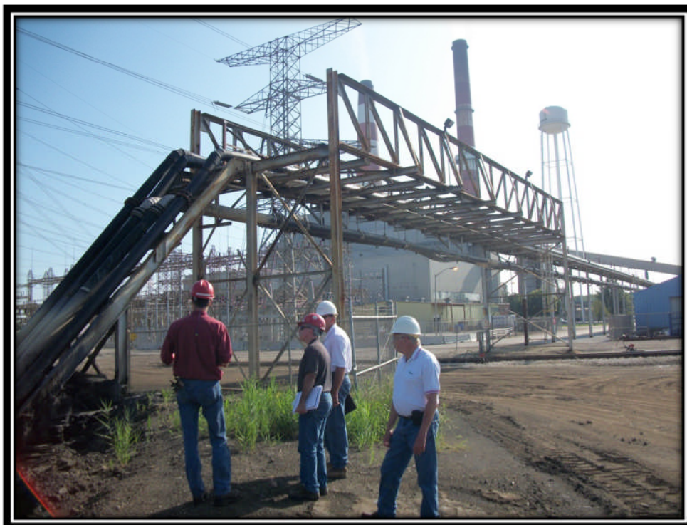
Photo 2 – Elevated Sluice Pipe Structure
