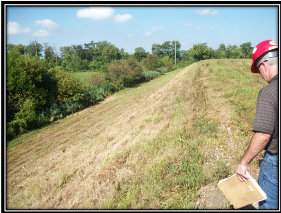
Photo 16 – Typical Southern Embankment of Clarification Pond
