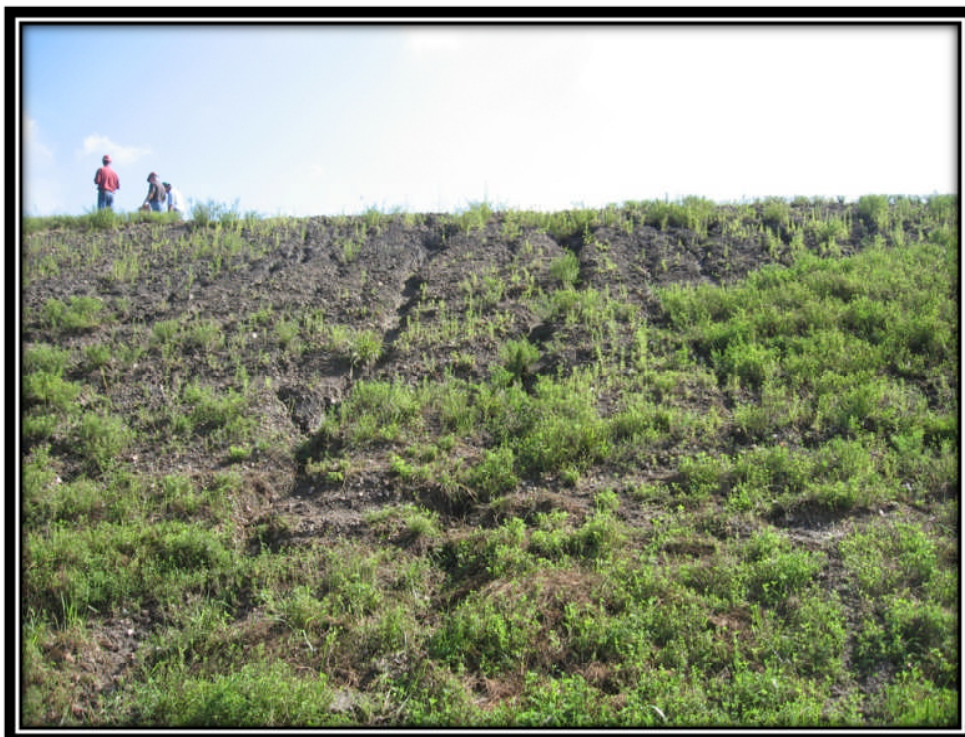
Photo 18 – Erosion and Sparse Vegetation on Downstream Slopes of Southern Embankment
