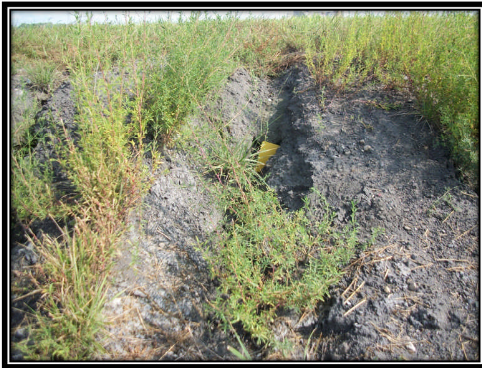
Photo 17 – Erosion Greater than 12 Inches Forming on Downstream Slopes of Southern Embankment
