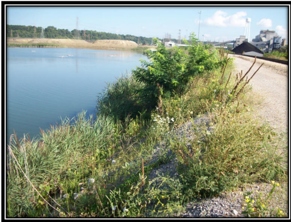
Photo 11 – Vegetation on Upstream Slope of Clarification Pond (Note Steep Slopes)
