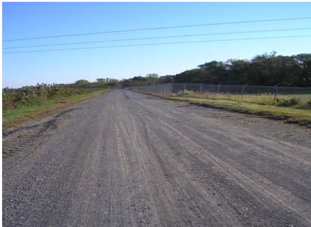
Figure 5.2.1-1: Ash Settling Pond South Crest Viewing West to East
