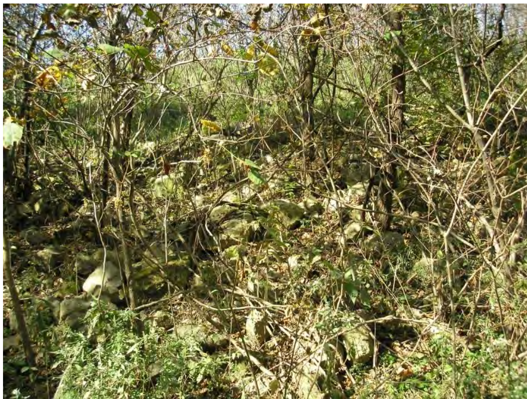
Figure 5.2.3-3: Ash Settling Pond South Dike Down-Gradient Slope Riprap Armoring
