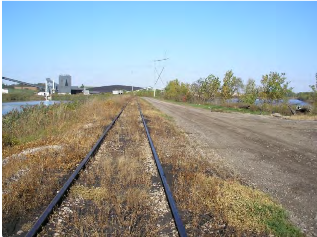
Figure 5.3.1-1: Ash Settling Pond North Dike Crest View East to West
