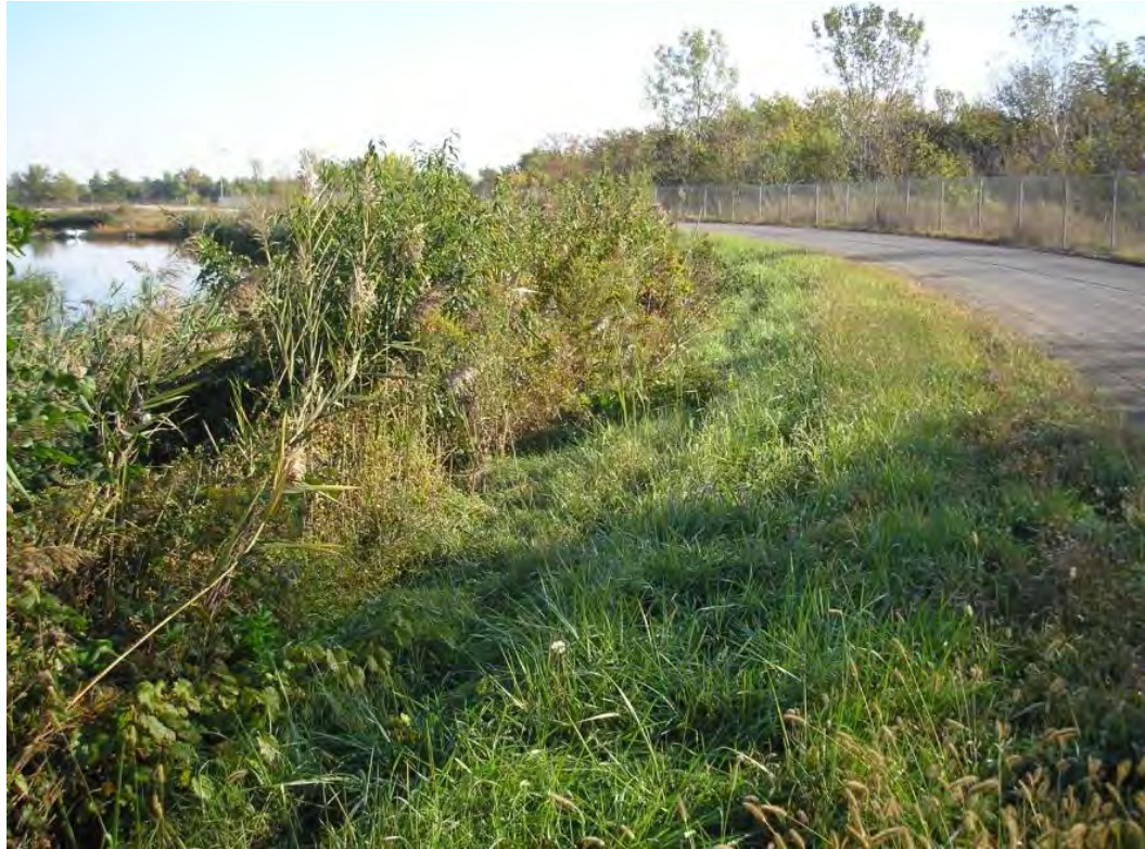
Figure 5.2.2-1: Ash Settling Pond South Dike Up-Gradient Slope at Center Section of Dike
