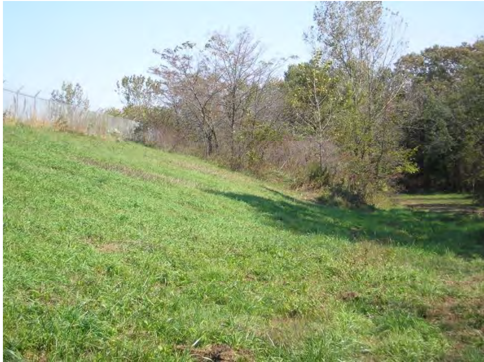
Figure 5.2.3-1: Ash Settling Pond South Dike Down-Gradient Slope at Western End of Embankment.
