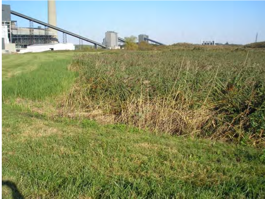
Figure 5.2.4-1: Ash Settling Pond South Dike Crest at Western Abutment
