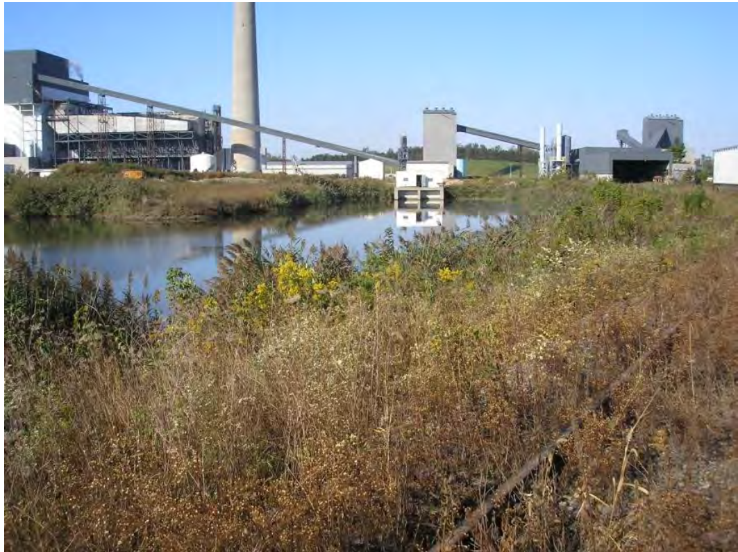
Figure 5.3.4-1: Ash Settling Pond North Dike Up-Gradient Slope West Abutment
