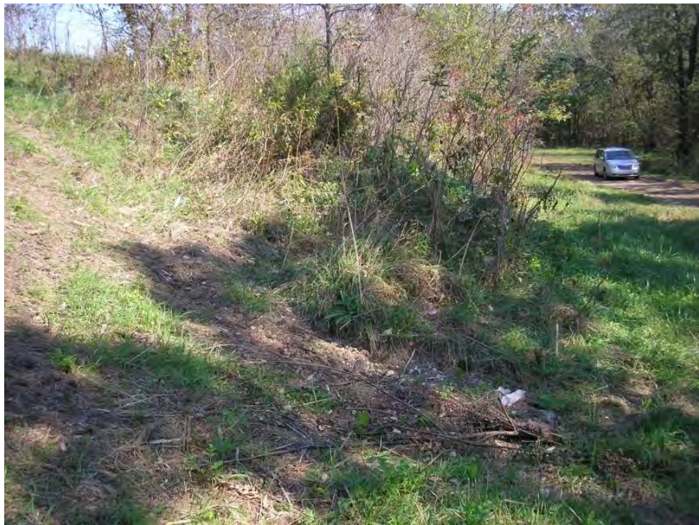
Figure 5.2.3-2: Ash Settling Pond South Dike Down-Gradient Erosion at Change from Grass Ground Cover the Woodlands
