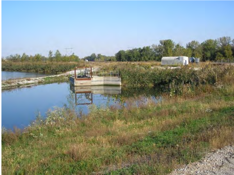
Figure 5.5.1-1 Ash Settling Pond Primary Spillway Riser Structure
