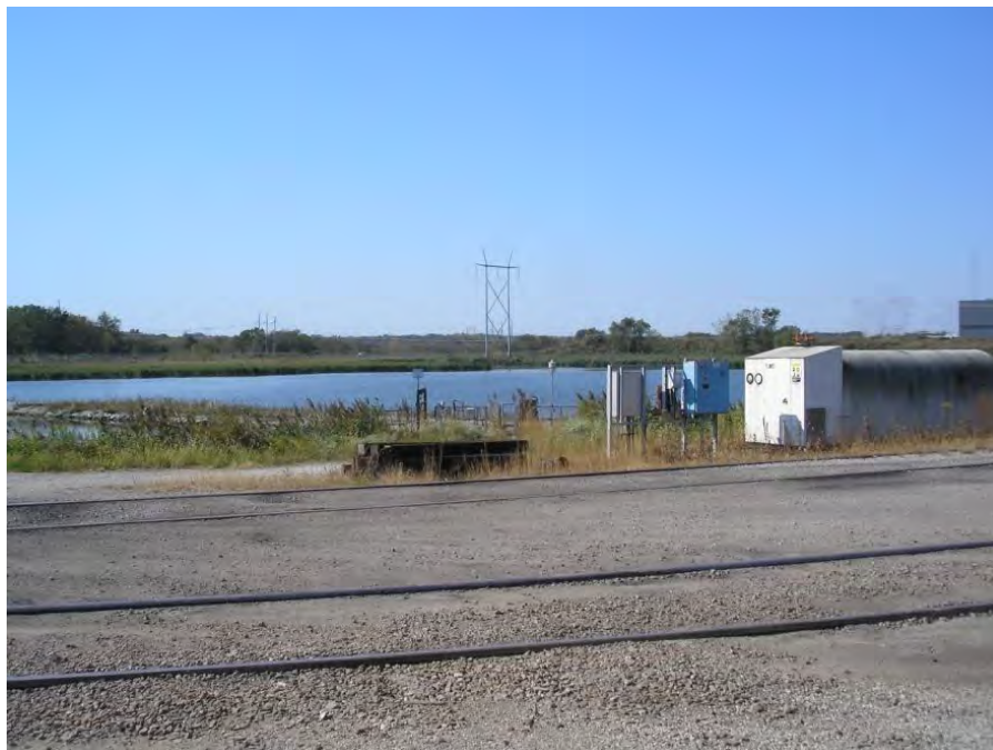
Figure 5.2.4.2: Ash Settling Pond South Dike Groin Crest at East End
