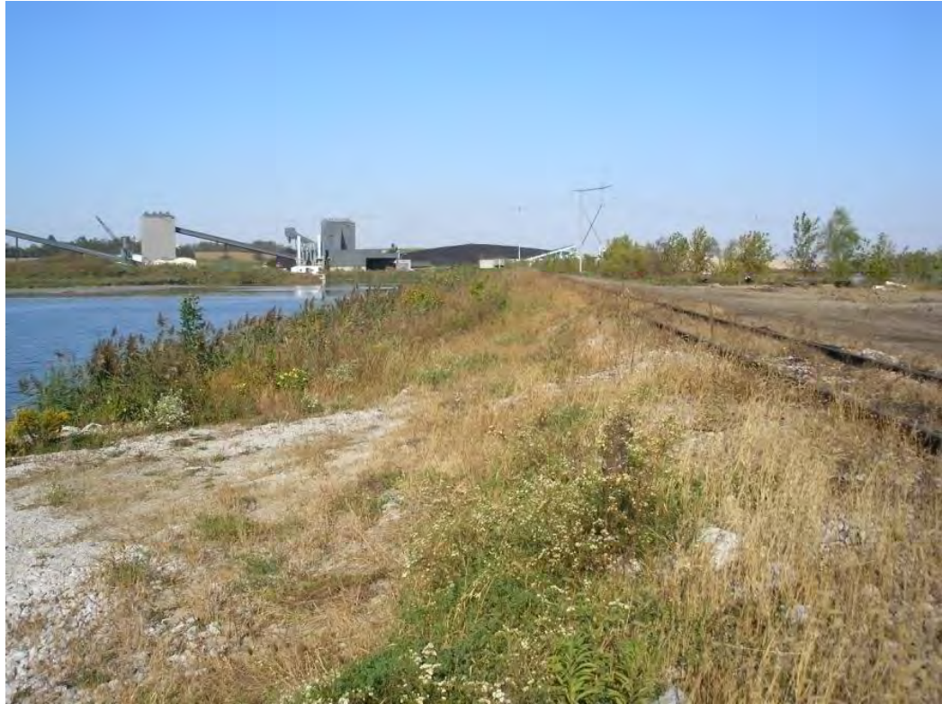
Figure 5.3.2-1: Ash Settling Pond Up-Gradient Slope View East to West
