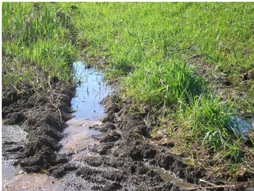
Figure 5.4.3-4: Zero Liquid Discharge Pond East Dike: Soft Wet Area Northern Section of Embankment Toe
