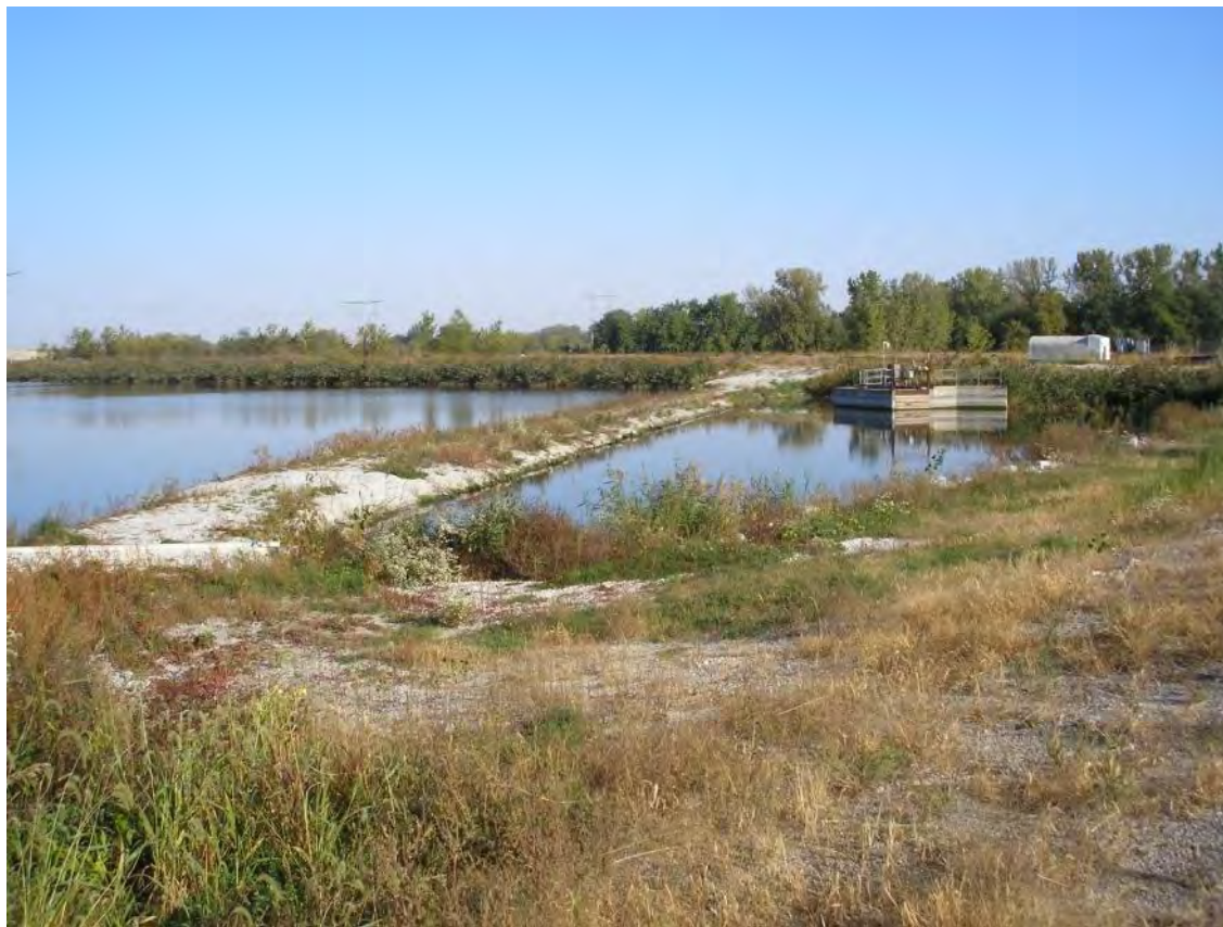
Figure 8.1-1: Low Dike and Final Settling Basin within Ash Settling Pond
