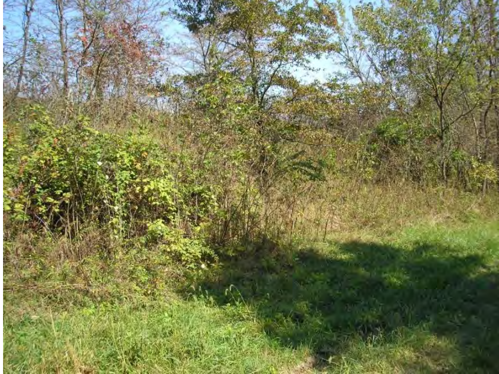
Figure 5.2.3-4: Ash Settling Pond South Dike Down-Gradient Toe
