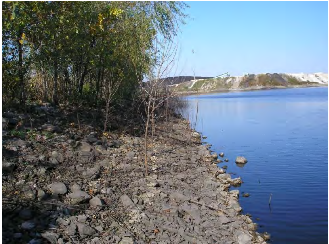
Figure 5.3.3-1: Ash Settling Pond North Dike Down-Gradient Slope
