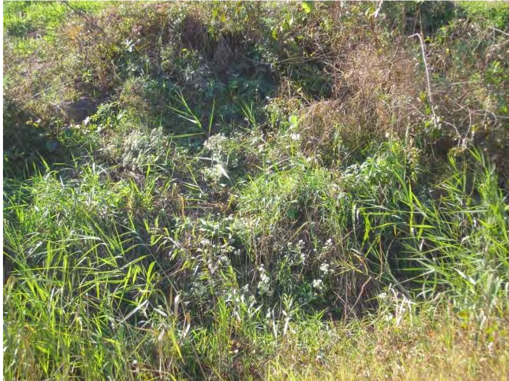
Figure 5.5.2-1: Ash Settling Pond Spillway Pipes Discharge Area. Pipe Ends Located near Upper Right Hand Corner
