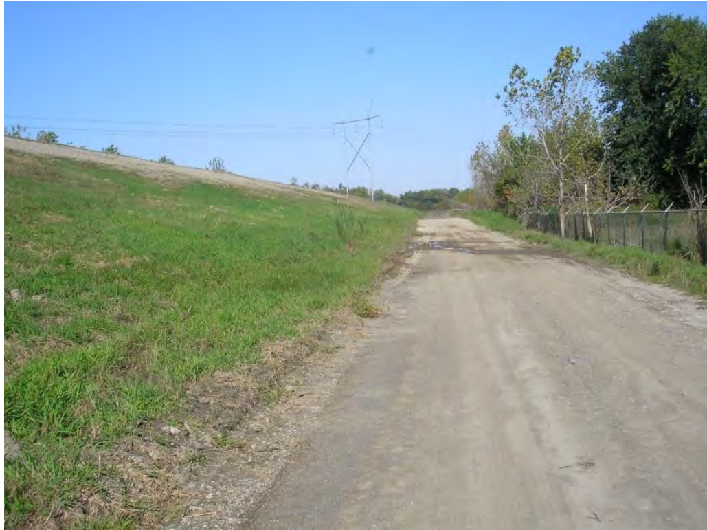
Figure 5.4.3-3: Zero Liquid Discharge Pond East Dike Toe
