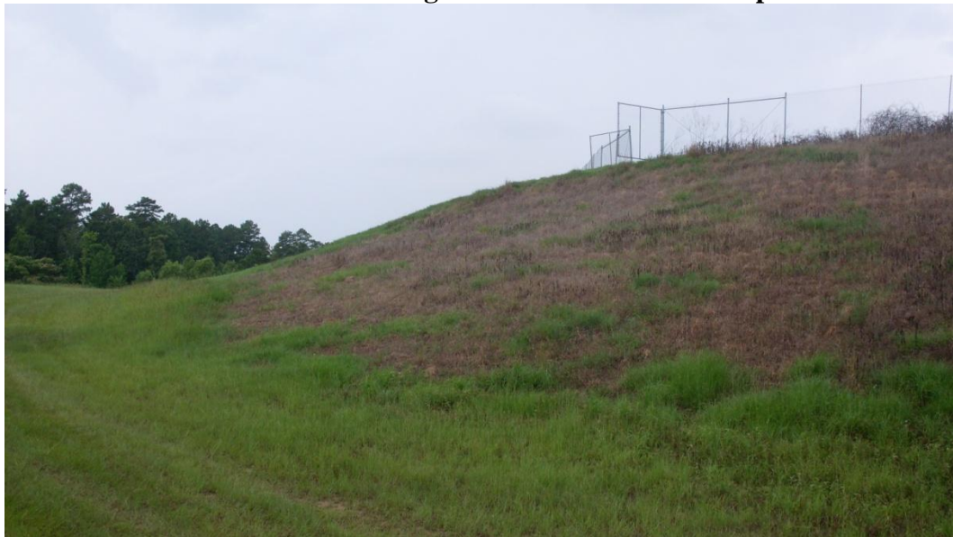
Figure 5-12: Active Bottom Ash Storage Pond Dam – exterior slope
