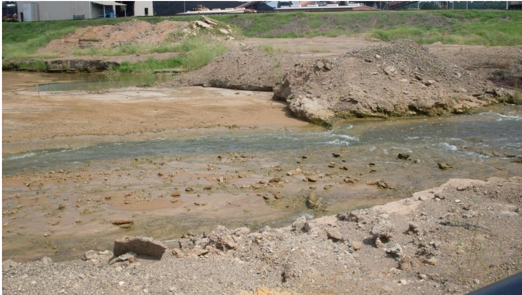
Figure 5-3 Primary Ash Pond Dam – interior slope
