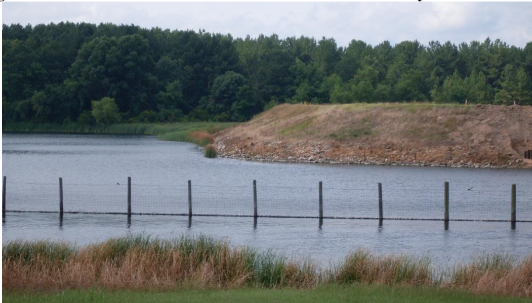
Figure 5-8: Crest and Exterior Toe around East End of Primary Ash Pond
