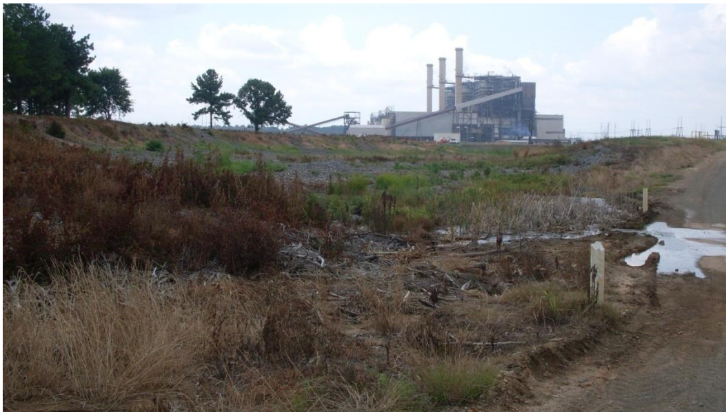
Figure 5-6: Emergency Spillway from Secondary Ash Pond to Welsh Cooling Water Reservoir
