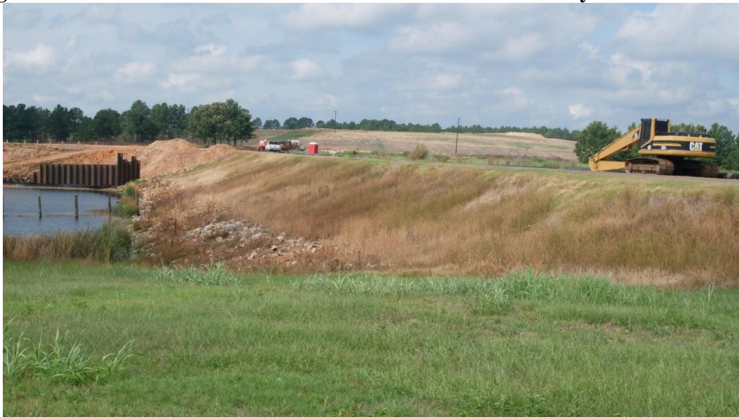
Figure 5-2: Crest and Exterior Toe around East End of Primary Ash Pond
