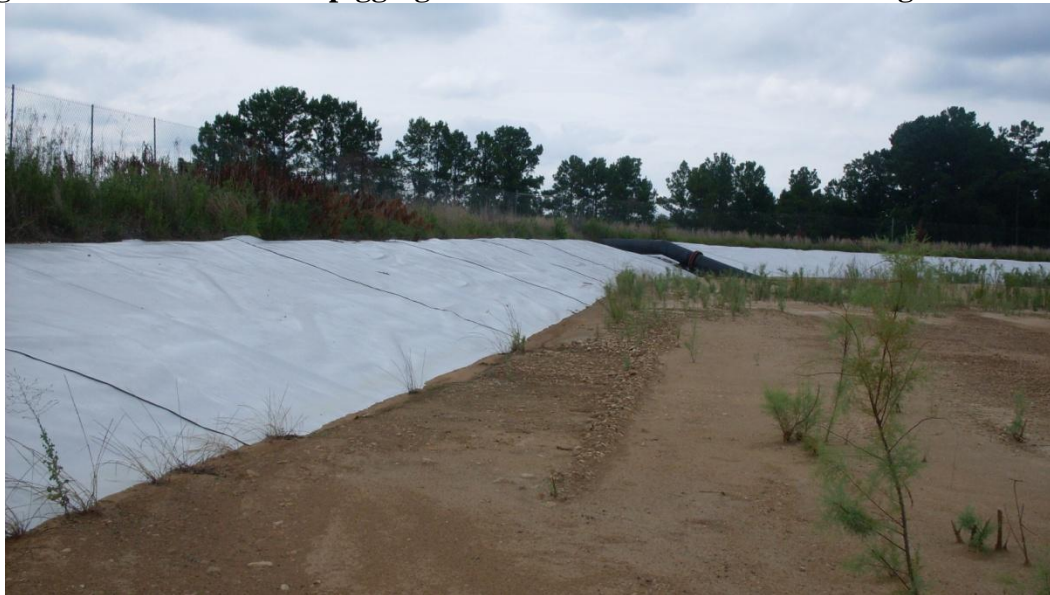
Figure 5-15: Maintenance pigging line into Active Bottom Ash Storage Pond
