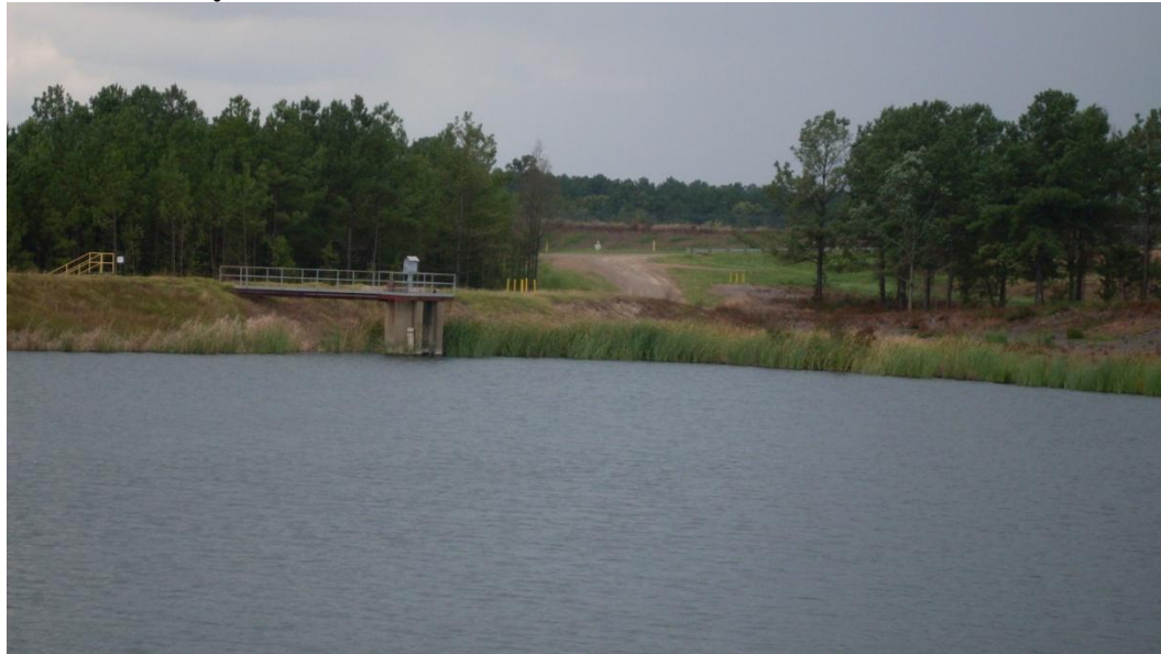
Figure 2-2: Secondary Ash Pond Outlet
