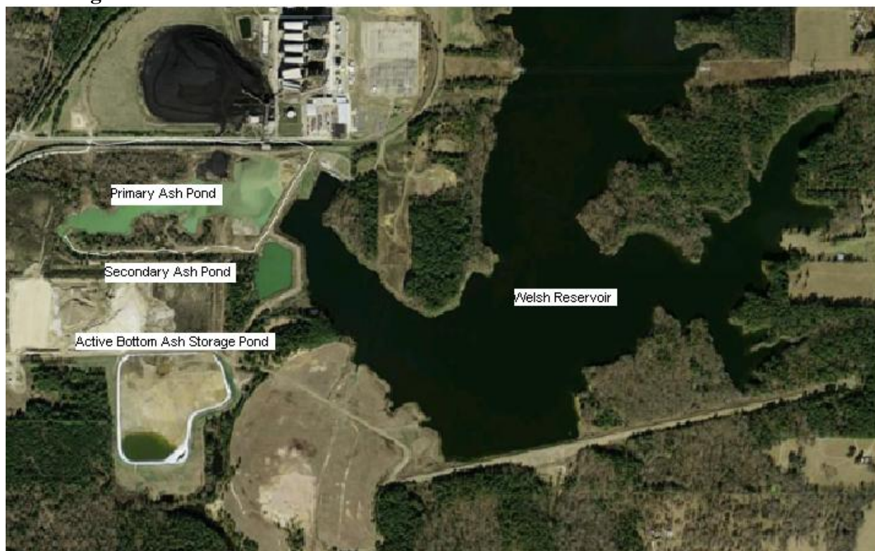
Figure 2-4: Aerial View of Ash Ponds and Welsh Reservoir
