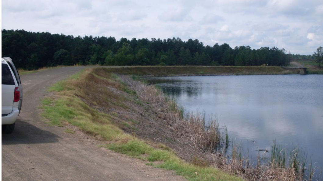
Figure 5-11: Secondary Ash Pond Dam – interior slope opposite of repairs
