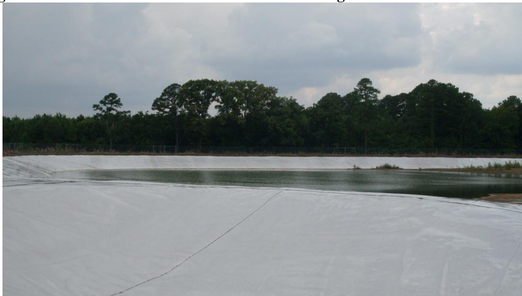
Figure 5-8: Interior Toe of Active Bottom Ash Storage Pond
