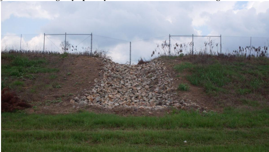
Figure 5-10: Emergency Spillway from Active Bottom Ash Storage Pond
