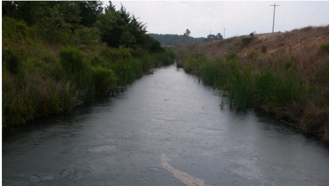
Figure 5-4: Interior Toe and Discharge Channel of Primary Ash Pond
