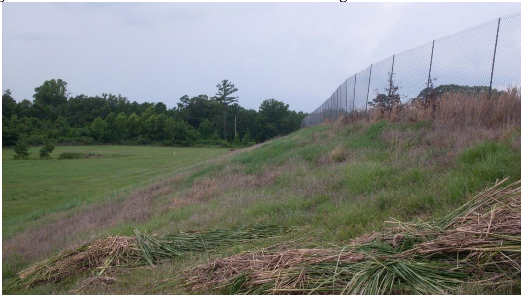
Figure 5-7: Exterior Toe of Active Bottom Ash Storage Pond
