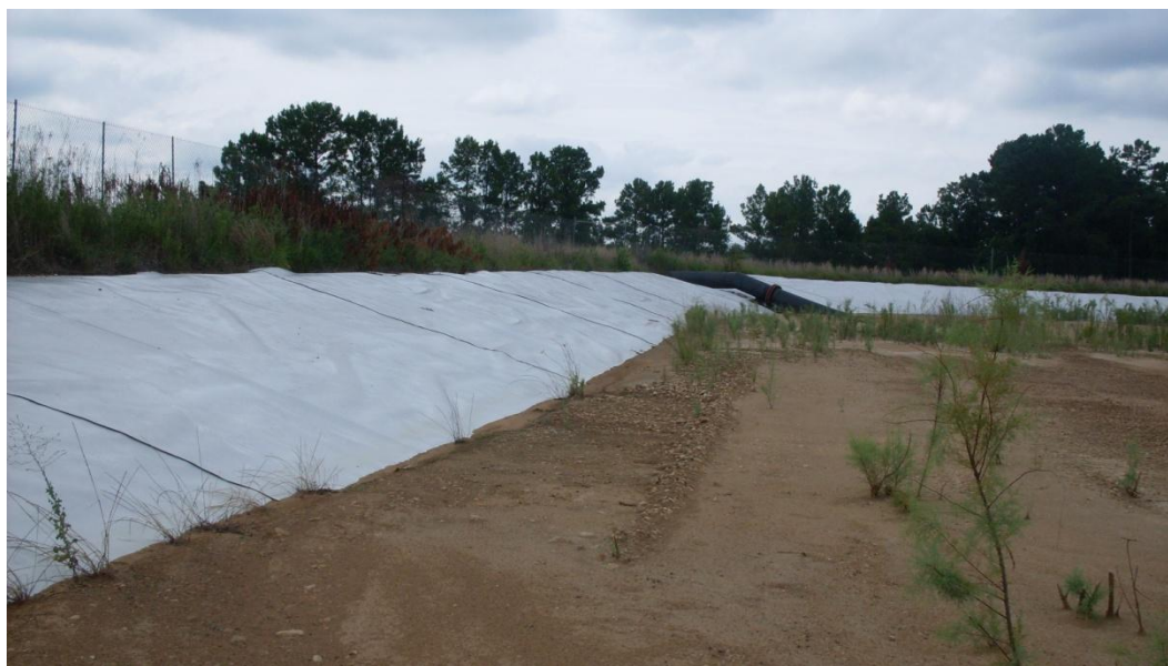
Figure 5-14: Active Bottom Ash Storage Pond Dam – interior slope
