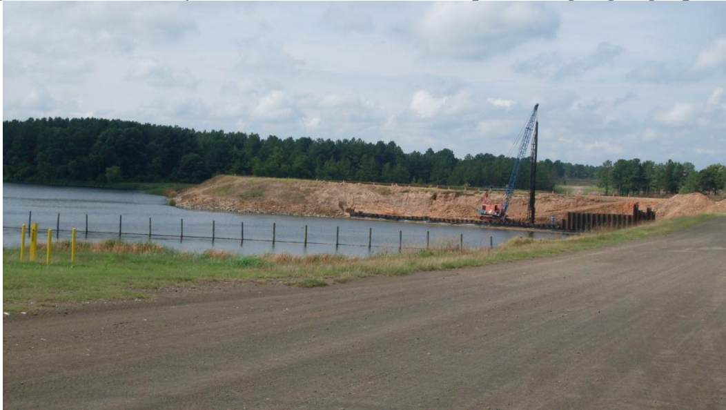
Figure 5-14: Secondary Ash Pond Dam – exterior slope showing ongoing repairs
