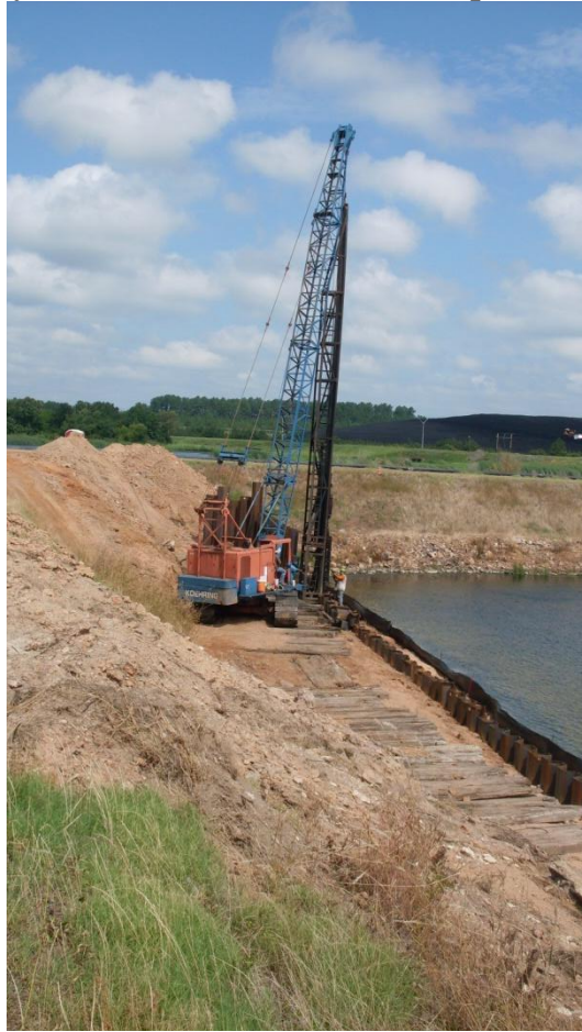
Figure 5-13: Secondary Ash Pond Dam – exterior slope showing ongoing repairs
