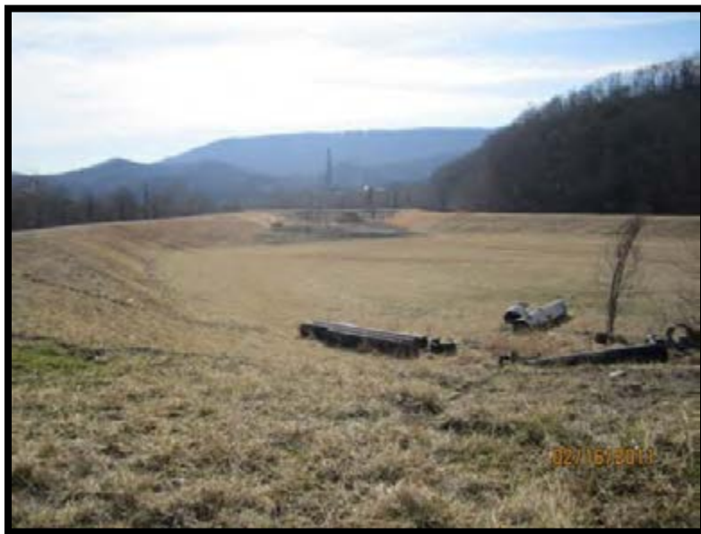
Figure 5.2.2-1: Upstream slope, Southeast. Note woody vegetation to right in foreground.
