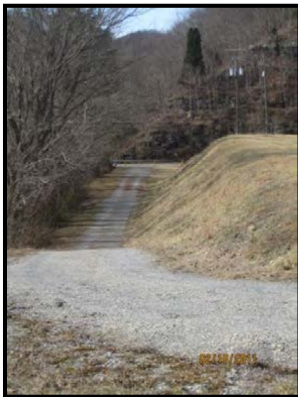
Figure 5.2.3-2: Downstream slope, Southwest.
