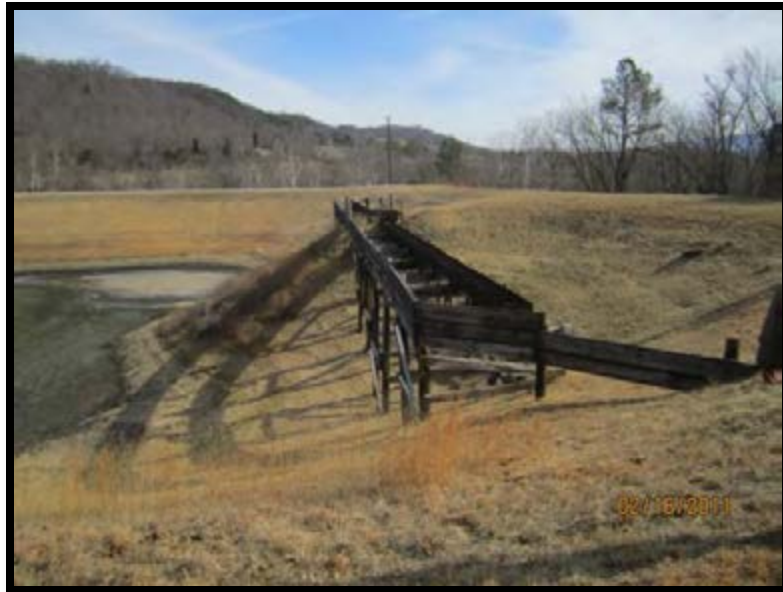
Figure 5.4.1-1: Outlet structure, Northeast.
