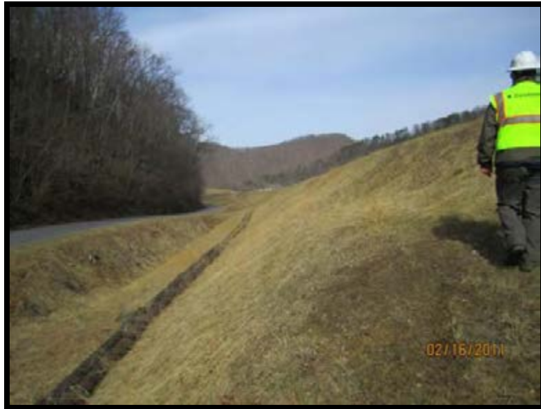
Figure 5.2.3-3: Downstream slope, Northwest.
