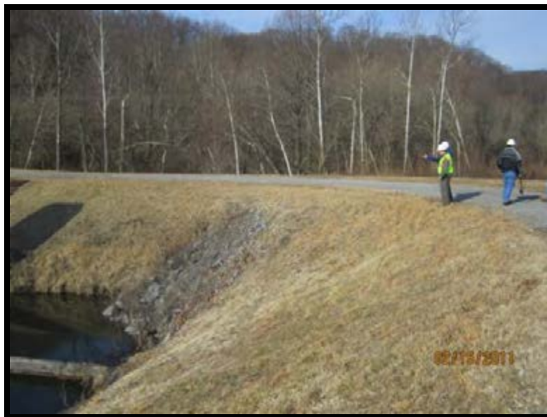
Figure 5.3.4: North groin, Note rip-rap placed in groin area.
