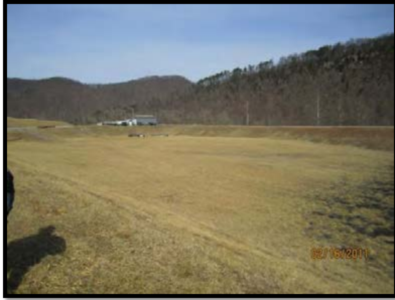
Figure 5.2.2-2: Upstream slope, North.
