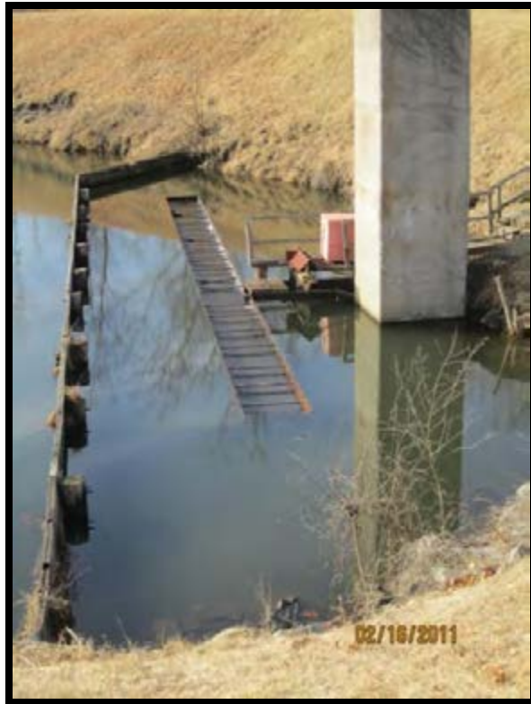
Figure 5.4.1: Outlet Structure, Southwest.
