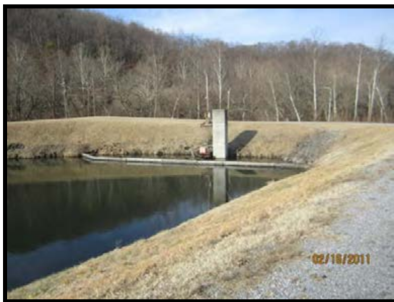
Figure 5.3.2-2: Upstream slope, Southwest. Outlet structure in the background with erosion repairs to the right.
