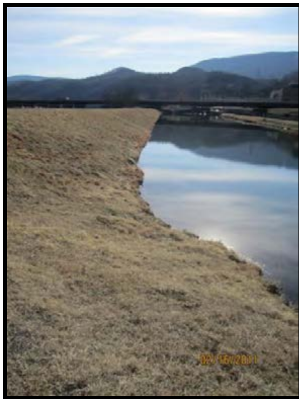
Figure 5.3.2-1: Upstream slope, Southwest.
