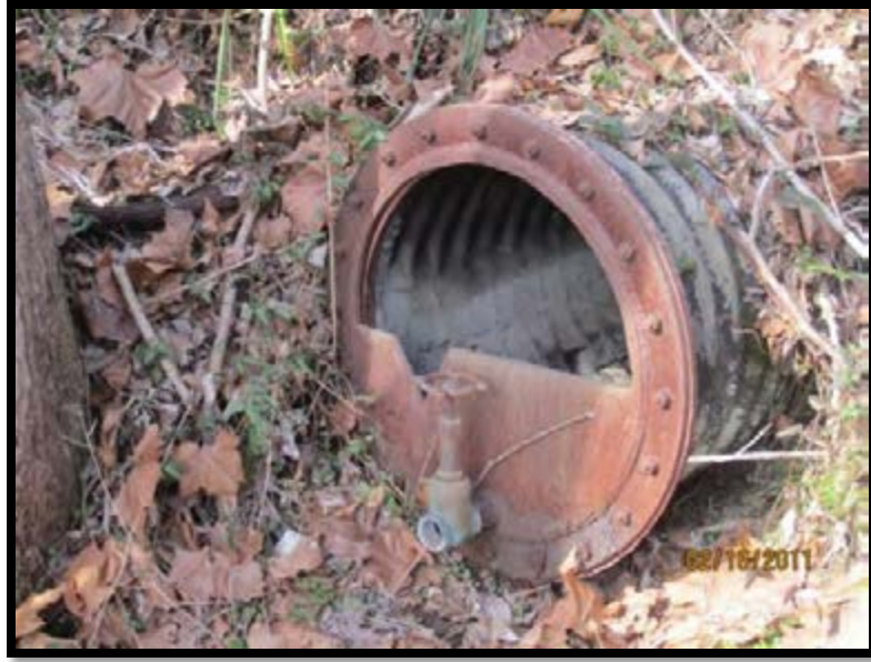
Figure 5.4.2-1: Fly Ash Pond outlet conduit to East River.
