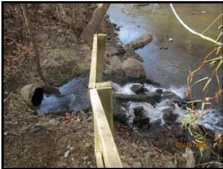
Figure 5.4.2-2: Bottom Ash Pond outlet conduit to East River.
