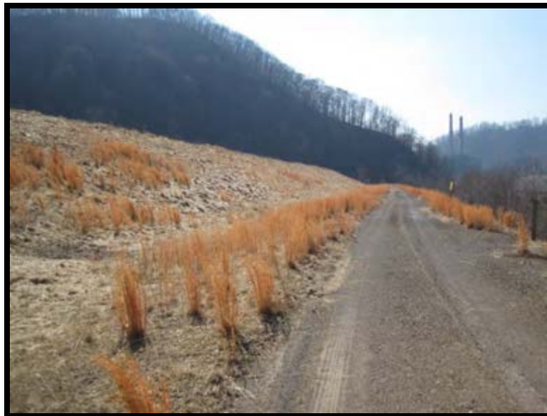
Figure 5.3.1-1: Lower dike crest, South.
