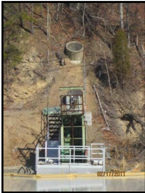
Figure 5.4.1-1: Overflow spillway structure
