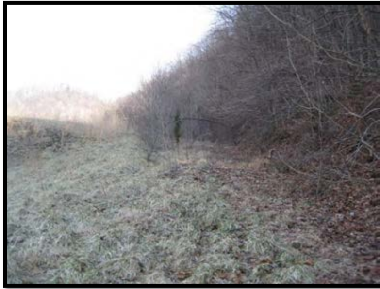
Figure 5.3.4: South abutment. Note tree growth to the right along hillside; Ash Pond 2 is to the left.
