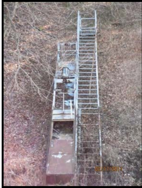
Figure 5.4.1-2: Ash Pond 2 overflow structure.
