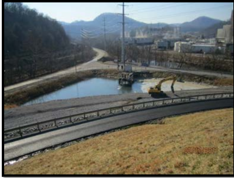
Figure 5.4.2-1: Outlet conduit outfall, reclaim pond at intersection of Route 616 and 665.
