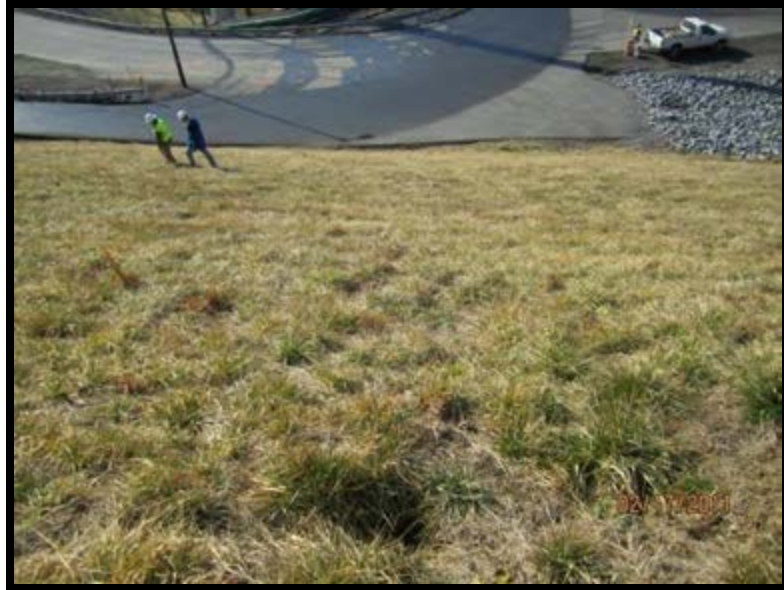
Figure 5.2.3-1: Downstream slope near access road entrance off Route 665. Note animal burrow near the crest.
