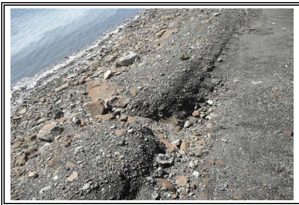
Up-close view of erosion noted in Photo # 11 showing large rock fragments in dike material.
