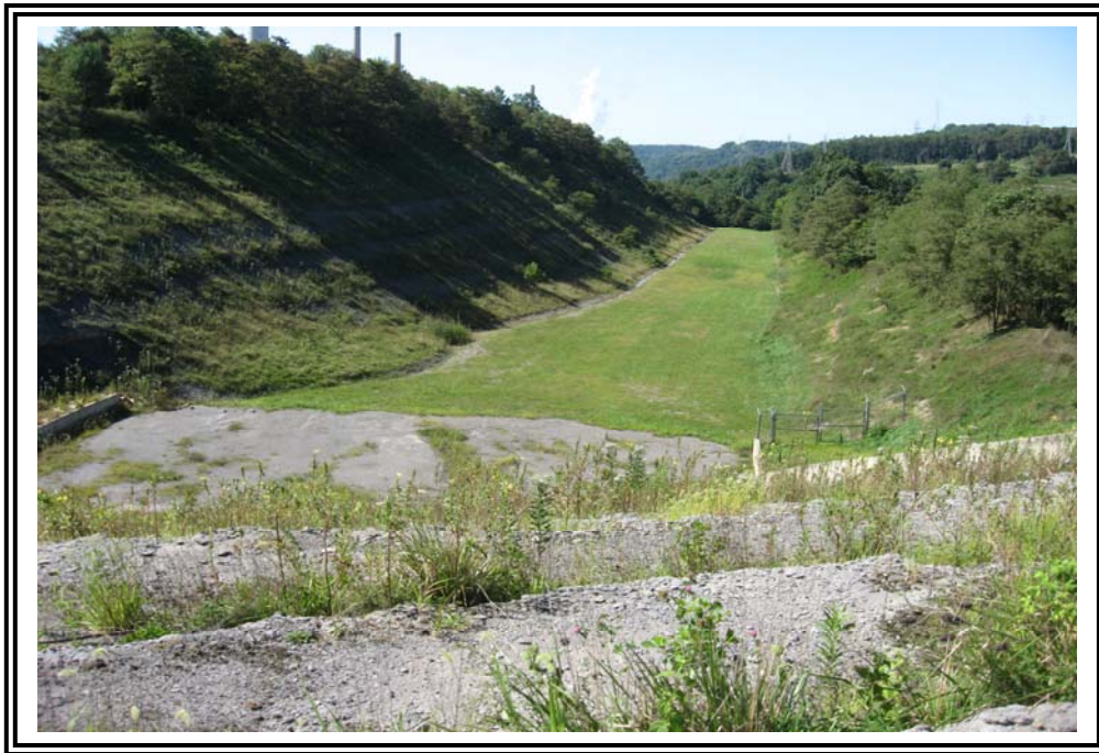
Emergency spillway, looking south from crest. Note that this spillway is excavated through hillside.
