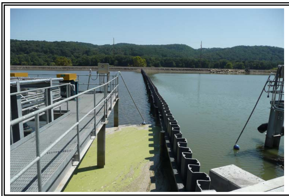
Vinyl sheet pile wall dividing recirculation pond to reduce treated water volume prior to discharge.
