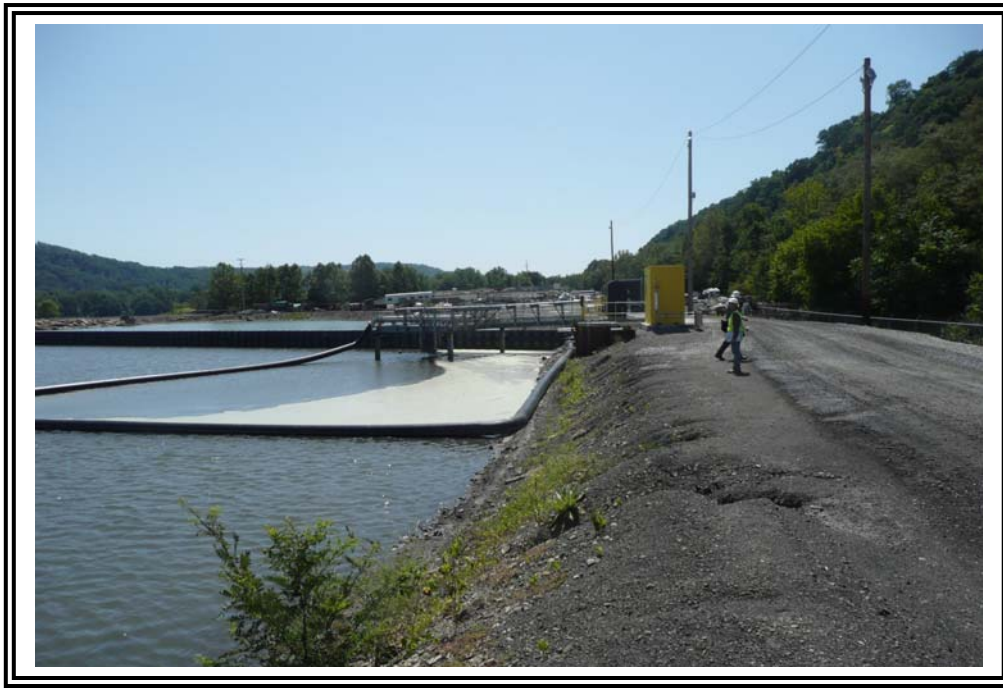
Upstream slope and crest of west dike, looking south. Note erosion feature and isolated brush. Vinyl sheet pile wall is in background.
