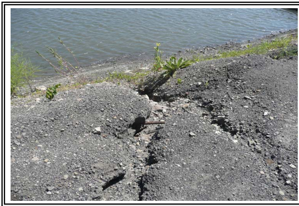
Closer look at erosion feature in Photo #36. Note exposed rebar debris in erosion gully.
