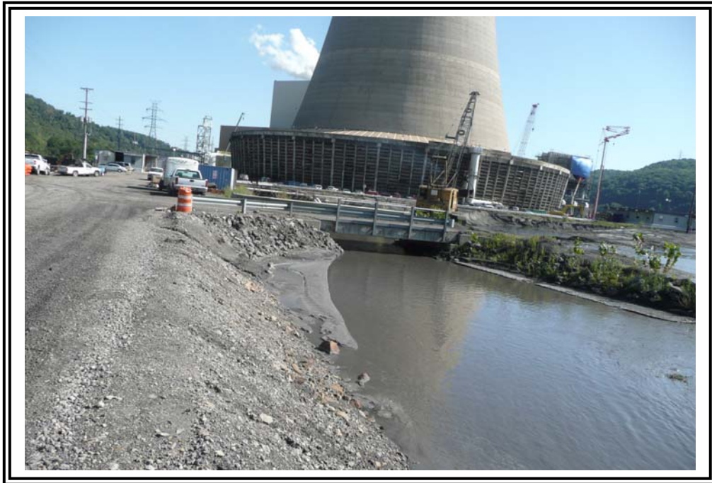
Upstream slope of west dike looking north.
