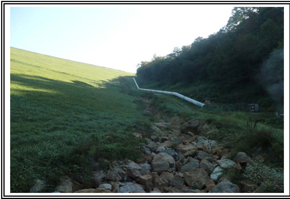
Looking upslope at left (east) rock groin and 42" diameter spillway outlet from toe drain
