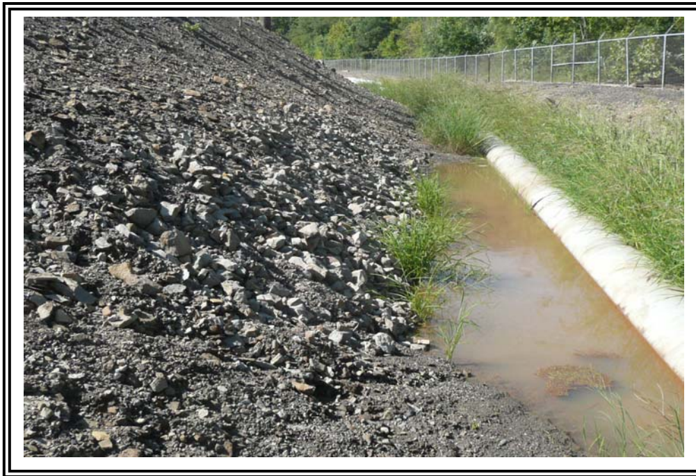
Toe of west dike where drainage has collected in pipe swale, looking south. Soil difficult to probe more than a few inches.
