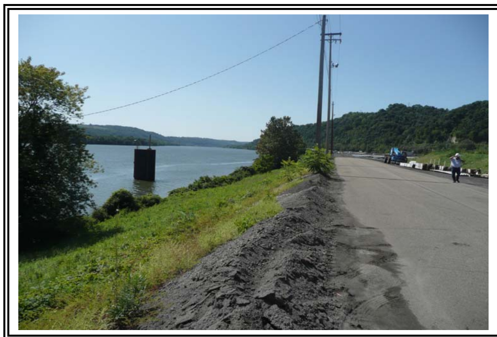
East dike crest alignment, looking south, showing ash build up at road edge due to grading activities.
