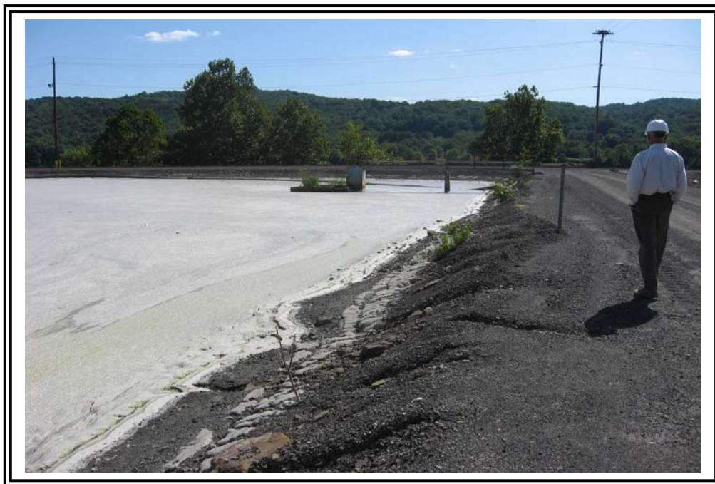
Upstream slope of separator dike, looking east. Sparse vegetation and erosion rills evident.
