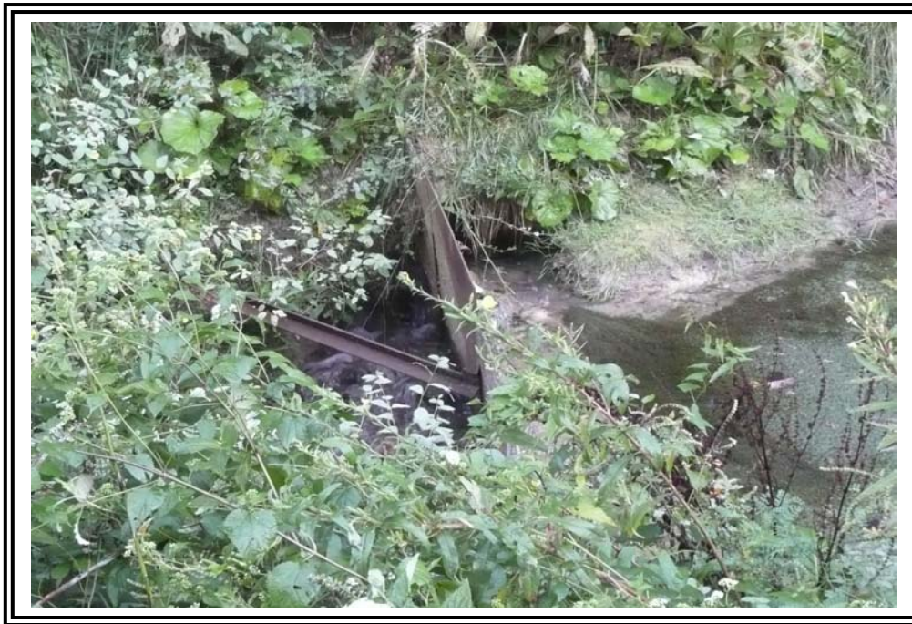
Ineffective steel V-notch weir where water flows along seepage path around weir.
