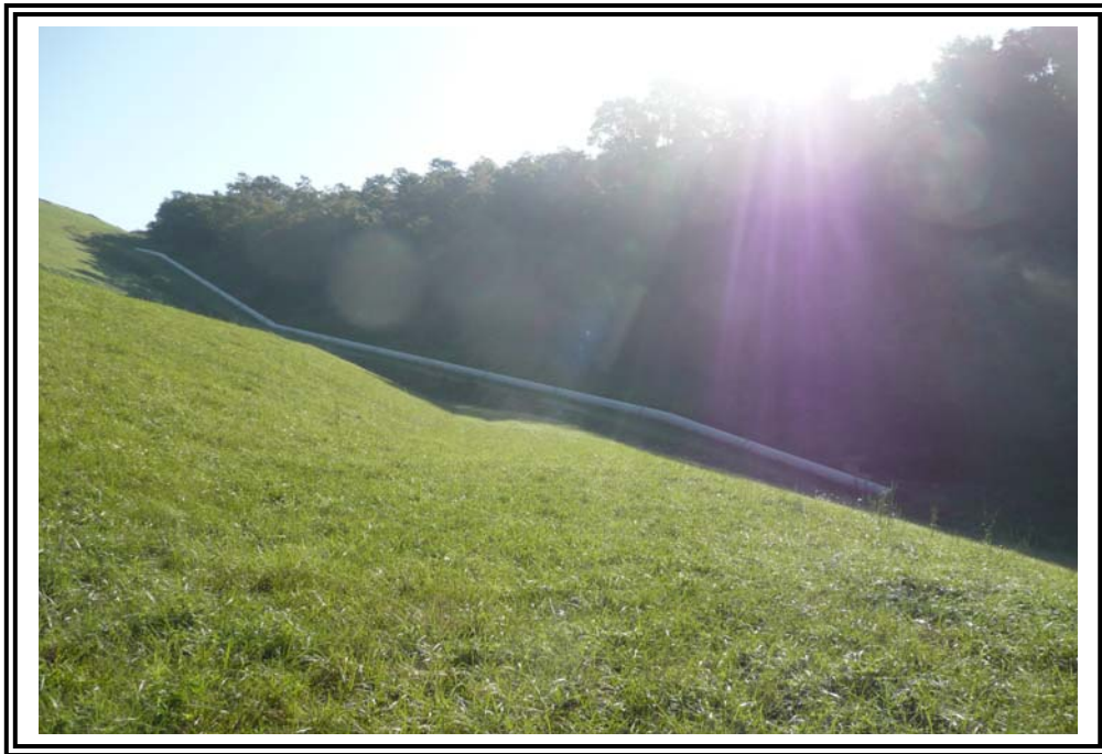
Downstream slope looking east on lower bench.
