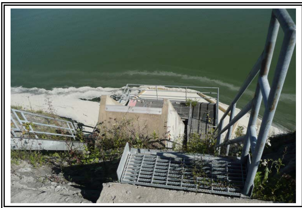
Inclined spillway from crest
