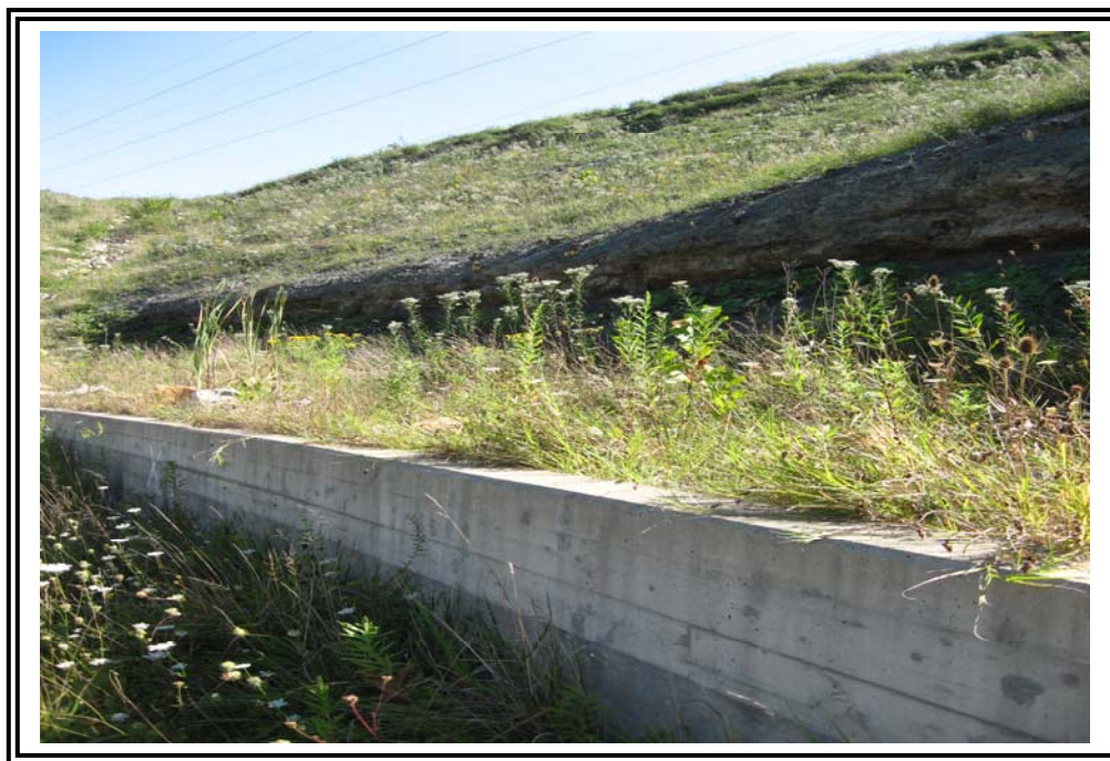
Left (east) concrete training wall at emergency spillway outfall channel. Note exposed bedrock.
