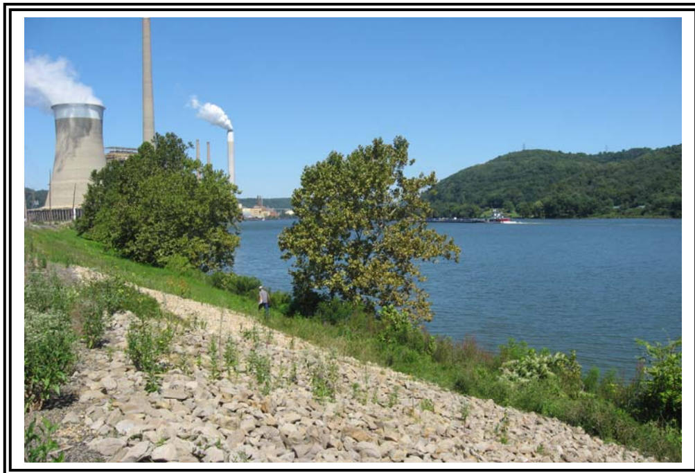
Looking north on east dike at stone facing in area of apparent seep. Seepage was not readily observed during site visit.
