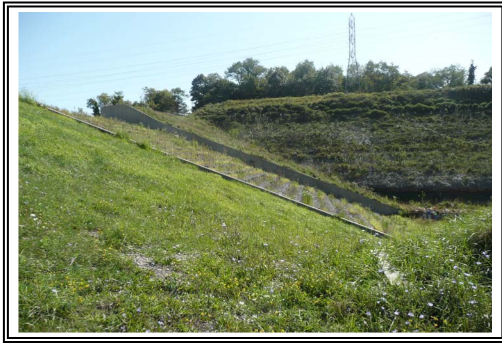
Downstream slope on RCC portion looking toward emergency spillway and left (east) abutment. Bedrock is exposed in far slope.
