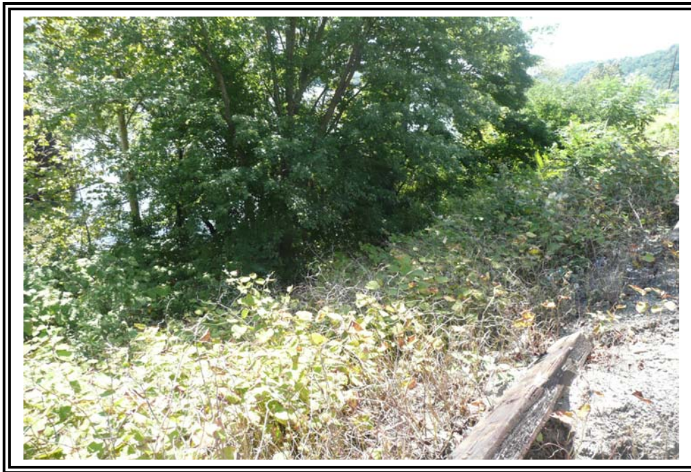
Downstream slope of east dike at northern extent of pond showing heavy vegetation and debris.
