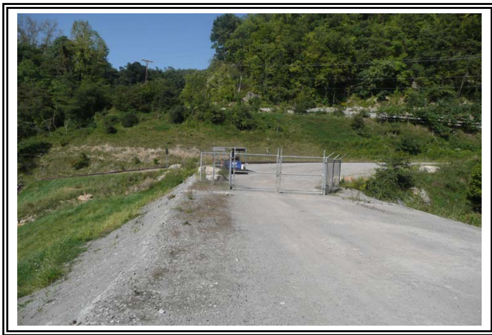
On crest looking at right (west) abutment
