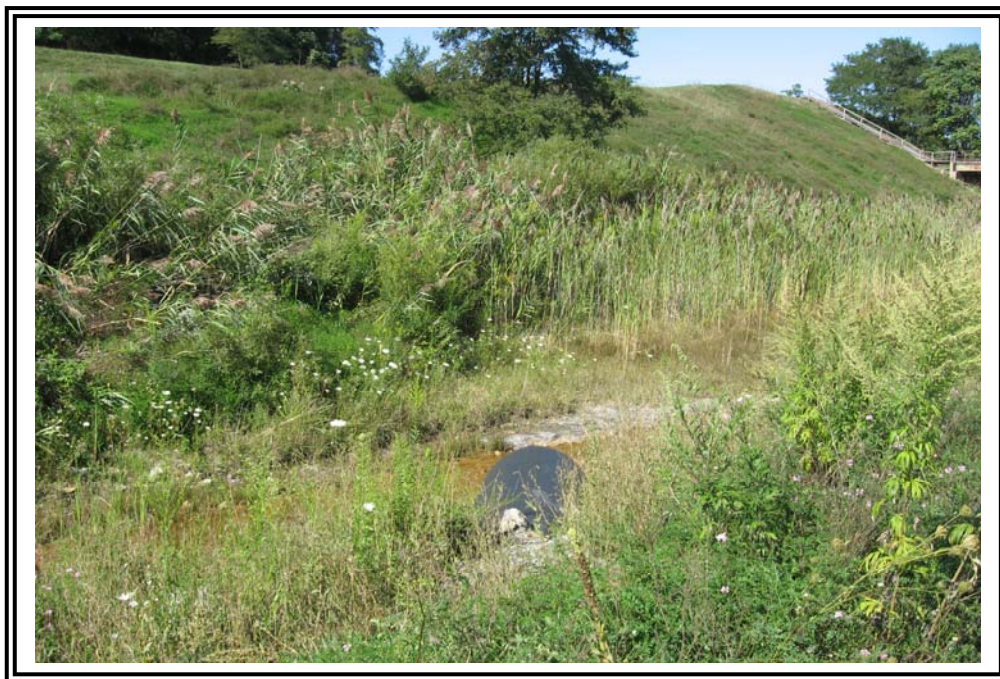
Storm runoff and site drainage outlet from landfill operation and old basin surface to emergency spillway.
