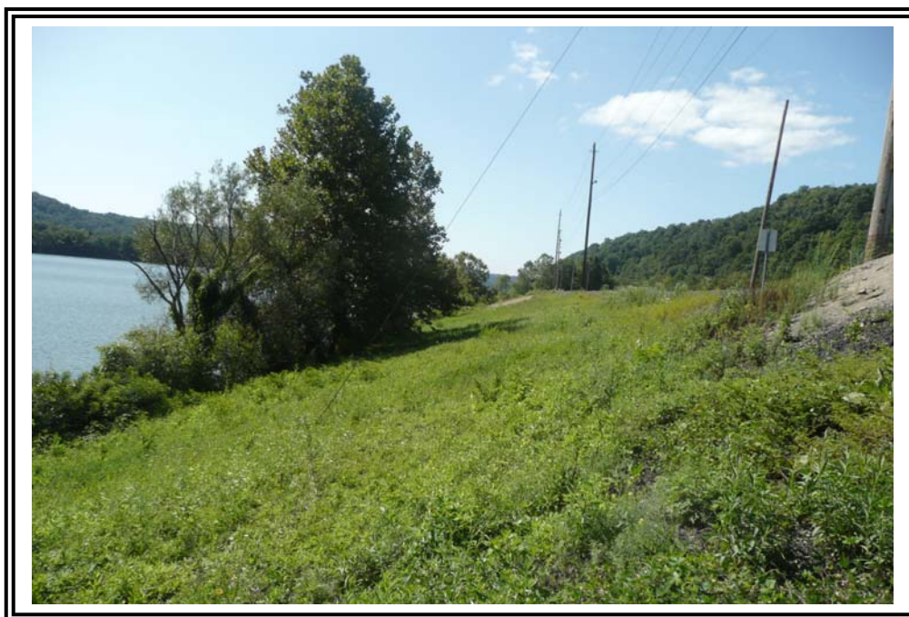
Downstream slope on east dike, looking south showing typical moderate, weedy vegetation cover on the slope face and larger brush with isolated trees at river bank.
