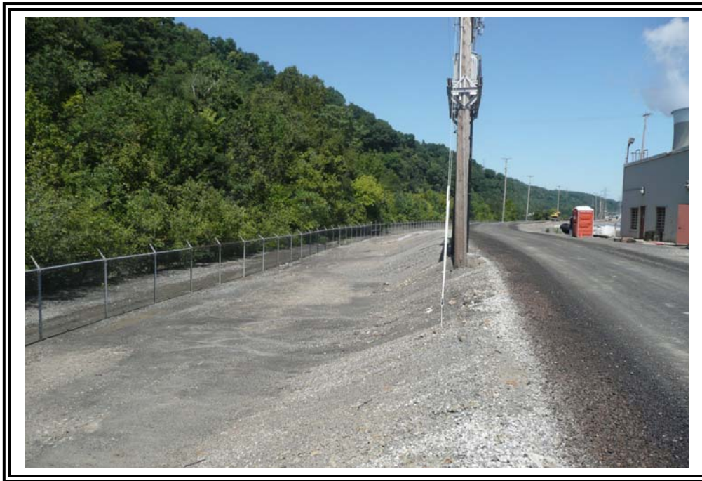
Downstream slope of west dike, looking north. Note fairly low height (about 5 feet tall) at this point.
