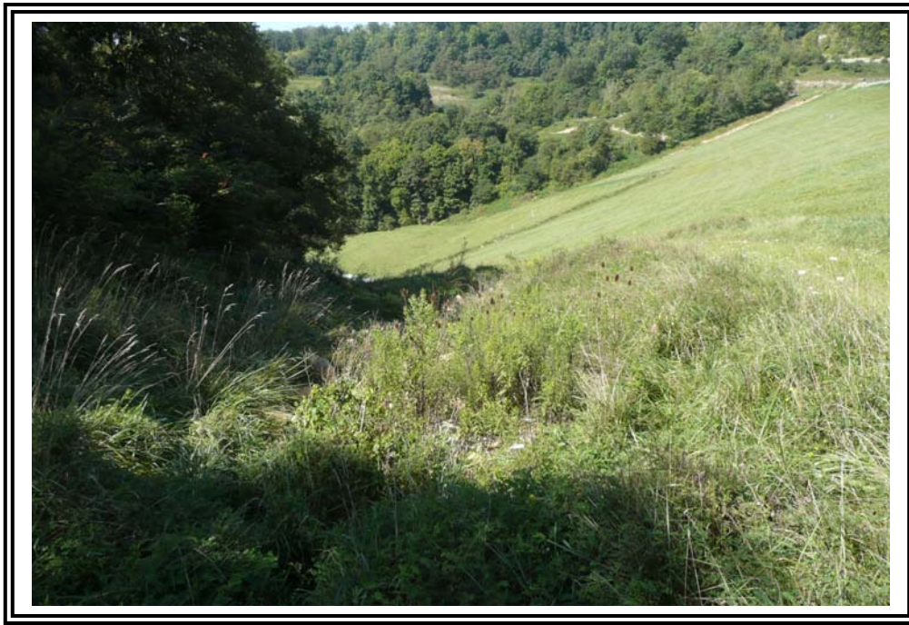
Left (east) rock groin at abutment contact. Note moderate to heavy vegetation.
