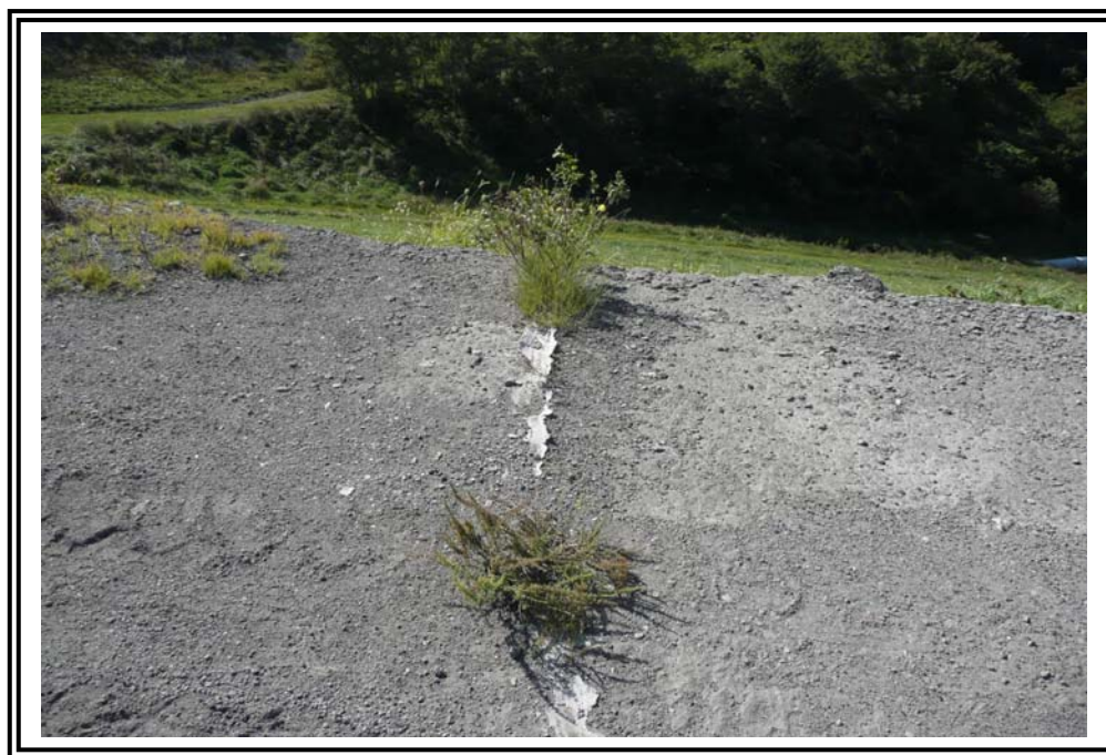
Surface expression of sealed crack at crest in RCC that initiated the diagonal joint the in inclined spillway.
