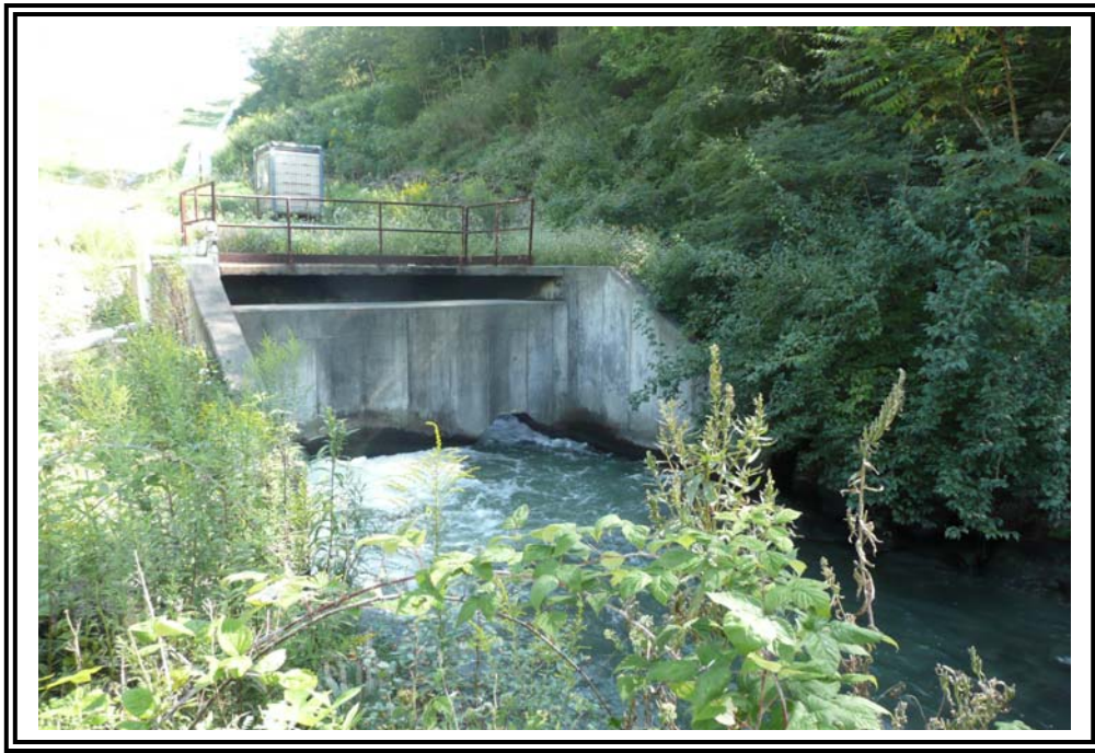
Spillway outfall and energy dissipation structure.
