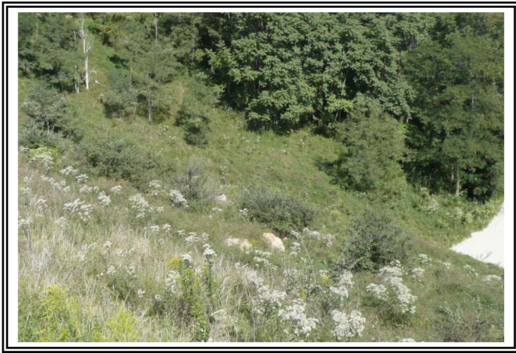
Downstream slope showing sporadic rip-rap (boulders).
