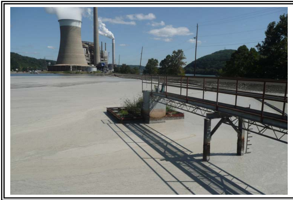
Pond spillway tower looking north.
