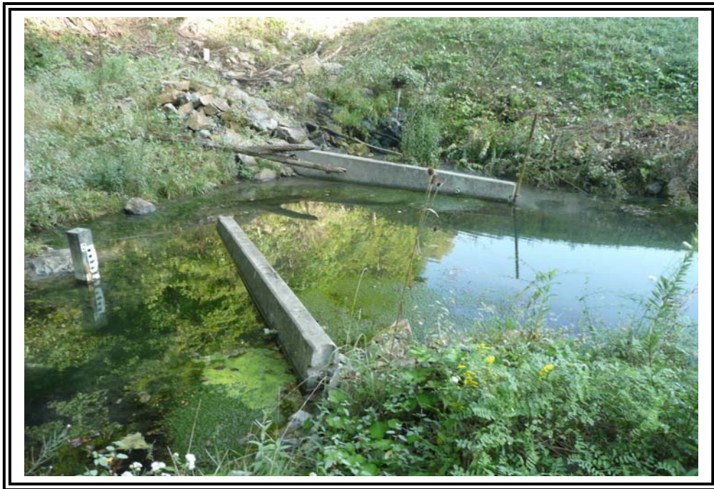
View of active toe drain discharge, seepage collection pool, and concrete baffles.
