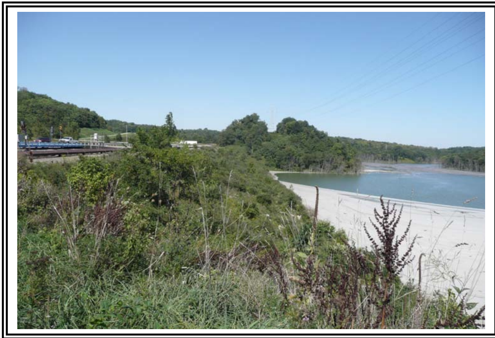
Downstream slope from right (south) abutment near crest. Note heavy wooded vegetation.
