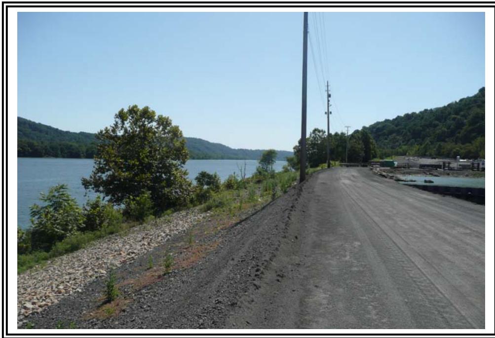
Crest and downstream slope of east dike, looking south. Note vertical limit of stone facing.
