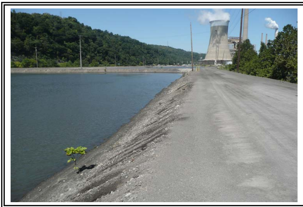
Crest and upstream slope of east dike at vinyl wall, looking north. Note typical erosion and sparse vegetation.
