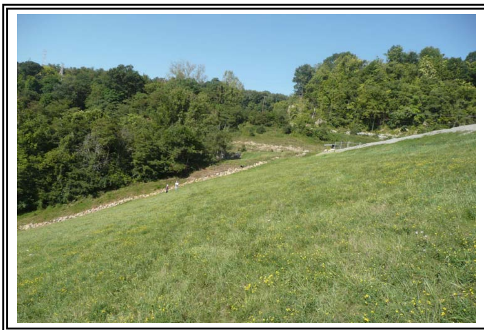
Downstream slope below crest at looking west toward right abutment. Note rock groin at abutment contact.
