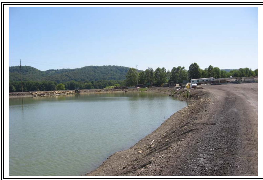
Inboard face at south wall, looking east. Pond is essentially incised in this location.
