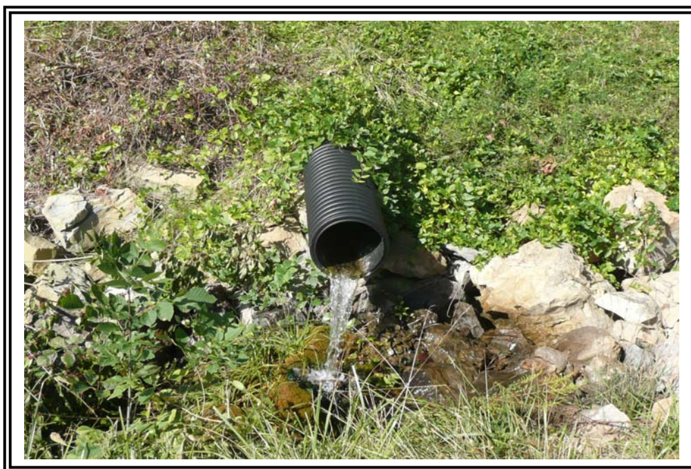
Active outlet from 12" pipe into west abutment rock groin from trench drain in natural hillside. Appears to supply most of the water flowing in the groin below about elevation 900.
