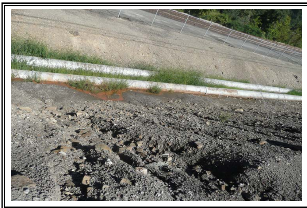
Downstream slope of the west dike, looking west. Note surface erosion and reddish brown water collecting in drainage swale around pipes showing signs of apparent corrosion and loss of coating.
