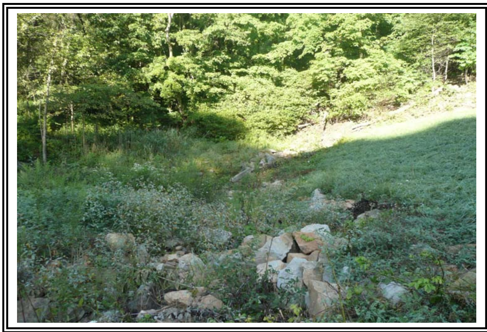
Looking west at rock toe and seepage pool in background. Note rip rap placement and vegetation.
