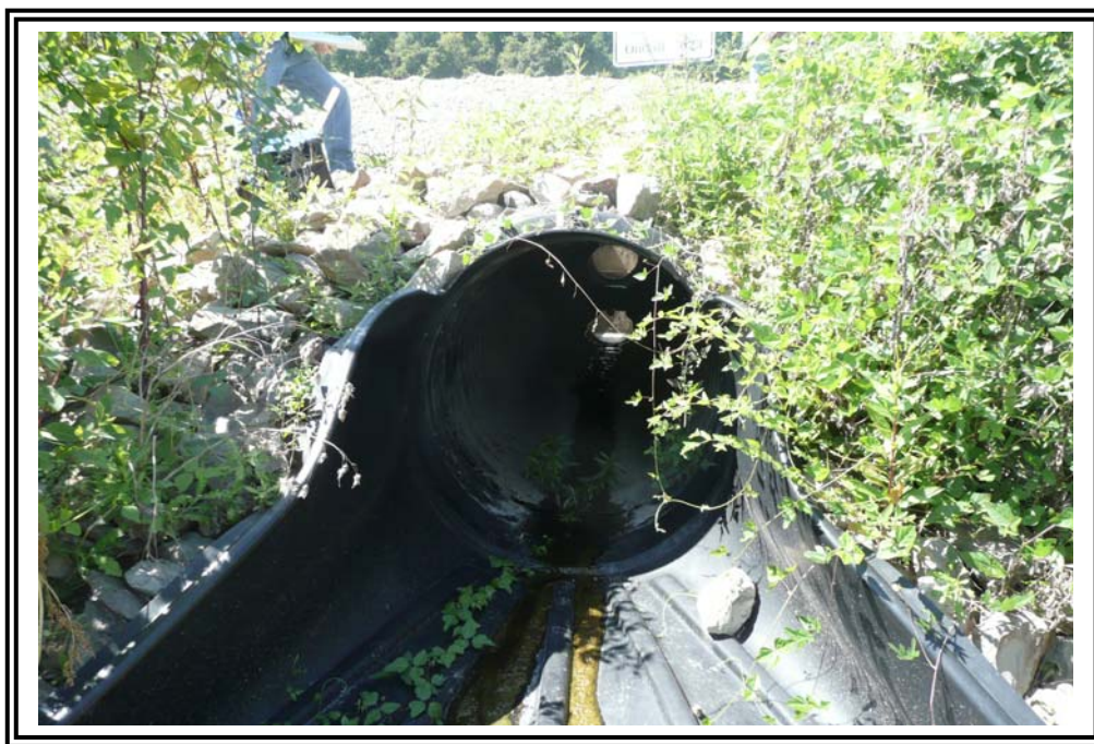
36" diameter Recirculation Pond outfall.
