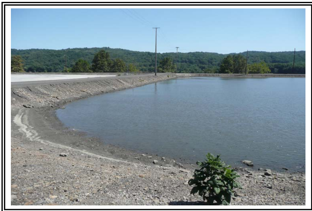
Downstream slope of the separator dike on the north side of the pond. Erosion features noted in separator dike slope.
