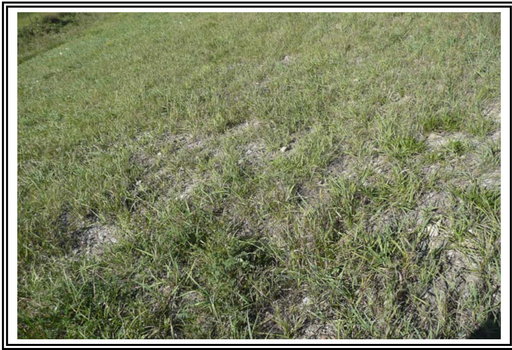
Isolated loss of grass cover and possible erosion on upper portion of downstream slope above slope groin.
