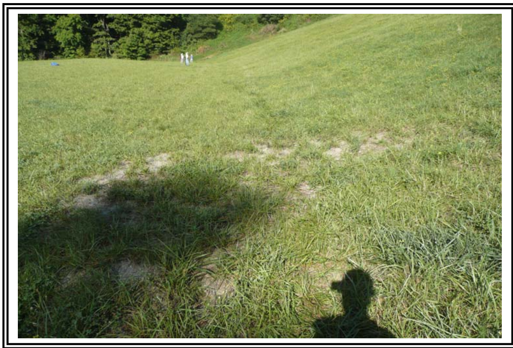
Sporadic loss of grass cover on upper bench adjacent to left (east) abutment
