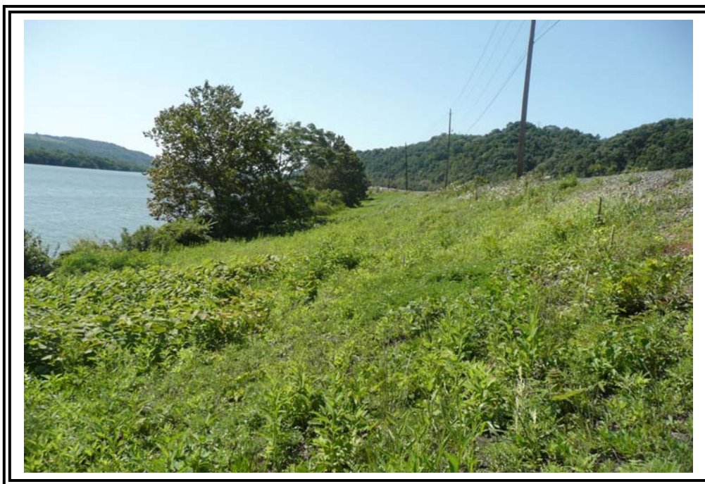
Downstream slope of east dike, looking south. Typical loss of vegetation shown at crest and change in vegetation shown adjacent to river bank.
