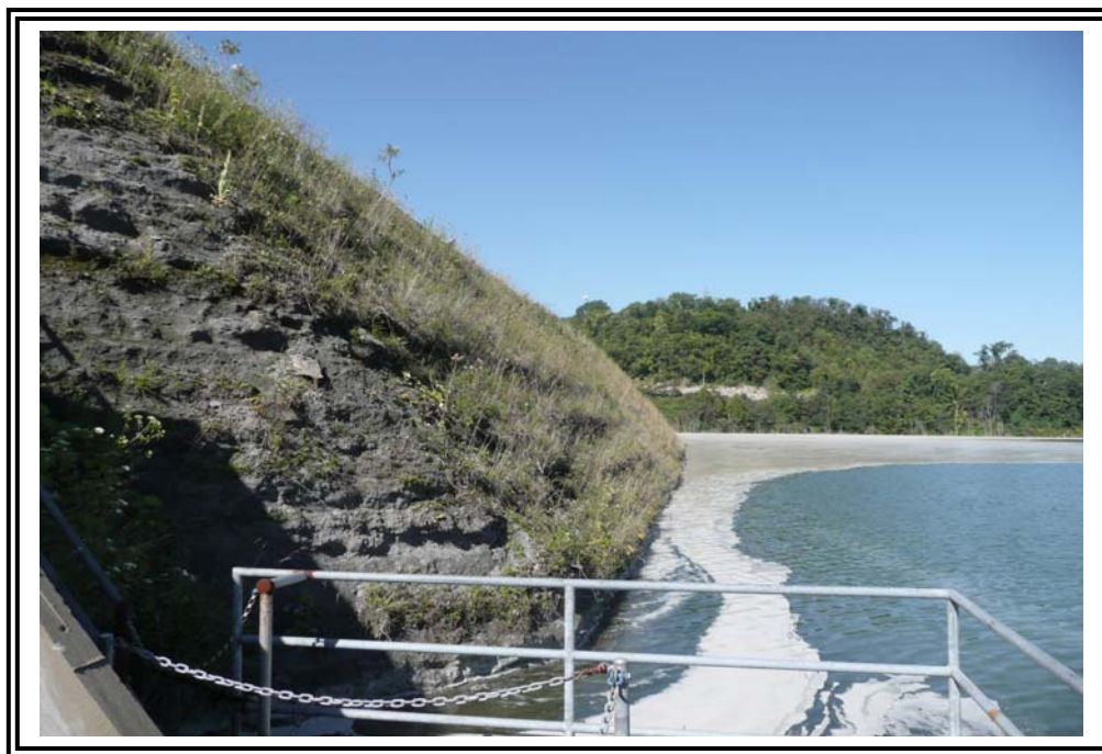
Upstream slope looking west from spillway.
