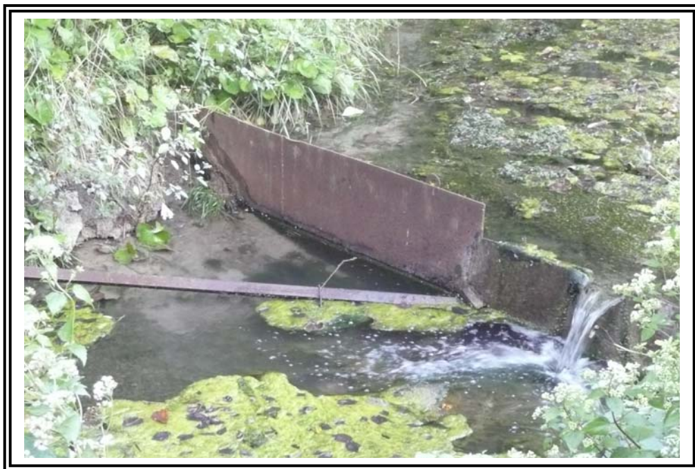
Steel V-Notch weir (typical) noted downstream of concrete weir shown in Photo No. 93
