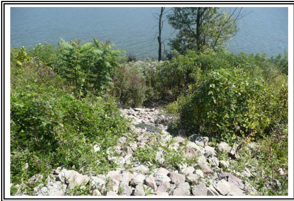
Slope protection below recirculation pond outfall.
