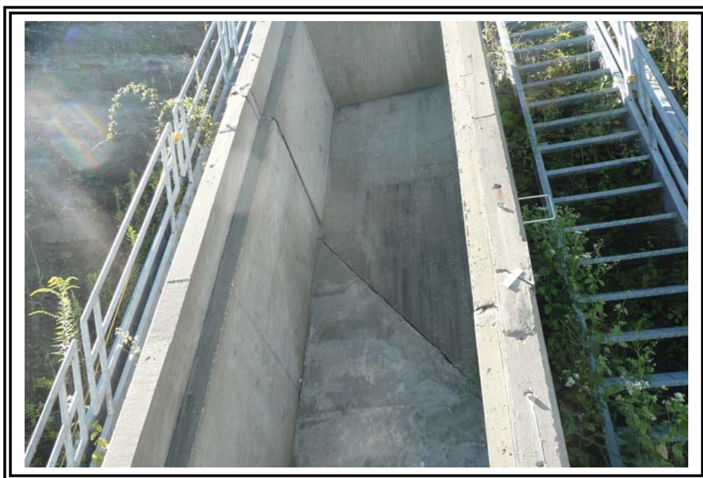
Inclined spillway looking at upstream face. Note diagonal construction deformation joint. Joint was formed to allow for some deformation due to crack in RCC during construction.
