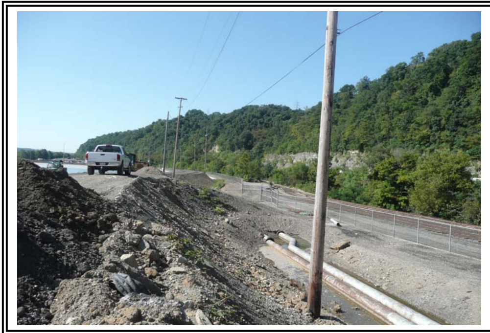
Downstream slope of the west dike looking south. Note water collecting around pipes in swale at slope toe which drains to the stormwater/wastewater and drainage sump in Photo # 9
