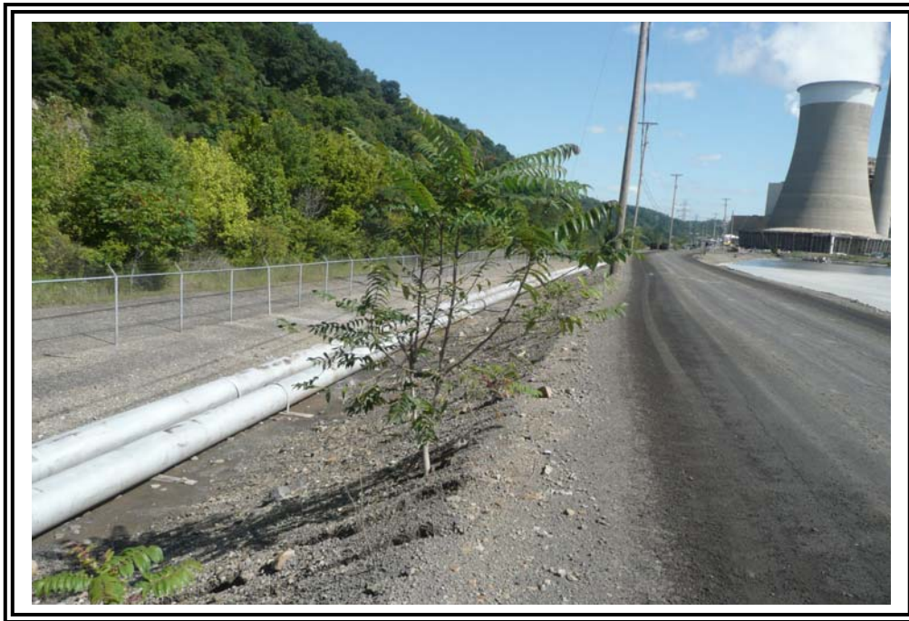
Wooded vegetation becoming established on downstream slope of west dike, looking north.
