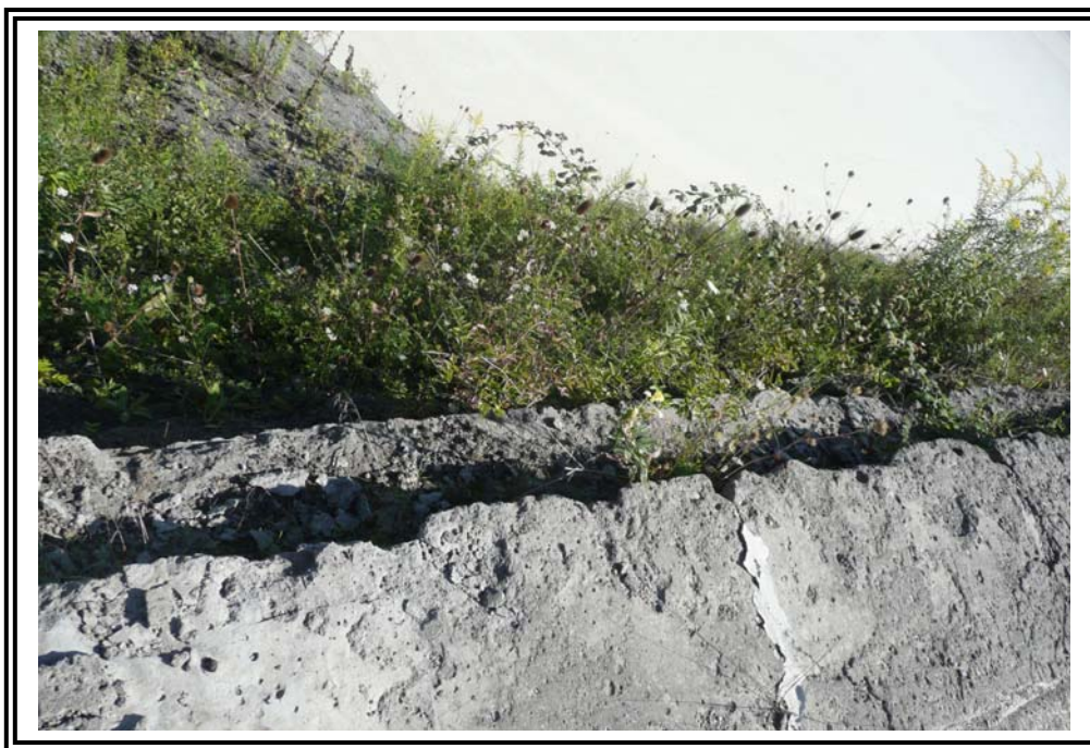
Close-up at weathered roller compacted concrete (RCC) surface and sealed crack on crest at upstream face. Note vegetation below crest level.
