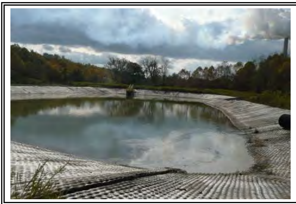
Sedimentation Basin No. 2 for general site runoff and outfall from Sedimentation Basin No.1.
