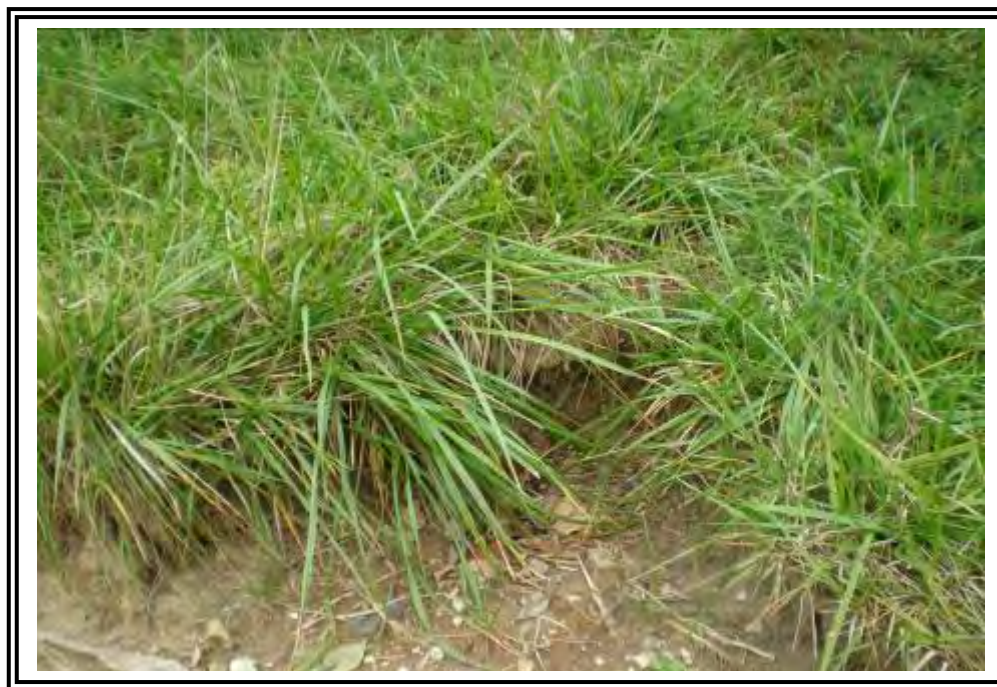
Close up of beaching erosion on upstream slope.
