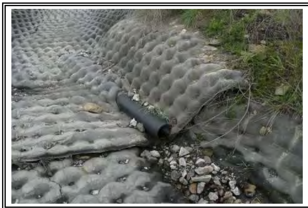
6" diameter abutment drain outlet to west (left) abutment groin below active bench; seepage clear. Groin dry above this level.
