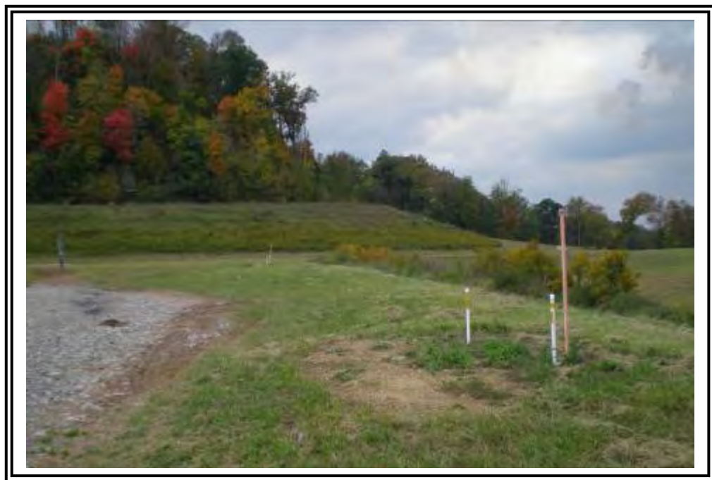
Instrumentation on the dam crest, looking west.
