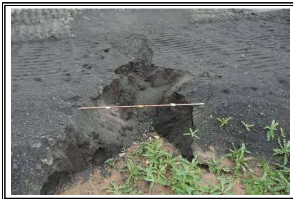
Erosion gully at top of the bottom ash drainage blanket being placed on the active buttress landfill bench.
