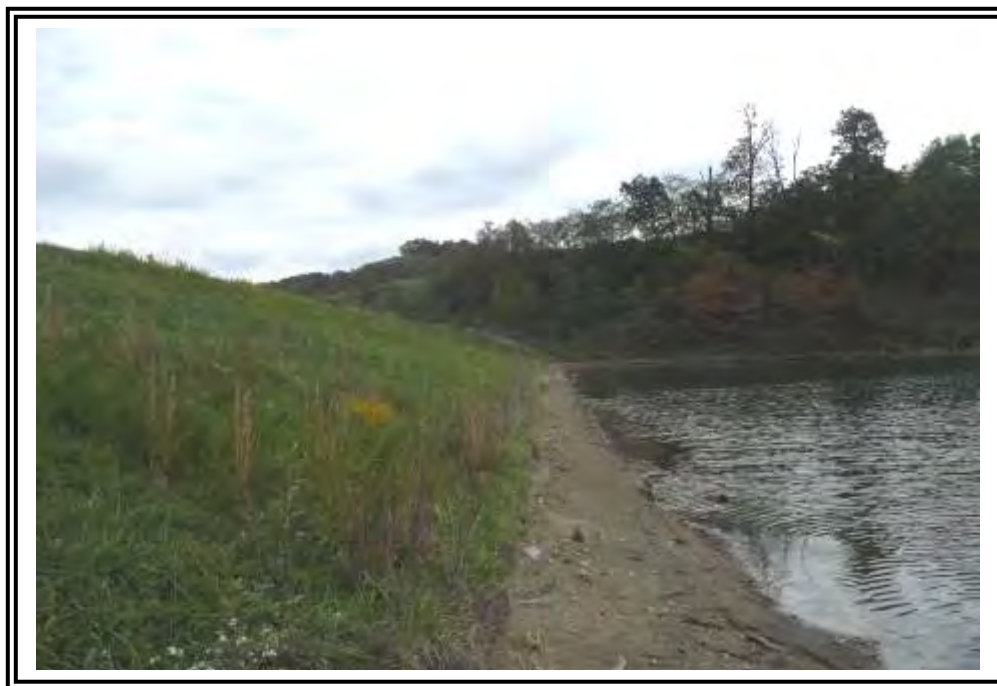
Looking east along upstream slope face with another view of the soil exposed below the grass line.
