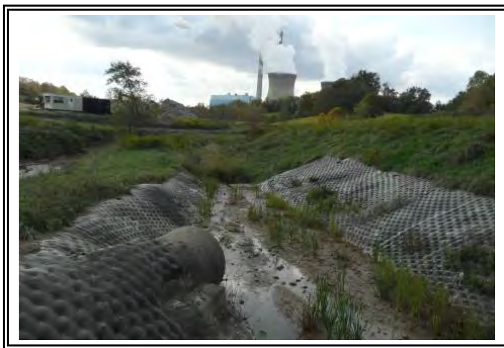
Looking downstream at spillway outlet basin.
