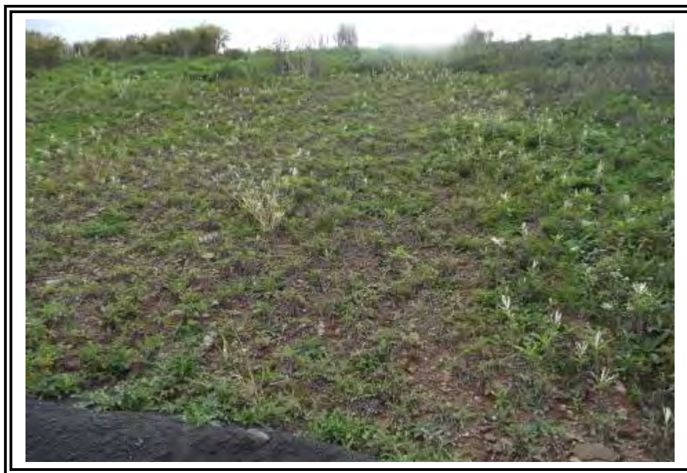
Another area of thinning grass cover and potential erosion above bottom ash drainage blanket.
