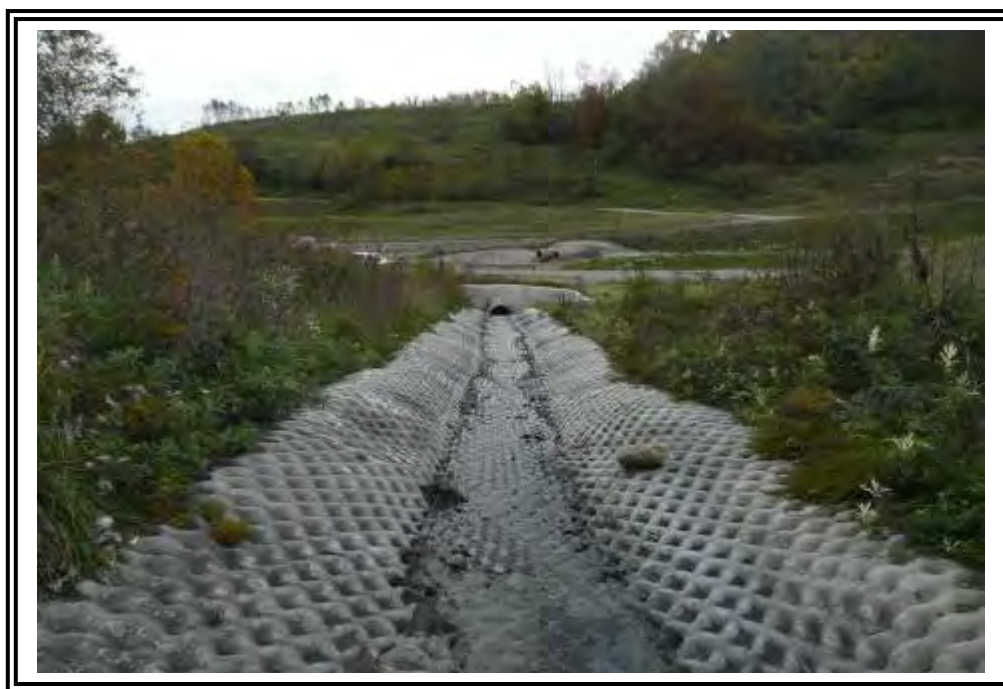
Looking down-slope at fabric formed concrete groin on west (left) buttress landfill abutment.
