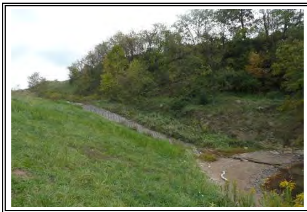
Upstream slope at right (east) abutment contact, looking east. Break in tree line above slope is location of upstream core trench at the right abutment contact. Note Fabriform lined groin at abutment contact.
