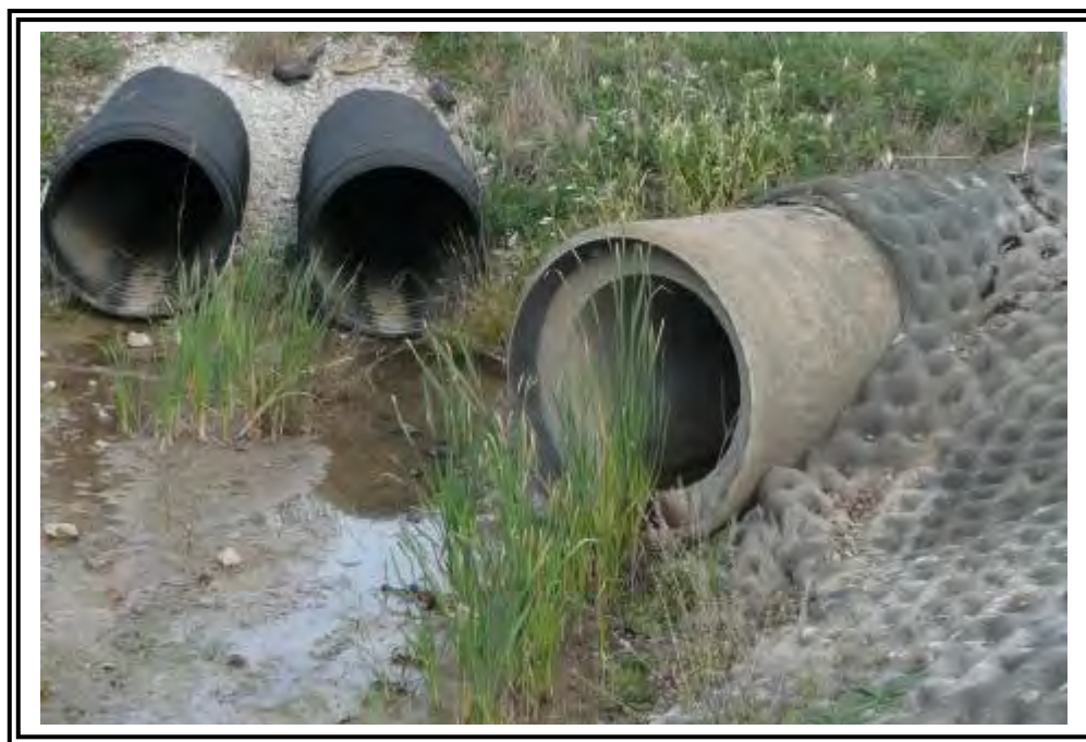
Concrete spillway outlet. Water does not normally flow through outlet. Water leaves outlet via a siphon with an outfall in the Ohio River.
