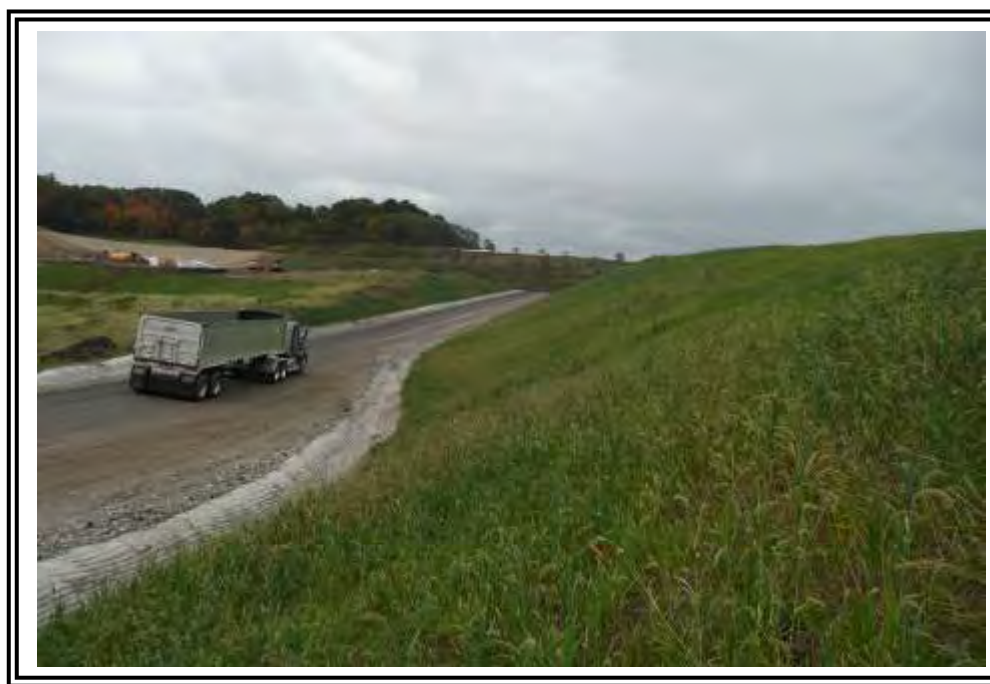
Looking southeast along the landfill buttress slope adjacent to active haul road. Slope is steeper adjacent to road.
