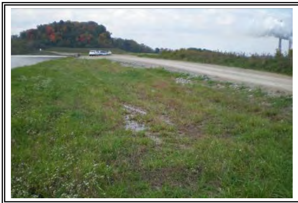
Downstream slope face, looking west, showing part of crest and access drive.
