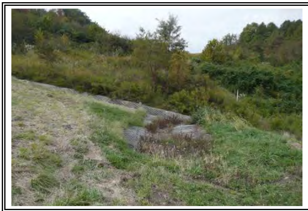
Fabric formed concrete lined tie-in from bench (Bench H) to left abutment groin. Note vegetation beginning to become established in sediment deposited in ditch over time.
