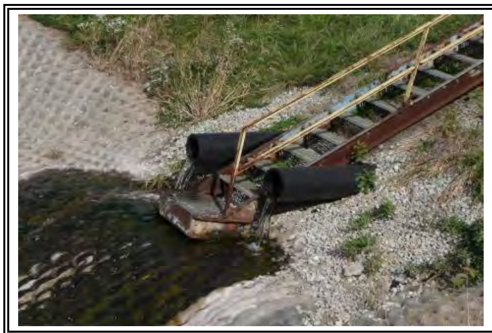
Blanket drain seepage collection system outlet. Approximately 36 gallons per minute. Seepage was clear.
