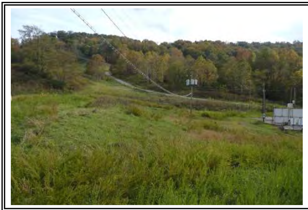
Downstream slope of Sedimentation Basin No. 2 showing pump house structure (right side of photo). Pump house conveys effluent from Sedimentation Basin No. 2 back up to the McElroy's Run Impoundment.
