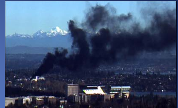
“UW Power plant malfunction sends black plume over Seattle” KOMO News, December 2 nd 2009
