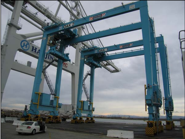
Figure 6. RTG cranes in front of an electric port crane.
